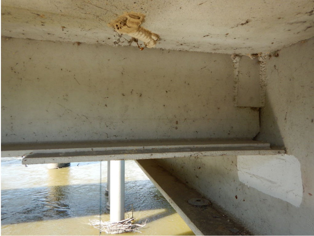
Photo 47: Stringer 1 connection to Floor Beam 2, Span 2
