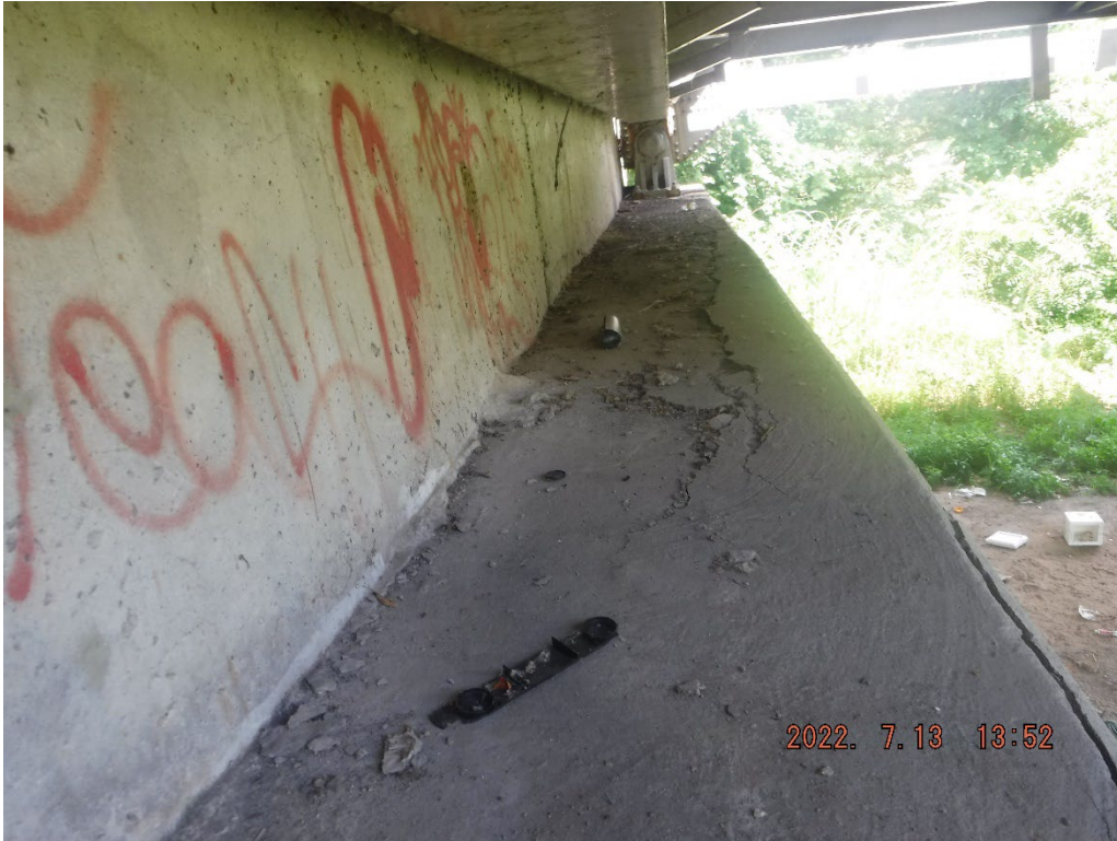
Photo 74: Rear Abutment seat looking North
