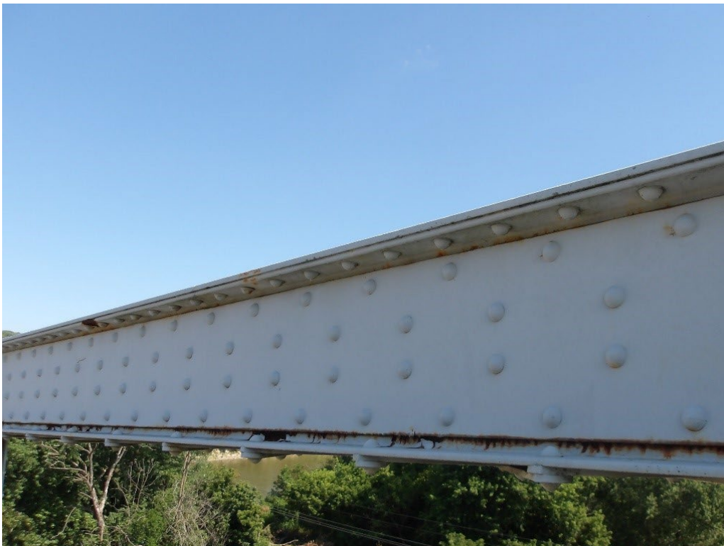
Photo 27: Corrosion on upper chord channel and web plate, U3U4, Span 3, North Truss
