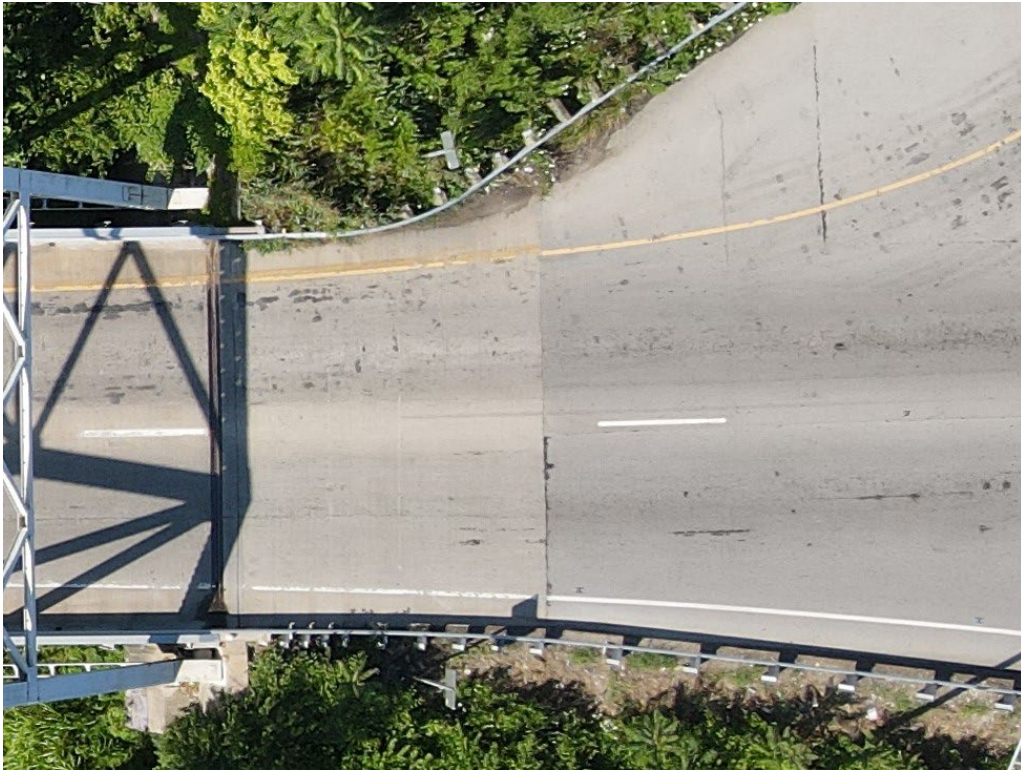
Photo 83: Forward approach wearing surface
