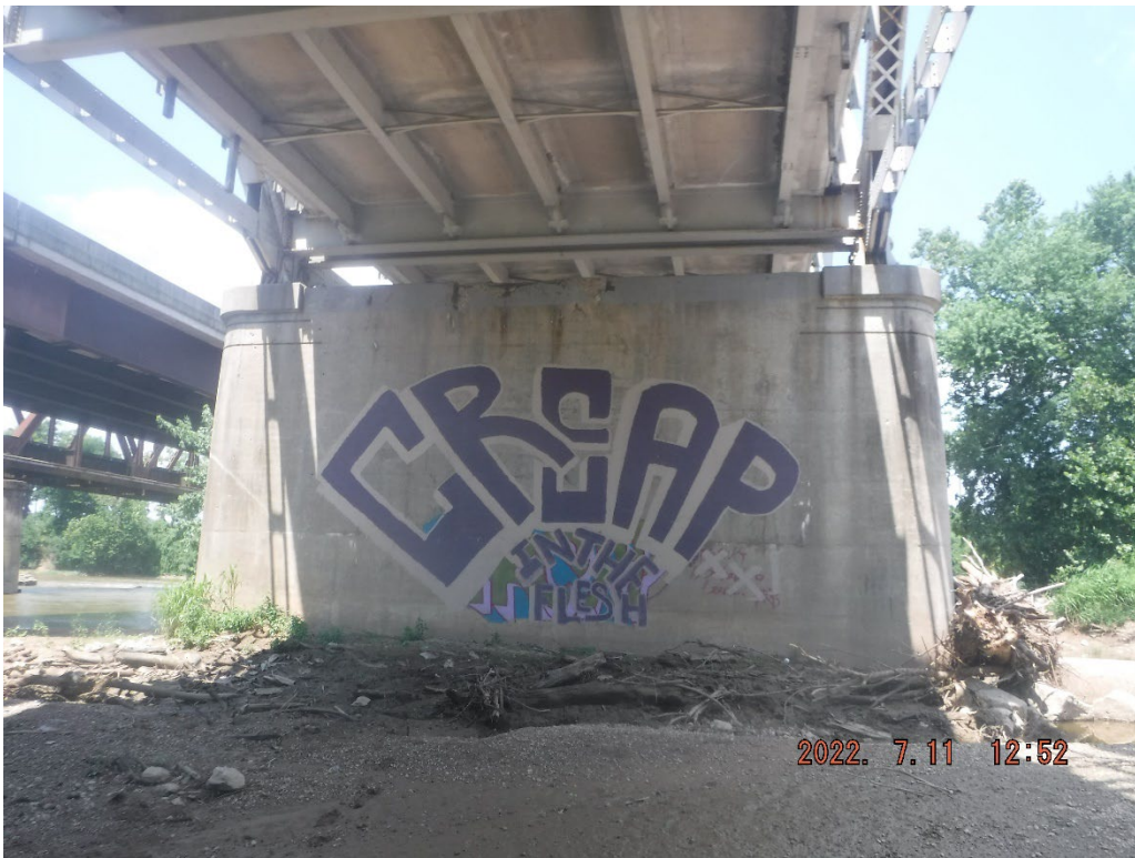
Photo 70: West face of Pier 3
