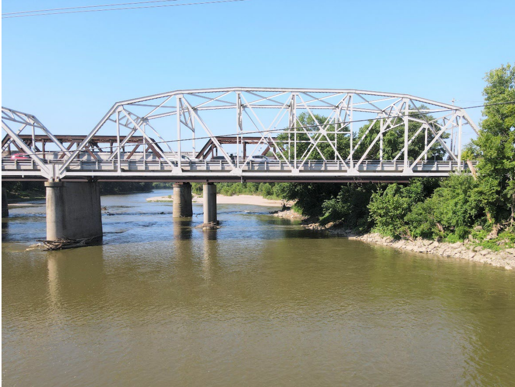
Photo 85: Channel under Span 1
