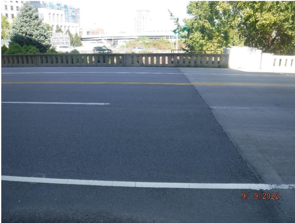
Photo 99: West approach pavement and transition
