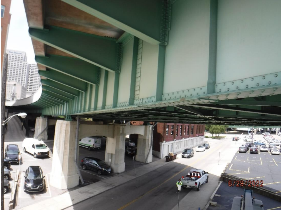
Photo 75: Typical paint condition on girder spans (Span 4 shown)
