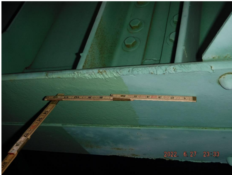
Photo 18: Example of girder scrape (Center Girder, Span 14 shown)
