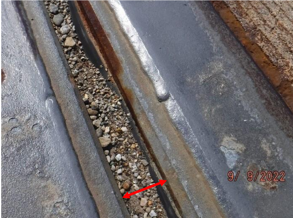
Photo 9: Typical expansion joint measurement location
