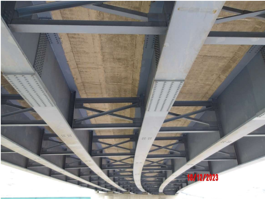
Photo 11- Span 23, Typical Underside
