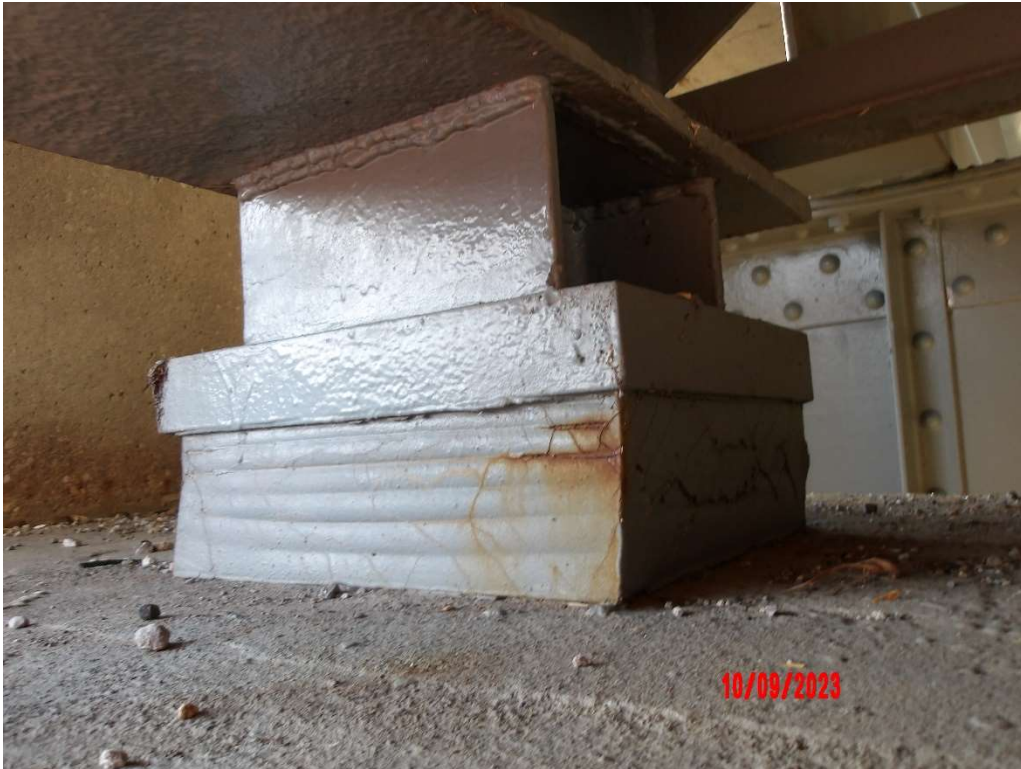
Photo 48- Pier 0, Bearing G
