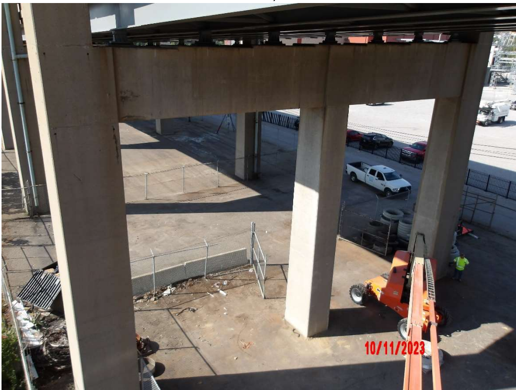
Photo 75- Pier 7, Front Face
