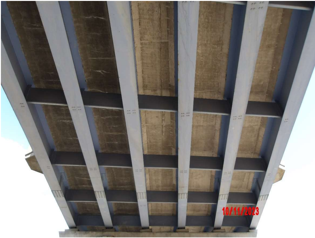
Photo 9- Span 21, Typical Underside, Typical
