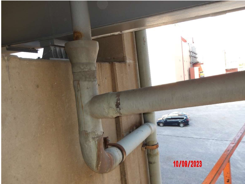
Photo 22- Drainage, Span 1, Pier 2
