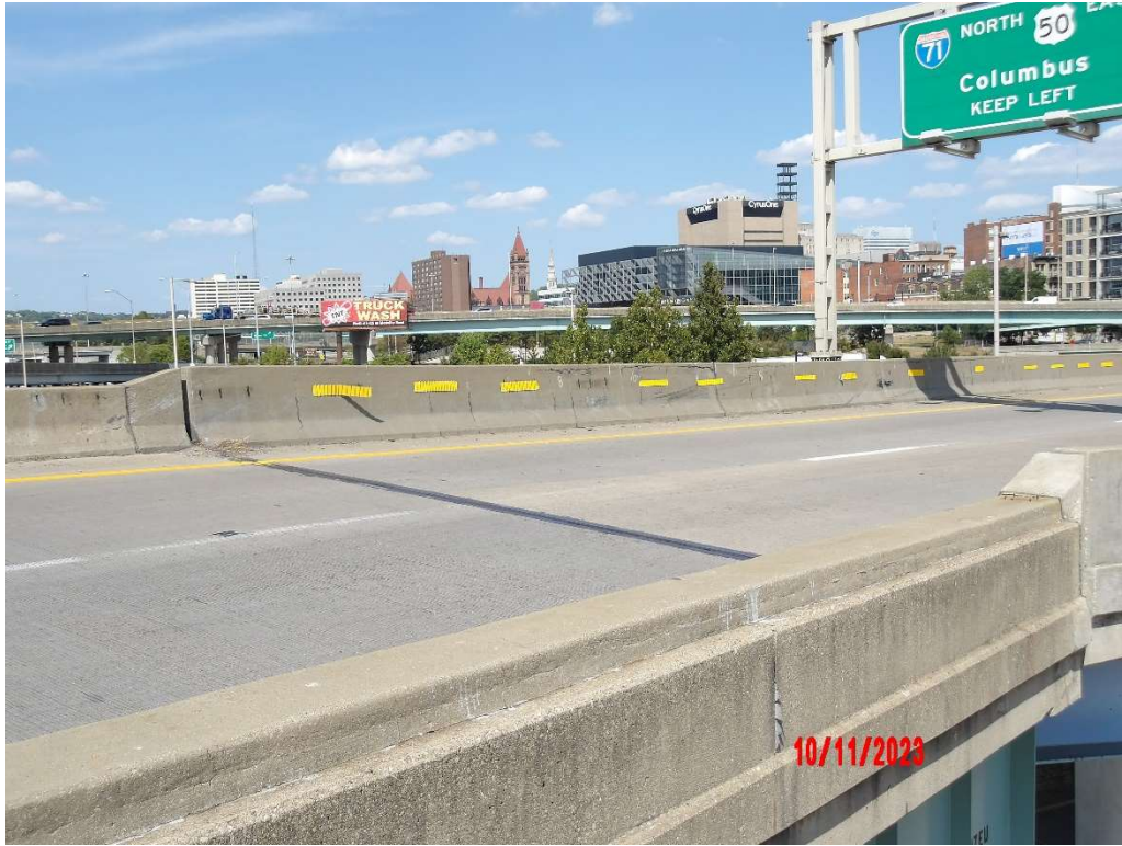
Photo 15- Typical Wearing Surface
