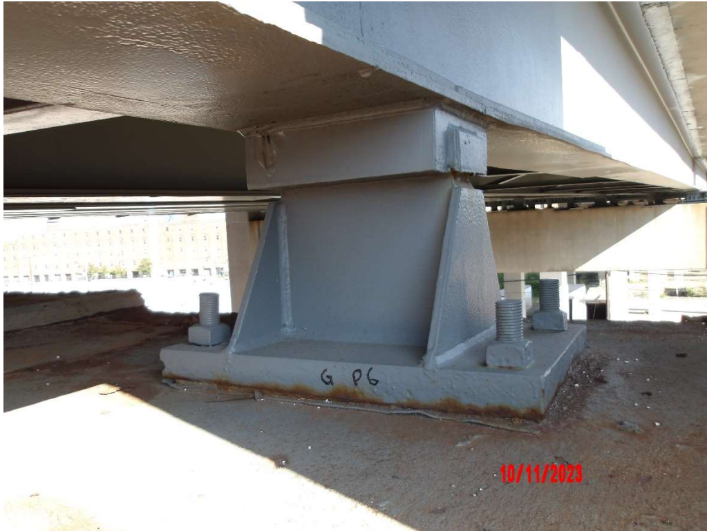
Photo 57- Pier 6 Bearing G
