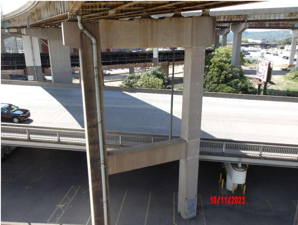
Photo 78- Pier 19D, Front Face
