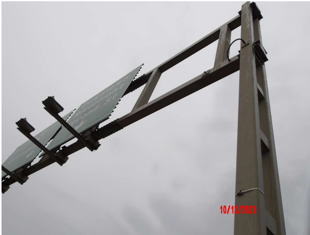
Photo 97- Sign Supports, Typical Good Condition
