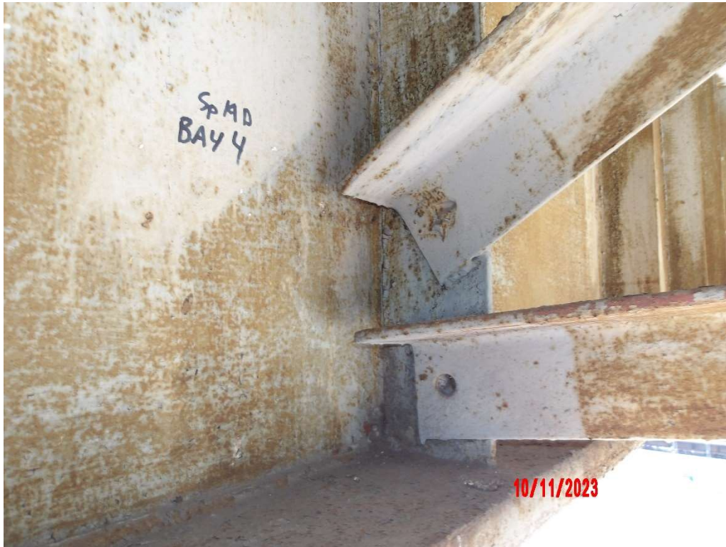
Photo 69- Cross Frame Details, Span 19, Bay 4
