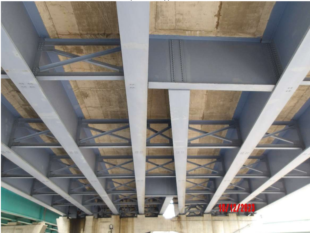
Photo 14- Typical Underside, Span 25
