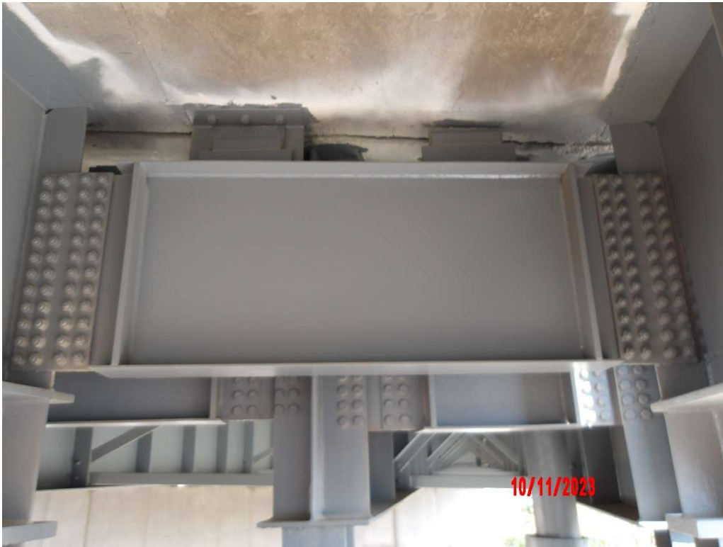
Photo 63- Cross Frame Detail, Span 12 Pier 12
