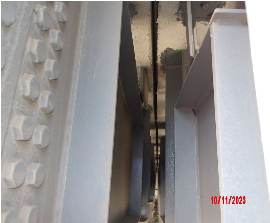
Photo 17- Pier 12 Joint, Typical
