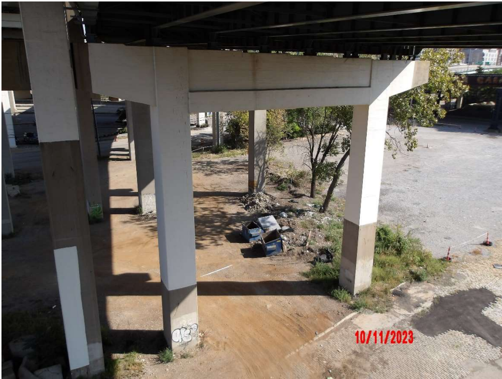
Photo 76- Pier 12, Back Face
