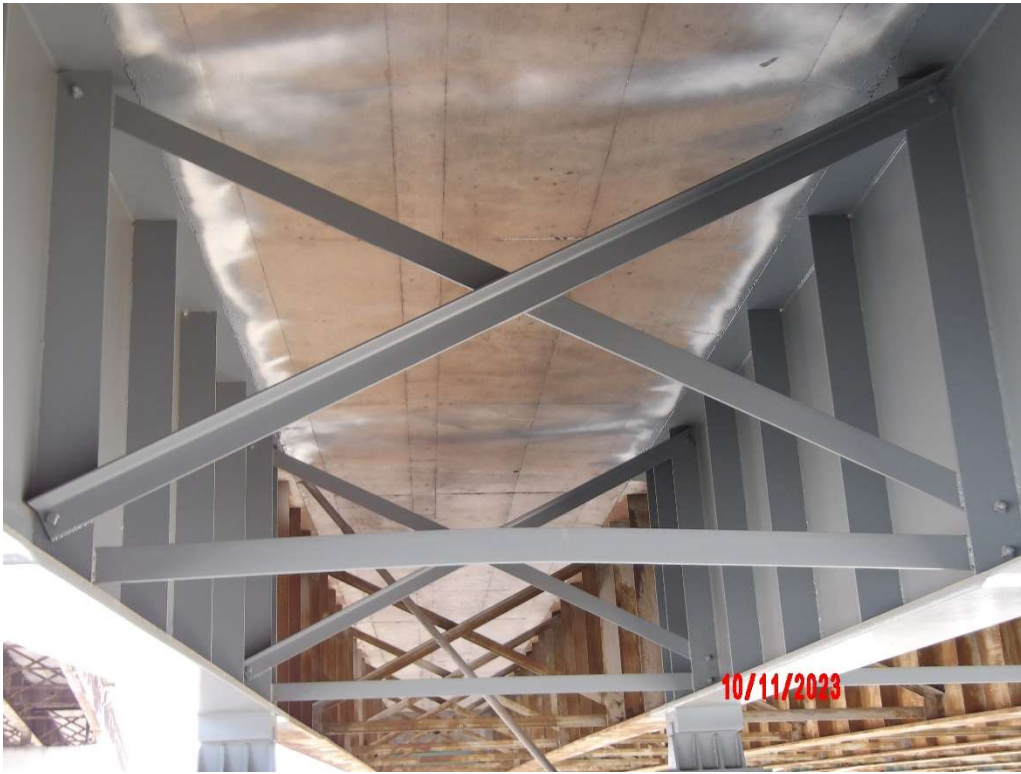
Photo 67- Cross Frame #5, Span 14, Bent
