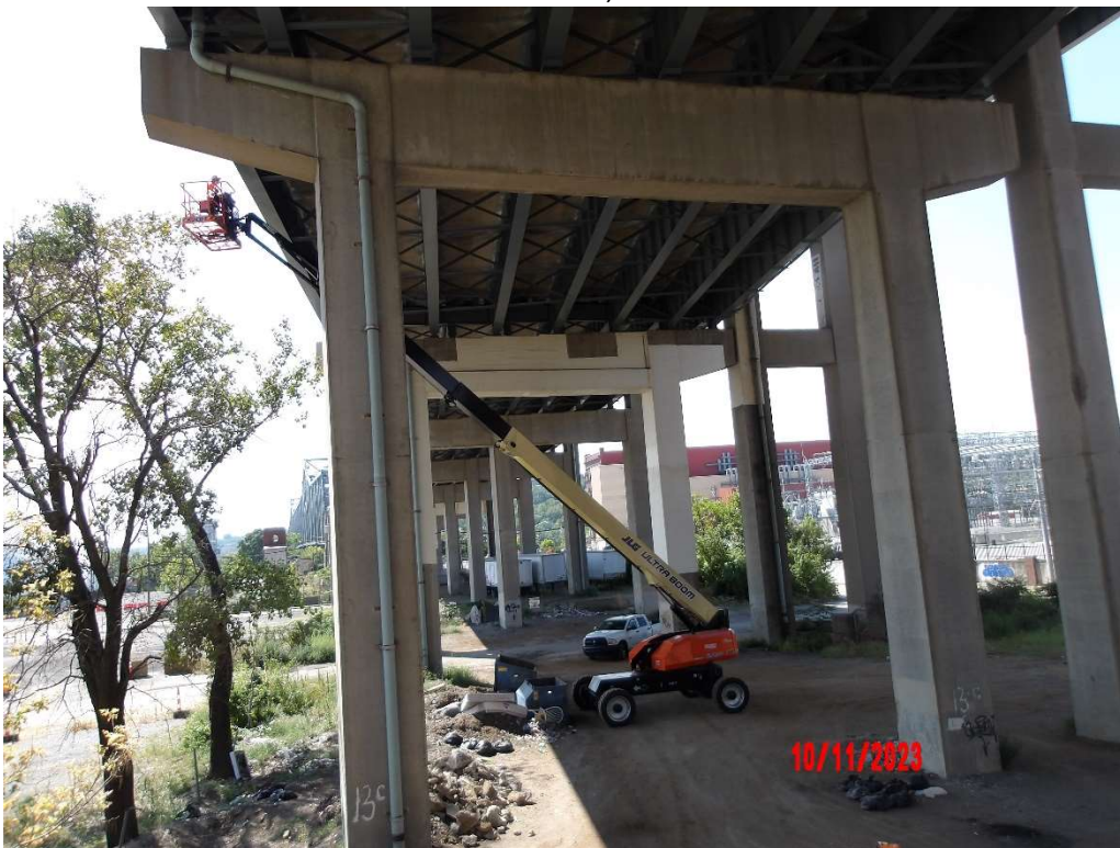
Photo 77- Pier 13, Front Face
