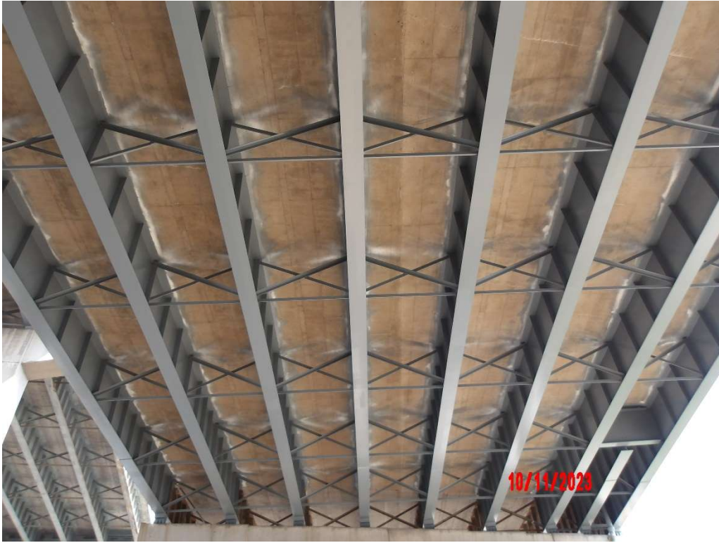
Photo 5- Span 14, Typical Underside
