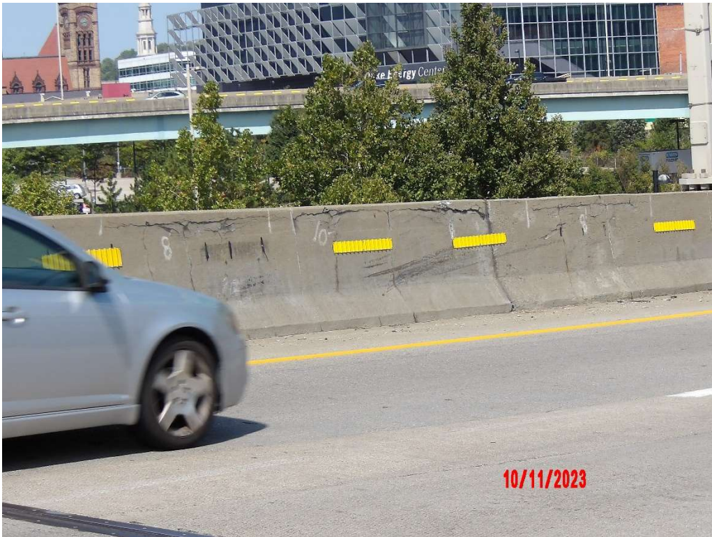
Photo 19- Barrier, Typical Conditions
