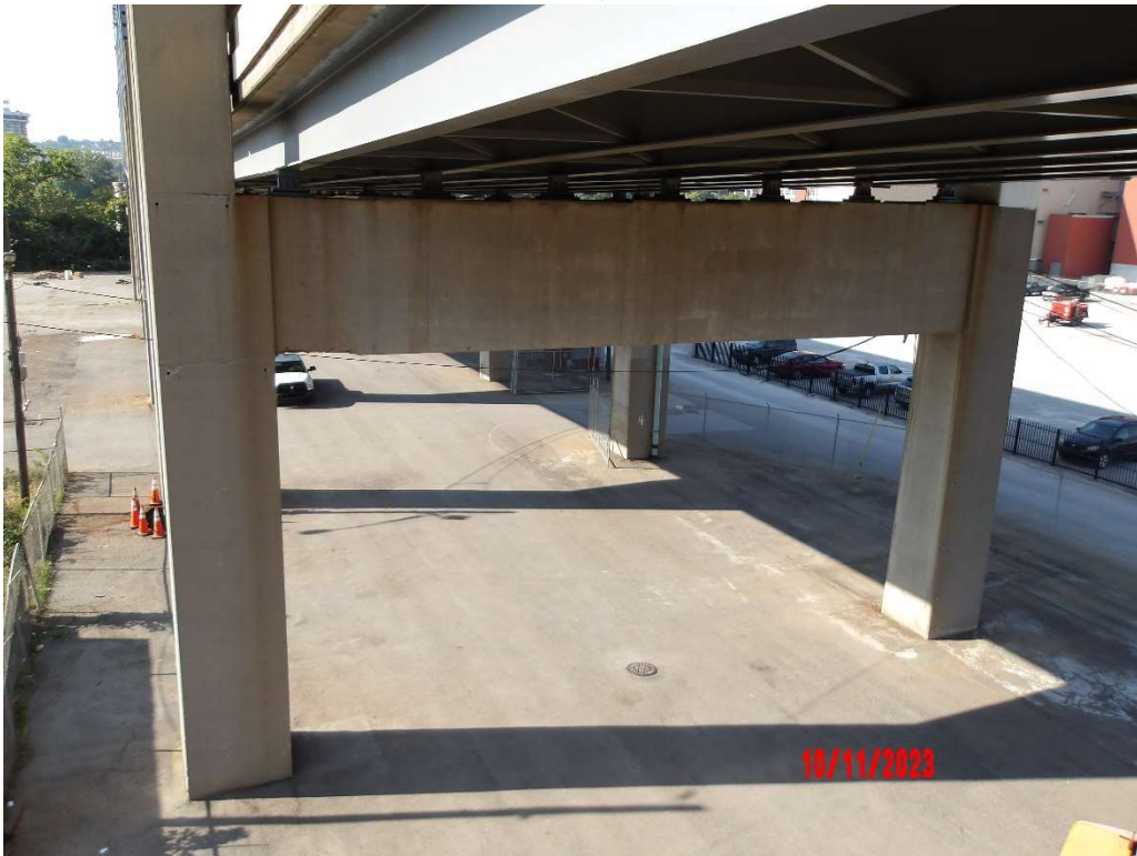
Photo 73- Pier 5 Front Face
