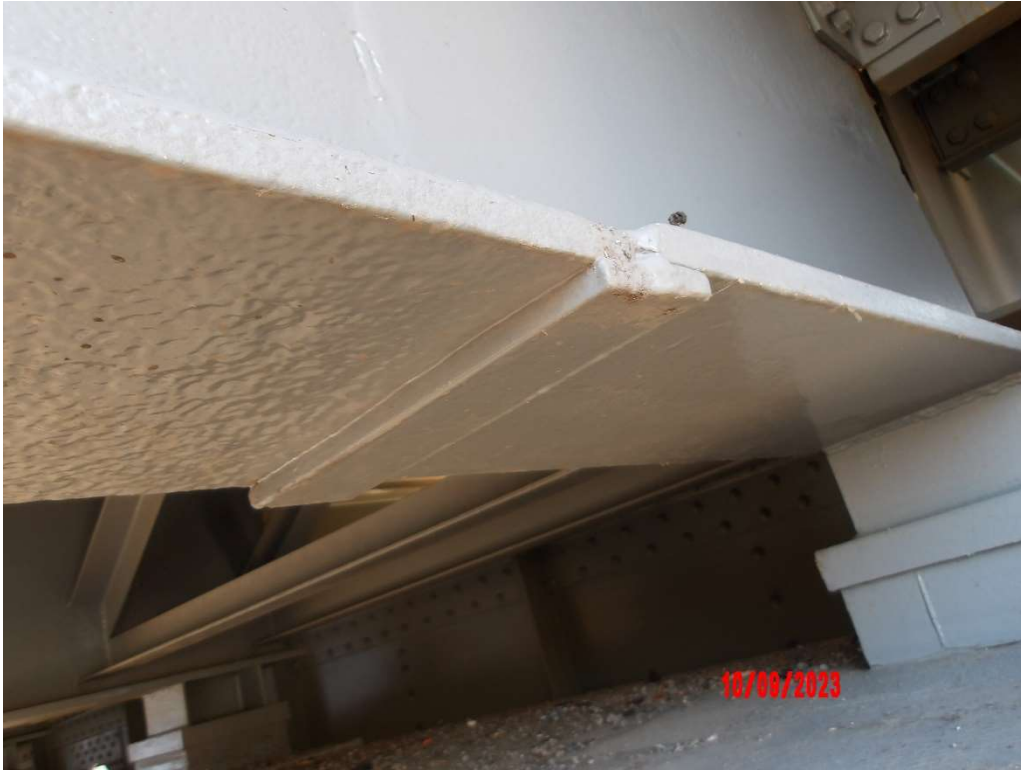
Photo 28- Girder A, Span 1, Backing Plate on Bottom Flange
