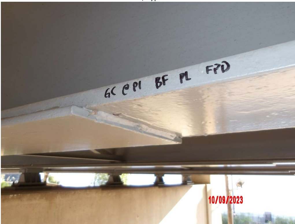
Photo 33- Girder C, Span 2, Bottom Flange Plate with End Weld
