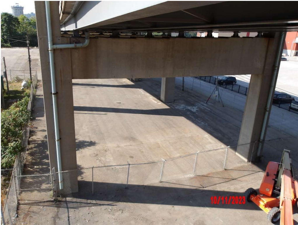
Photo 74- Pier 6, Front Face
