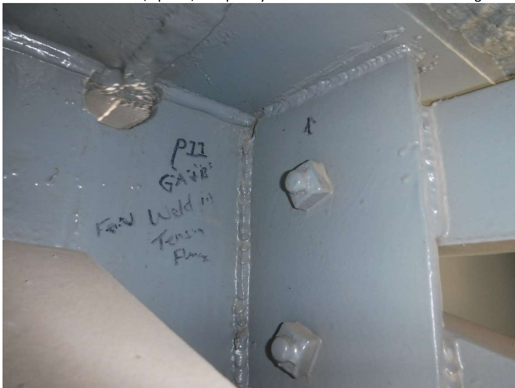
Photo 39- Girder A, Pier 11, Field Welds in Tension Flange
