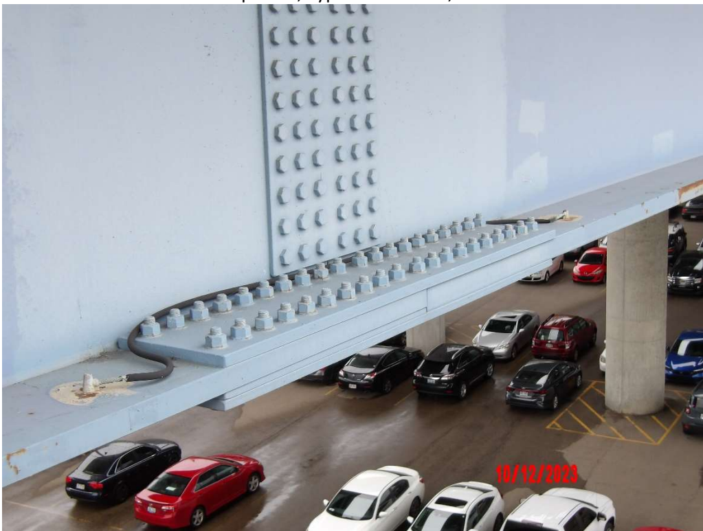
Photo 47- Grounding Wire Detail, Span 24 Fascia at Splice Plate
