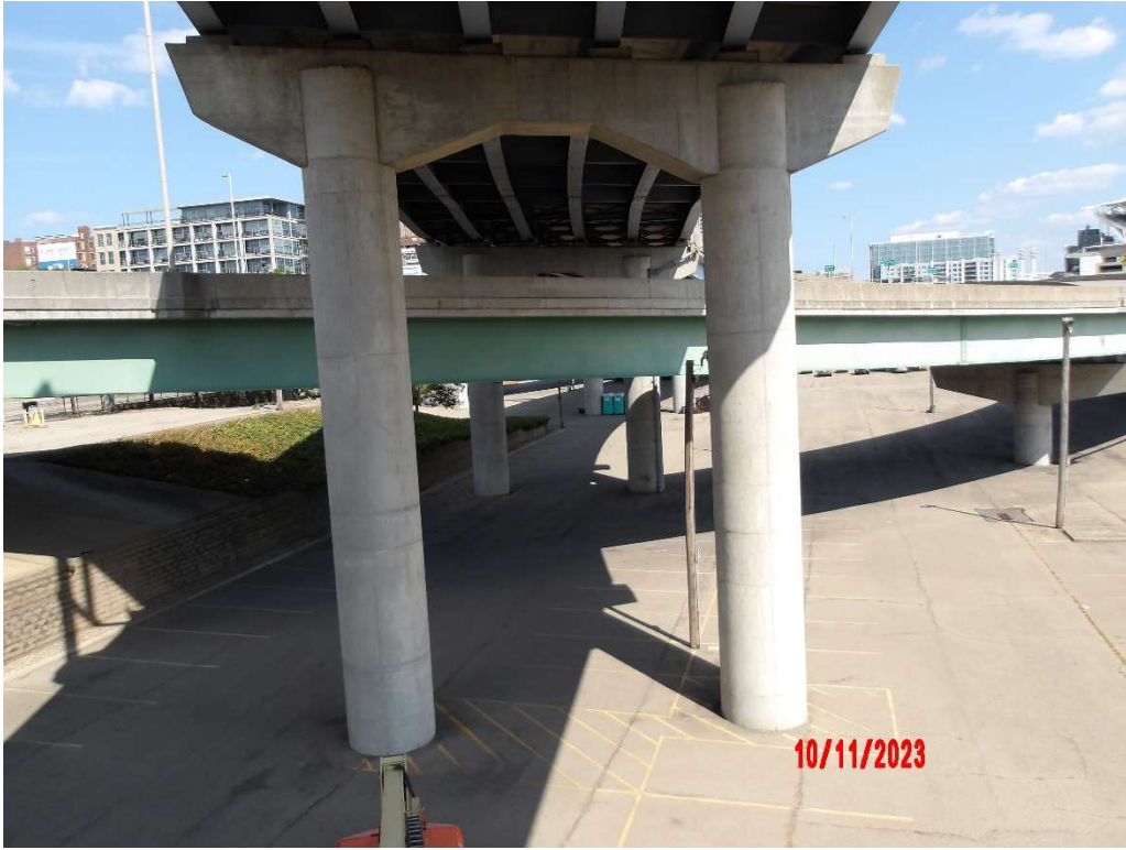
Photo 83- Pier 21D Back Face
