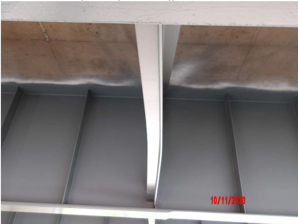
Photo 66- Cross Frame #5, Span 14, Bent
