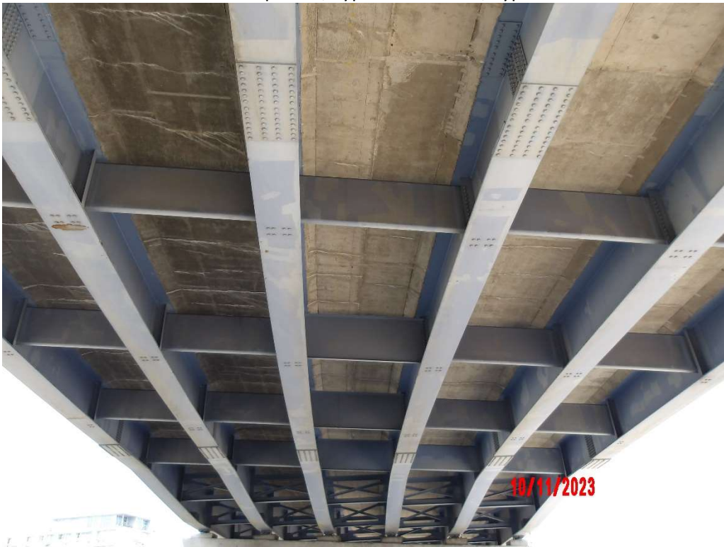
Photo 10- Span 22, Typical Underside
