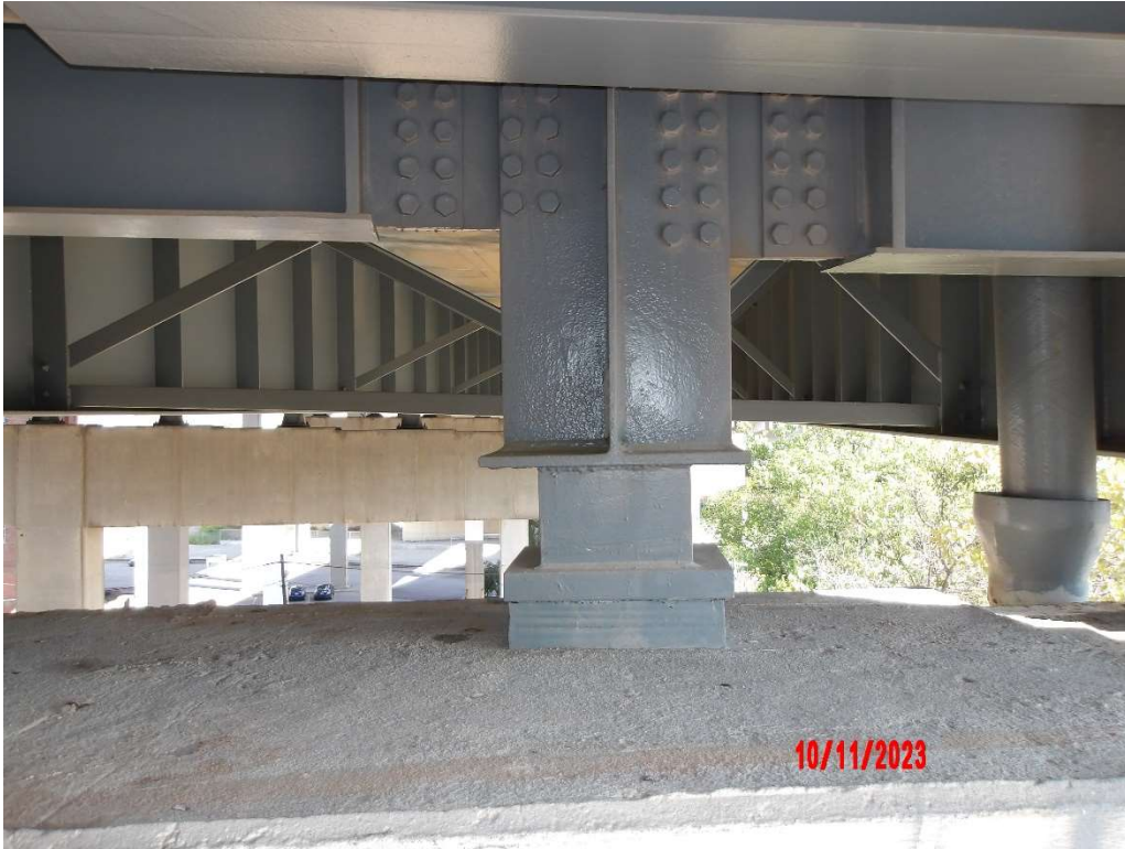
Photo 50- Pier 12 Bearing G, Span 13
