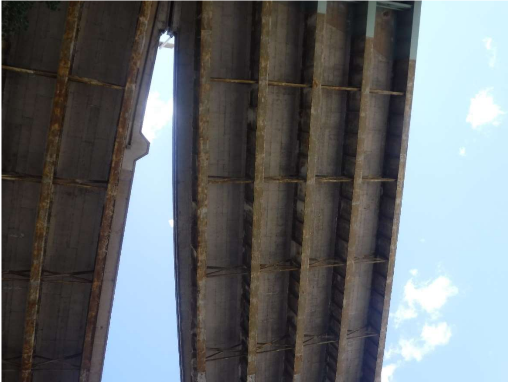
Photo 7- Typical Underside, Span 16
