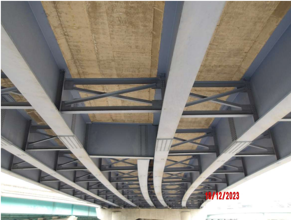
Photo 13- Span 24, Typical Underside
