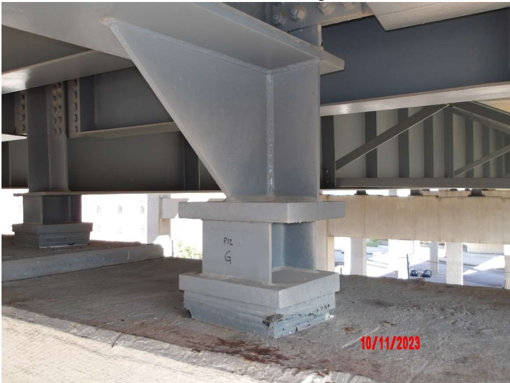
Photo 49- Pier 12 Bearing G, Span 12
