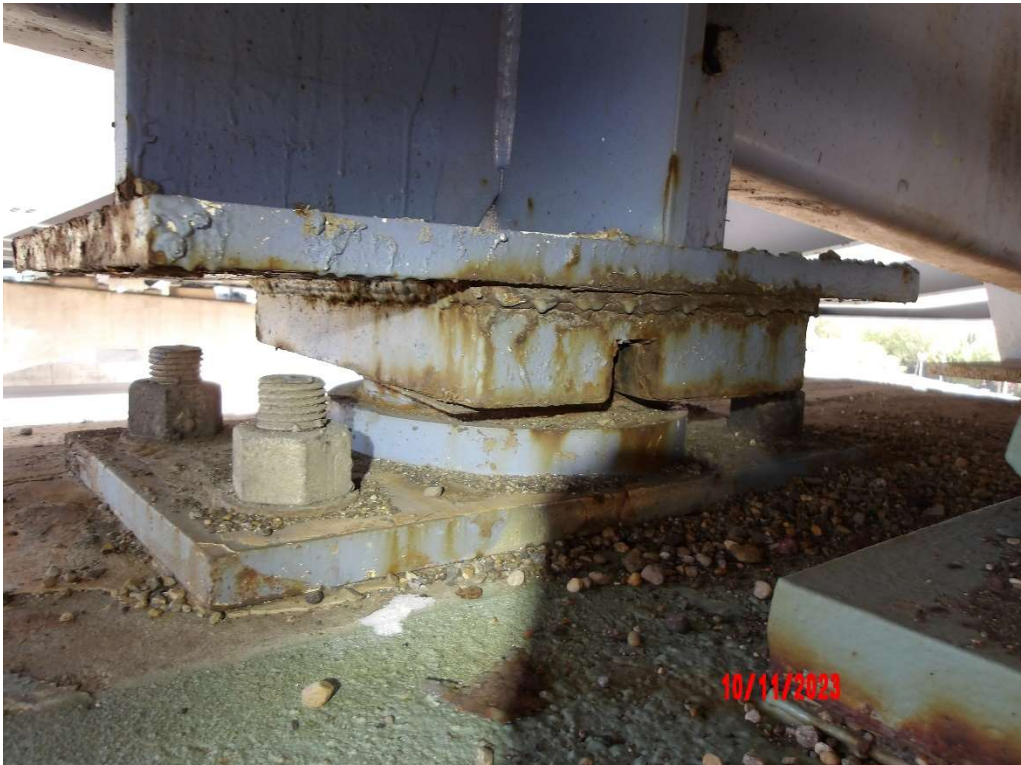
Photo 59- Pier 20D, Bearing B, Span 21, Typical Condition
