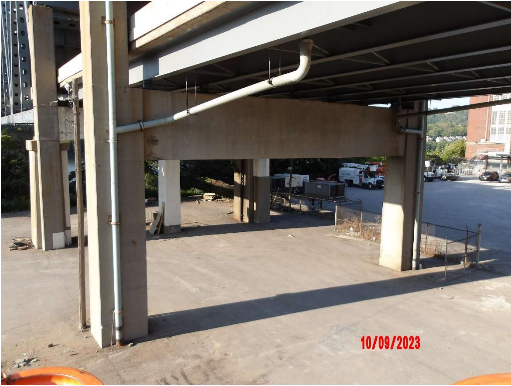
Photo 72- Pier 2, Front Face
