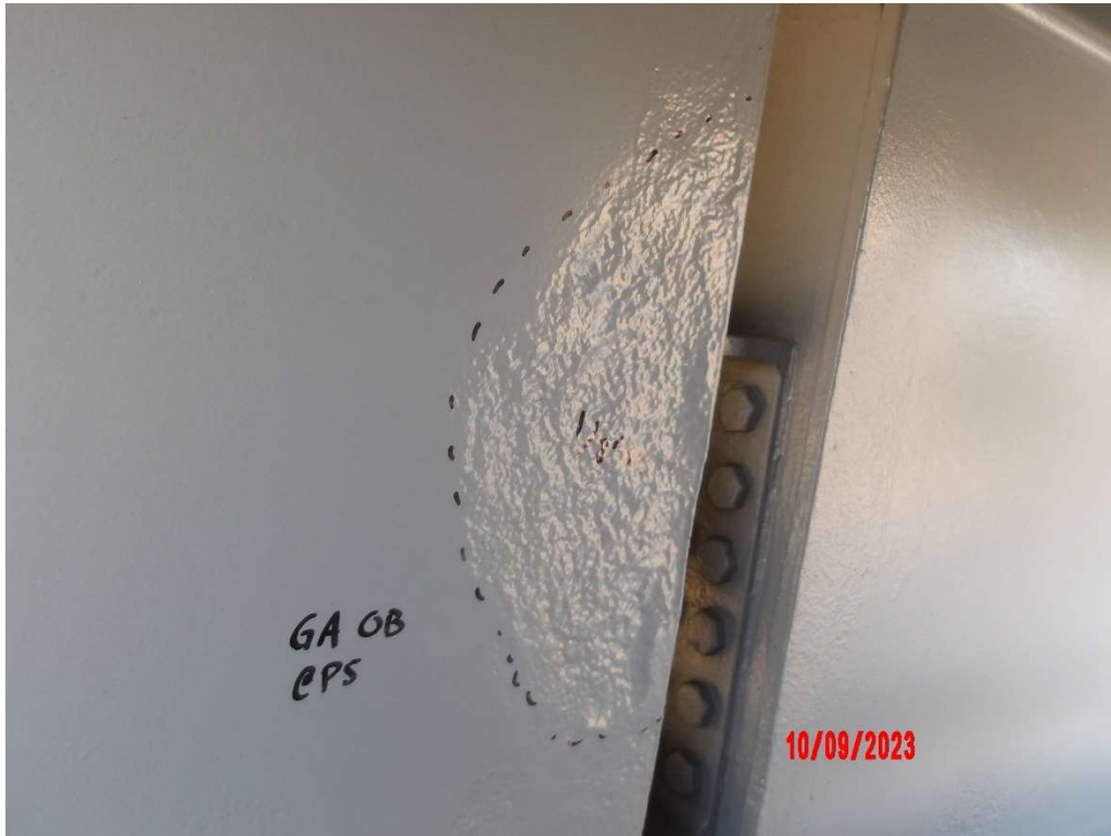
Photo 36- Girder A, Web at Pier 5, Section Loss 1/8" Web
