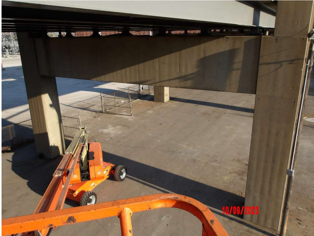
Photo 71- Pier 1, Back Face
