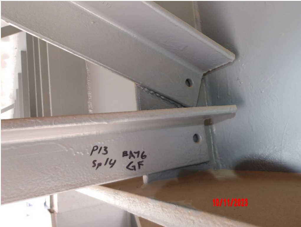
Photo 65- Pier 13, Span 14, Bay 6, Girder F, Typical Welded Cross Frame Details
