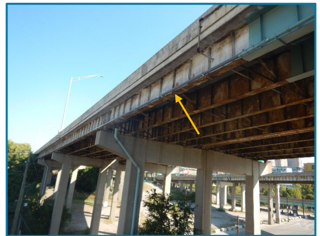
Photo 31 – Conduit along the exterior bottom flange of Girder A (looking northeast).
