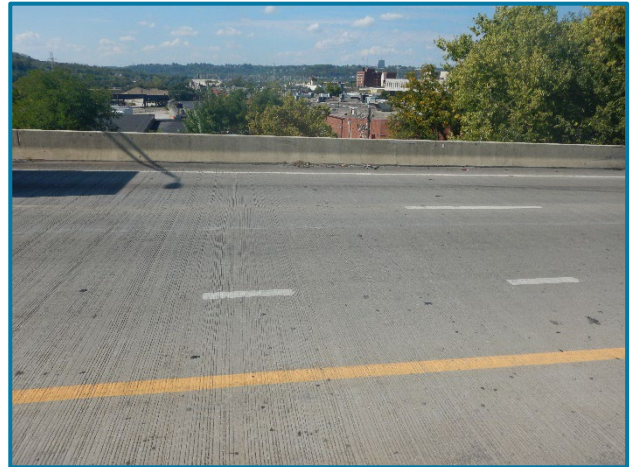
Photo 6 – Typical wearing surface (looking west in Span 24A at midspan).
