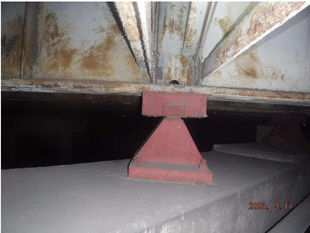
Photo 35- Pier 29, Bearing C, Typical
