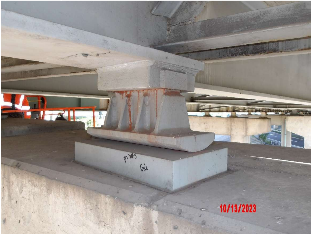
Photo 30- Bearing G, Pier 23J
