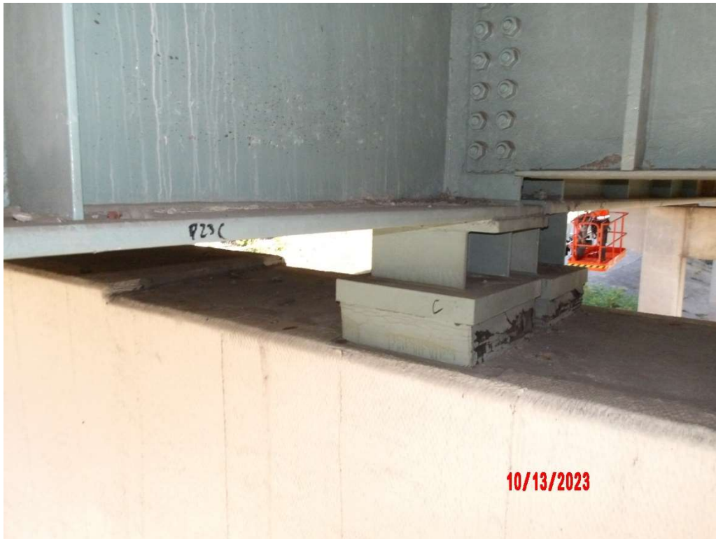
Photo 28- Bearing C, Pier 23J
