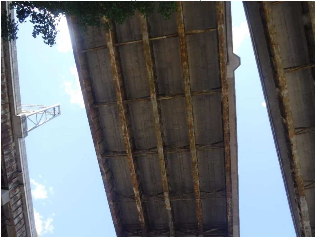
Photo 3- Typical Underside, Span 16
