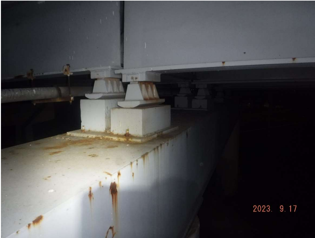
Photo 32- Pier 25J, Bearings Typical
