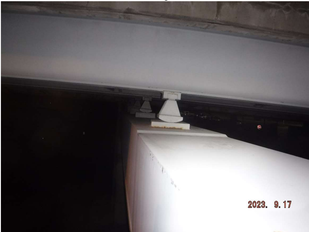
Photo 31- Pier 25C, Bearings Typical
