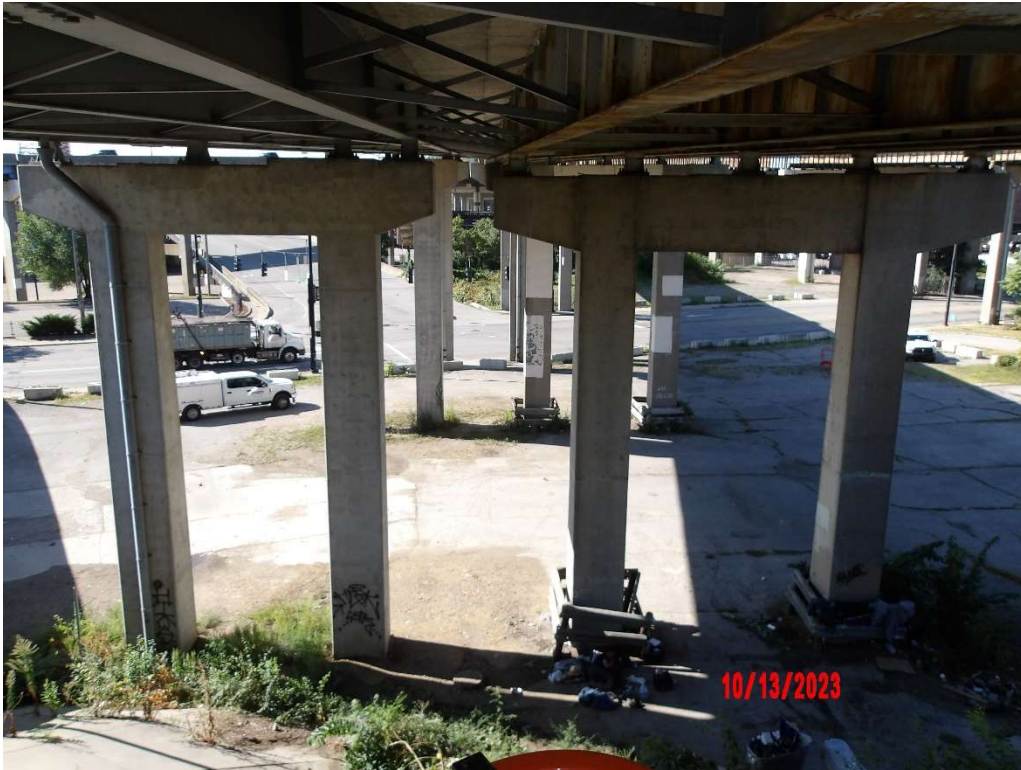
Photo 44- Pier 24J, Front Face
