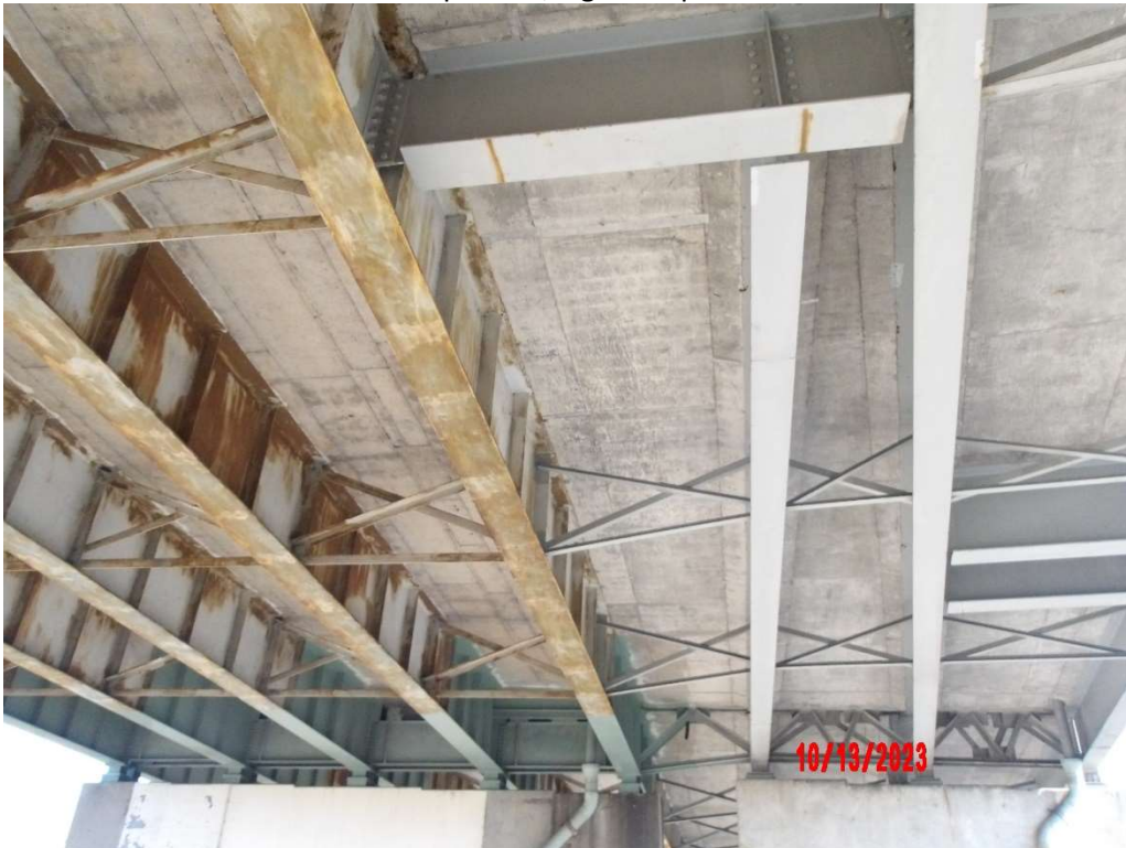
Photo 7- Span 23J, Typical Underside
