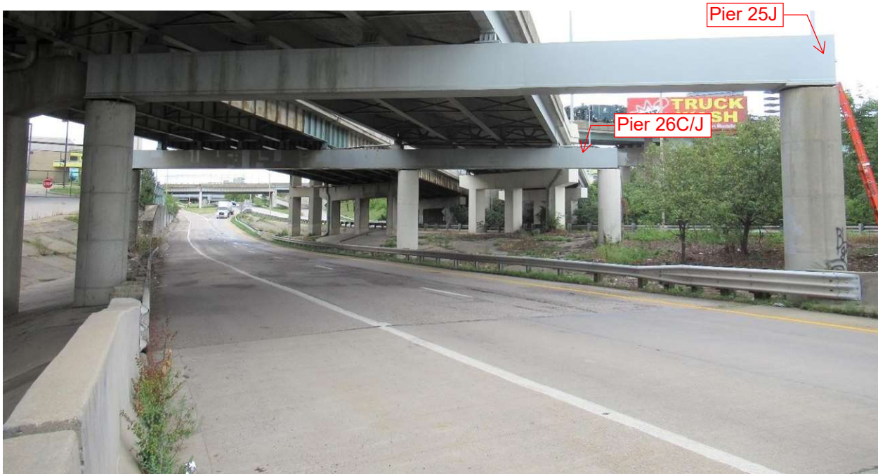
Photo 50- Fracture critical steel box pier cap members looking north
