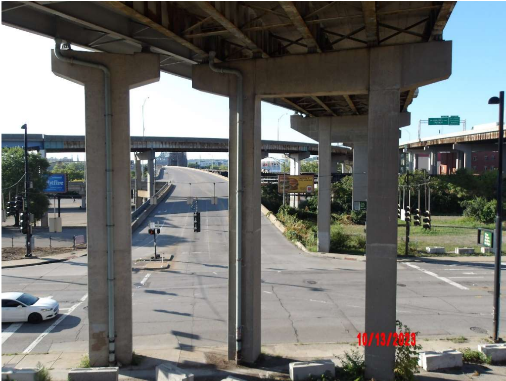
Photo 42- Pier 22C, Front Face
