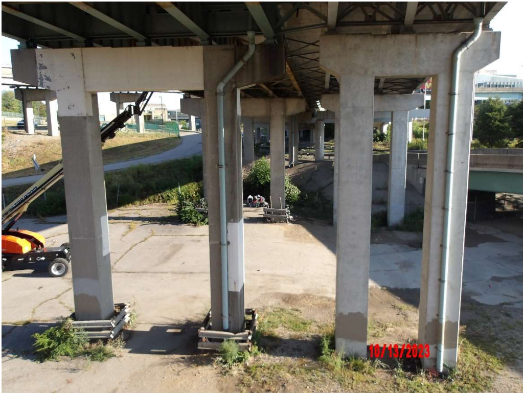
Photo 43- Pier 23, Back Face
