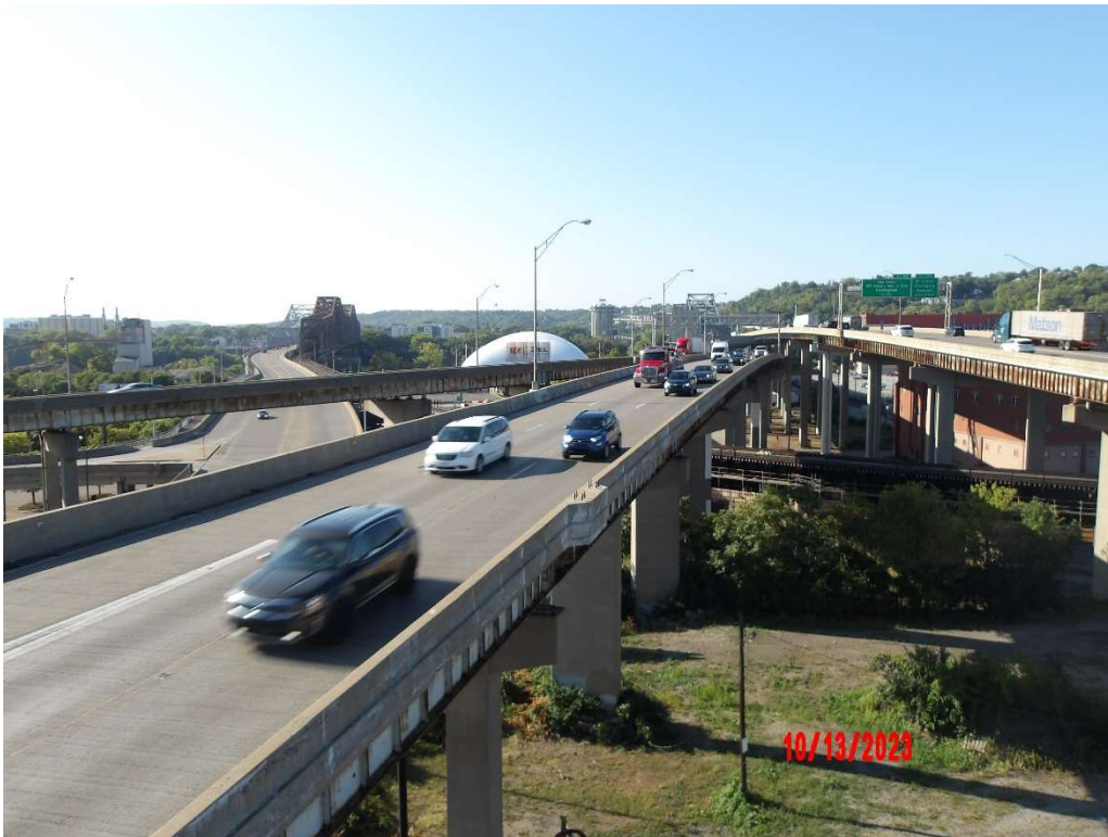
Photo 1- Bridge Deck, Typical Condition
