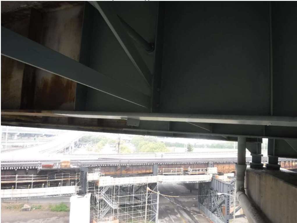
Photo 20- Girder G, Span 16, Typical Weld Remnants on Girders
