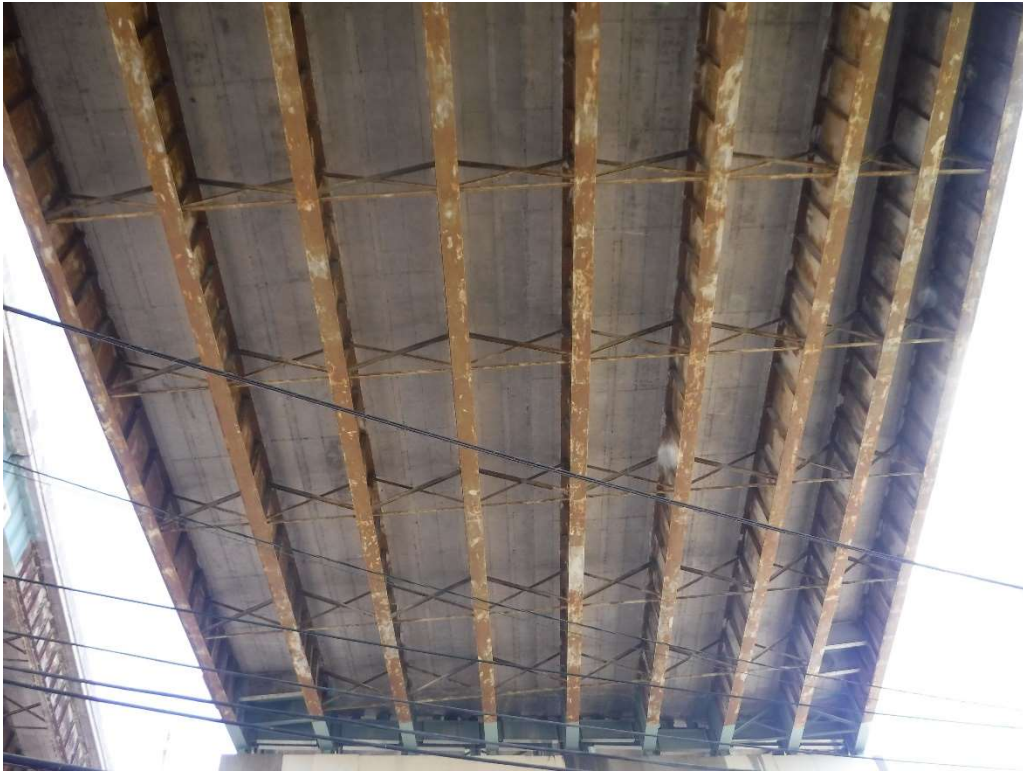
Photo 2- Typical Underside, Span 15
