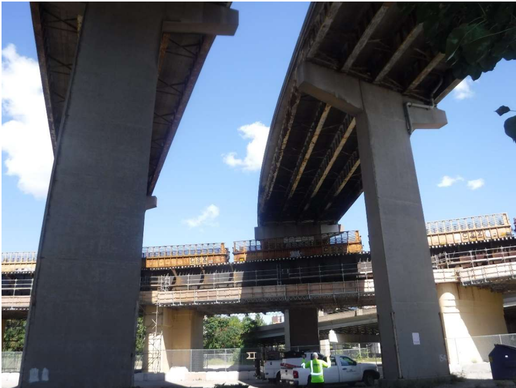
Photo 41- Pier 16 Back Face
