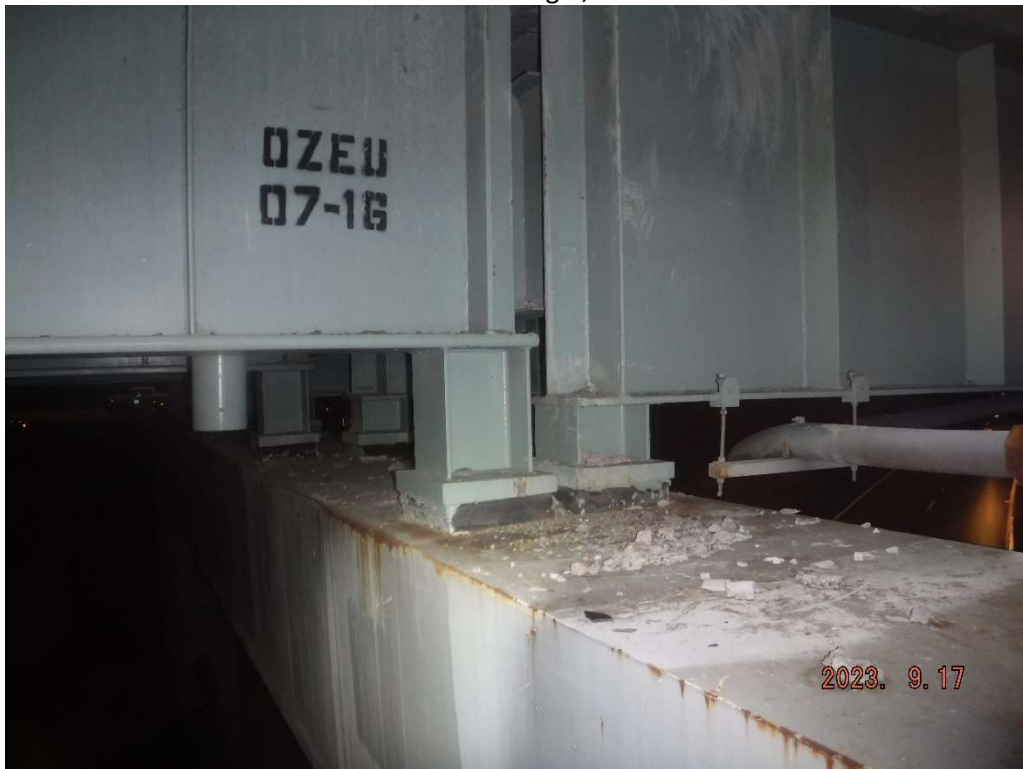
Photo 29- Pier 25C, Bearings Typical
