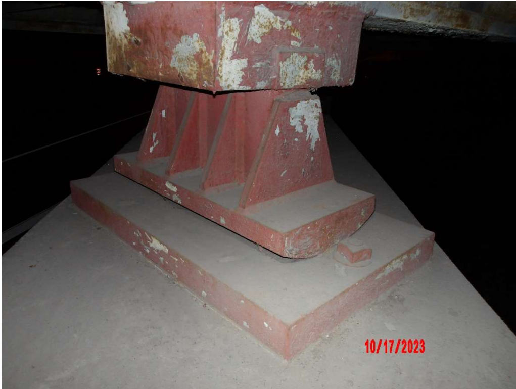
Photo 34- Pier 28, Bearing A, Typical
