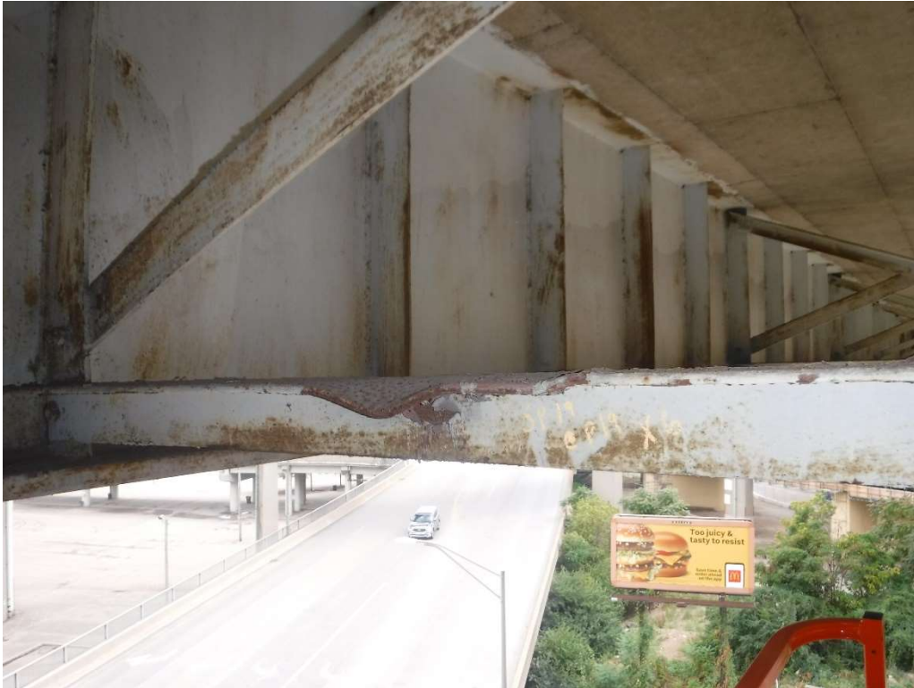
Photo 36- Cross Frame #6, Span 19, Bent
