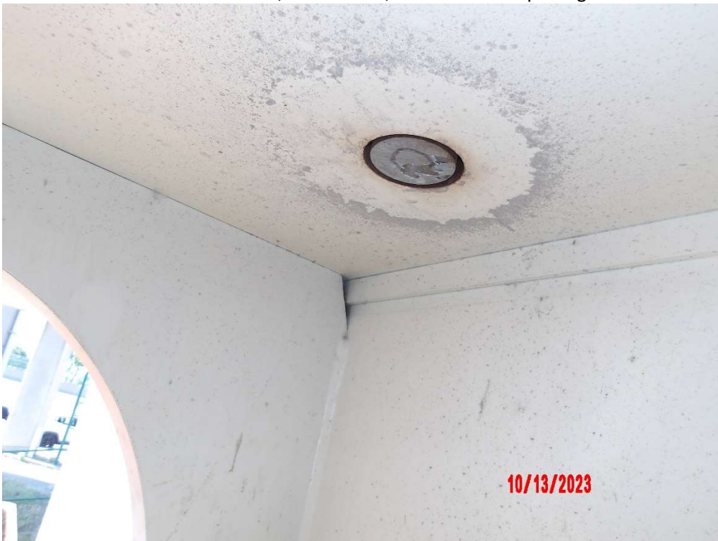
Photo 64- Pier 26J, West End, Drill Holes in Top Flange
