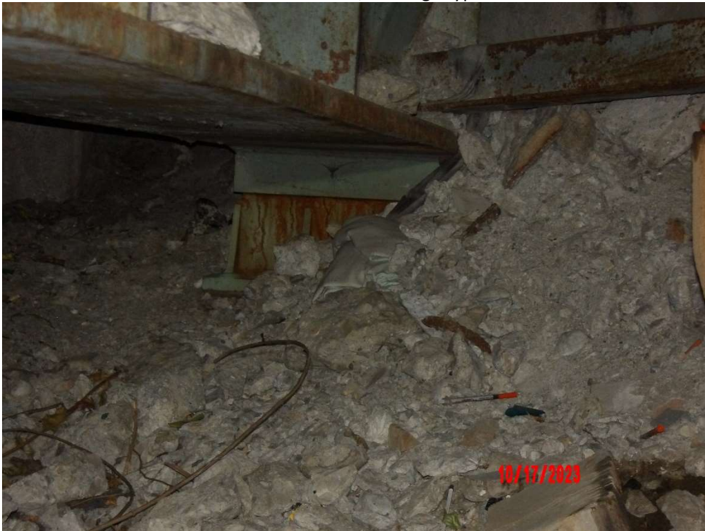
Photo 33- Abutment C, Bearing A, Covered in fill
