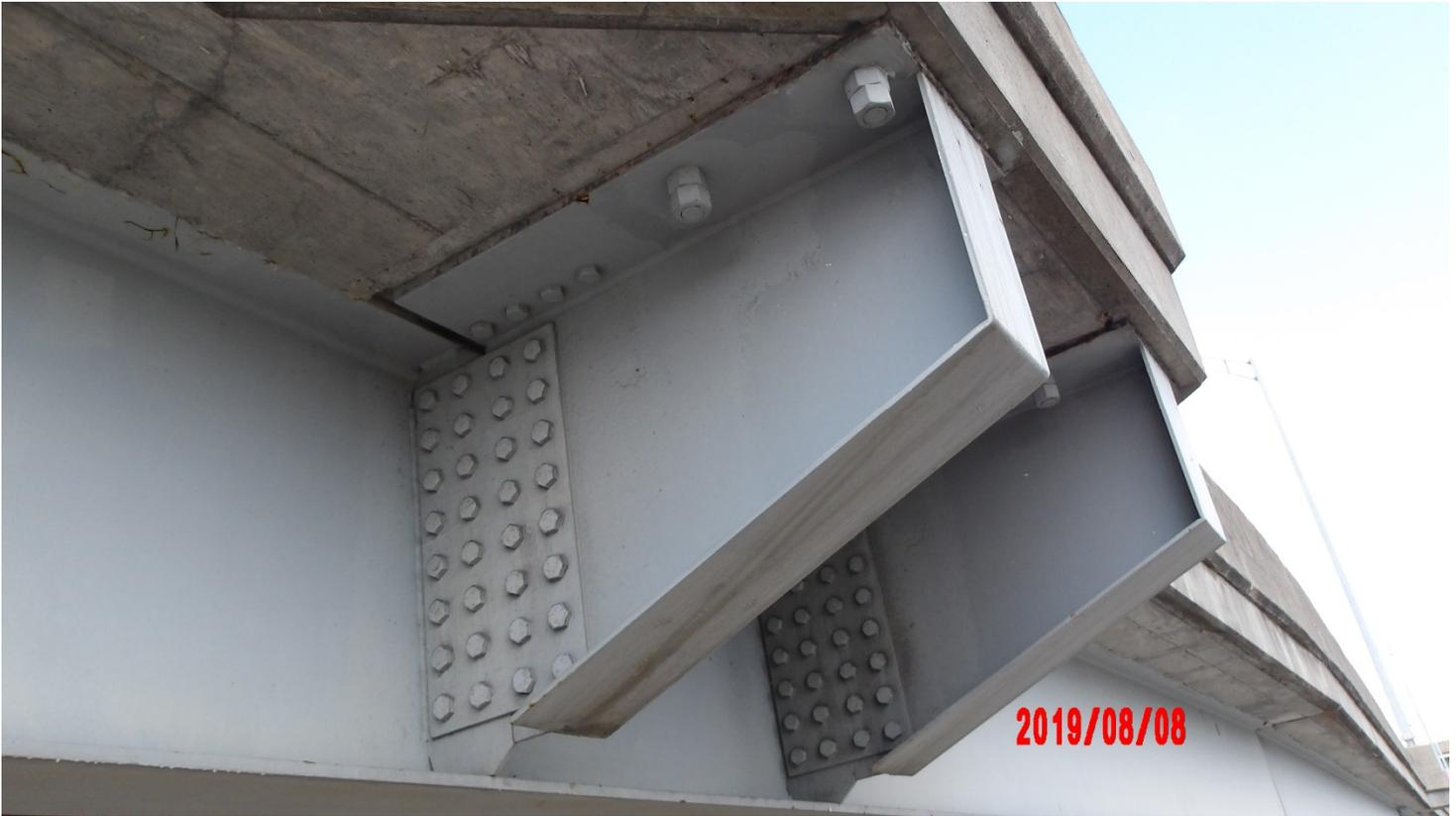
PHOTO 45. SIGNS, BUMPOUT OVERHANG FOR SIGN MOUNTS
