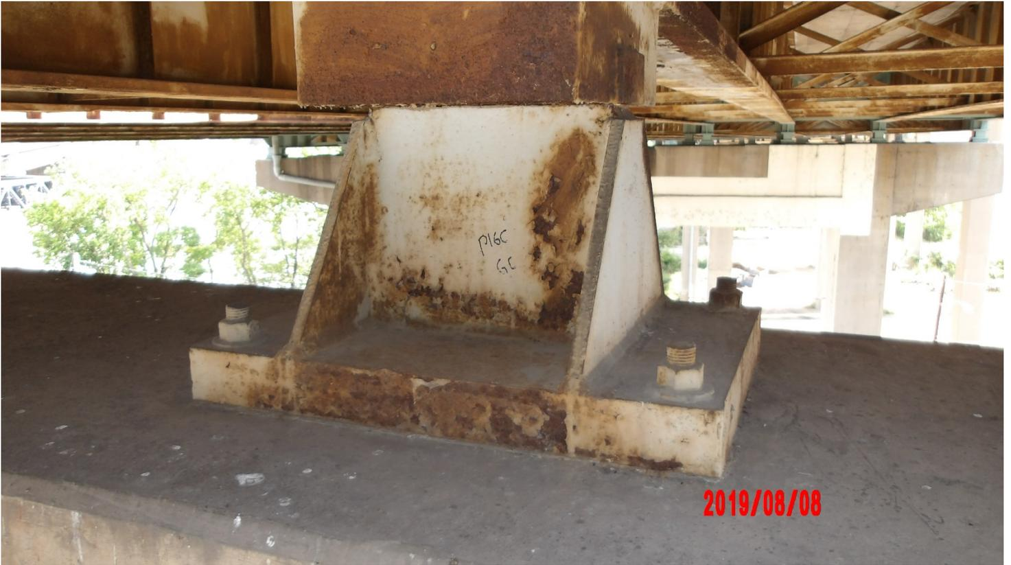
PHOTO 24. FIXED BEARING C PIER 16C
