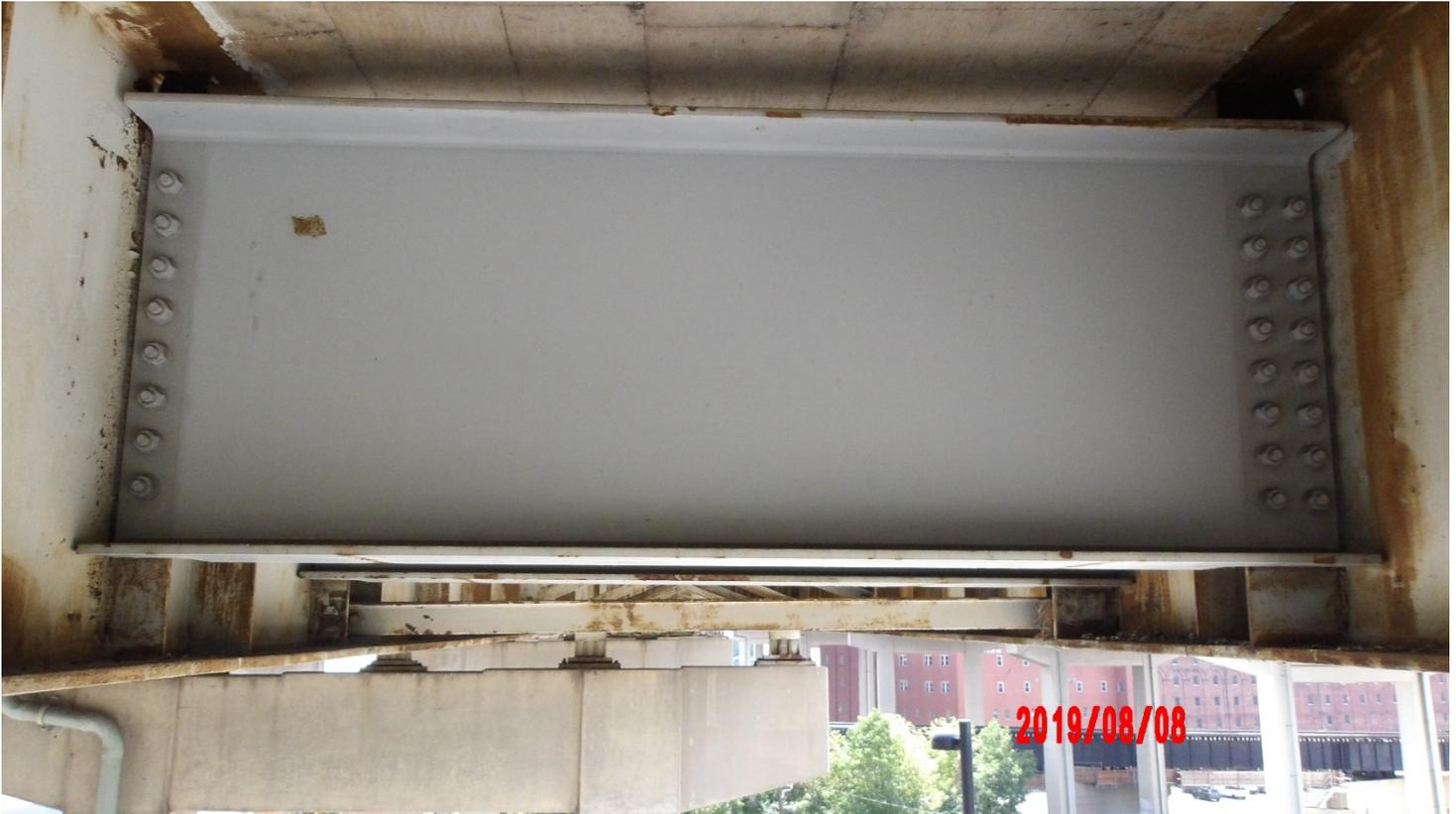
PHOTO 27. DIAPHRAGM, RETROFIT DIAPHRAGM SPAN 24
