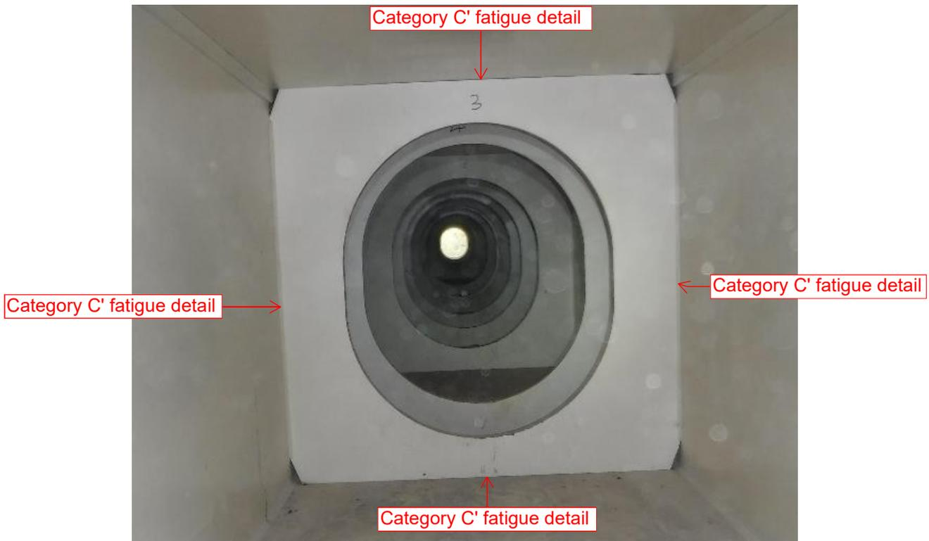
Photo 2 - Category C' fatigue detail- Diaphragm fillet welds to webs and flanges
