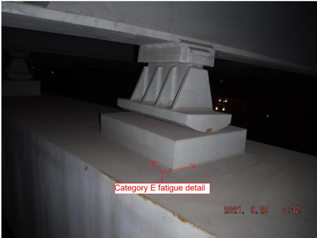
Photo 1 - Category E fatigue detail - Steel bearing pedestal welded to top flange
