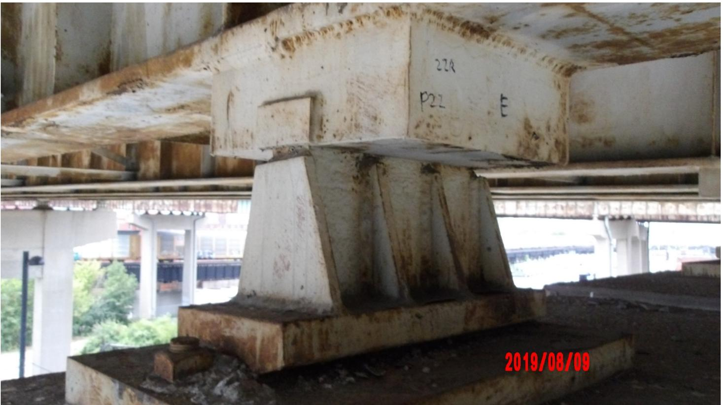
PHOTO 20. MOVABLE BEARING E PIER 22C
