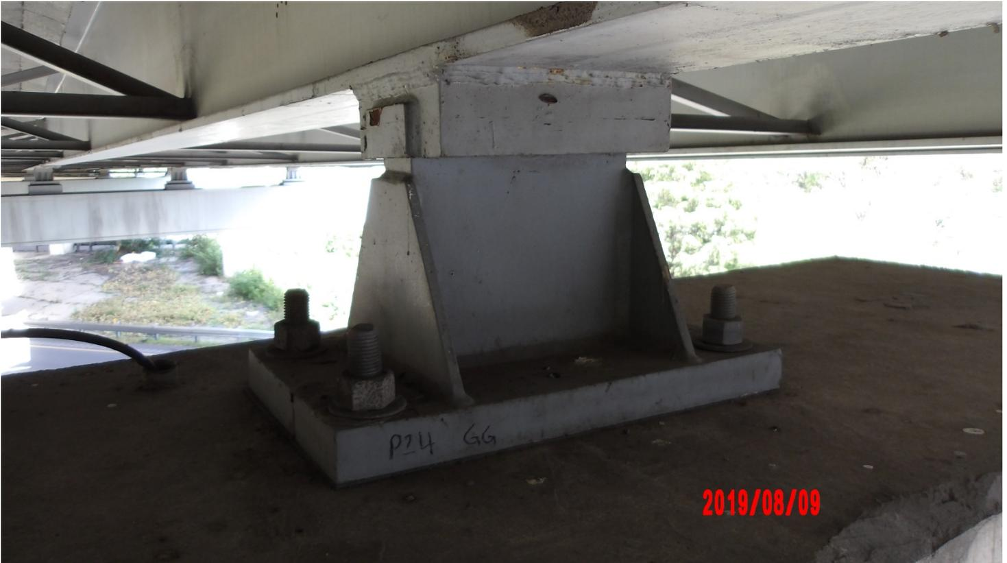
PHOTO 26. FIXED BEARING G PIER 24C
