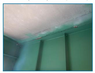
Photo 2 – 8' L shallow haunch spall in the deck (Girder A, Span 2, looking northeast).
