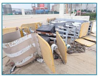
Photo 13 - Impact damage to the crash attenuator at the exit (South Approach, looking west).
