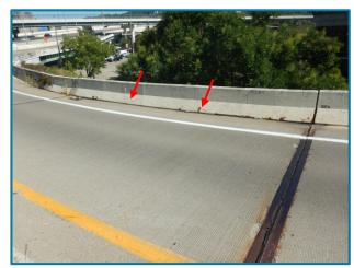
Photo 5 - Bridge railing with longitudinal cracking with rust stains (looking east).
