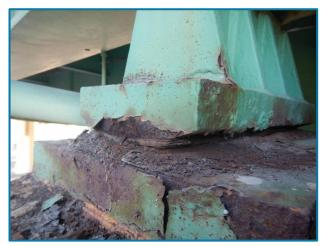
Photo 9 – 1/2" pack rust between the rocker and the masonry plate (Girder A, Pier 2, Span 3, looking south).
