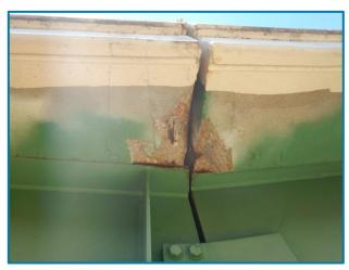
Photo 3 – 1'-6" L x 1' W x 6" D spall in the deck overhang (Girder A, Spans 1-2, looking west).
