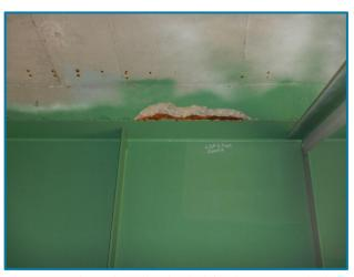
Photo 1 - 2'L haunch spall in the deck (Girder B, Span 2, looking southwest).
