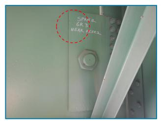
Photo 8 – Gouges in the plate at the hinge over Pier 1 (Pier 1, Girder A, looking east). The markings on the bridge as shown in the photo are incorrect.
