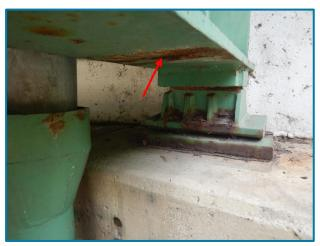
Photo 7 – Surface corrosion to the girder bottom flange (Girder A, Span 1, looking north).
