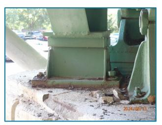
Photo 11 – Loose anchor nut and section loss (Girder A, Pier 4 (HAM-50-2180N), Span 3, looking east).
