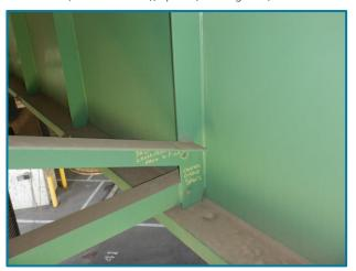
Photo 12 – Insufficient weld length and missing connection (Girder A, Span 2, looking north).
