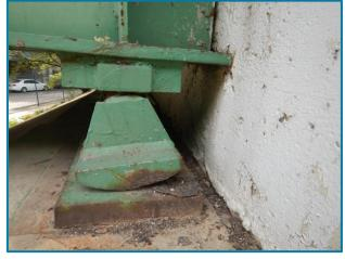
Photo 10 – Corrosion to the bearing and Girder A contacting the backwall (Girder A, Rear Abutment, 4, looking west).
