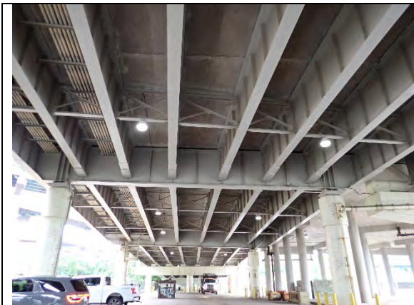
Photograph 16: Pier 19 Elevation, Looking North.
