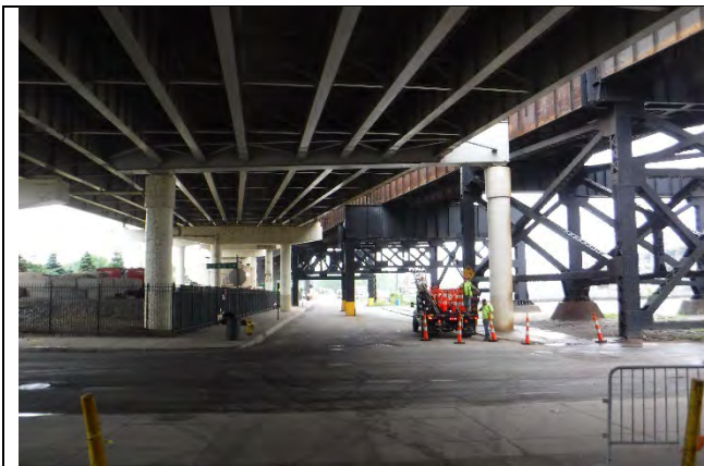
Photograph 3: Overall Elevation, Looking South.
