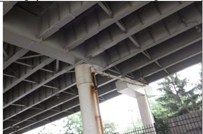
Photograph 6: Pier 18 Underview, Looking Southwest.
