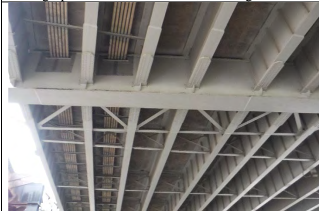
Photograph 5: Pier 18 Underview, Looking North.
