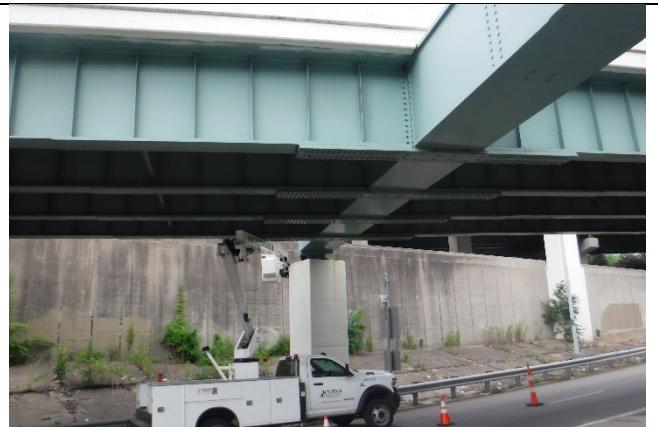
Photograph 2: Overall View, Looking West.
