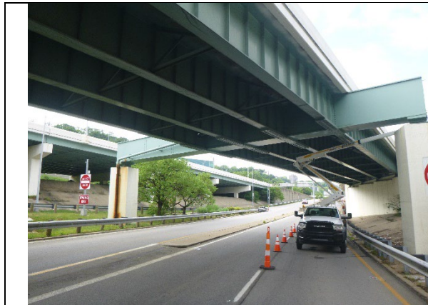
Photograph 1: Overall View, Looking South.
