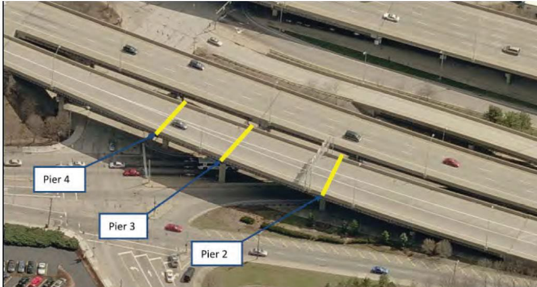
Aerial View looking east
