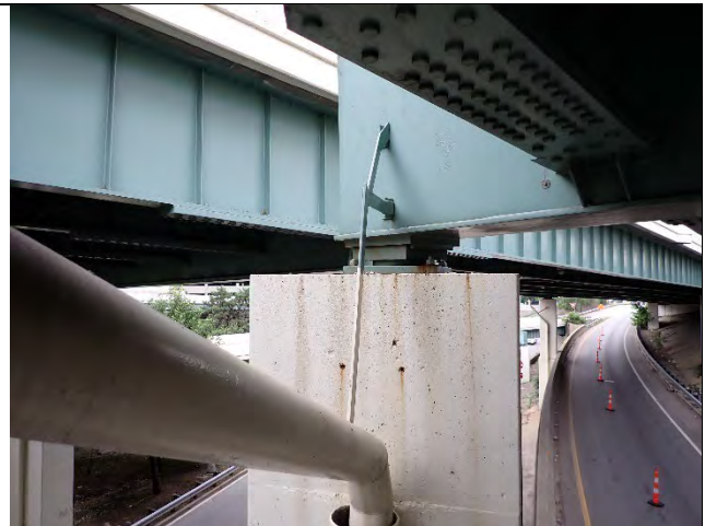
Photograph 17: View of Bolted Drainpipe Support Connection. No Change, Looking South.
