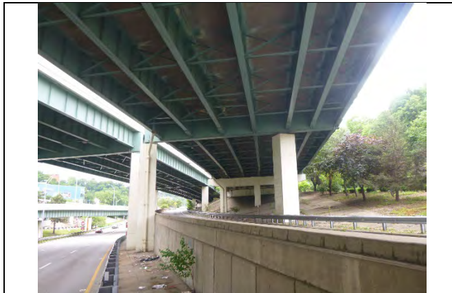
Photograph 3: General Elevation of Pier Cap 2, Looking South.
