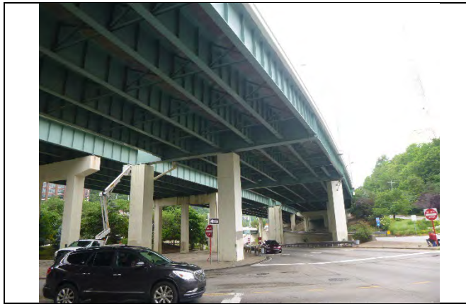
Photograph 31: General Elevation View of Pier Cap 4, Looking South.
