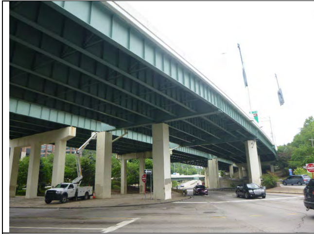
Photograph 1: Bridge Elevation, Looking Southeast.
