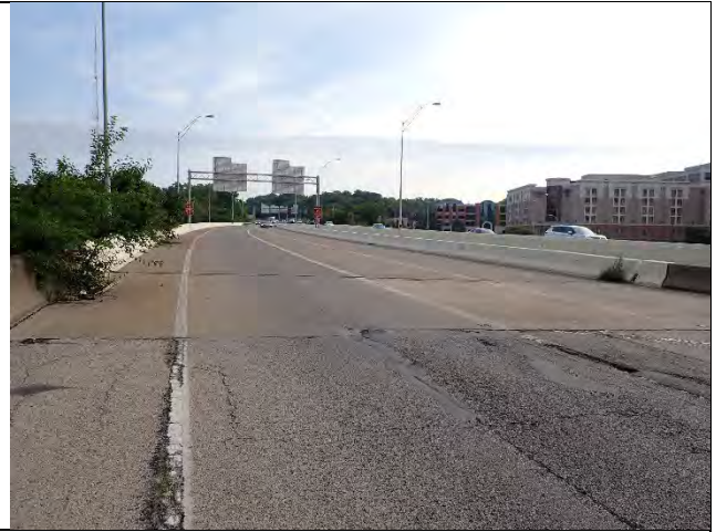
Photograph 2: Bridge Endview, Looking North.
