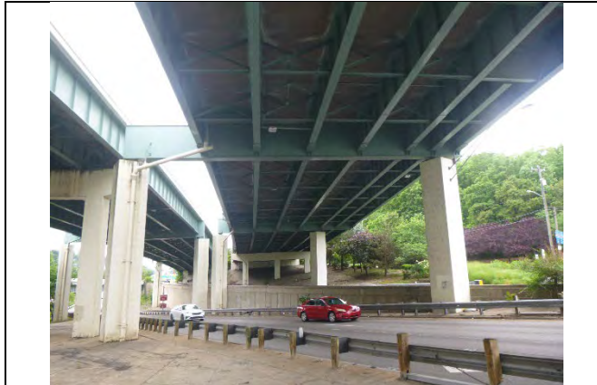
Photograph 18: General Elevation of Pier Cap 3, Looking South.
