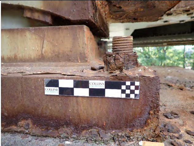
Photograph 16 – General Example of Heavy Bird Debris at Girder to Cap Web Plate Connections. West Cap Plate Shown, Looking East.
