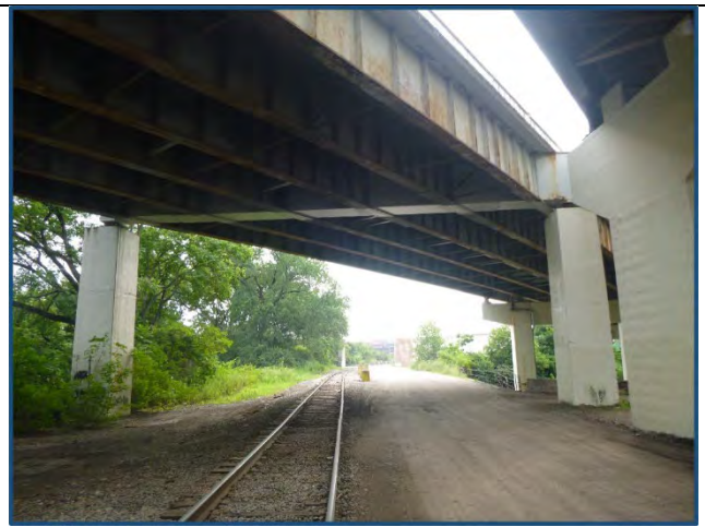
Photograph 2 – Elevation View of Pier Cap 5N. Looking East.
