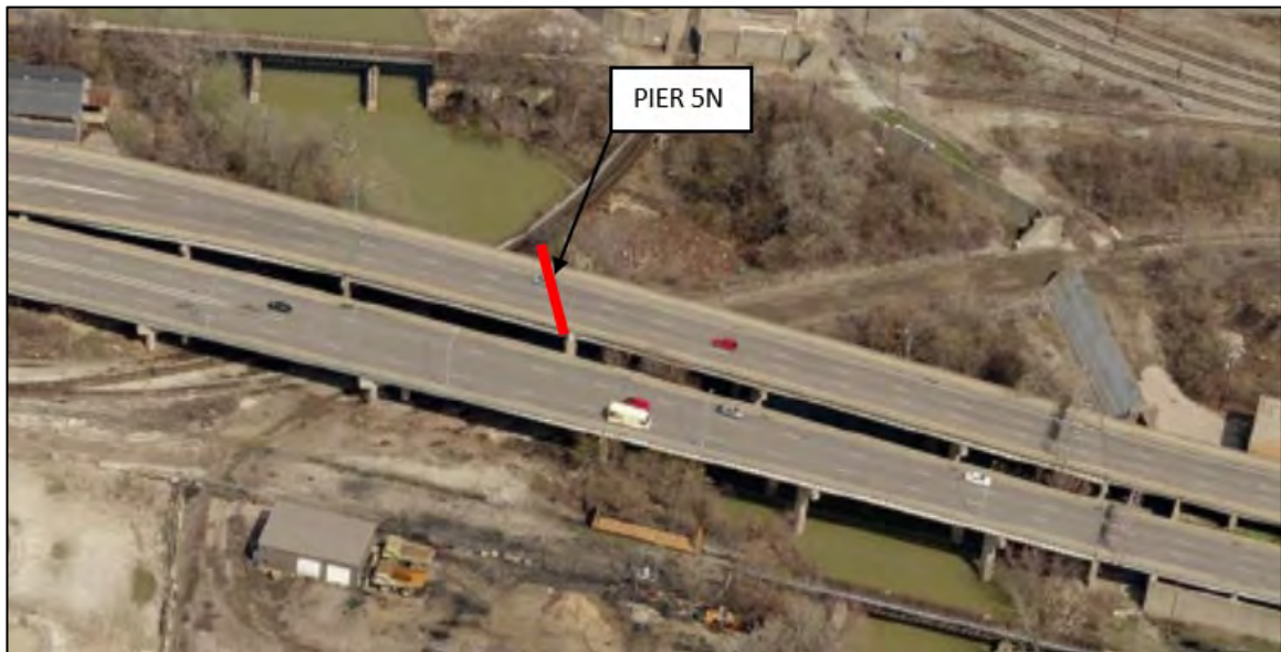
Figure 2: Fracture Critical Pier Cap Location
