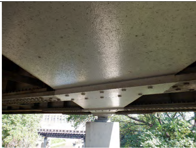
Photograph 1 – View of Pier Cap 5N. Looking north.
