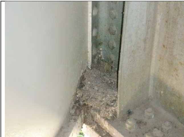
Photograph 16 – General Example of Heavy Bird Debris at Girder to Cap Web Plate Connections. West Cap Plate Shown, Looking East.
