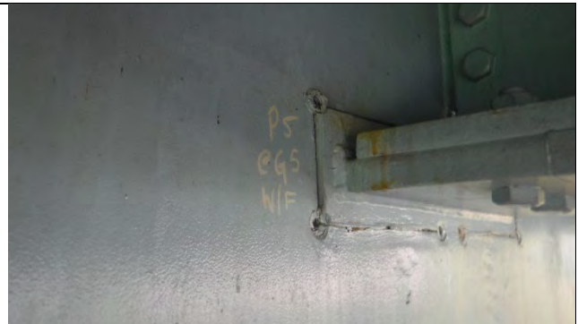
Photograph 24: Typical 1993 Rehabilitation Drill and Saw Cut Retrofits with Web Deflection.
