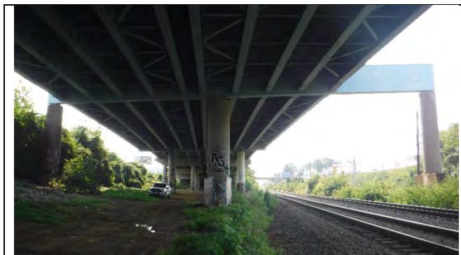
Photograph 44: General Elevation of Pier Cap 8, Looking East.
