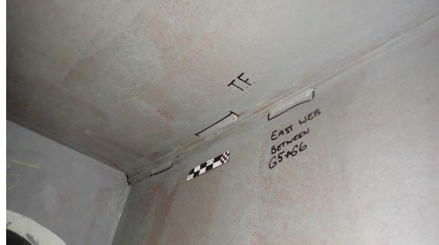
Photograph 55: Typical Fillet Welds Along Backer Bar Between Girders 5 and 6, Looking Northeast.
