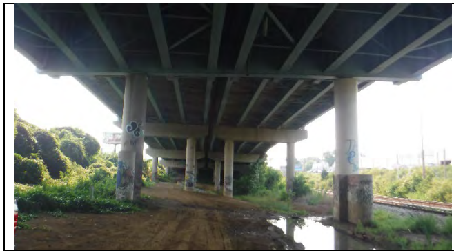
Photograph 52: General Elevation of Pier Cap 9, Looking East.
