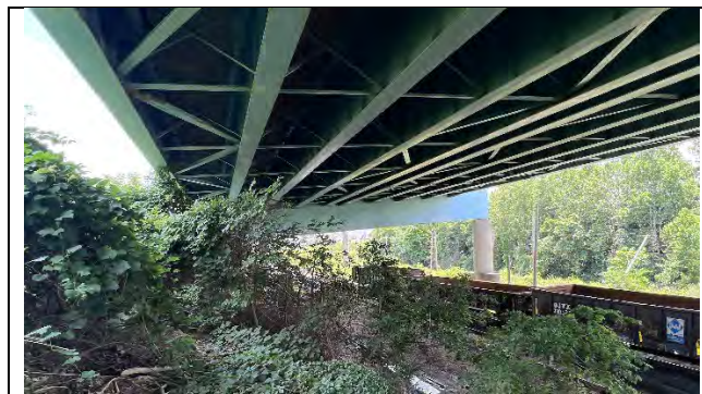
Photograph 37: General Elevation of Pier Cap 7, Looking East.
