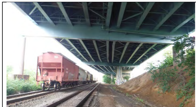
Photograph 27: General Elevation of Pier Cap 6, Looking West.
