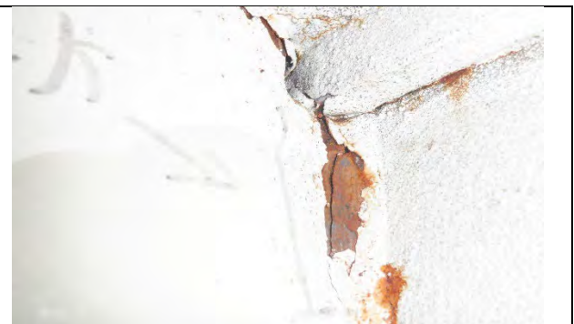
Photograph 29: View of 1.5 in. Weld Crack at the Top of the Fillet Weld for the Diaphragm to West Web Plate at Girder 6, North Side of Diaphragm. Perspective View, Looking South.
