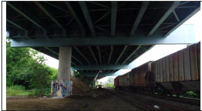
Photograph 1: General Elevation of Pier Cap 4, Looking West.
