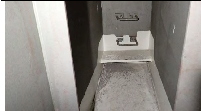
Photograph 53: Typical Interior Condition of Pier Cap 9, Looking South.
