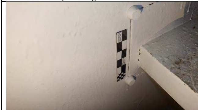
Photograph 19: Tack Welds on the Webs on the South Side of Girder 8 Bottom Flange, Looking West.
