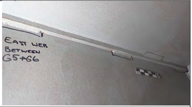
Photograph 54: Typical Fillet Welds Along Backer Bar Between Girders 5 and 6, Looking Southeast.
