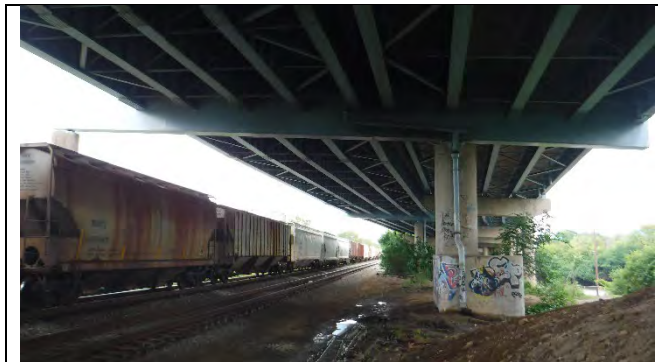
Photograph 14: General Elevation of Pier Cap 5, Looking West.
