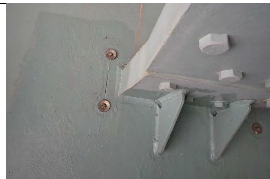
Photograph 9: Typical Example of Drilled Hole Retrofits at Girder Bottom Flanges/Tie Plates.
