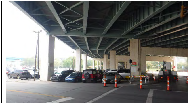
Photograph 21: General Elevation of Pier Cap 2W, Looking Roadway North.
