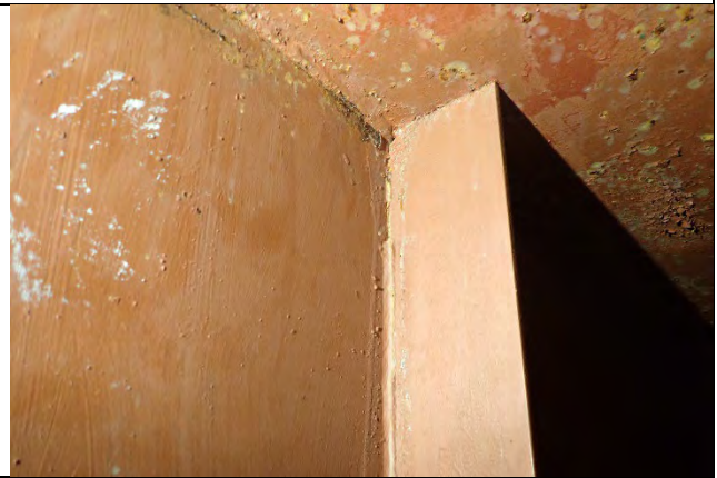
Photograph 25: View of Discontinuous Weld Noted on the North Web Stiffener between Girders A and B.
