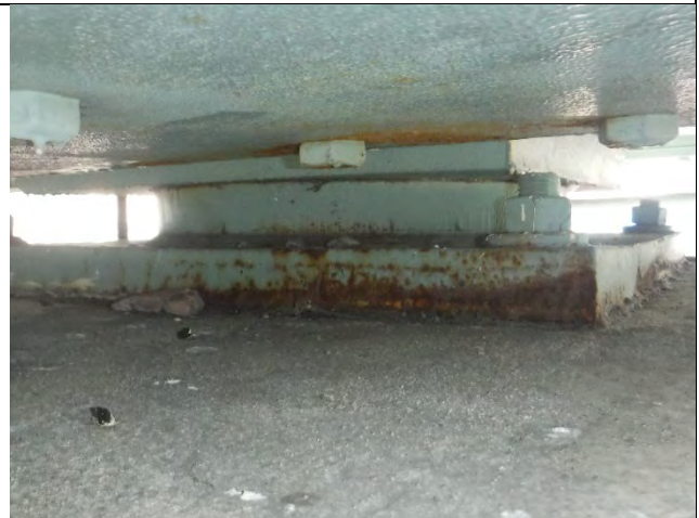
Photograph 54: View of the Typical Bearing Condition.
