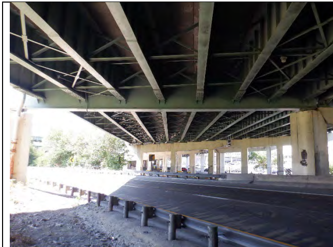
Photograph 60: Overall Cap Elevation, Looking Roadway South.
