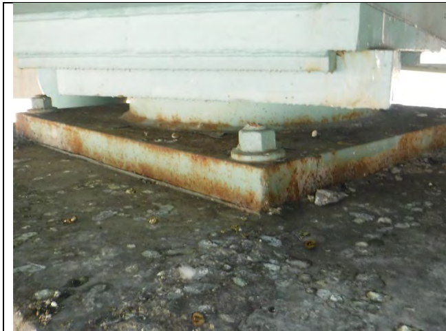
Photograph 38: View of the Typical Bearing Condition.
