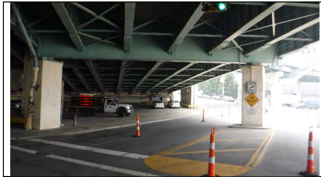
Photograph 3: General Elevation of Pier Cap 1W, Looking Roadway South.
