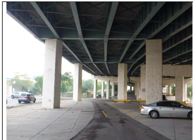
Photograph 40: General Elevation of Pier Cap 3W, Looking North.
