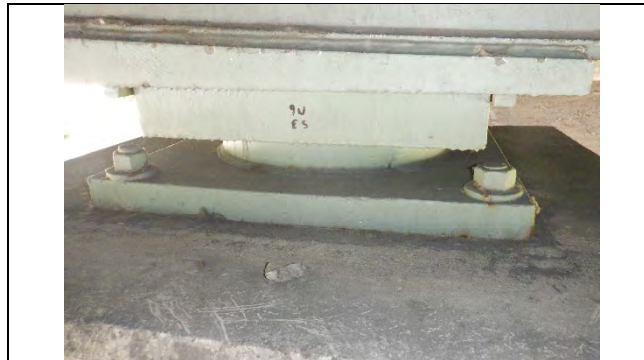
Photograph 77: Typical Bearing Condition, East Bearing Shown.
