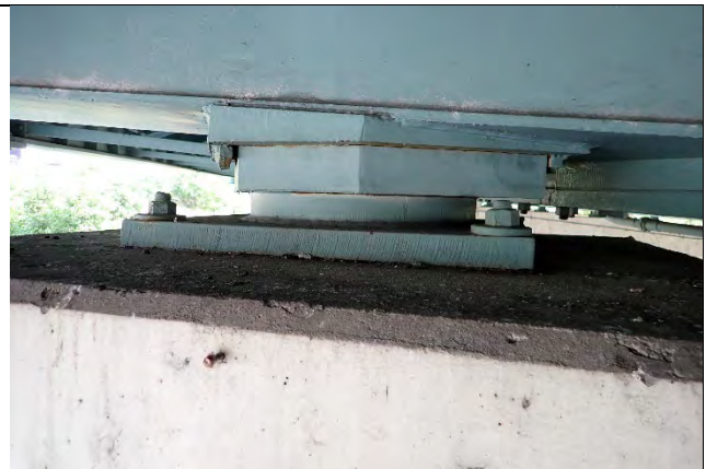
Photograph 59: View of the Typical Bearing, West Bearing Shown.
