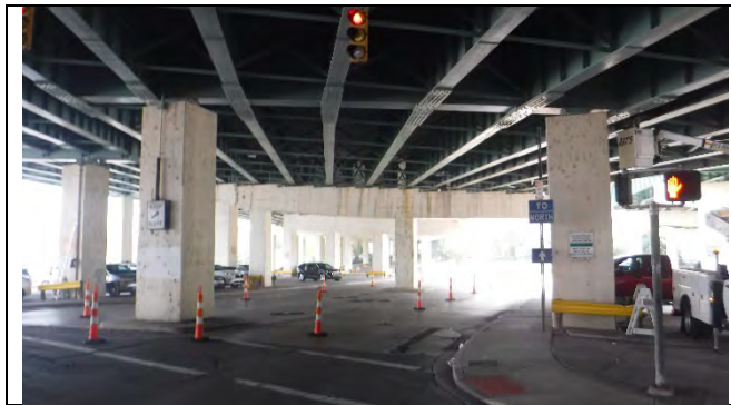
Photograph 12: General Elevation of Pier Cap 2E, Looking Roadway North.
