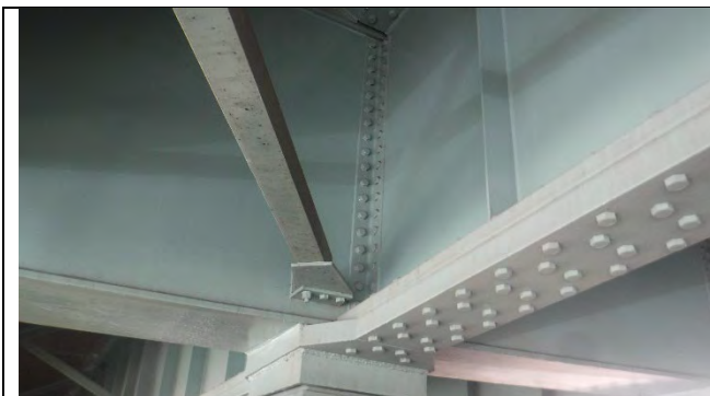
Photograph 8: View of Bolted Lateral Brace Connection Replacing Welded Connection, Looking Southwest.
