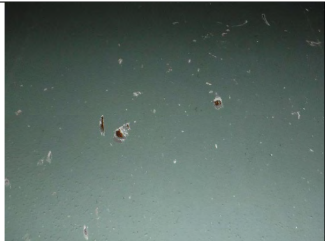
Photograph 33: View of Scratches seen throughout on Both North and South Webs of the Pier.
