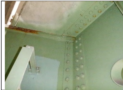
Photograph 10: General View of Bolted Drainpipe Connection in Place With Updated Drain Members and Configuration.
