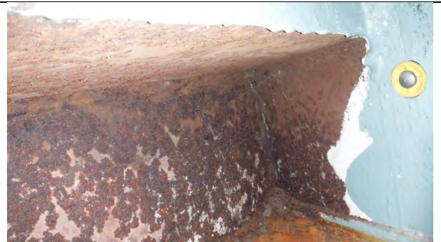
Photograph 5: View of Active Surface Corrosion Located Under Tie Plate on the South (Compass West) Face of Girder T Diaphragm.
