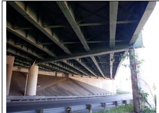
Photograph 3: Elevation Photograph of Pier Cap 1 Looking South.
