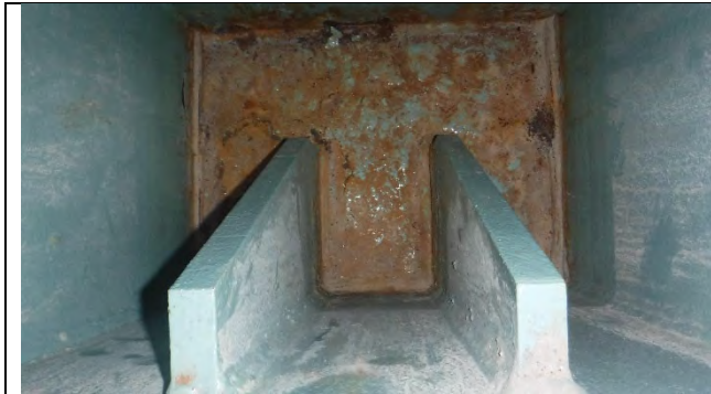
Photograph 4: View of Cap Bottom Plate Between the East (Compass South) Bearing Stiffener and End Plate. Note No Ponded Water. Looking Down.
