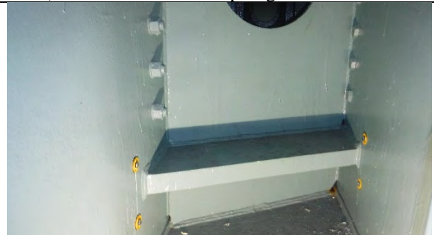
Photograph 5: View of Active Surface Corrosion Located Under Tie Plate on the South (Compass West) Face of Girder T Diaphragm.
