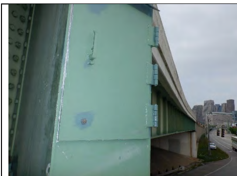
Photograph 1: View of Hatch Exterior, West Hatch Shown. Looking South.
