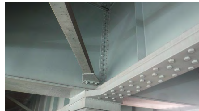
Photograph 12: Bolted connection of Web Plates to Girder A, Looking Southwest.
