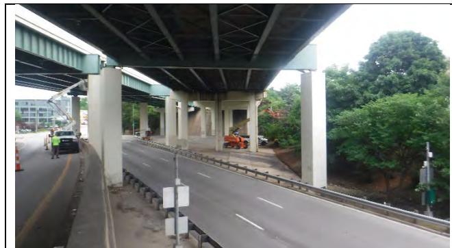
Photograph 23: General Elevation of Pier Cap 3, Looking North.
