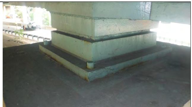
Photograph 13: Typical Example of Missing Nuts at Pier 1, West Bearing, Looking Northeast.
