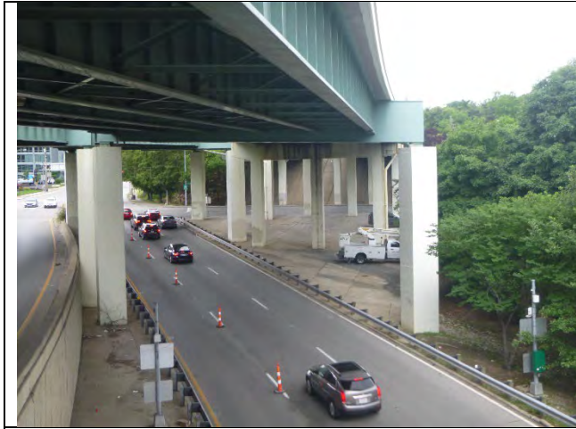
Photograph 1: Bridge Elevation, Looking North.
