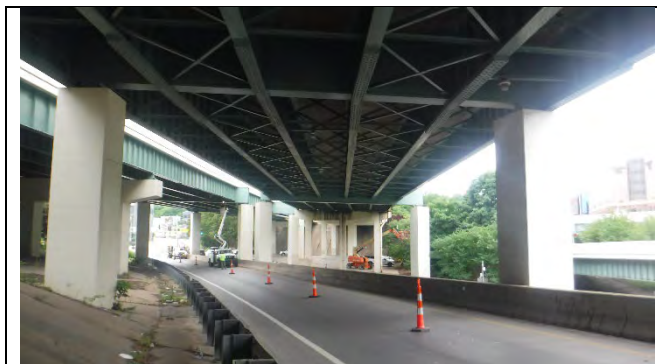
Photograph 15: General Elevation of Pier Cap 2, Looking North.
