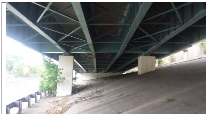
Photograph 3: General Elevation of Pier Cap 1, Looking South.
