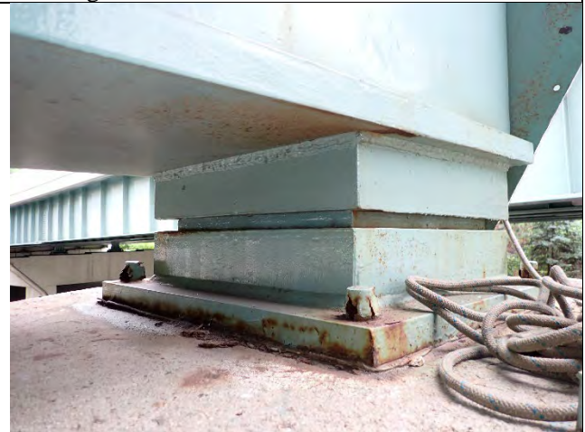
Photograph 29: View of the Typical Bearing Conditions, Looking West.
