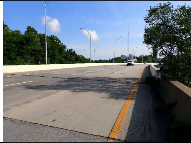
Photograph 2: Bridge Endview, Looking North.
