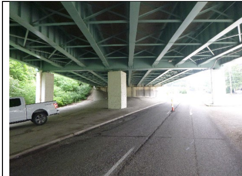
Photograph 43 – Overall View of Pier Cap 12 Looking North.
