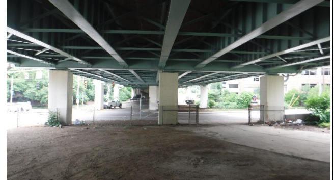
Photograph 2: General View of Superstructure, Looking North From Pier 9.
