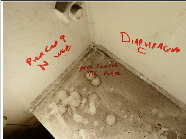
Photograph 7 – General Example of Triaxial Weld Connection. North Cap Web at Diaphragm C, West face shown.
