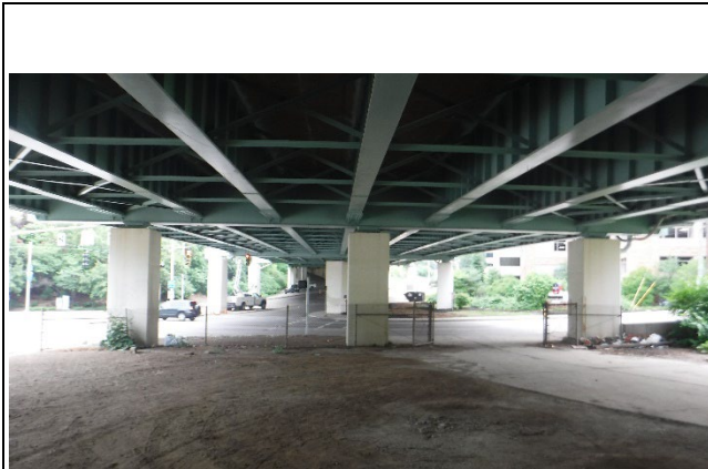
Photograph 3 – Overall View of Pier 9, Looking North
