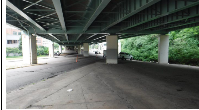
Photograph 1: General View of Superstructure, Looking South From Pier 12.
