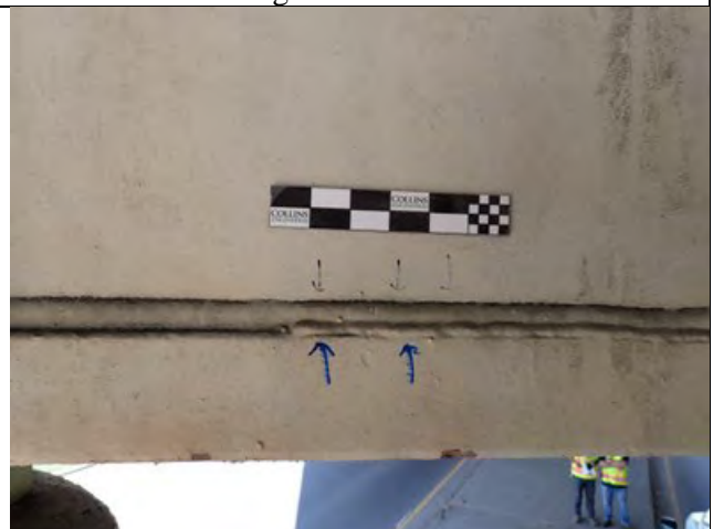
Photograph 29 – General Example of Multipass Welds, North Side Shown. Looking South.
