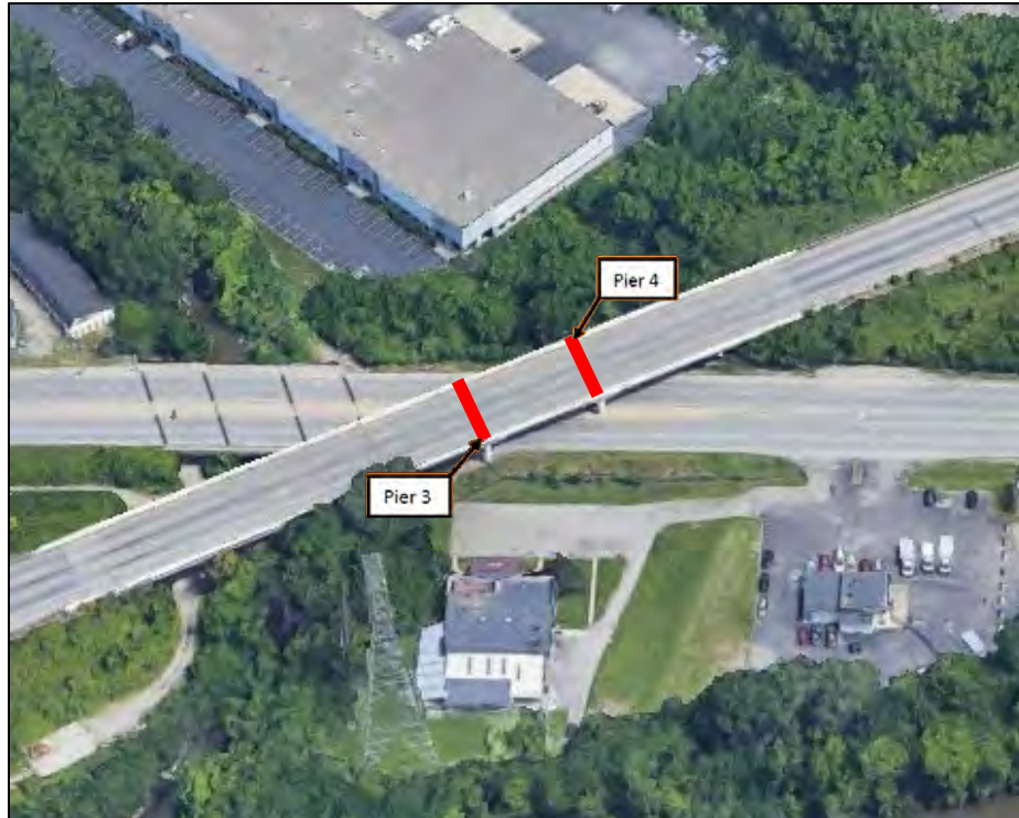
Figure 2: Fracture Critical Pier Cap Location
