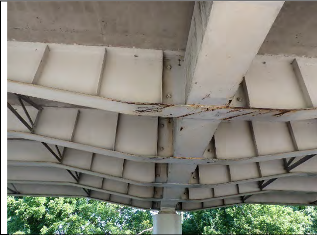
Photograph 19 – General Underview Pier Cap 4. Looking west.
