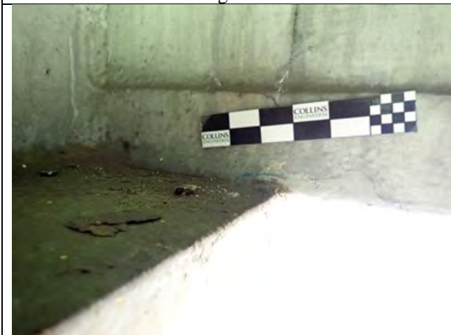
Photograph 28 – View of a 2 in. Tack Weld On West Side of Girder 2, North Face of Pier Cap. Looking Southeast.
