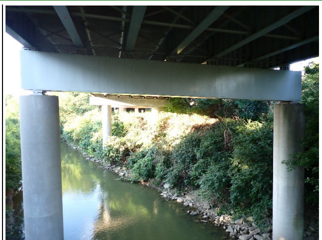
Photograph 2 – Elevation View of Pier 5. Looking South.
