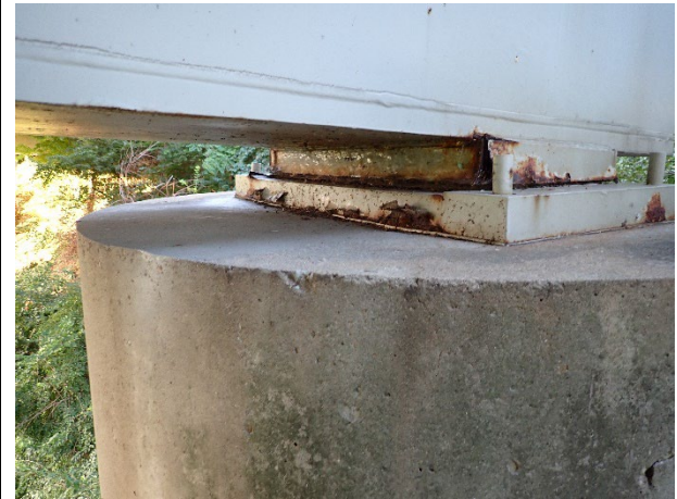
Photograph 11 – View of Bearing at Pier Cap 5.
