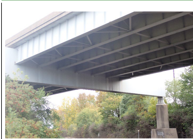
Photograph 1 – Elevation View of Pier 16. Looking Northeast.
