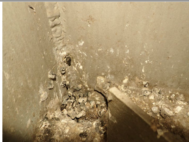
Photograph 24 – General Example of Cut Out Portion of Lateral Bracing Retrofit at the Girder.
