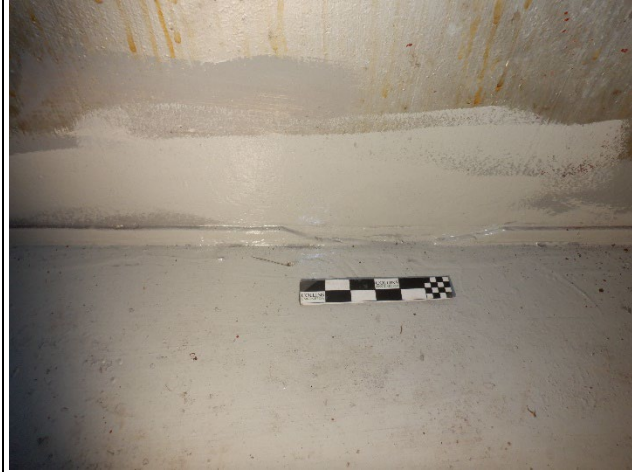
Photograph 5 – View of the Typical Backer Bar Removal, East of Girder 2 Shown.
