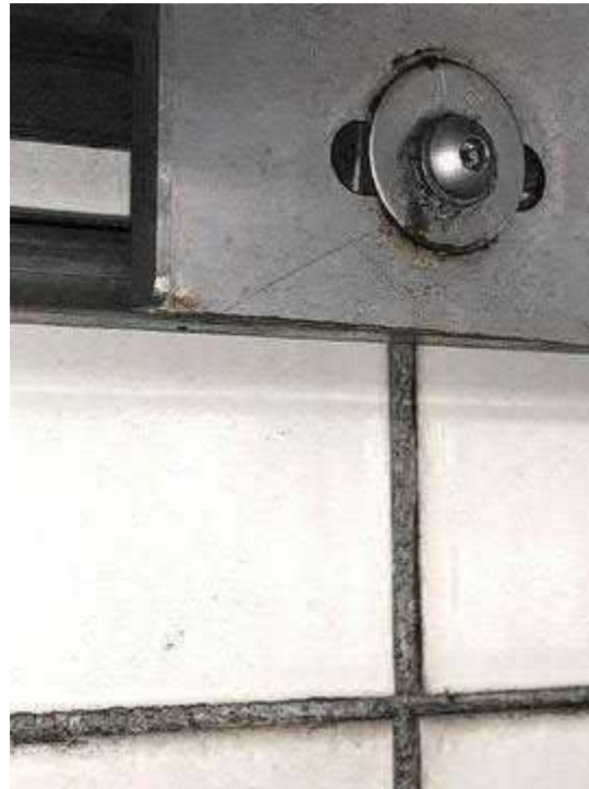
Tunnel Lighting Section
