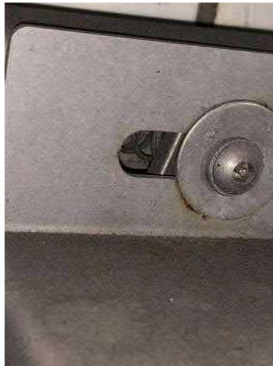
Tunnel Lighting Section
