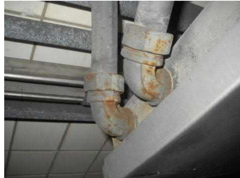
Tunnel Lighting Section
