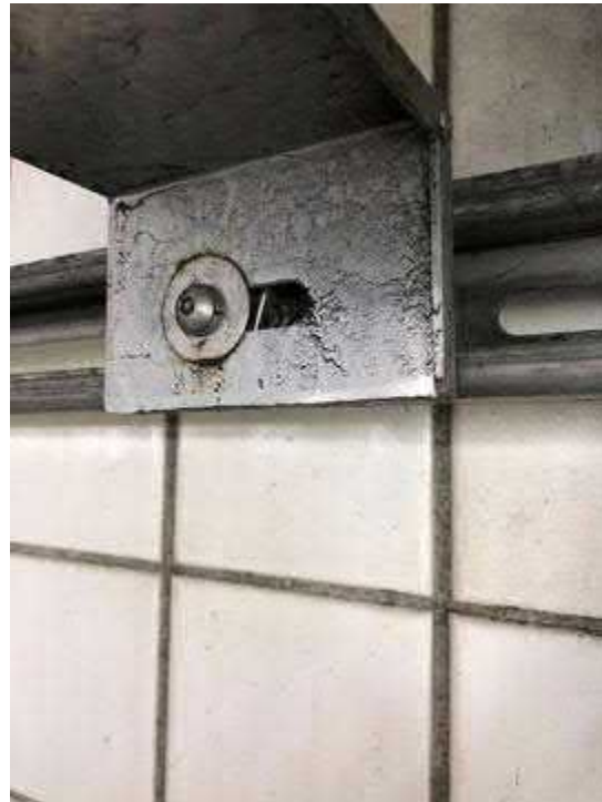
Tunnel Lighting Section
