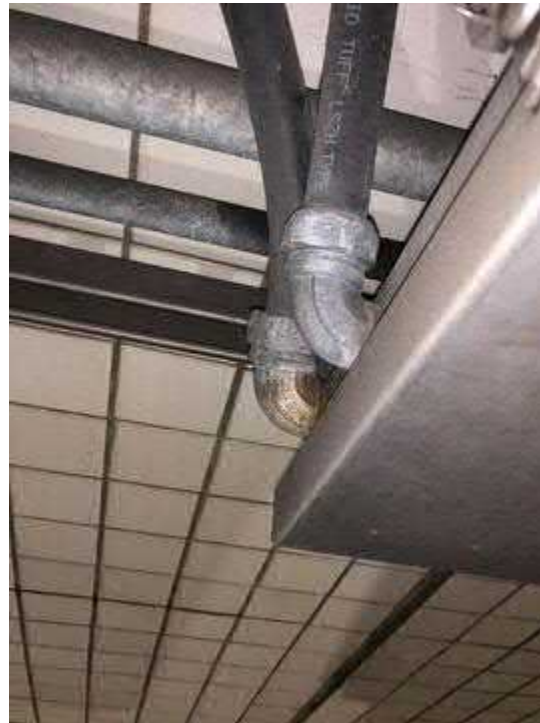
Tunnel Lighting Section
