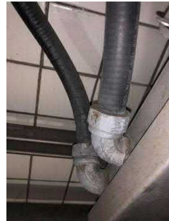
Tunnel Lighting Section
