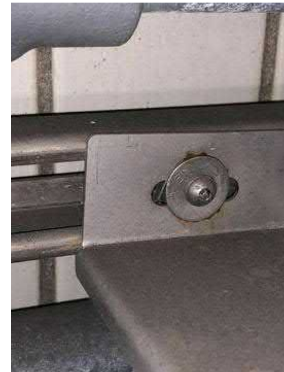
Tunnel Lighting Section
