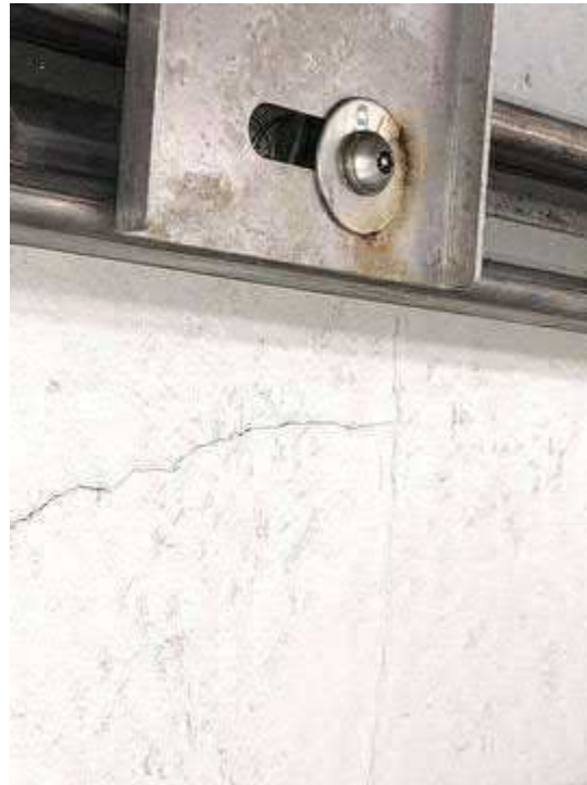
Tunnel Lighting Section
