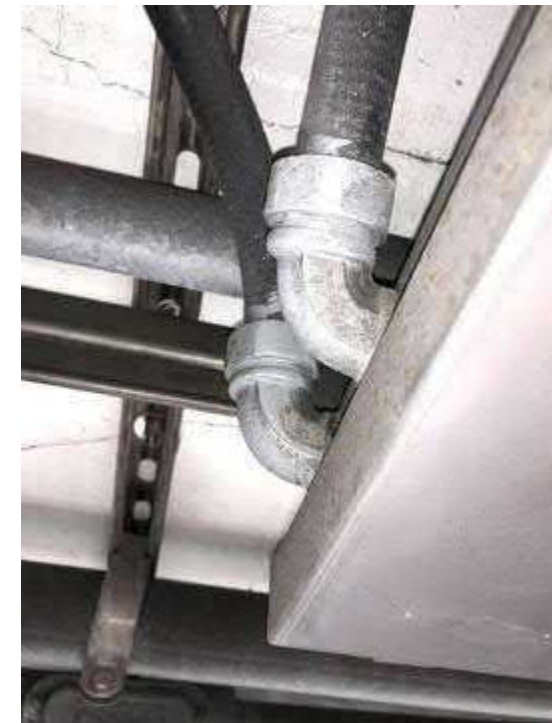
Tunnel Lighting Section
