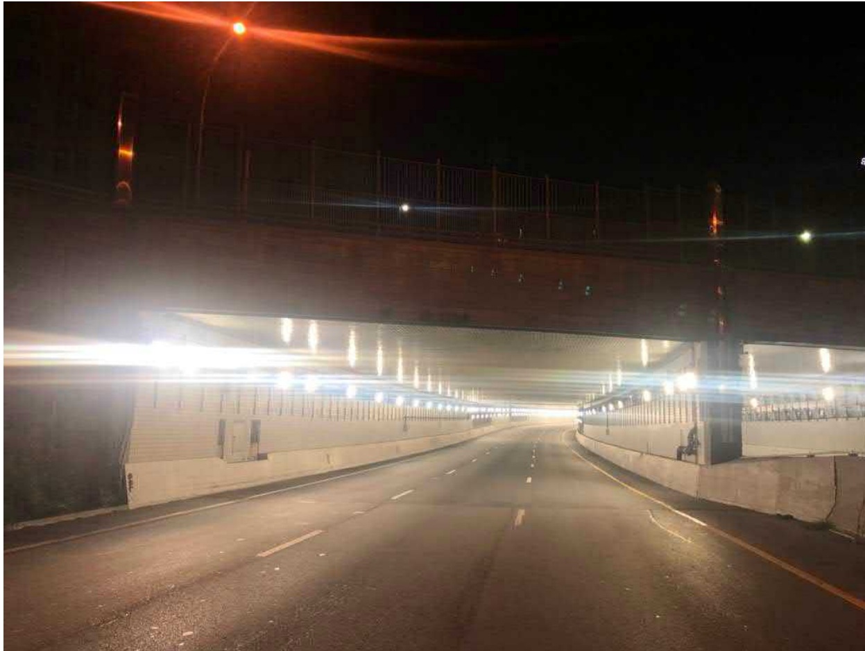
1-7 Inventory Photo: Northbound Looking South
