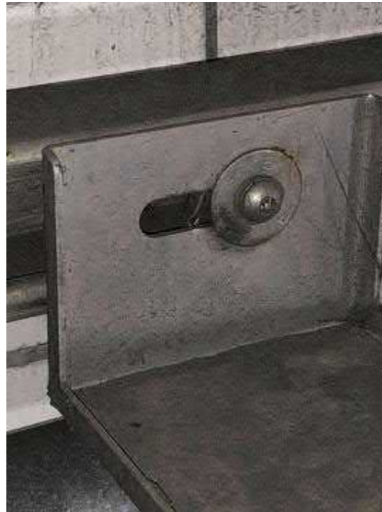
Tunnel Lighting Section
