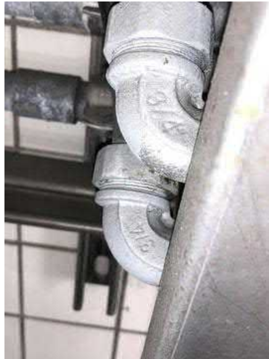
Tunnel Lighting Section
