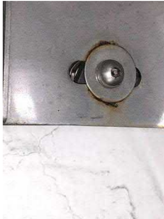
Tunnel Lighting Section
