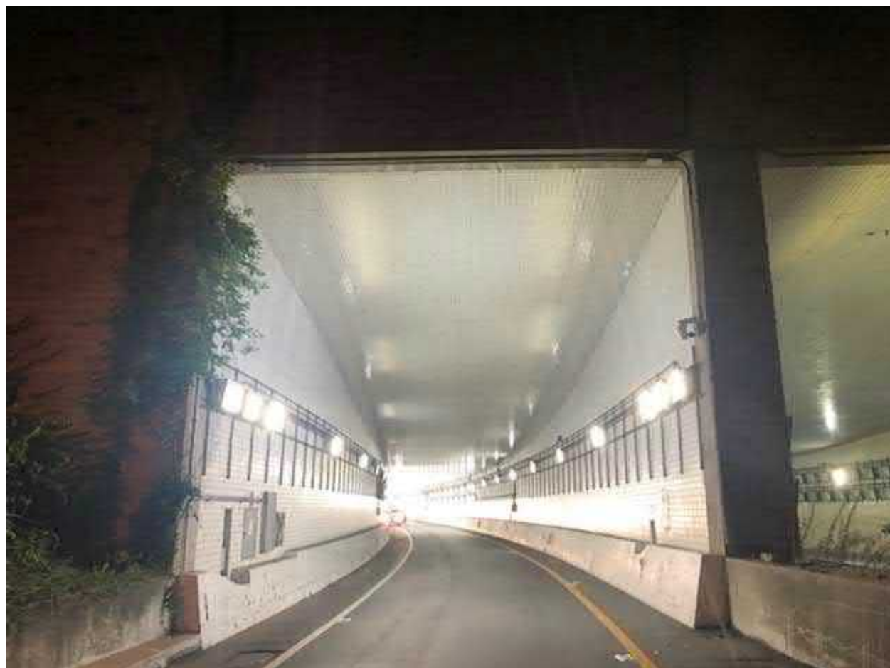
1-9 Inventory Photo: 3 rd Street Ramp Looking North
