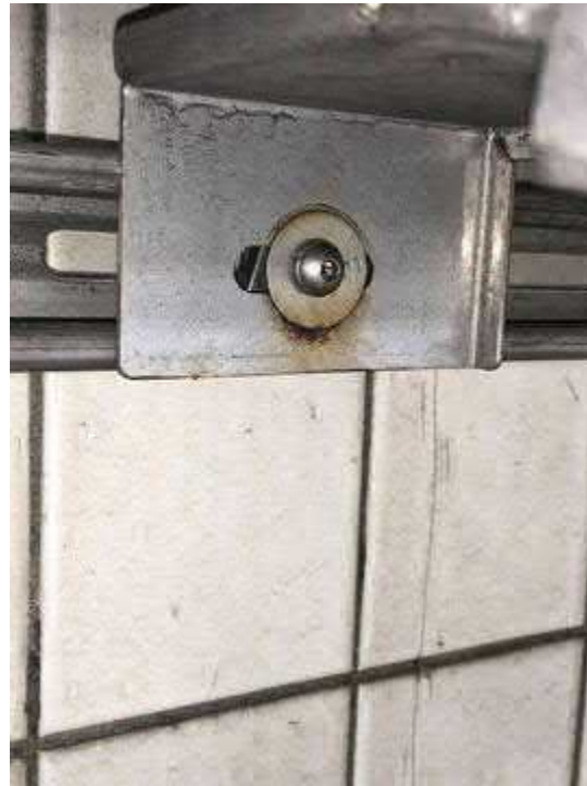
Tunnel Lighting Section
