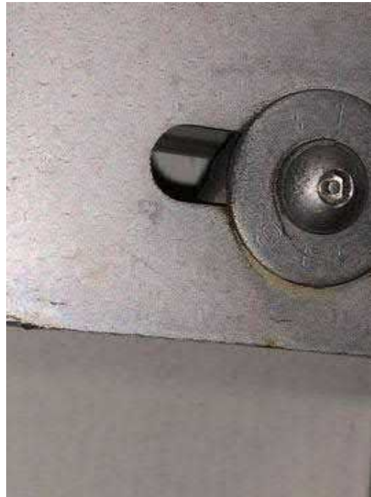
Tunnel Lighting Section
