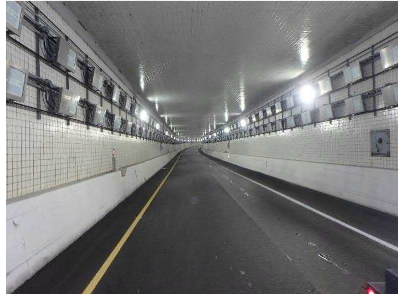
1-8 Inventory Photo: 3 rd Street Ramp Looking South
