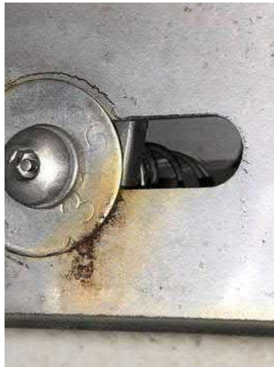
Tunnel Lighting Section
