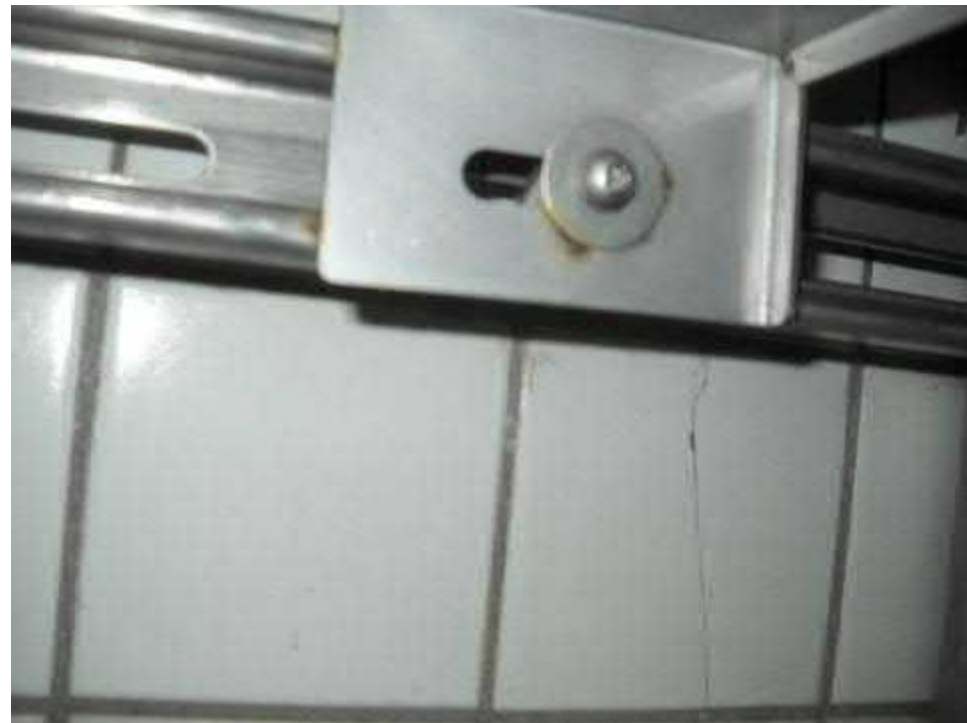
Tunnel Lighting Section
