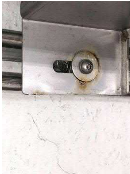
Tunnel Lighting Section
