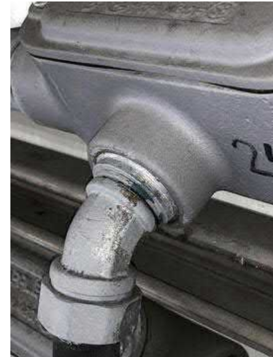
Tunnel Lighting Section
