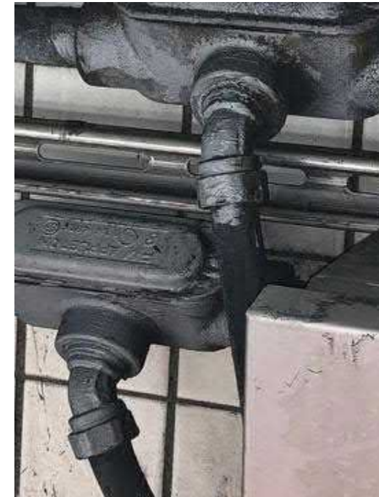
Tunnel Lighting Section
