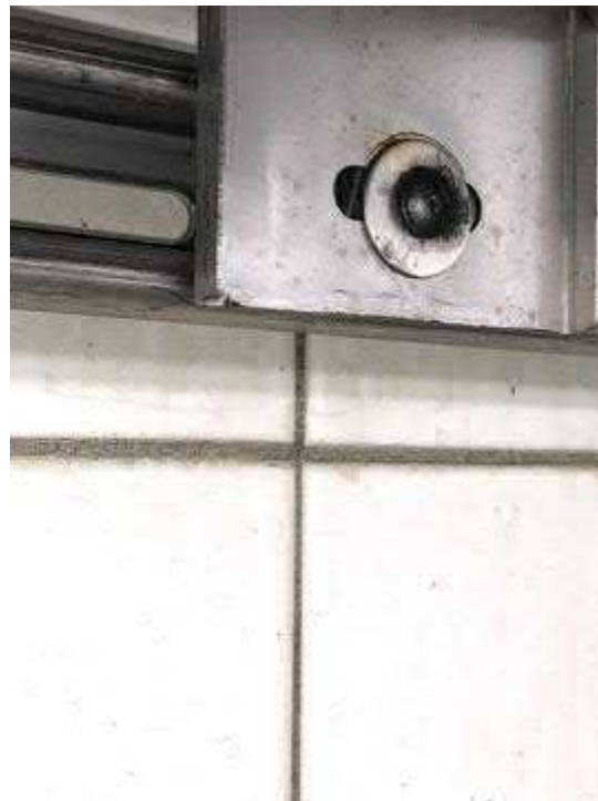
Tunnel Lighting Section
