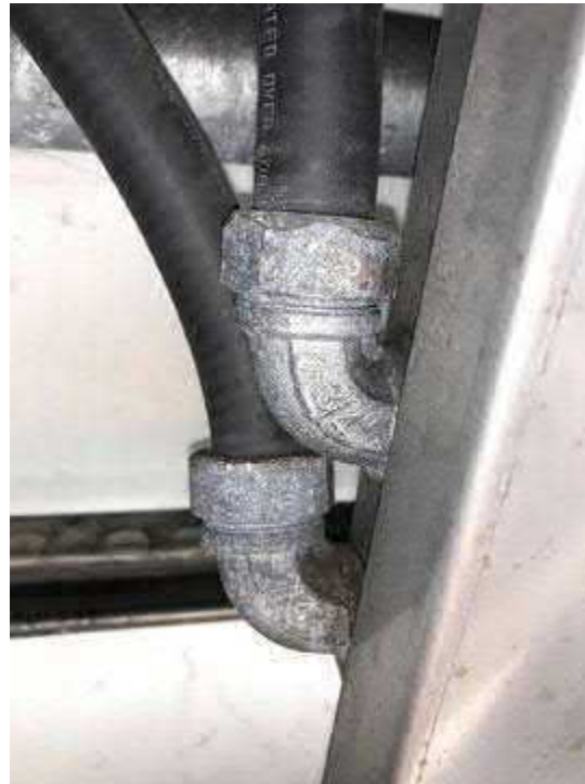
Tunnel Lighting Section
