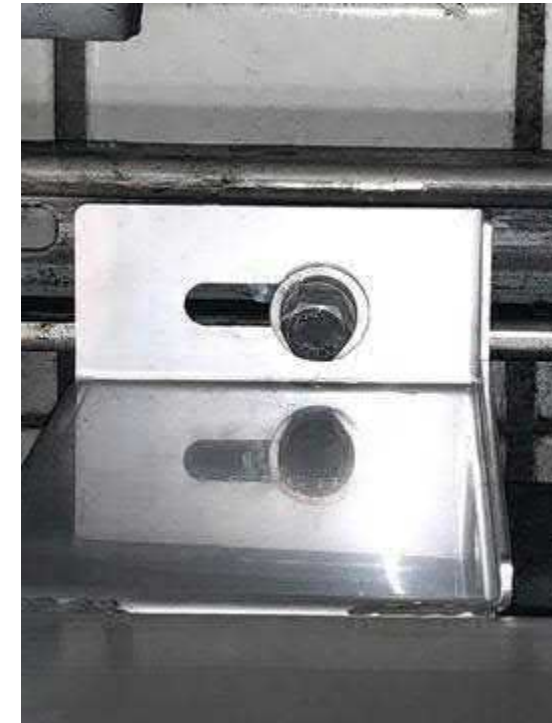
Tunnel Lighting Section
