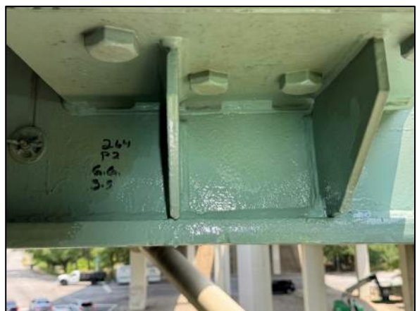
Photo 11: Retrofit at South Web and Bottom of Knee Brace at Girder G
