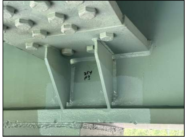
Photo 26: Retrofit of drilling out cracks in Fillet Weld Between Knee Brace and South Web Below Girder B
