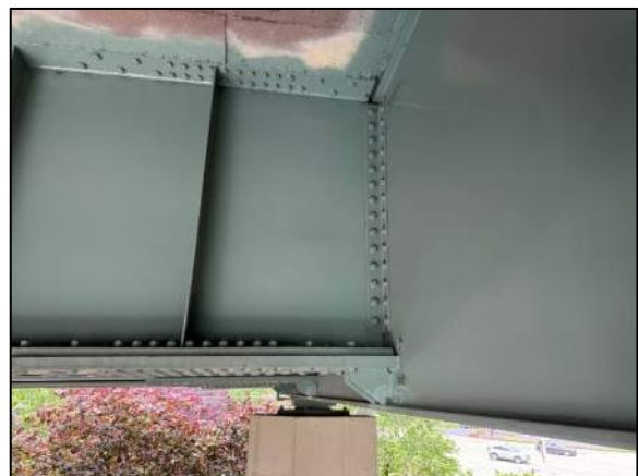
Photo 36: Typical Girder to Pier cap connection with knee plate retrofit
