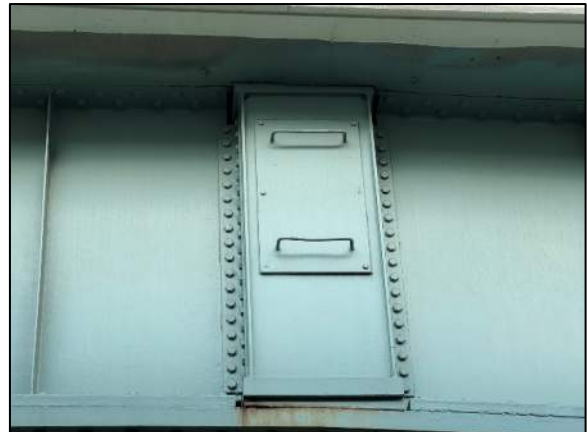
Photo 9: West Hatch for Pier 2
