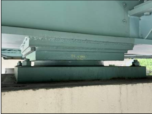
Photo 37: Typical West Bearing
