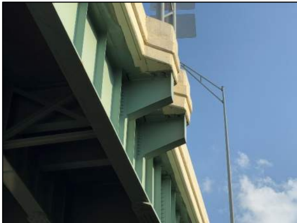
Photo 44: Sign Support Brackets Connected to Fascia Girder, North of Pier Cap 3
