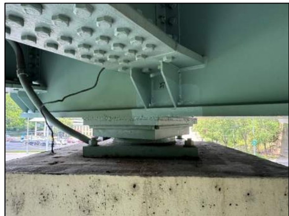
Photo 23: Typical view of West bearing
