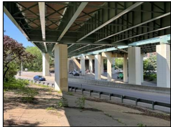
Photo 1: Pier Cap 2 Elevation
