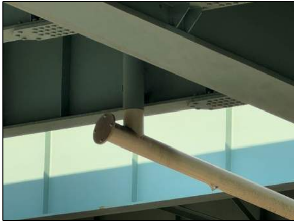
Photo 41: Down Spout Scupper Connection
