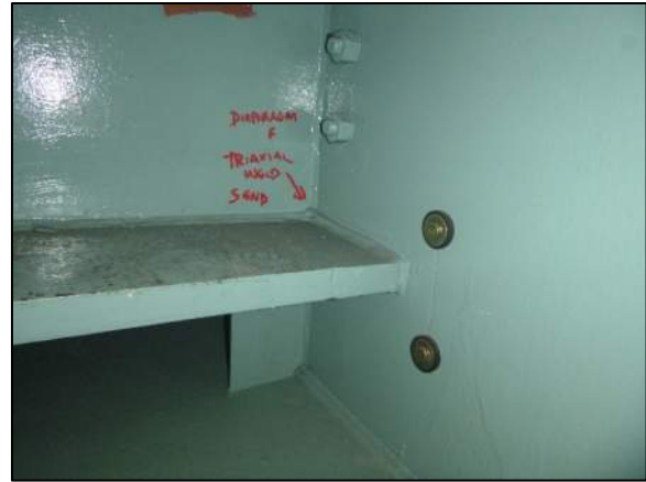
Photo 20: Triaxial Weld at Diaphragm F
