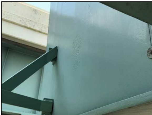
Photo 8: Bolted Connection Retrofit for Drain Connection
