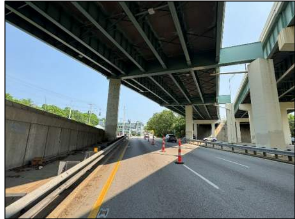
Photo 14: Pier Cap 3 Elevation
