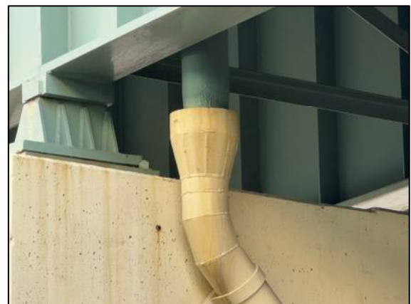
Photo 40: Down Spout Scupper Connection
