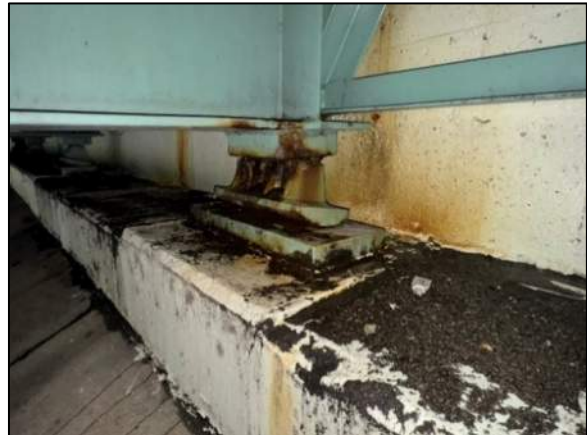
Photo 48: Debris on the Masonry Plate at Rocker Bearing Below Girder B
