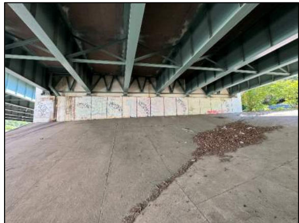
Photo 49: Typical View of Abutment 1
