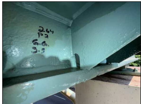
Photo 10: Retrofit at Bottom of Knee Brace at Girder G
