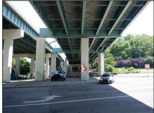
Photo 27: Pier Cap 4 Elevation
