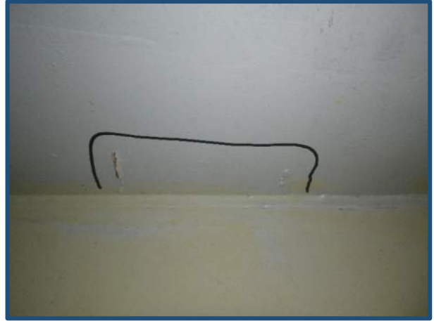
Photo 7: Two tack welds on the top flange north of Girder 1
