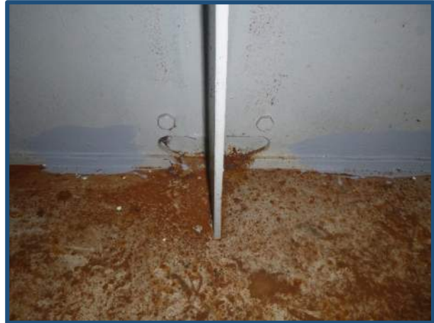
Photo 1: Typical stiffener retrofit
