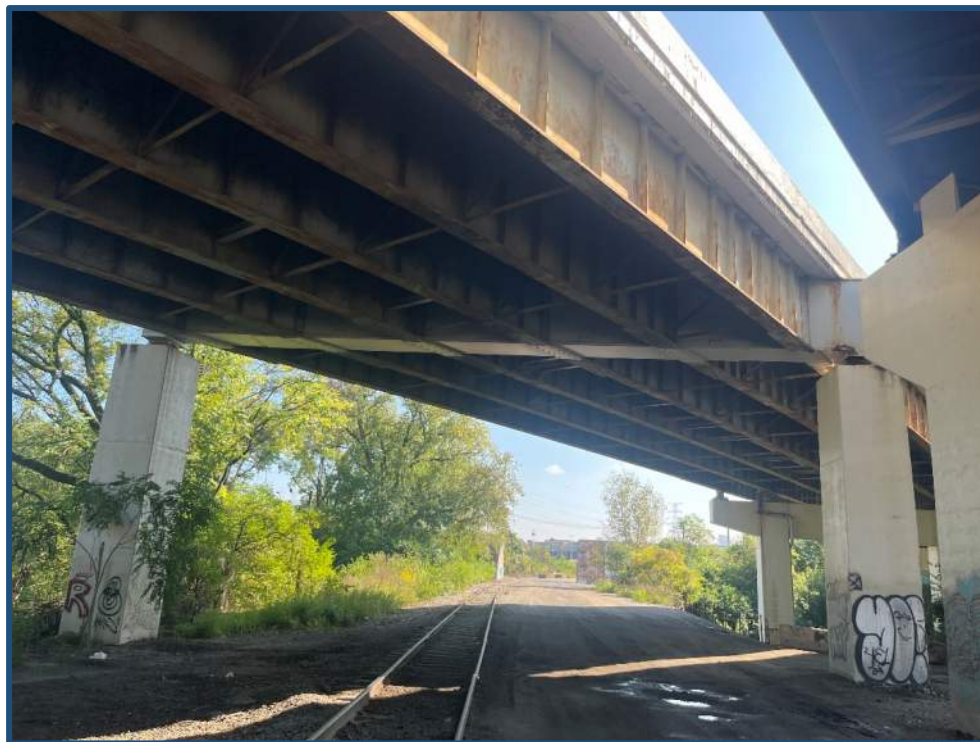
Figure 3: Elevation of Pier Cap 5N
