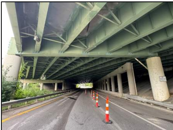
Photo 1: Pier Cap 1 Elevation
