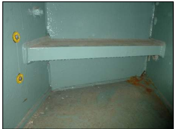
Photo 3: Previously Reported Area of Ponding Water on the Bottom Flange Tie Plate of Girder T Not Present. Dry During 2025 Inspection
