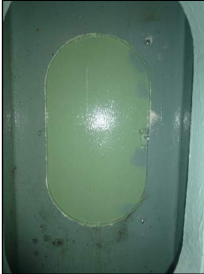
Figure 3: Interior Photo of North Hatch. Note No Interior Latch
