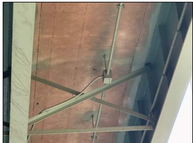
Photo 34: Typical Condition; East Face Girder A, South of Pier 4
