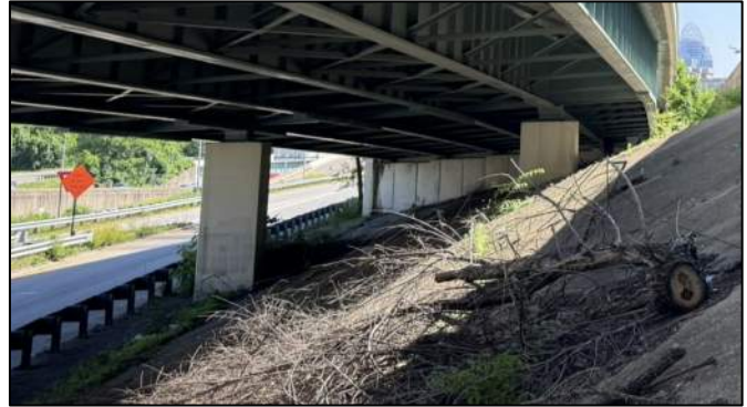
Photo 1: Pier Cap 1 Elevation
