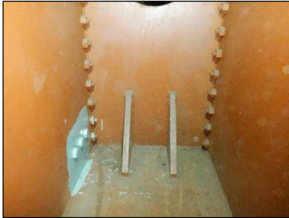
Photo 5: Typical Diaphragm Bracing
