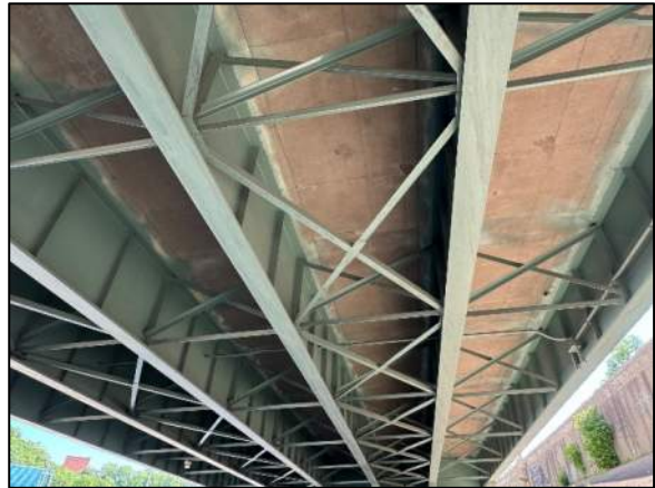
Photo 35: General view of Superstructure
