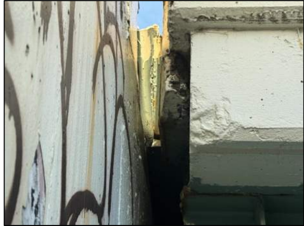
Photo 32: Typical condition of underside of Abutment 2 Joint
