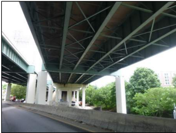
Photo 19: General Elevation Pier Cap 3
