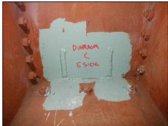
Photo 2: Knee Braces Removed and Fillet Welds Ground Out at Girder C Diaphragm
