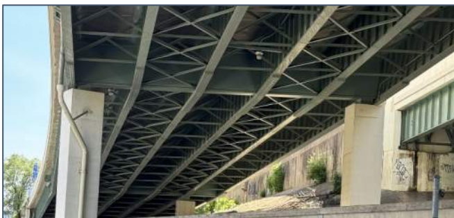
Photo 11: General Elevation Pier Cap 2
