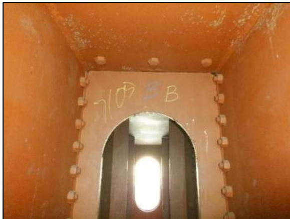
Photo 6: Girder B connection
