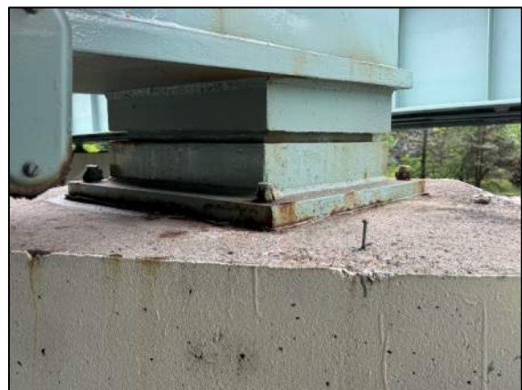
Photo 25: Typical, West Column Pot Bearing
