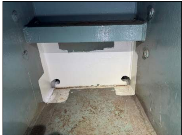
Photo 21: Corners of Girder Diaphragms Coped and Painted
