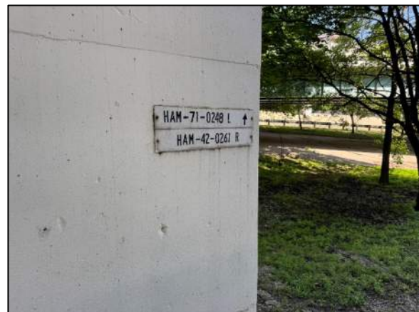
Photo 44: Bridge Placard on Pier 3
