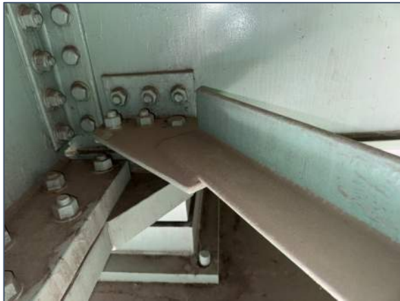
Photo 9: Retrofitting with Bolted Connections in Lateral Bracing
