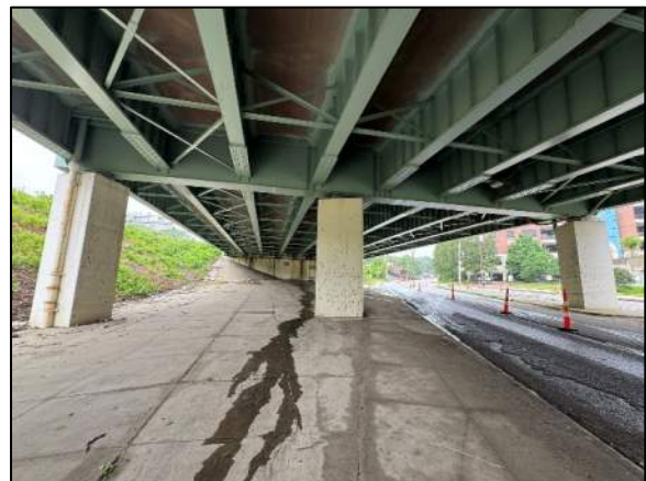
Photo 41: Pier Cap 12 Elevation
