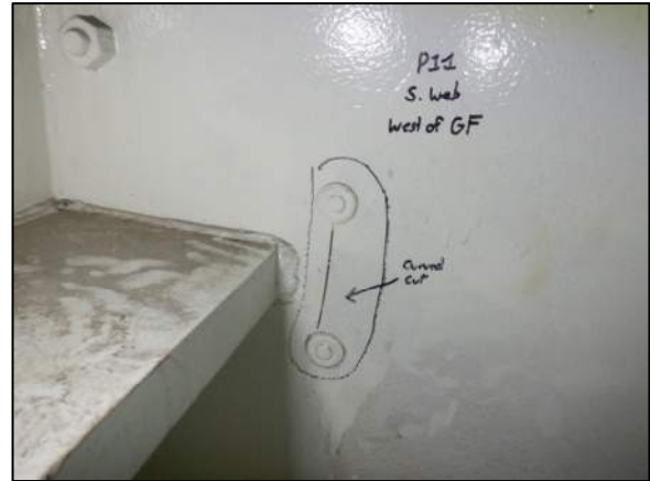
Photo 33: Curve in dog bone retrofit cut on South Web, West of Girder F
