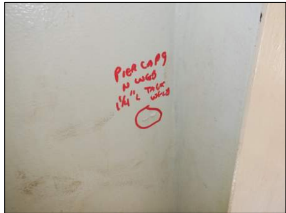
Photo 6: North Web Between East End and The Girder J Diaphragm; 1-1/4" L Tack Weld
