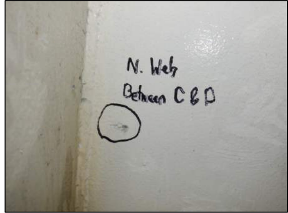
Photo 21: Tack Weld Between Girder C and D in North Web
