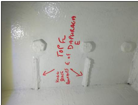
Photo 9: East Face of Girder E Diaphragm and Top Flange; Knee Brace Remnants at The Top Flange
