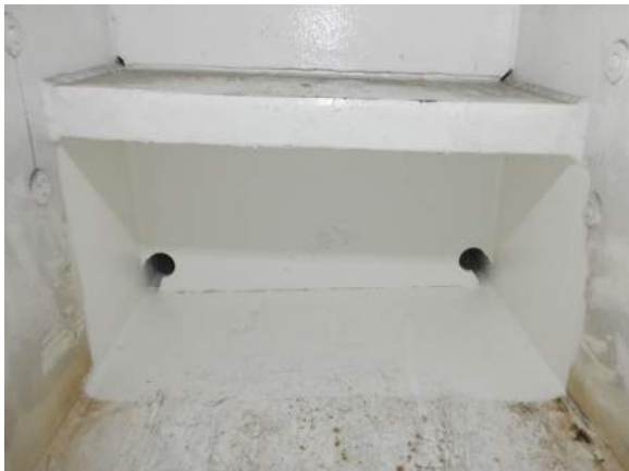
Photo 20: Underside of Bottom Flange Tie Plate, Recently Painted
