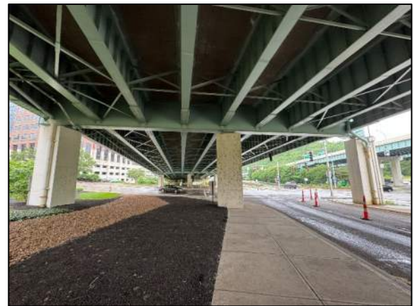
Photo 17: Pier Cap 10 Elevation
