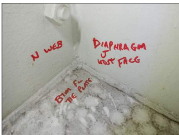
Photo 32: Triaxial Weld Between North Web, West Face of Diaphragm J and Bottom Flange Tie Plate
