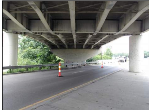
Photo 1: Pier Cap 3 Elevation
