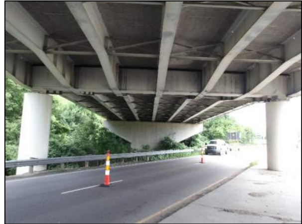
Photo 23: Pier Cap 4 Elevation
