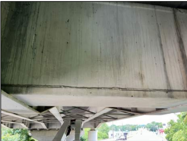
Photo 35: Typical multiple passes and overlap in the bottom flange groove weld of Pier Cap 4.
