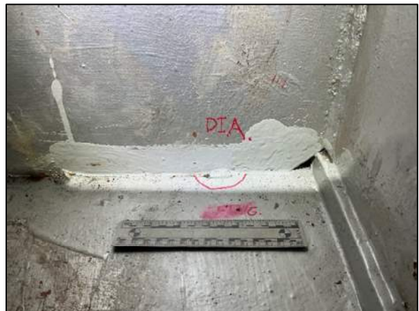
Photo 9: 1" tack weld on the Pier Cap 3 bottom flange at the diaphragm east of the west bearing.
