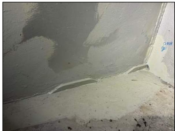
Photo 24: Typical bottom flange backer bar removal from a previous rehabilitation of Pier Cap 4.
