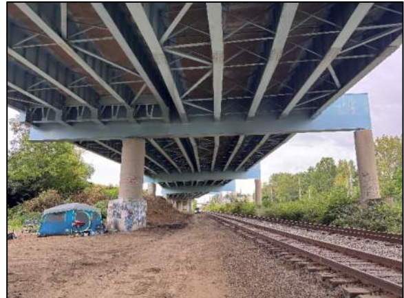
Photo 18: Elevation of Pier Cap 5
