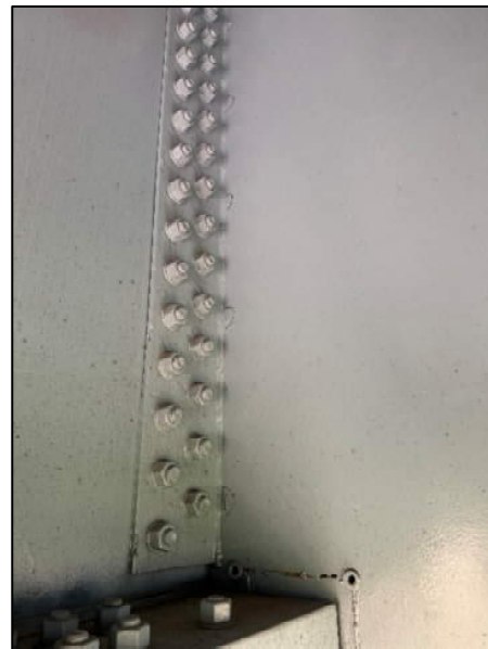
Photo 12: Five 1" tack welds on the west web at the south face of Girder 9
