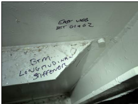
Photo 50: Typical longitudinal stiffener retrofit detail
