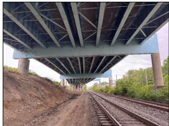
Photo 33: Elevation of Pier Cap 6
