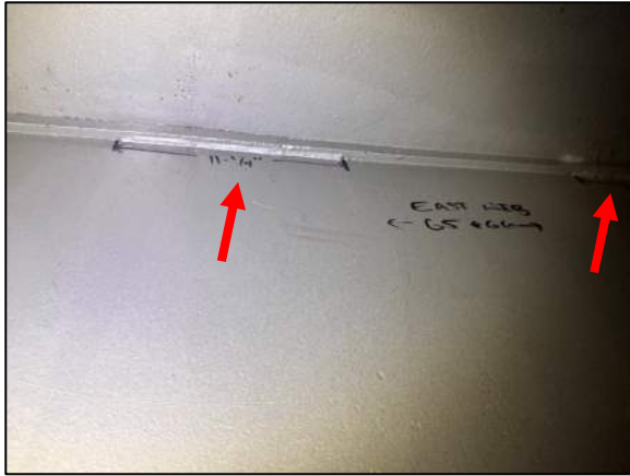
Photo 21: 6" & 11-1/4" long fillet welds between the top flange and east web between Girders 5 and 6
