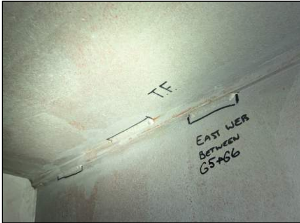
Photo 74: Fillet welds between the east web and top flange between Girders 5 and 6
