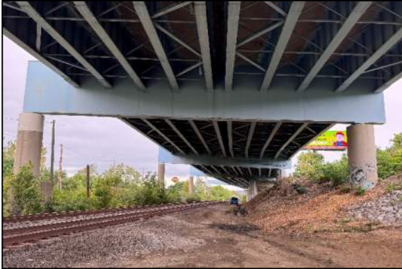
Photo 48: Elevation of Pier Cap 7
