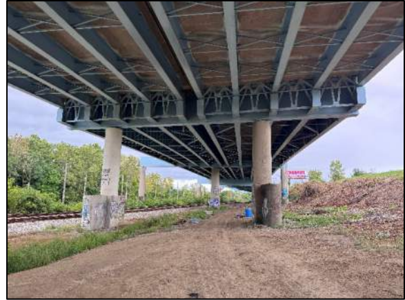
Photo 71: Elevation of Pier Cap 9
