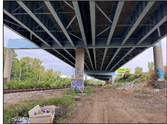
Photo 59: Elevation of Pier Cap 8
