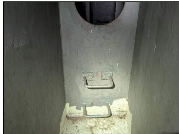
Photo 72: Typical interior paint condition (Girder 5 shown)
