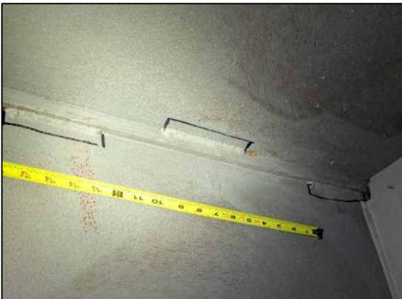
Photo 75: Fillet welds between the east web and top flange between Girders 5 and 6
