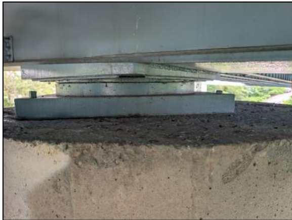
Photo 81: Pier 5 typical bearing condition (north bearing shown)
