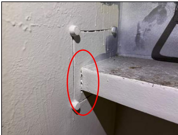
Photo 22: Tack welds on webs on the south side of Girder 8 bottom flange
