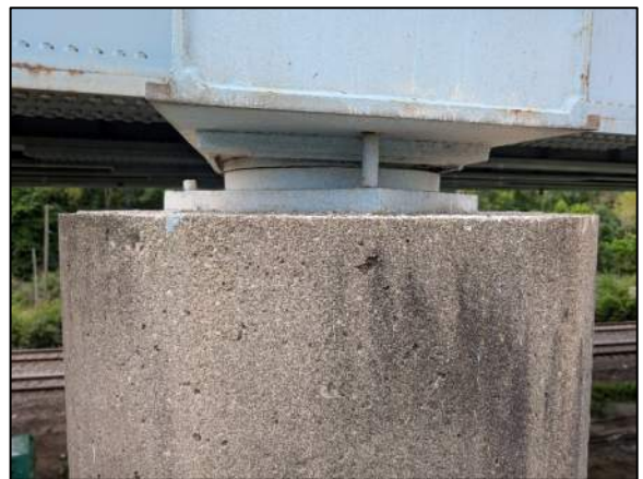
Photo 84: Pier 8 typical bearing condition (north bearing shown)
