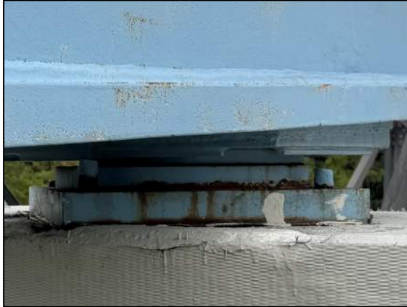
Photo 80: Pier 4 typical bearing condition (south bearing shown)
