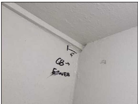
Photo 64: 4" fillet weld between the east web and top flange at Girder 8
