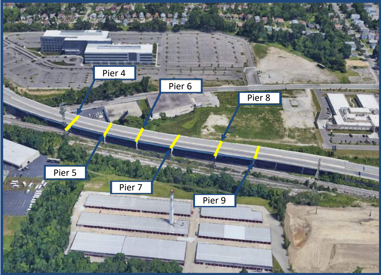
Figure 2: Fracture Critical Pier Cap Locations
