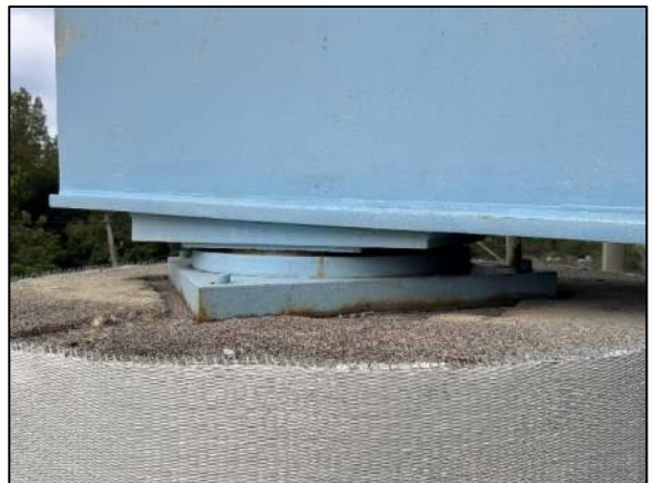
Photo 83: Pier 7 typical bearing condition (south bearing shown)
