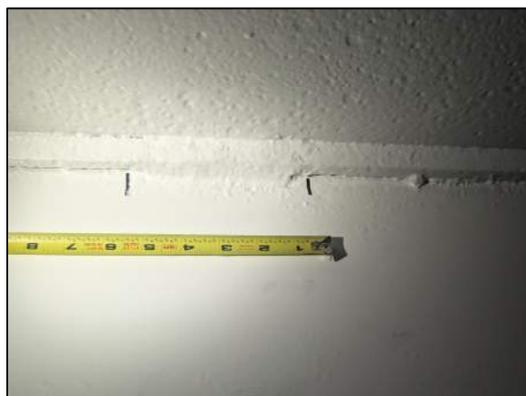
Photo 7: 5" fillet weld along backer bar between the top flange and east web plate between Girders 9 and 9A
