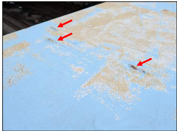
Photo 66: Fillet welds on the top flange at the southern end of the pier cap
