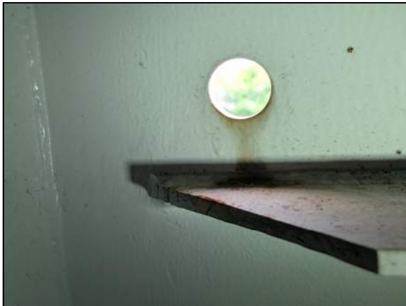
Photo 9: Crack arrest retrofit on the west web, south of Girder 10
