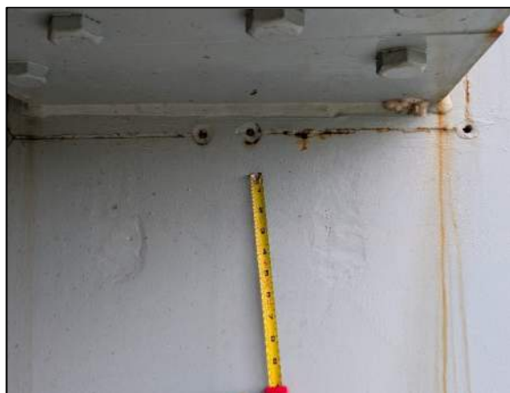
Photo 32: Typical overgrinding on web plate during girder knee brace removal (Girder 10 west web)
