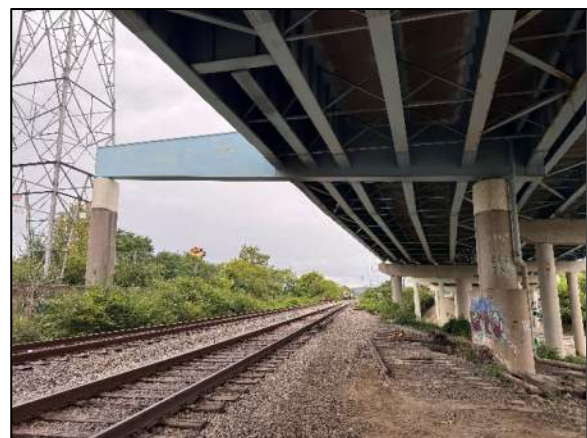
Photo 1: Elevation of Pier Cap 4
