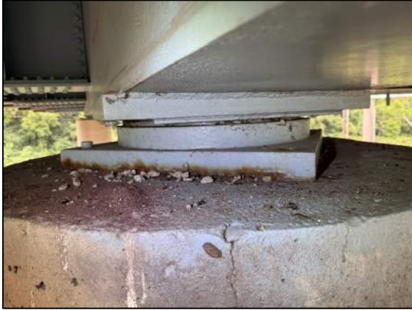
Photo 85: Pier 9 typical bearing condition (north bearing shown)
