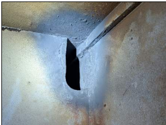
Photo 34: Typical view of upper corner retrofit between the diaphragms and web at Girder 6
