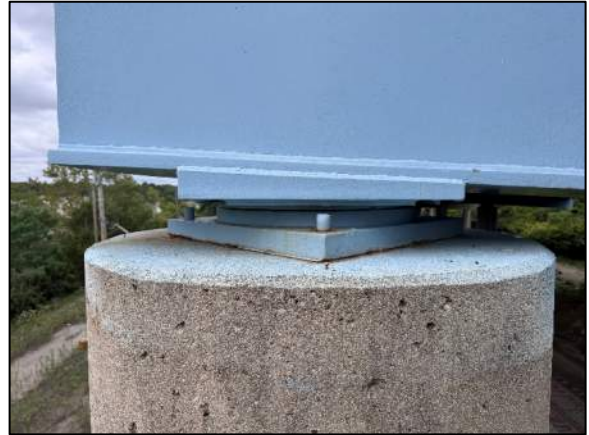
Photo 82: Pier 6 typical bearing condition (south bearing shown)
