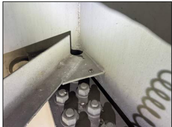
Photo 33: Typical lateral bracing cope detail at Pier Cap 16, fillet welds not completely removed
