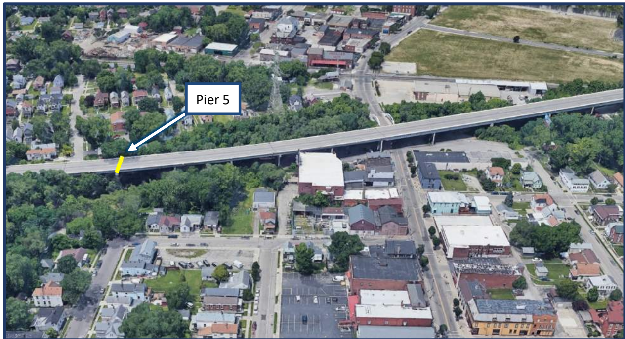
Figure 2: NSTM Pier Cap Location – Pier 5
