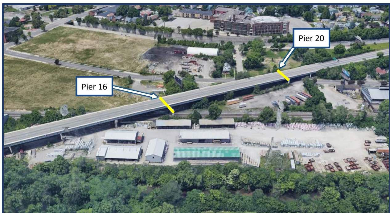
Figure 3: NSTM Pier Cap Location – Pier 16 & Pier 20
