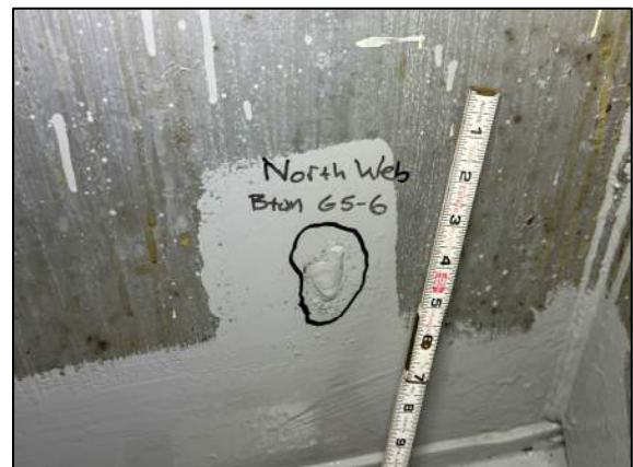
Photo 9: 2" x 1" plug weld on the north web of Pier Cap 5, between Girder 5 and Girder 6
