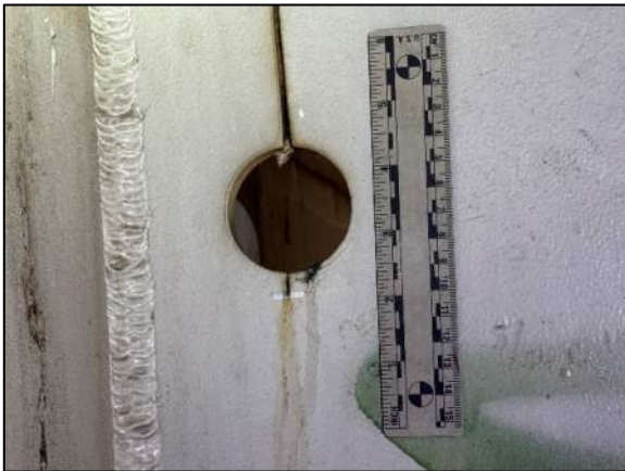
Photo 31: Sawcut retrofit extending 5/16" past the stress relief hole on Girder 3 at the north web of Pier Cap 16
