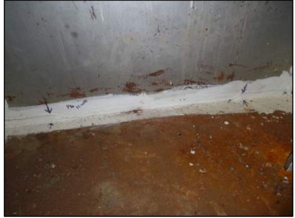
Photo 22: Typical bottom flange backer bar retrofit of Pier Cap 16
