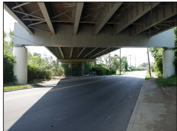
Photo 36: Elevation of Pier Cap 20
