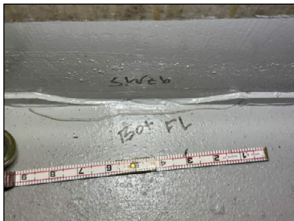
Photo 3: Typical Bottom Flange backer bar retrofit of Pier Cap 5, east of Girder 2
