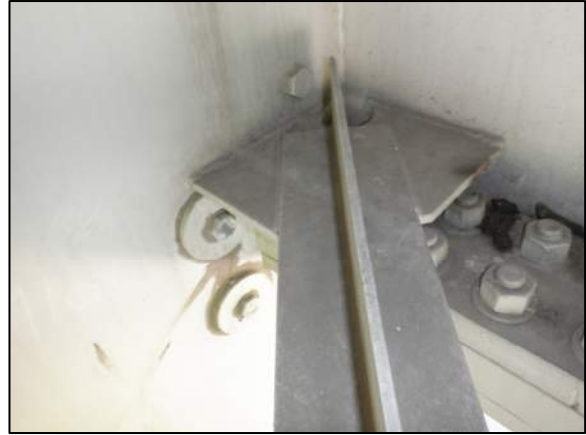
Photo 50: Typical lateral bracing cope detail at Pier Cap 20, fillet welds not completely removed
