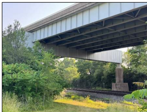
Photo 17: Elevation of Pier Cap 16
