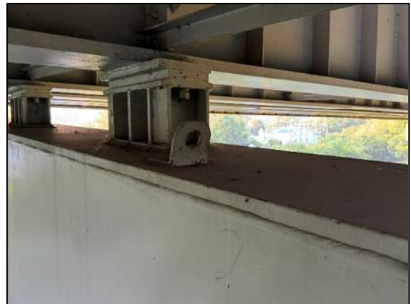
Photo 12: Lifting angle welded in place on top of Pier Cap 5 at Girder 2
