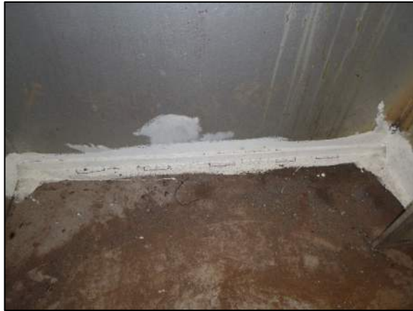
Photo 39: Partially ground fillet welds from the bottom flange backer bar retrofit at Pier Cap 20
