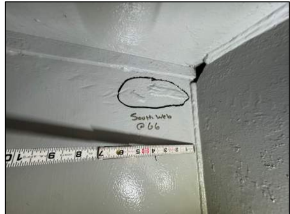
Photo 8: 3" x 1" plug weld on the south web of Pier Cap 5, east of Girder 6
