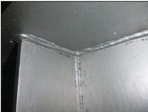
Photo 40: Typical triaxial welds at the girder bottom flanges and Pier Cap 20 diaphragms
