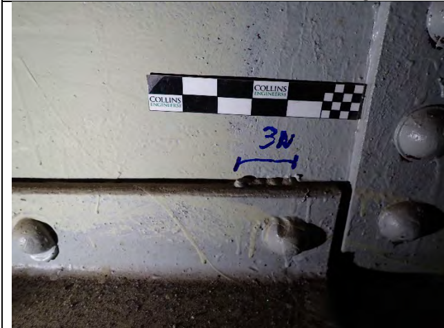
Photograph 9 – View of 1-1/2 in. and 2-1/2 in. Tack Welds On The Cap Top Flange Plate at the East Cap Web at the North Side of Girder 1. Looking east.
