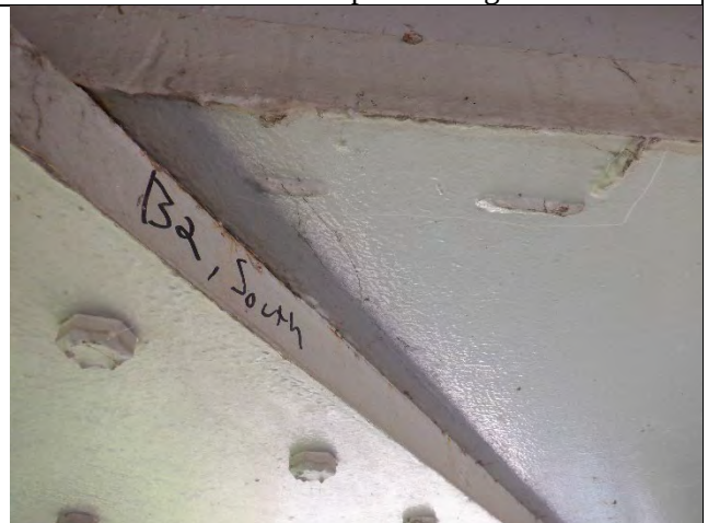
Photograph 15 – View of 3 Tack Welds Present on the West Side of the Cap Bottom Flange Between Girders 2 and 3. Looking East.
