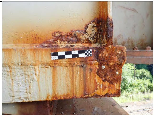
Photograph 13 – View of Laminating Corrosion on the South End of the Cap, Lower East Corner, With Isolated Pits to 1/8 in. Deep. Looking North.
