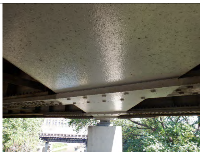
Photograph 1 – View of Pier Cap 5N. Looking north.
