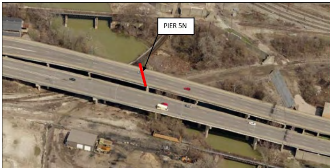
Figure 2: Fracture Critical Pier Cap Location
