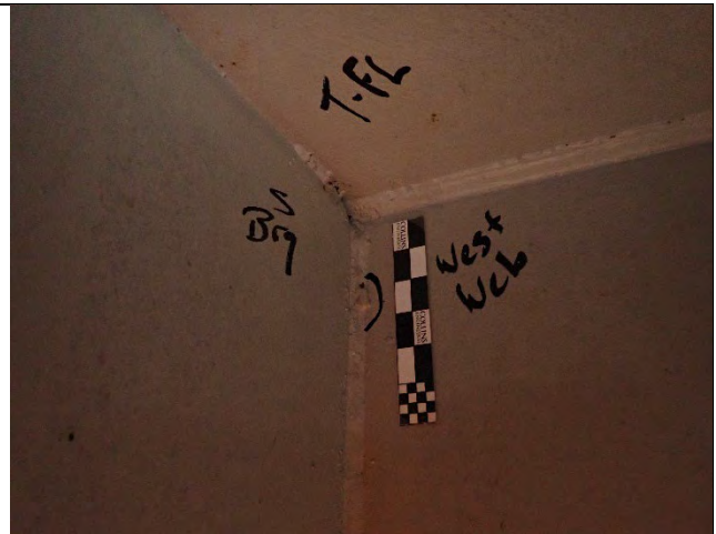
Photograph 10 – View of Tack Weld Located At the South Bearing Stiffener, West Cap Web Plate. Looking Southwest.
