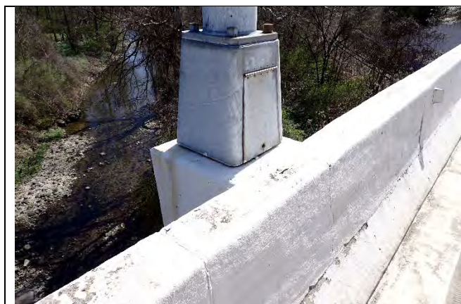
Photograph 41: Typical bridge light, looking southwest.
