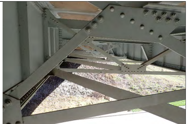
Photograph 12: Typical girder configuration, looking east.
