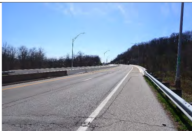
Photograph 2: General endview, looking west.
