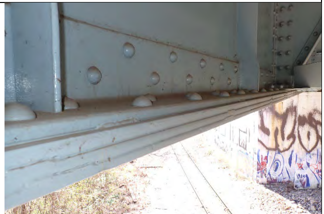
Photograph 14: Typical example of tack welds between bottom flanges and plates, looking south.
