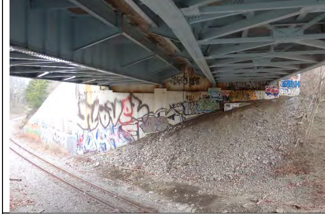
Photograph 26: Overall view of Rear Abutment, looking west.
