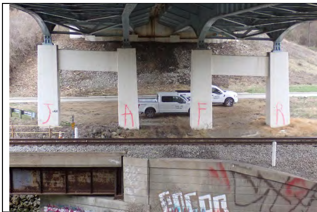
Photograph 23: Typical pier configuration (Pier 2 shown), looking east.
