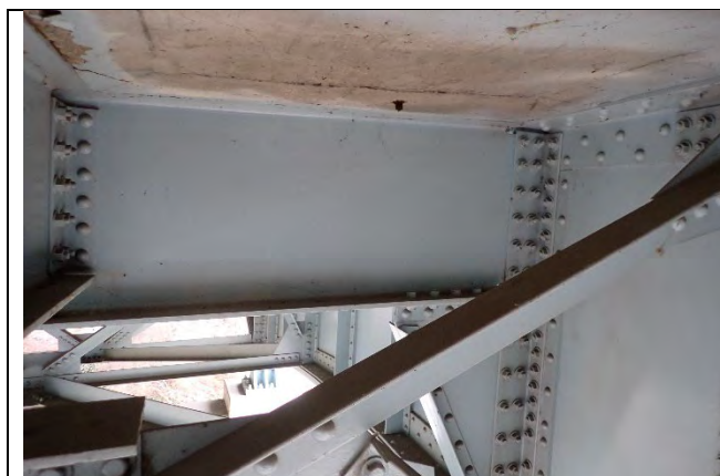
Photograph 18: Typical floor beam and floor beam connection condition in Span 3 near Floor Beam 1 shown, looking west. Note: no major defects.
