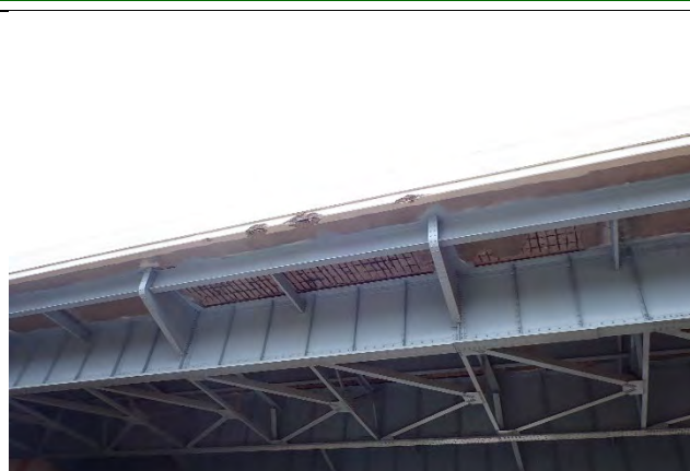
Photograph 6: Typical exterior deck condition, looking south.
