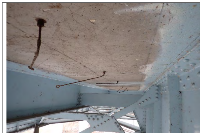
Photograph 3: Typical Span 2 soffit, looking west.
