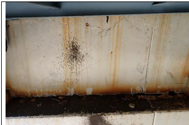
Photograph 39: Rear Abutment backwall, typical, looking west.
