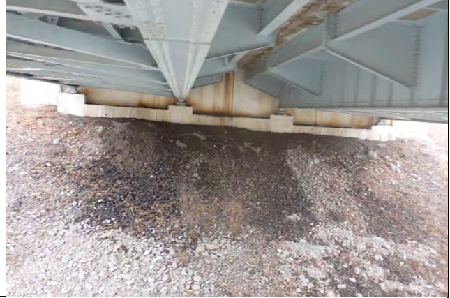
Photograph 27: Overall view of Forward Abutment, looking east.
