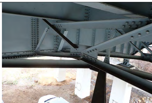
Photograph 19: Typical floor system steel and paint condition (Span 3 near Floor Beam 1 shown), looking southwest. Note: no major defects.
