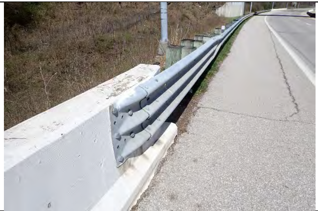
Photograph 32: Typical approach rail transition configuration, looking northeast.
