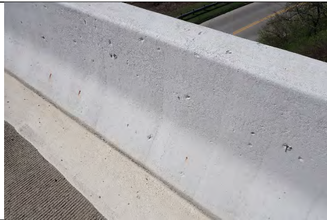
Photograph 31: Typical rail configuration, north rail in Span 3 westbound shown, looking northwest.
