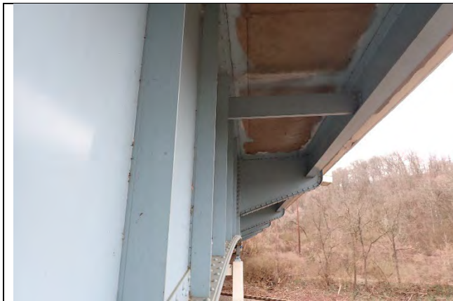
Photograph 11: Typical exterior floor beam cantilever configuration and condition (Span 2 north exterior shown), looking west.
