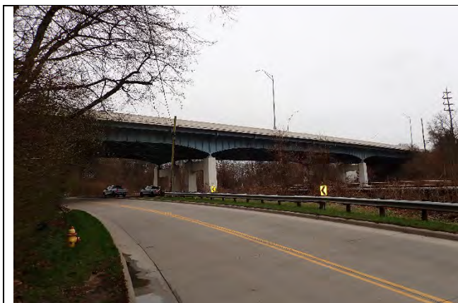
Photograph 1: General elevation, looking southwest.
