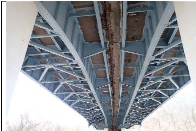
Photograph 15: General view of the superstructure, looking east.
