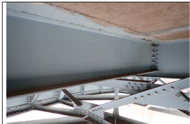
Photograph 17: Typical stringer condition (Span 3 near Floor Beam 1 shown), looking southwest.
