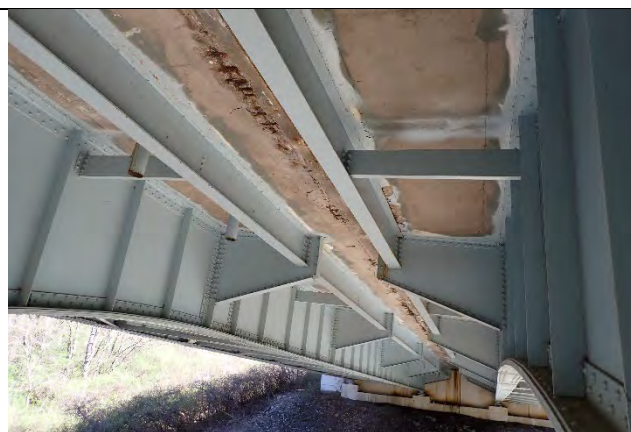
Photograph 4: Typical condition and configuration of the soffit between the two bridges from Pier 2, looking northeast.
