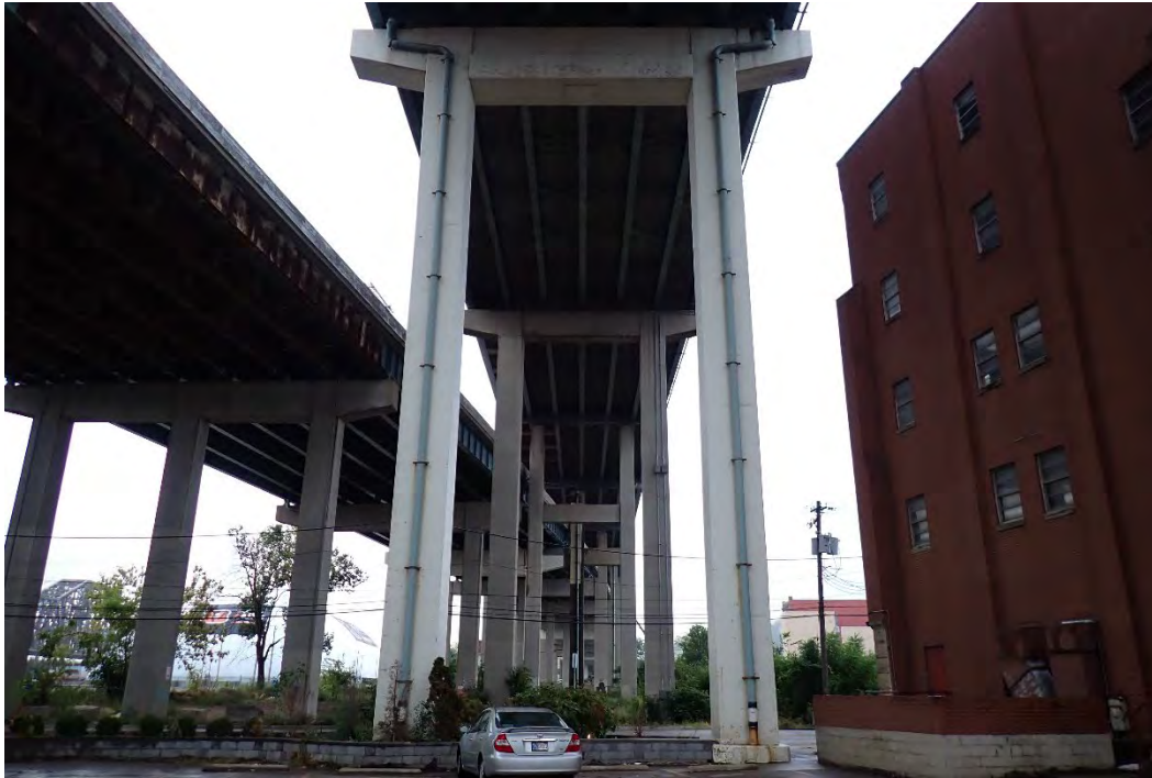
Photo 111 - Elevation of Pier 15A, looking south. Note: Pier columns wrapped in FRP, and deck drainpipes fastened to pier columns.
