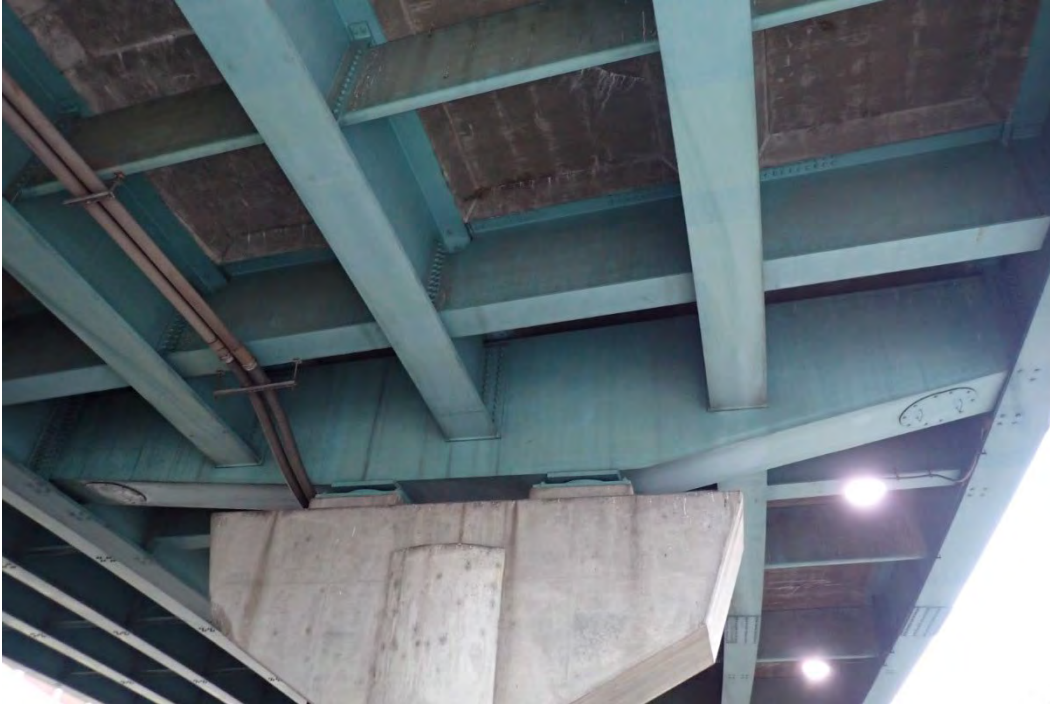
Photo 89 - East elevation of box cap at FWW Pier 2, looking west.
