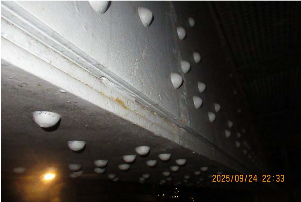
Photo 63 – Typical tack welds between the north edge of the bottom flange plate and the north bottom flange angle.
