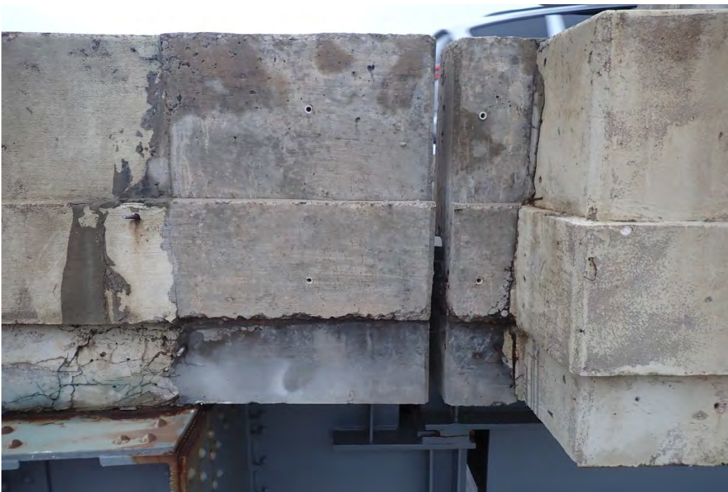
Photo 21 - Typical concrete bridge railing repair at a joint location at Pier 7A, looking east.
