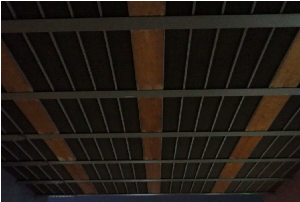
Photo 30 - Typical girder layout with debris screens between River Pier and Pier 13A, Span 1A looking east.
