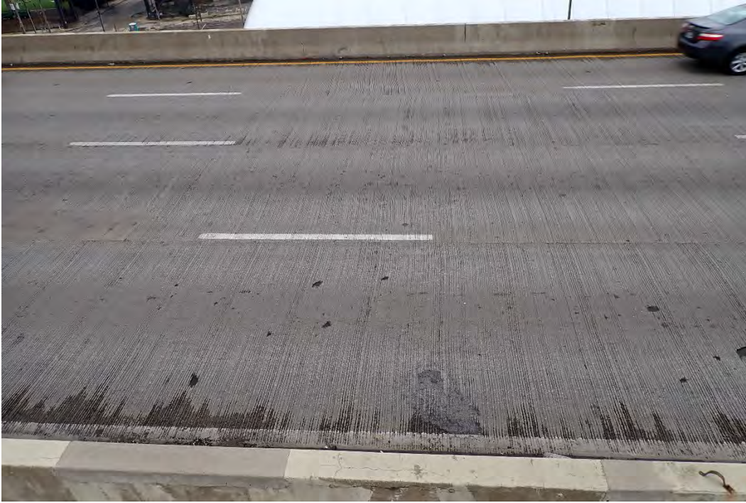
Photo 12 - Typical high-friction deck top at Span 5A, looking east. Note: Minor concrete popouts/ spalls in far west travel lane.
