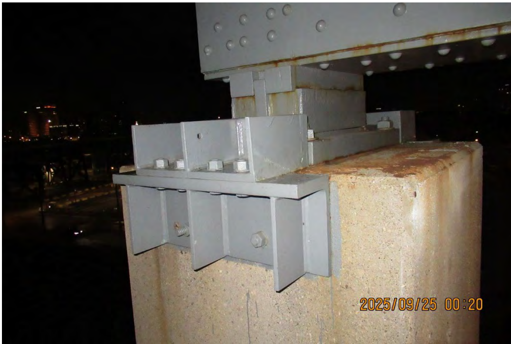
Photo 94 - Retrofit to east bearing sole plate of Pier 11A, looking east.
