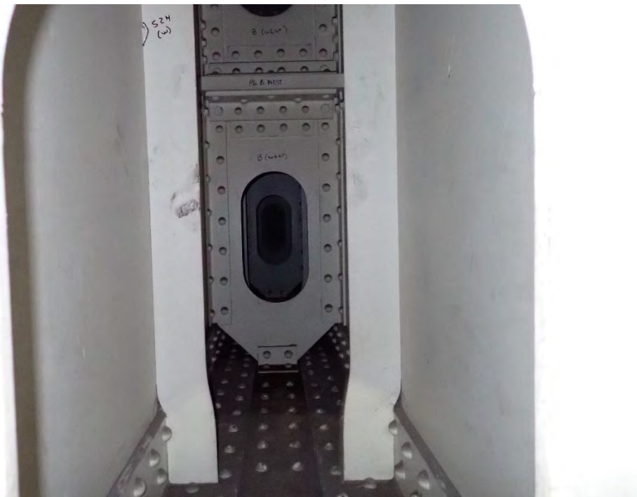
Photo 43 - Typical box cap interior view at Pier 6A, looking east.
