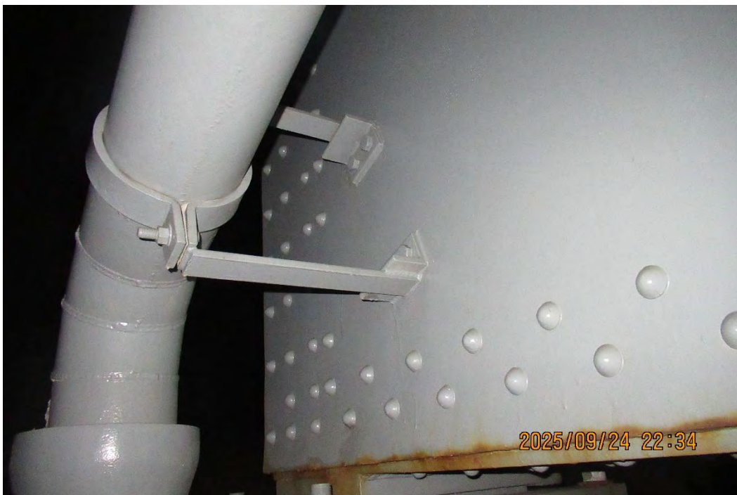
Photo 64 – Typical drainpipe support brackets attached to the north web with bolts.
