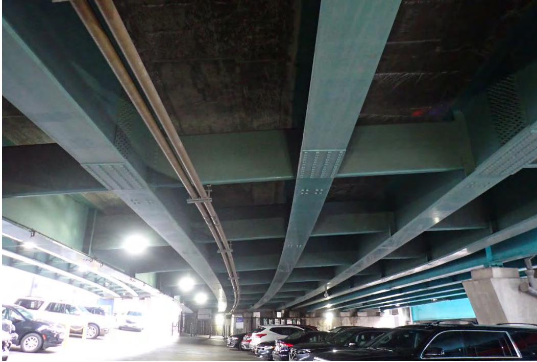
Photo 106 - Typical solid diaphragms at Span 1, looking east.
