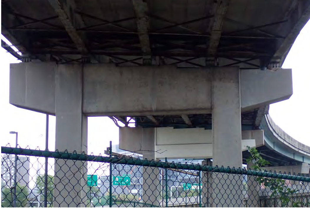
Photo 121 - Typical pier cap at Pier 27B, looking north.
