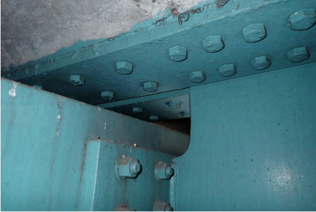
Photo 91 - Typical girder connection to FWW Pier 2 on west face, looking southwest.
