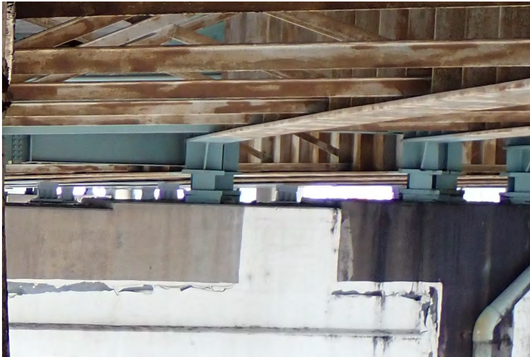
Photo 93 - Typical Elastomeric bearings on Pier 15A, looking south.
