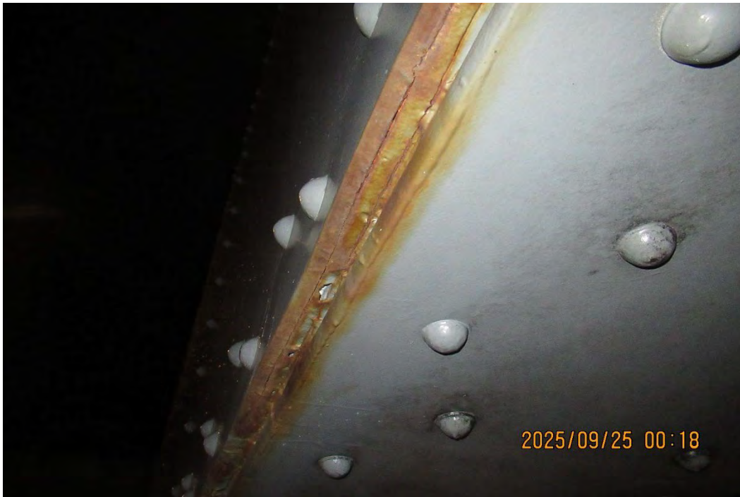
Photo 79 - Bottom flange angles that has been filled with steel putty and painted along the entire width of the pier cap.
