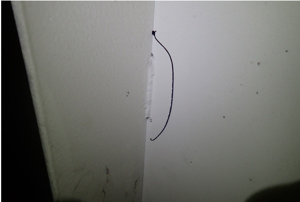
Photo 54 - Typical tack welds in box cap interior at Pier 3A.
