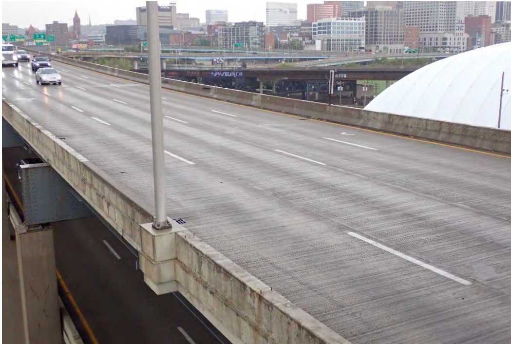
Photo 1 - Typical top of deck at Span 1A, looking northeast.
