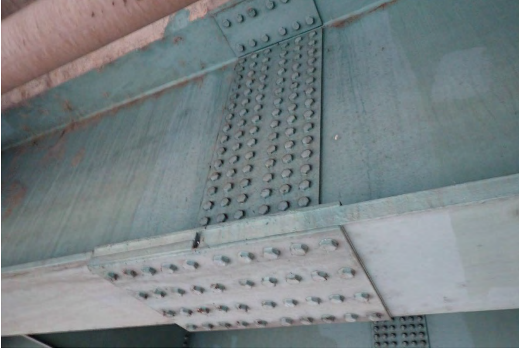
Photo 40 - Typical girder bolted connection at FWW Span 3, looking north.
