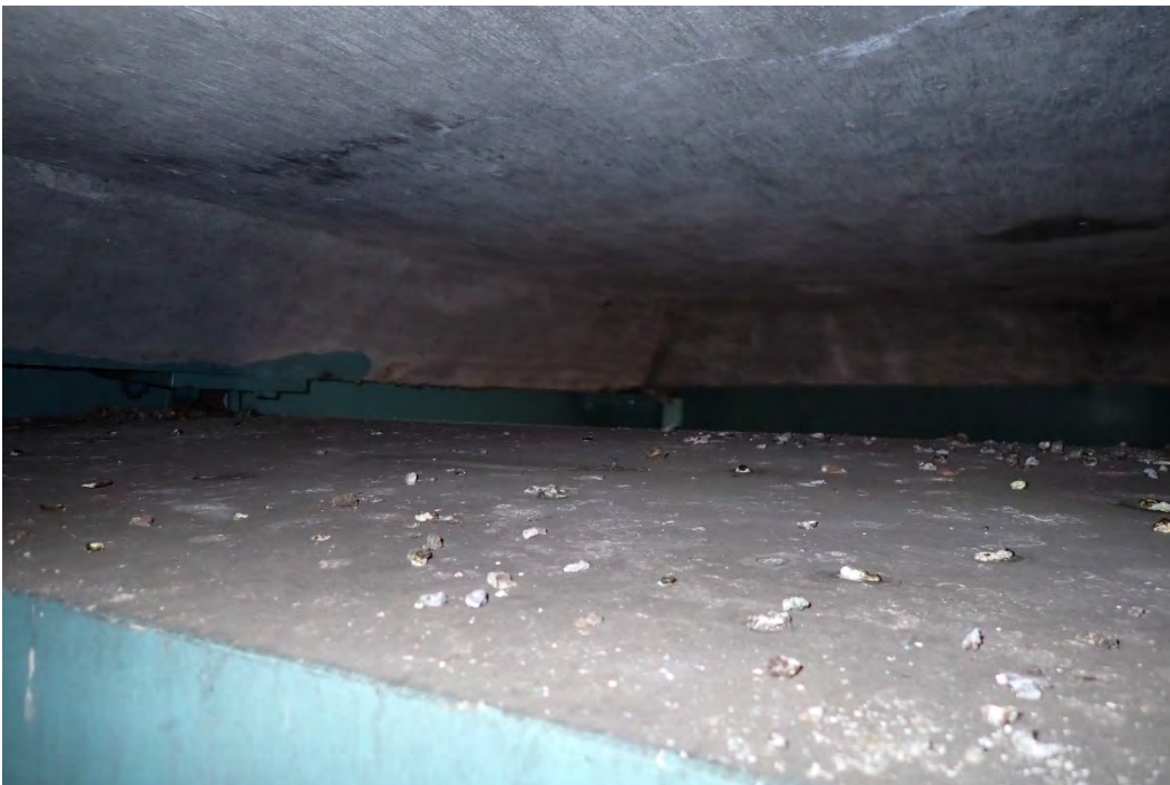
Photo 90 - Top side of top flange of box cap at FWW Pier 2, looking north.
