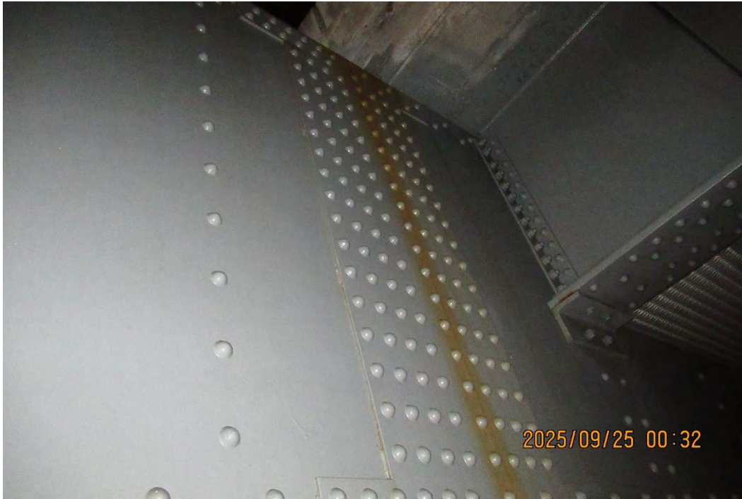
Photo 80 - Protective coating system on the exterior of the pier cap is in good condition at Pier 11A, looking north.
