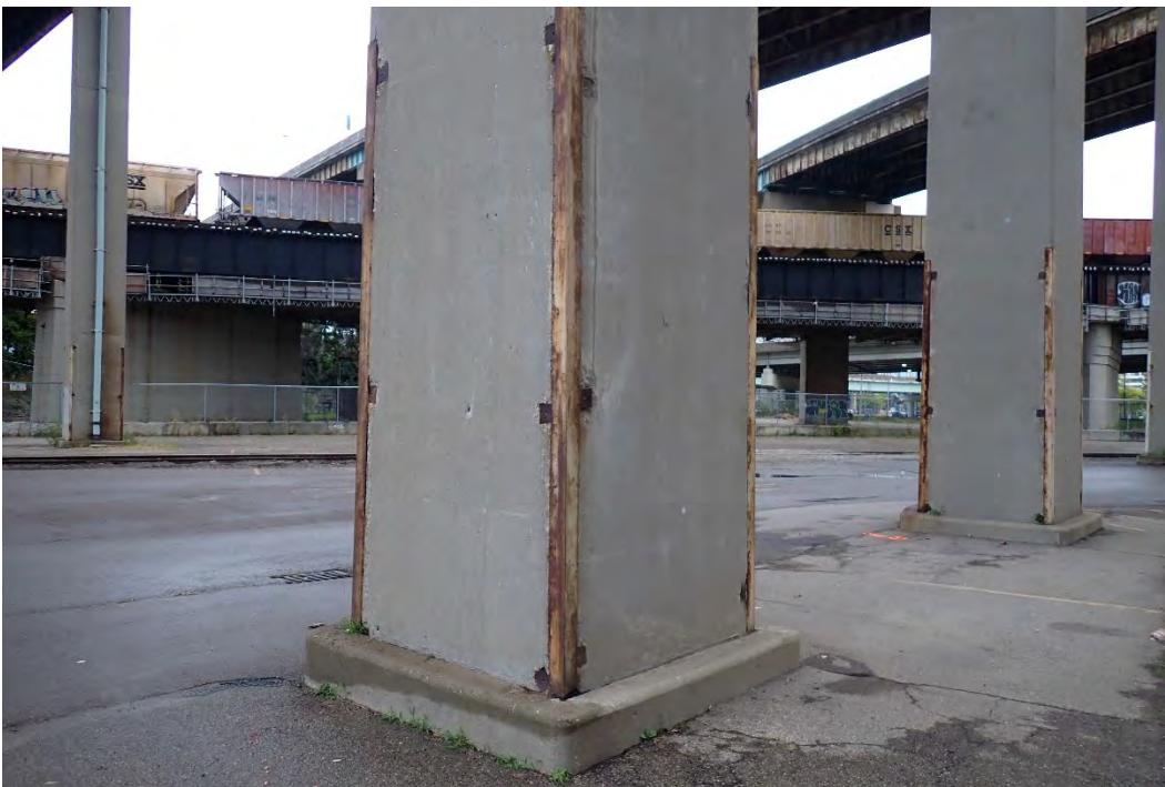
Photo 118 - Non-typical column corner armor at Pier 16A, looking northeast. Note: Armor is also present on Pier 17A.
