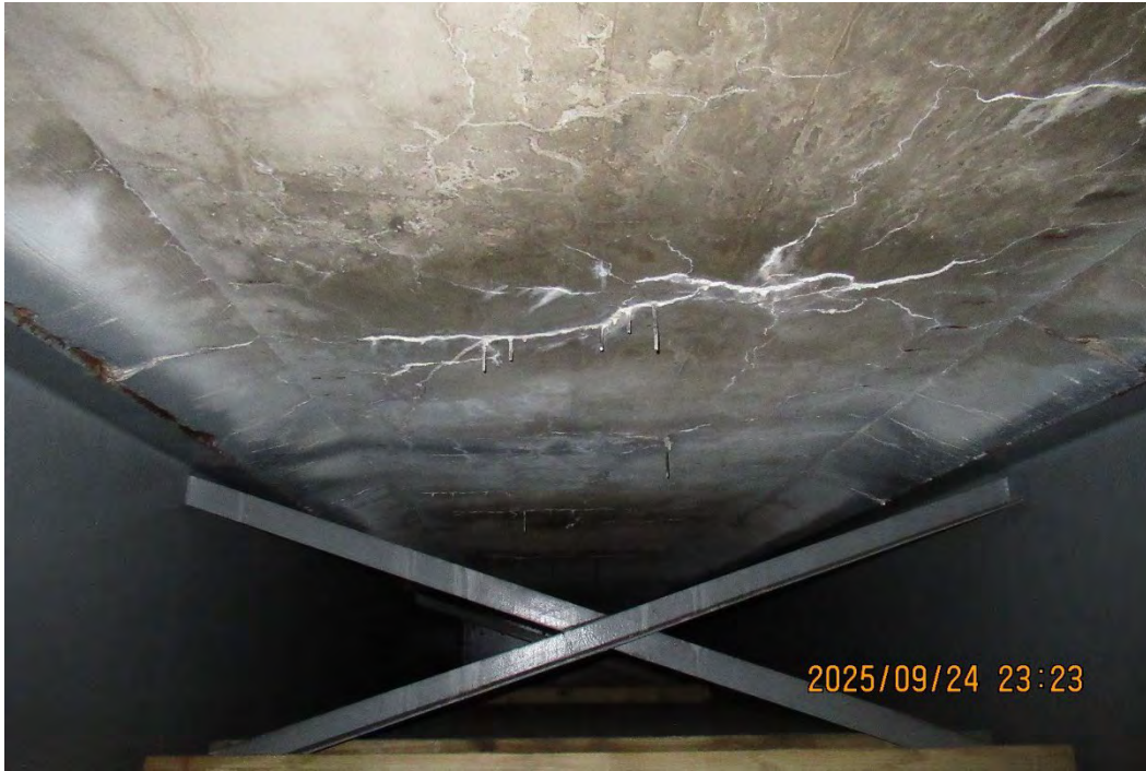
Photo 108 - Typical cross-frame diaphragm for spans between the River Pier and Pier 15A.
