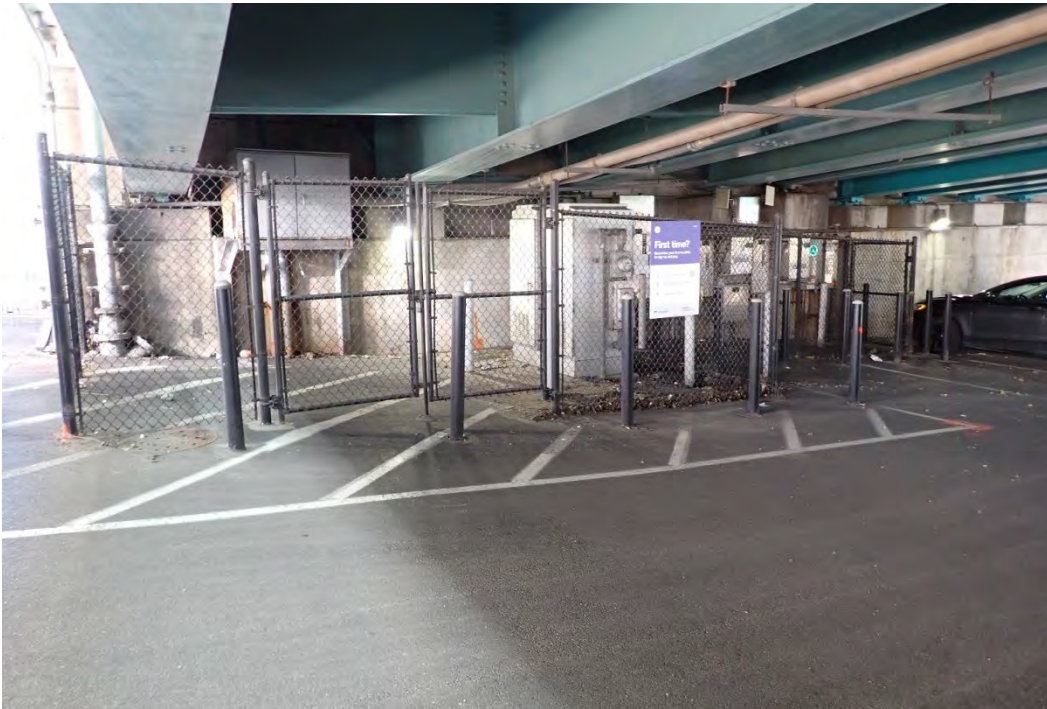
Photo 120 - FWW Wall Pier, looking East.
