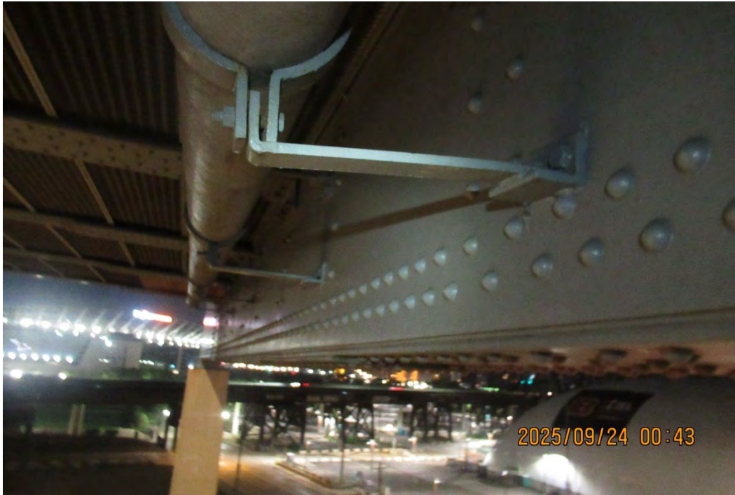
Photo 77 - Typical pipe connection bracket on the north face of Pier 10A, looking east.
