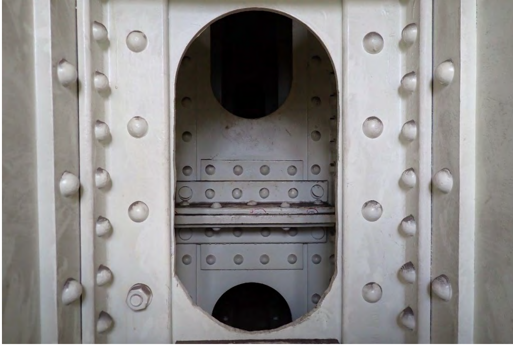
Photo 83 - Interior of the cap was dry with no signs of moisture intrusion at the time of the inspection.
