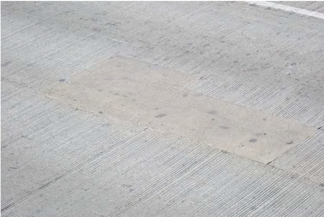
Photo 13 - Typical concrete deck repair at Span 5A, looking northeast.
