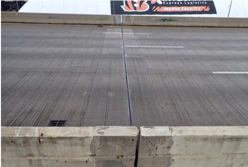
Photo 16 - Typical strip seal joint at Pier 4A, looking east.
