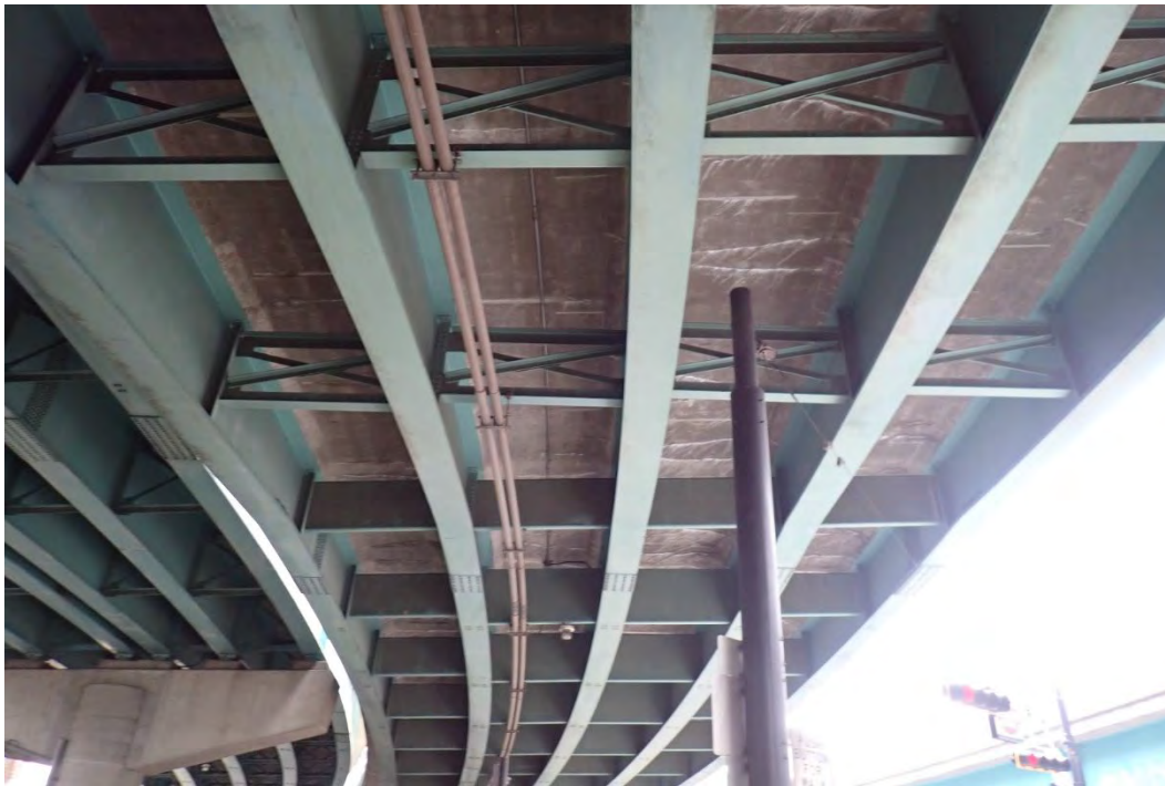
Photo 103 Typical protective coating condition of superstructure from Pier 28B to Wall Pier. Photo of FWW Span 3, looking east.
