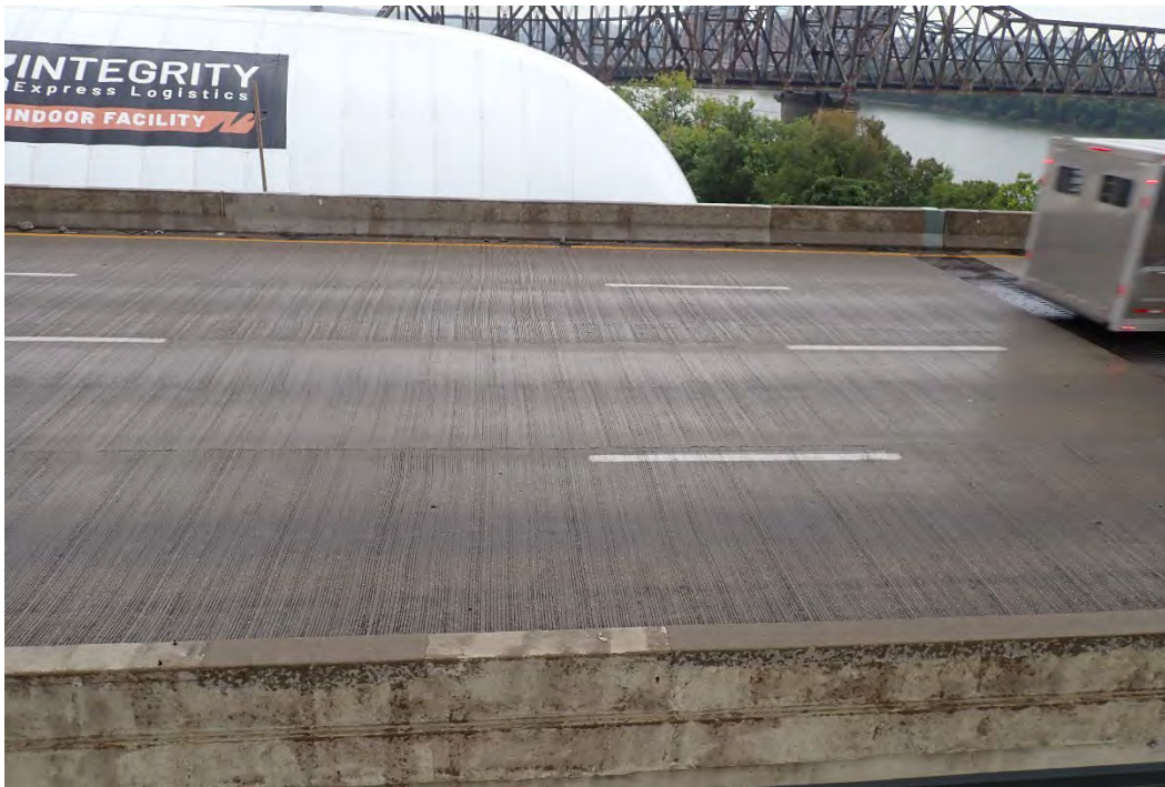
Photo 11 - Typical top of deck at Span 1A, looking east.
