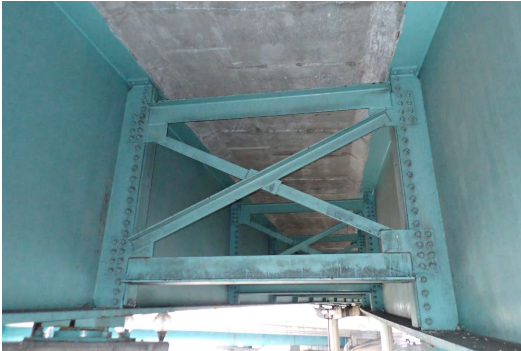
Photo 105 - Typical cross-frame diaphragm of FWW spans, at FWW Pier 3, looking west.
