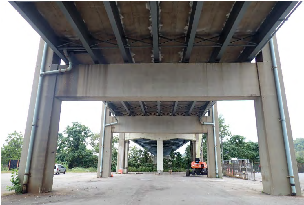
Photo 109 - Elevation of Pier 2A, looking south.
