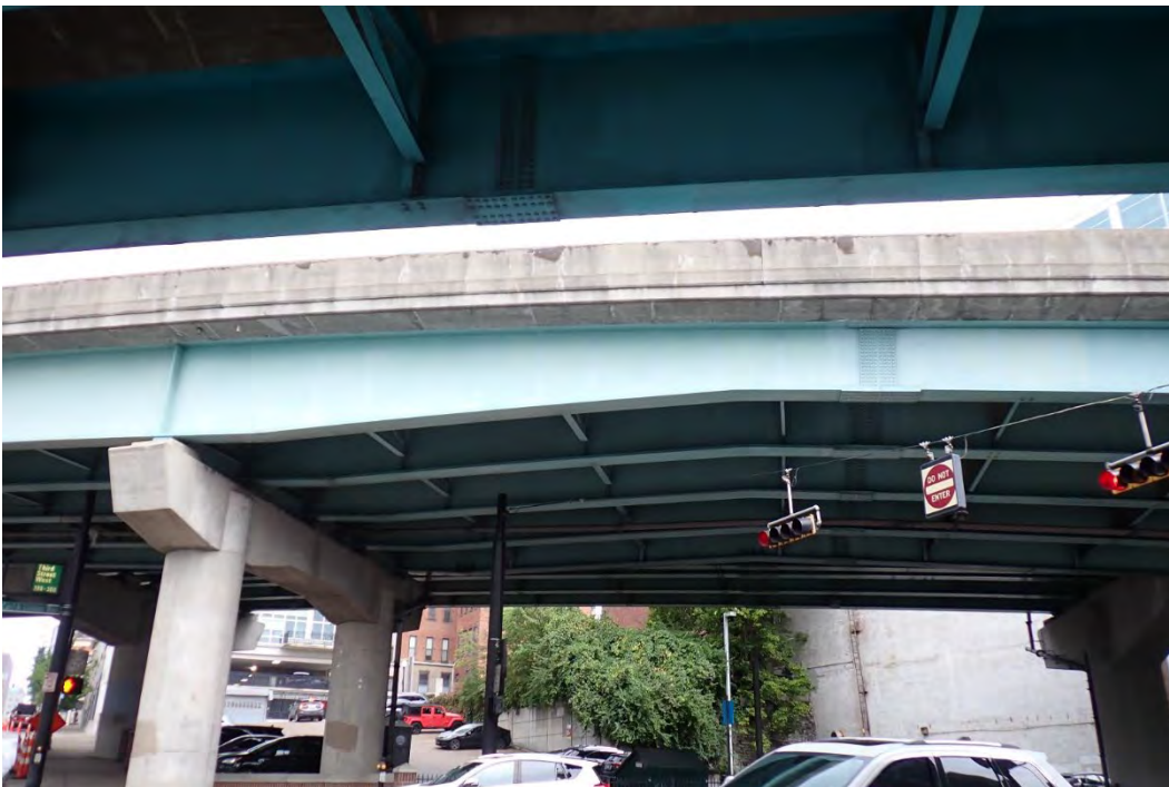
Photo 41 - Typical girder depth transition at FWW Span 4, looking north.
