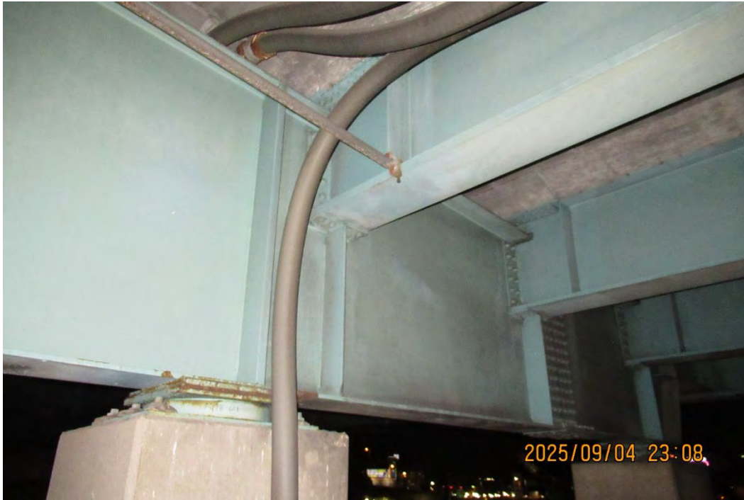
Photo 86 - West elevation of pier cap at Pier 29B.
