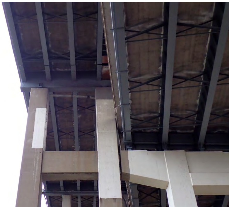
Photo 112 - Typical FRP application on Pier 12A, looking north.
