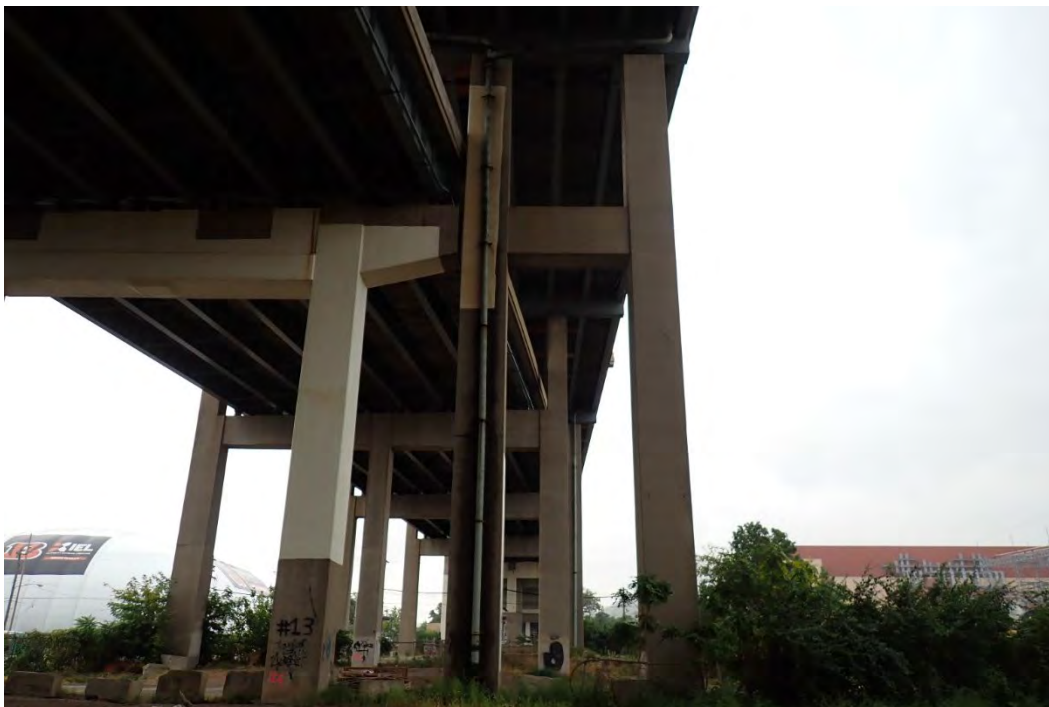
Photo 110 - Elevation of Pier 12A, looking south.
