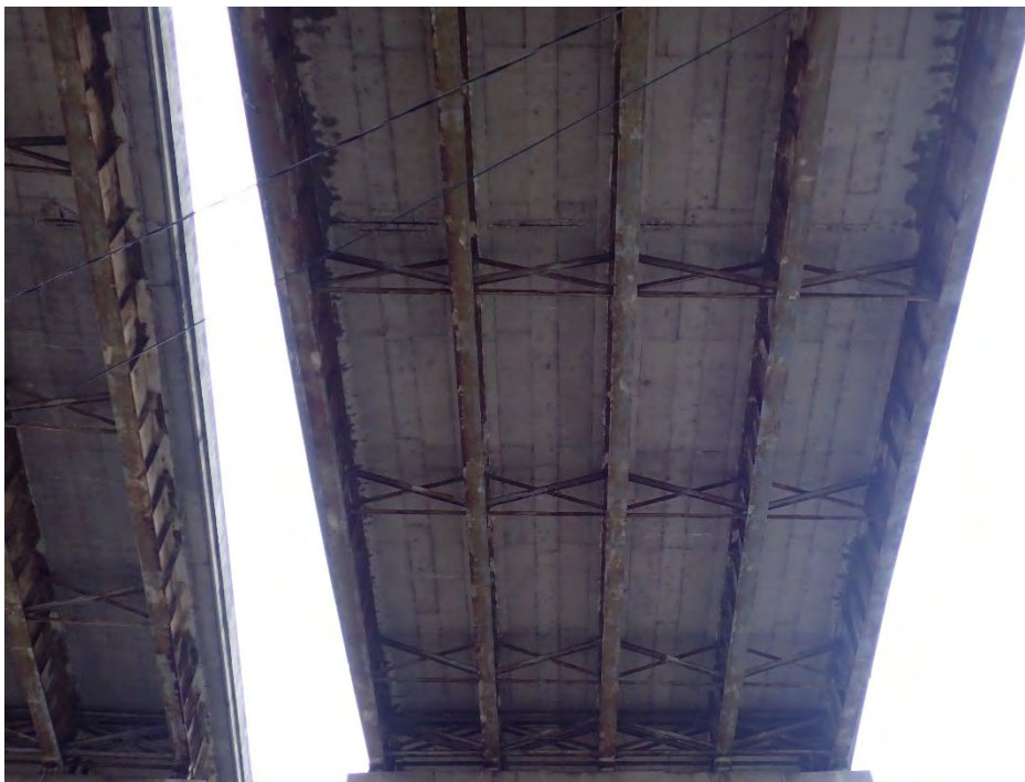
Photo 107 - Typical cross frame layout in Span 21B, looking north.
