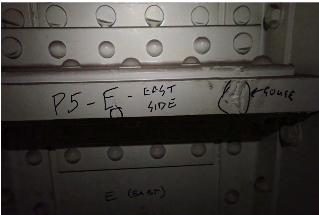
Photo 62 - Interior box cap coating in good condition at East end of Pier 5A.
