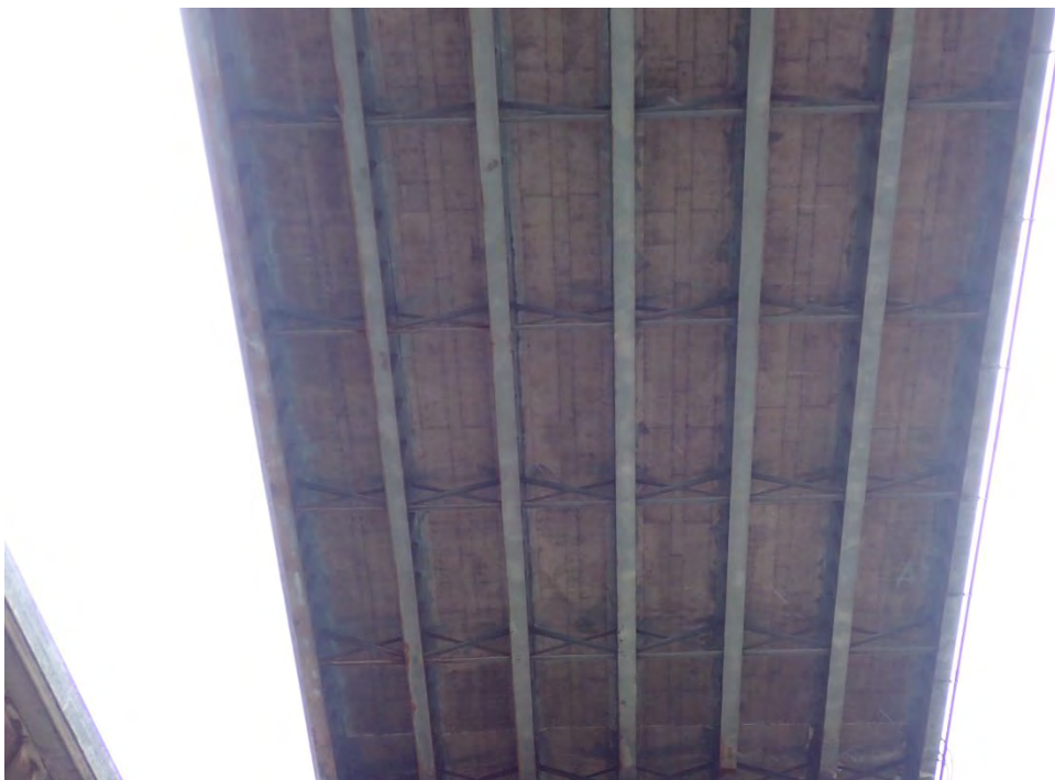
Photo 2 - Typical deck underside at Span 15A, looking south.
