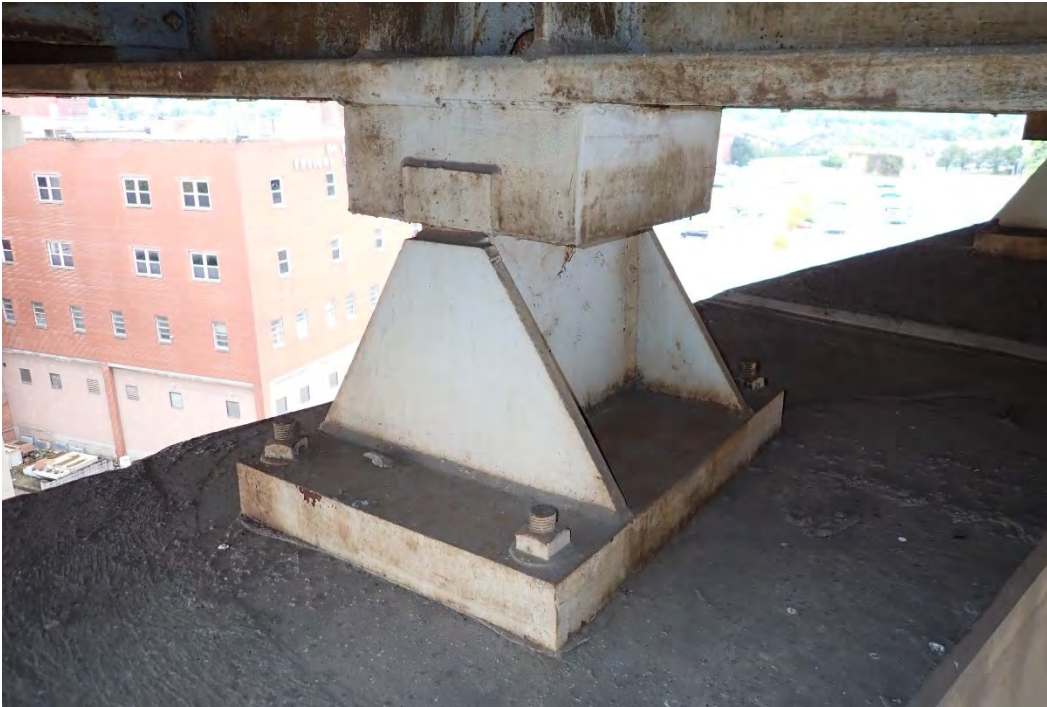
Photo 97 - Typical fixed bearing at Pier 17A, looking east.
