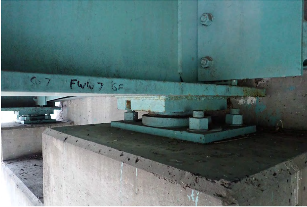
Photo 98 - Typical pot bearing at FWW Pier 7, looking southwest.
