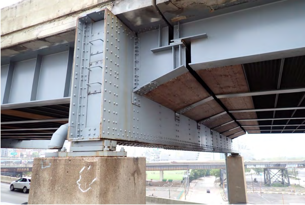
Photo 42 - Typical box cap elevation view at Pier 8A, looking northeast.
