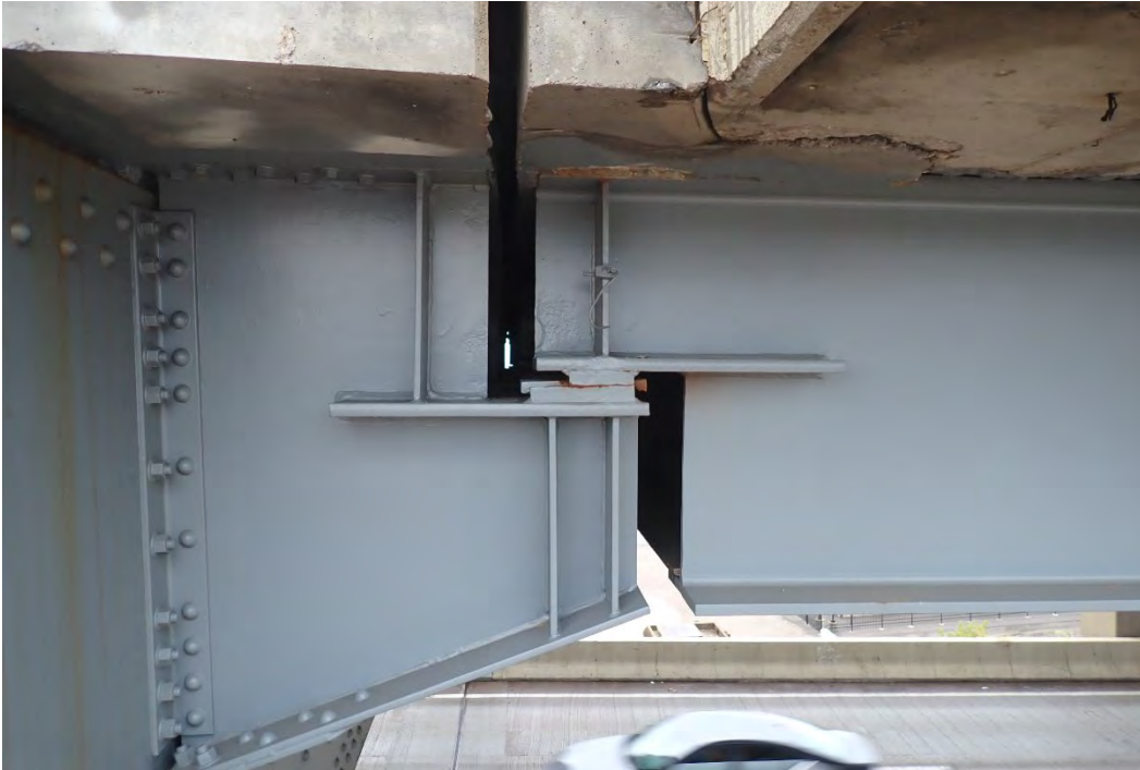
Photo 104 - Typical girder seat assembly detail at Pier 7A, looking east.
