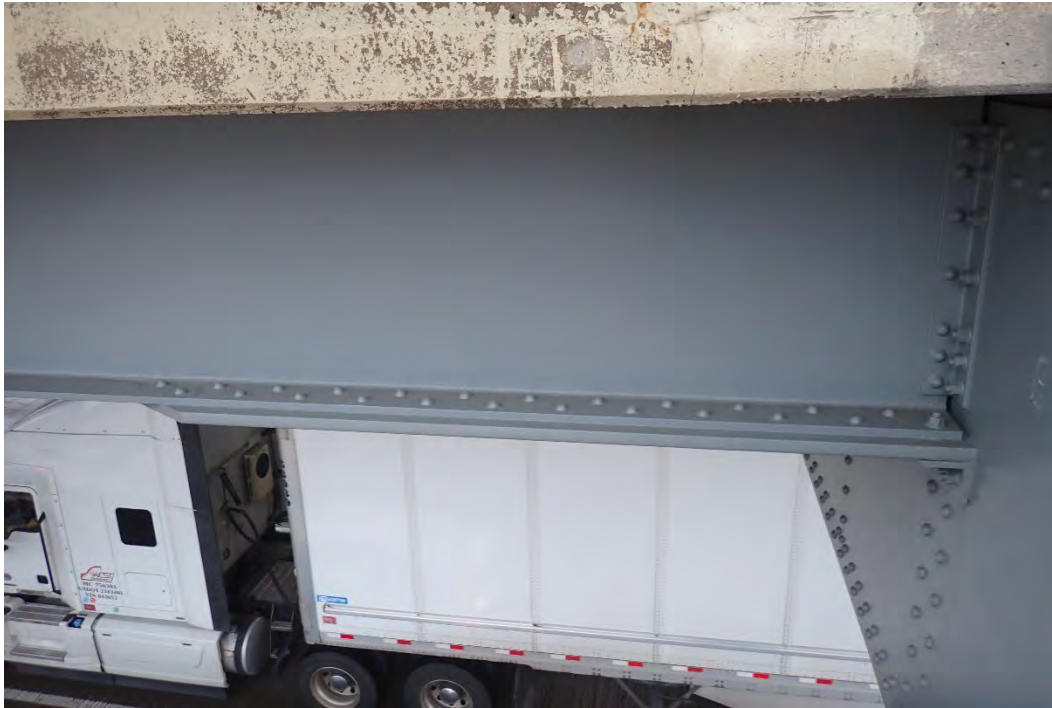
Photo 100 - Typical girder protective coating in good condition overall, from River Pier to Pier 15A. Photo of Pier 7A, looking east.
