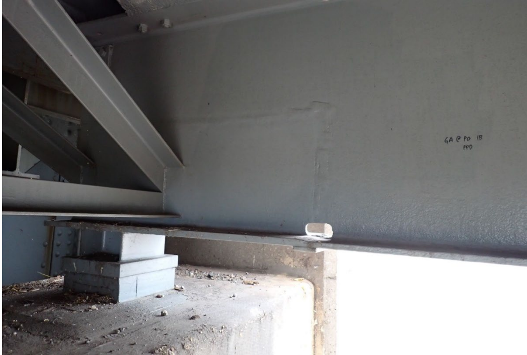
Photo 36 - Welded retrofit web and bottom flange replacement on Girder A over the River Pier, looking west.
