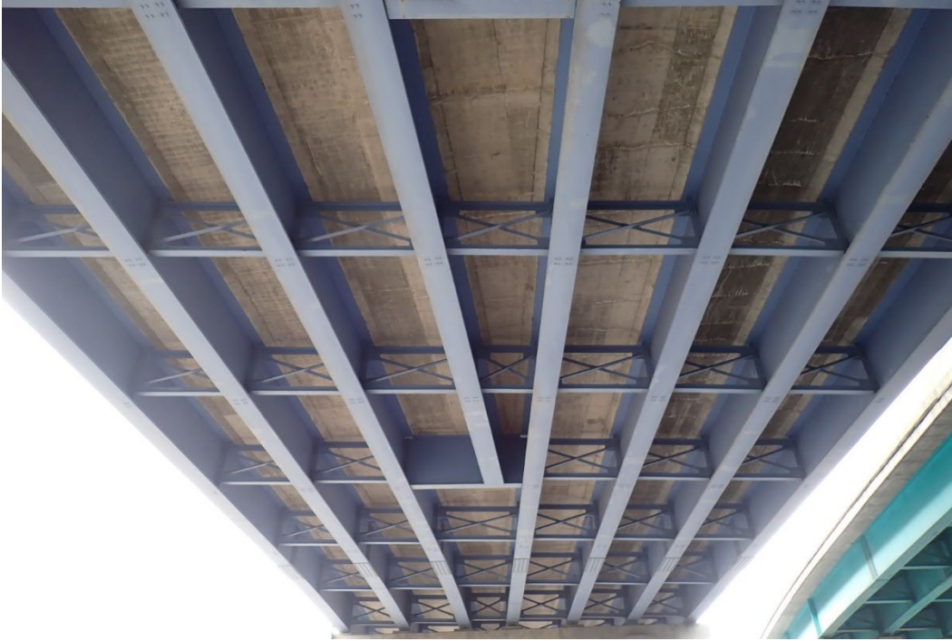
Photo 52 - Typical cross frame and diaphragm layout on the underside of Span 5, looking west.
