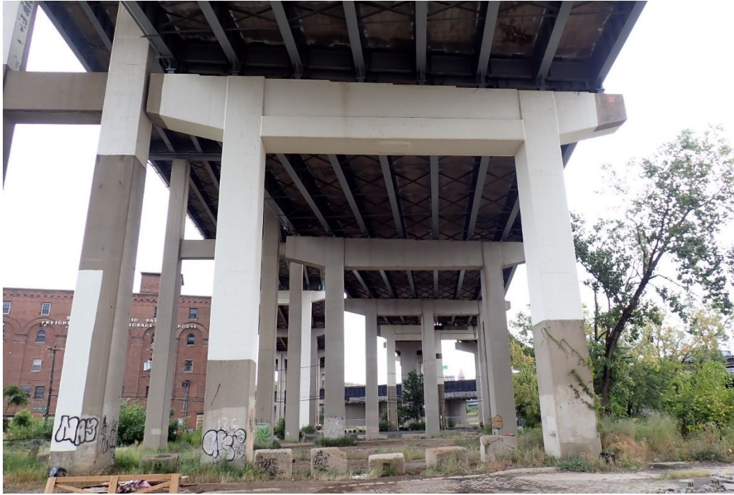
Photo 68 - Typical FRP wrap of pier cap and columns, at Pier 12C, looking north.
