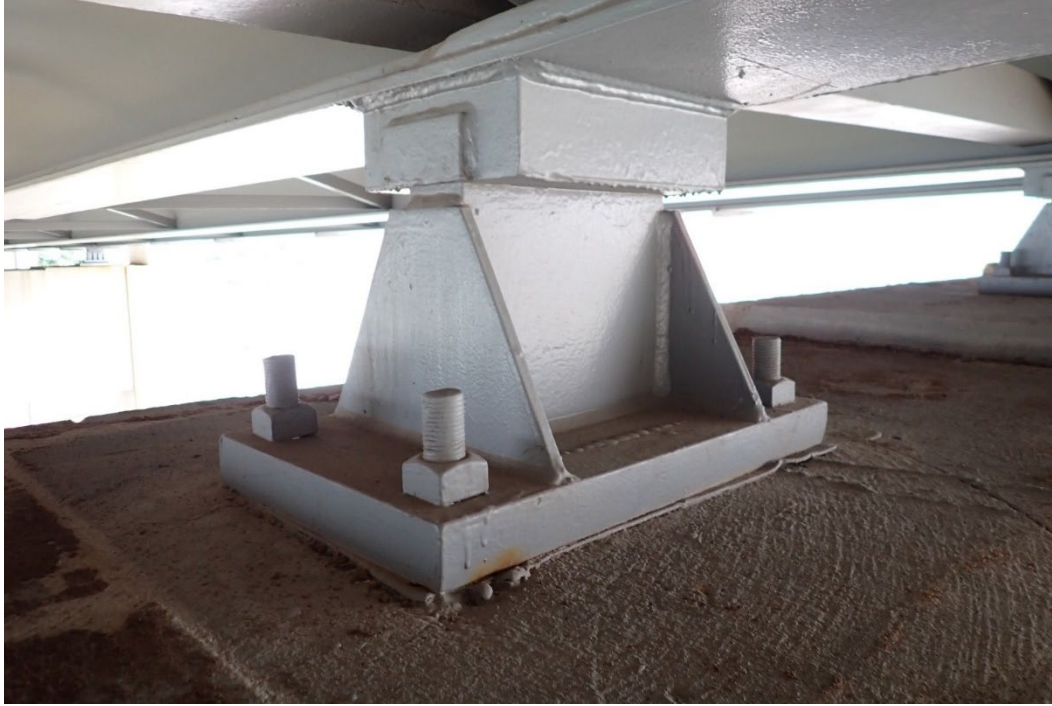
Photo 47 - Typical fixed bearing at Girder C of Pier 6A, looking southwest.
