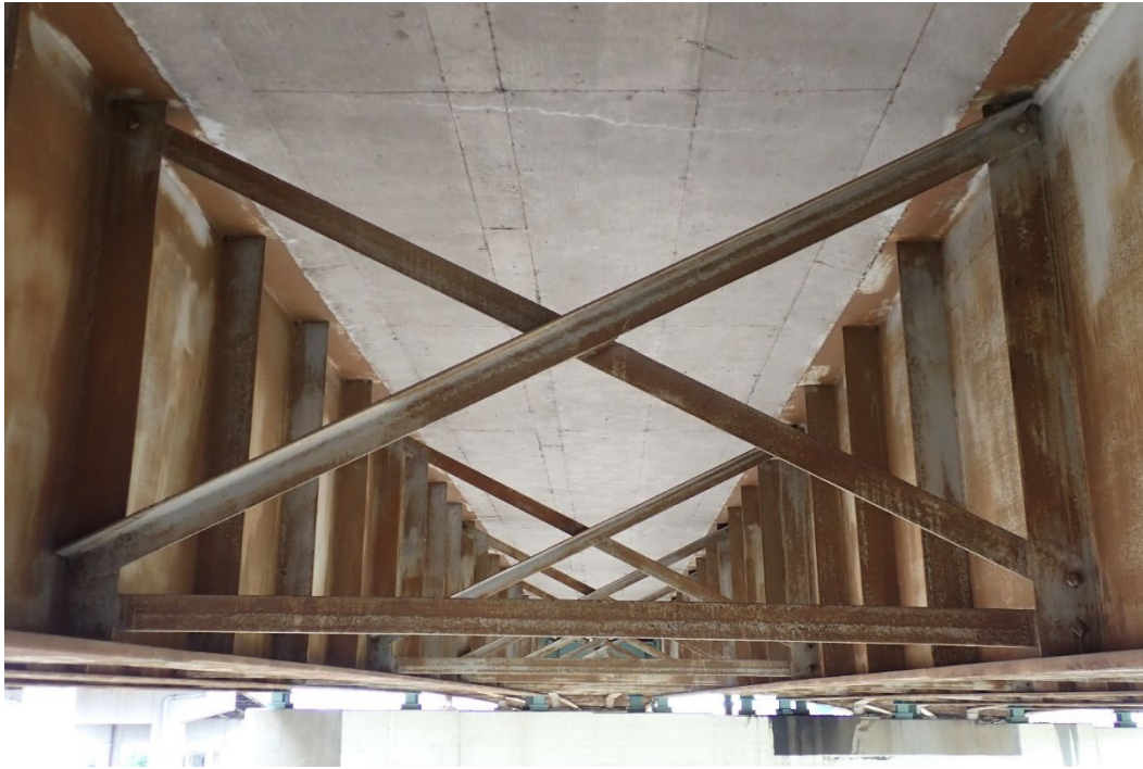
Photo 53 - Typical cross brace diaphragm at Span 15C, Bay 3, looking north.
