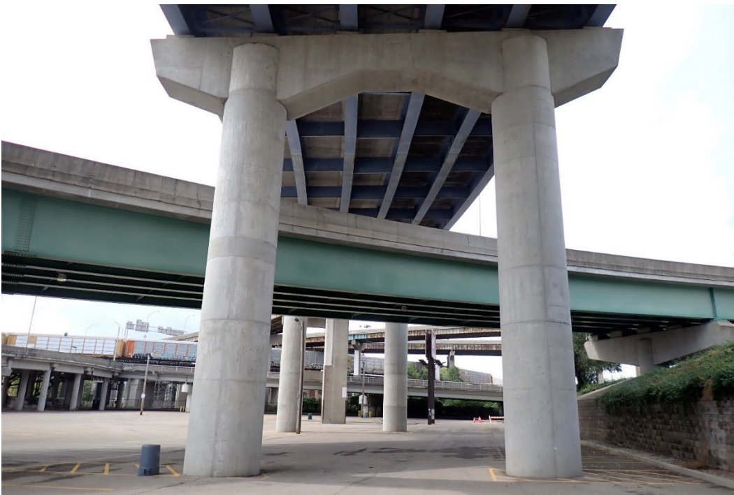
Photo 59 - Typical concrete pier elevation at Pier 2, looking west.
