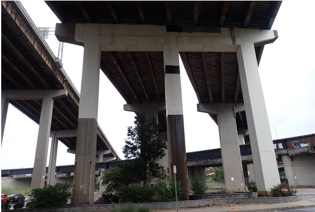
Photo 60 - Typical FRP wrap on Pier 15C, looking north.
