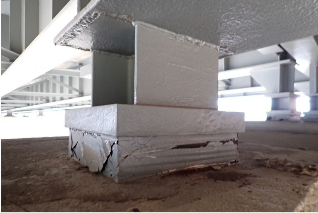
Photo 41 - Typical bearing pad at Girder D in Pier 12C, looking southwest.
