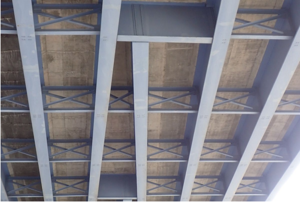
Photo 51 - Typical coating condition for Spans 1 to 5 is in good condition at Span 5, looking east.
