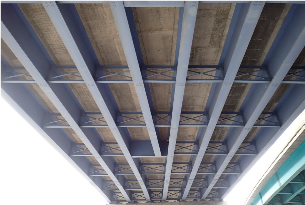
Photo 39 - Typical reconfigured span in good condition at Span 5, looking east.
