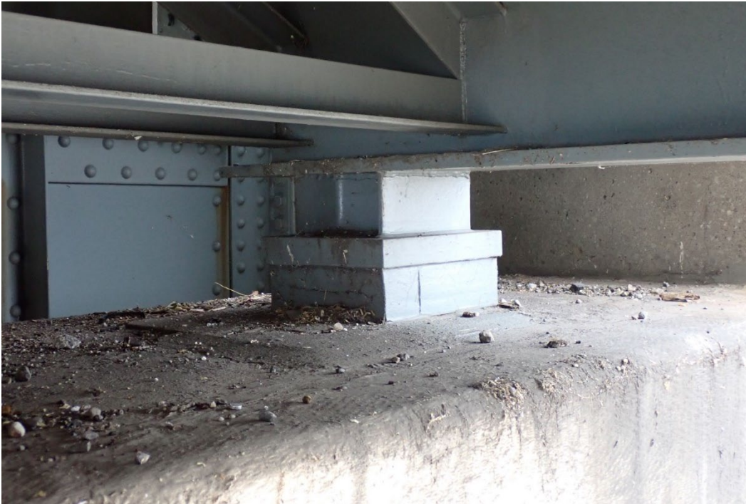
Photo 40 - Typical elastomeric bearing at River Pier, looking west.
