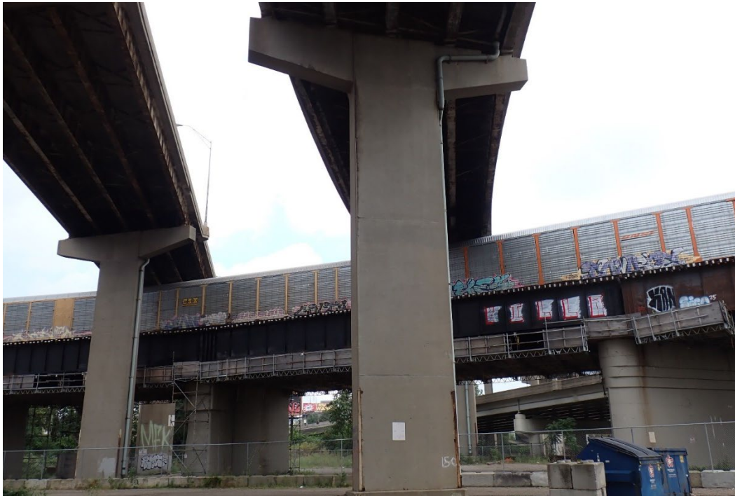
Photo 62 - Typical Elevation View of hammerhead pier at Pier 16D, looking north.
