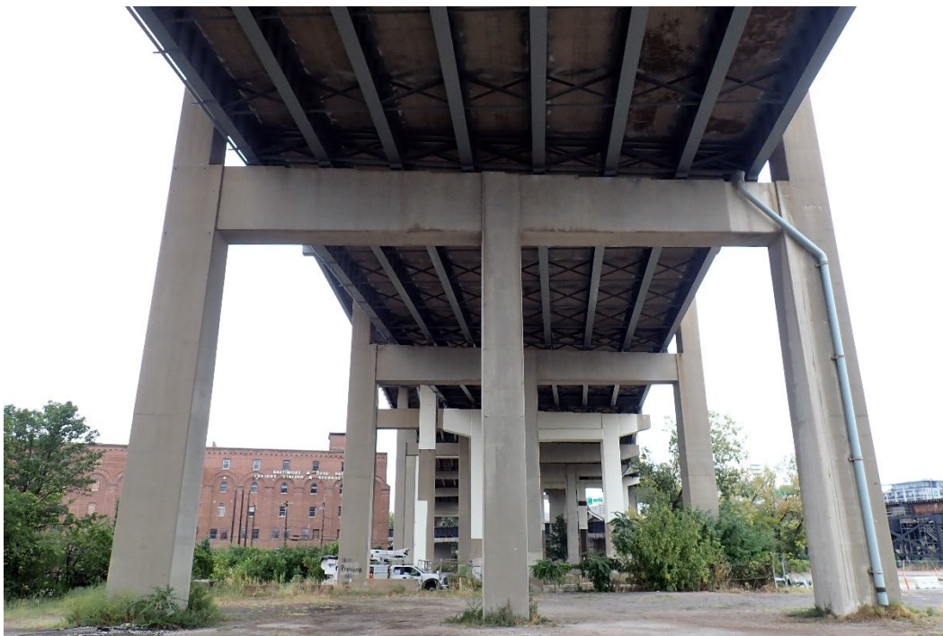
Photo 55 - Typical three-column Pier at Pier 10A, looking north.
