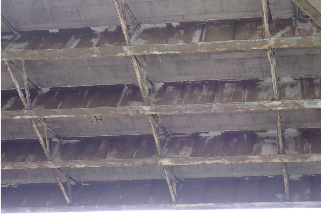
Photo 34 - Typical girder condition for Spans 15C to 20D, at Span 18D, looking north.
