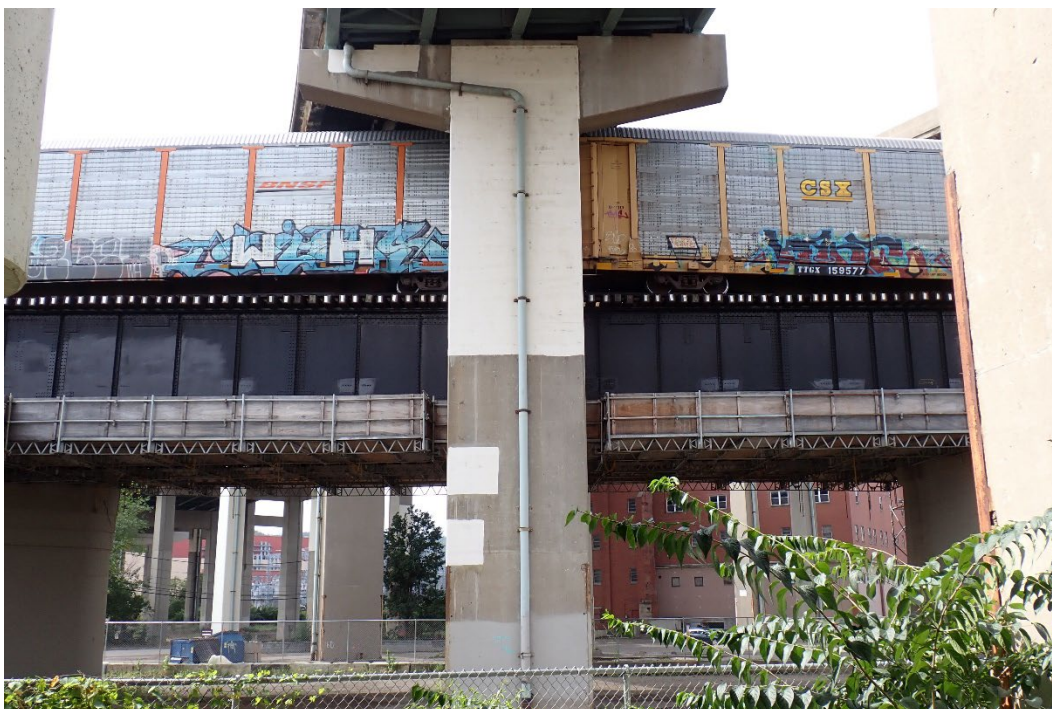
Photo 64 - Typical FRP wrap on pier wall at Pier 17D, looking south.
