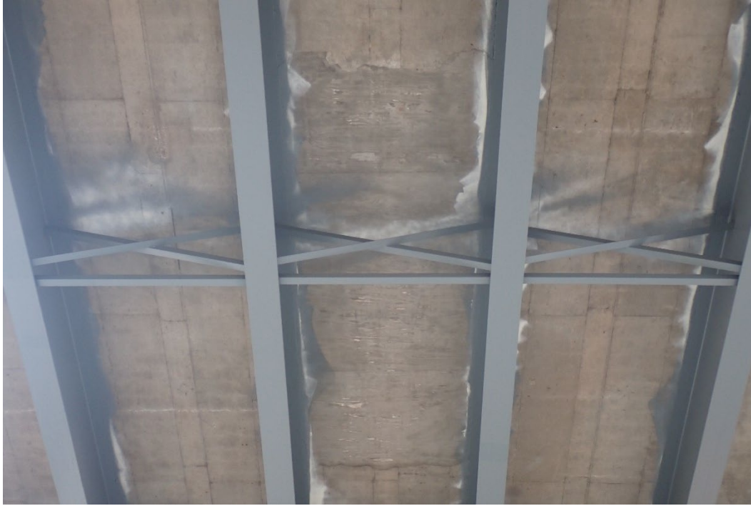
Photo 2 - Typical full bay width patch at Span 2A Bay 3.
