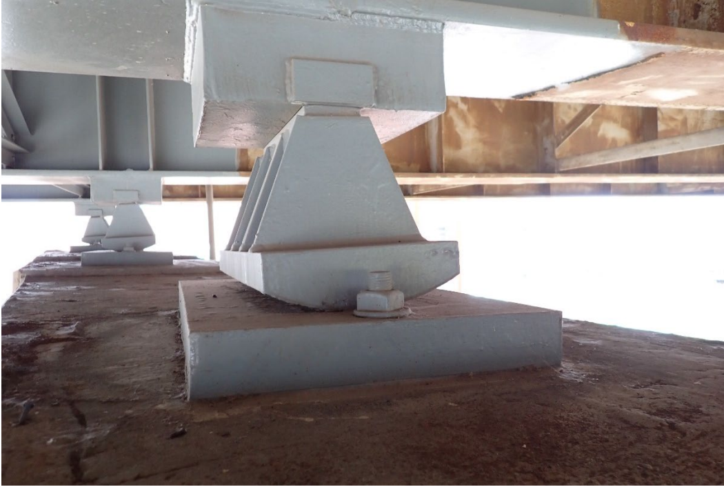
Photo 42 - Typical rocker bearing at Girder C at Pier 14C, looking northwest.
