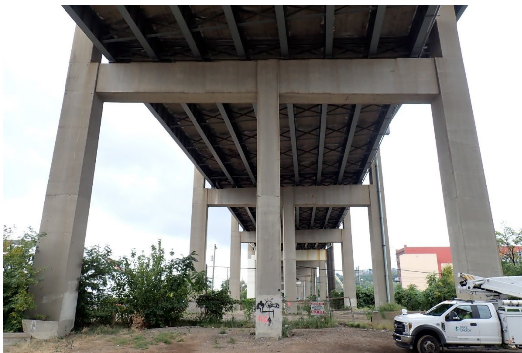
Photo 65 - Pier 11A looking south.
