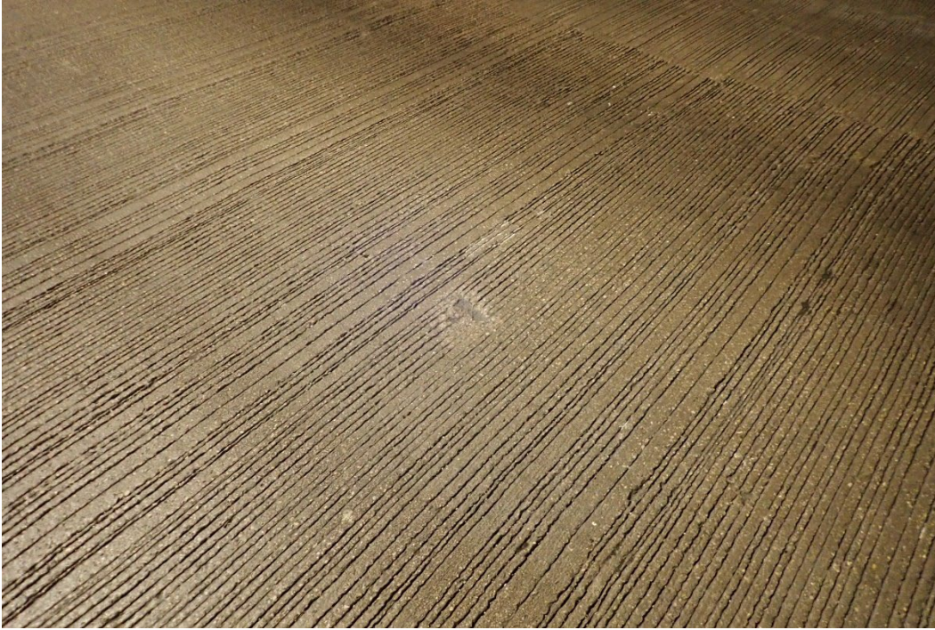
Photo 14 - Typical 6" diameter x 1/2" deep surface spall in Span 9A.
