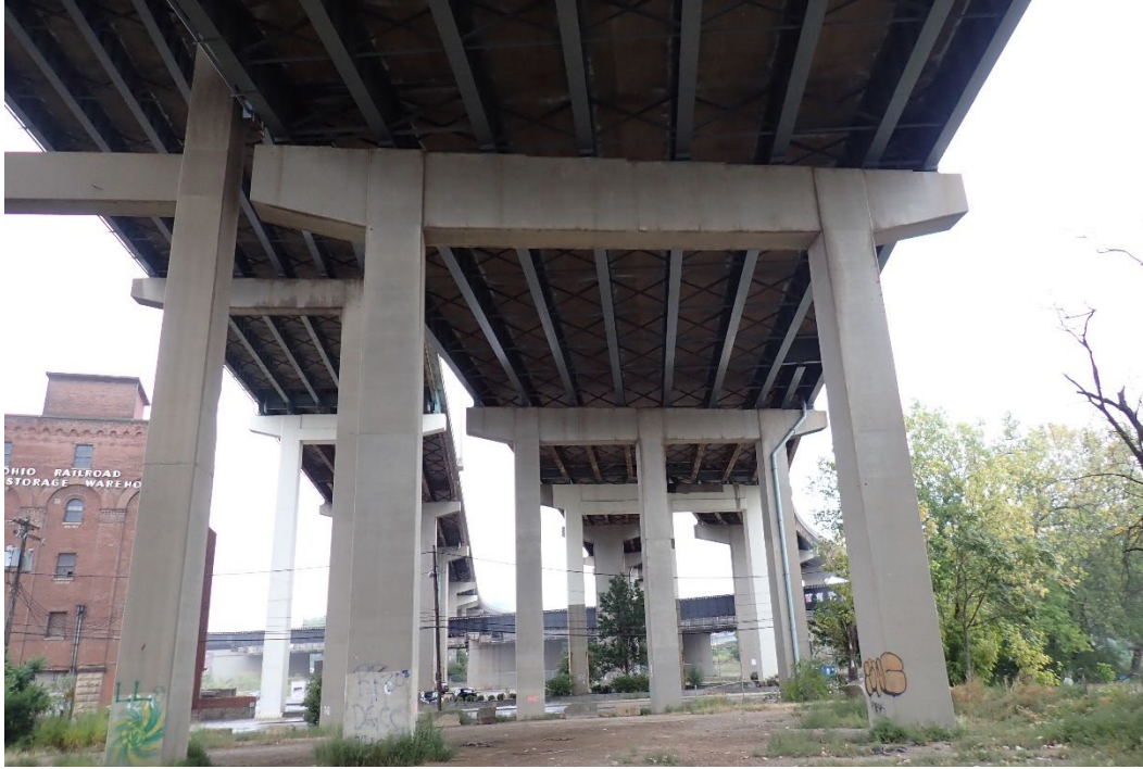
Photo 56 - Typical two-column pier at Pier 13C, looking north.
