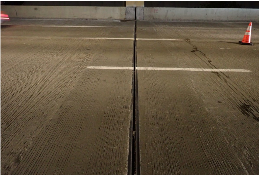
Photo 19 - Typical strip seal expansion joint at Pier 4, looking west.
