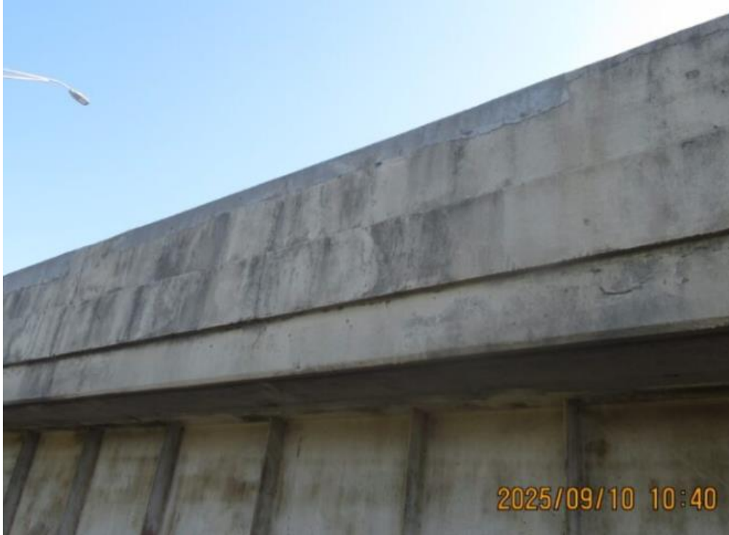
Photo 20: Typical concrete patch in west railing (Span 23A shown)
