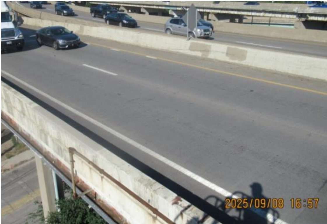
Photo 6: Wearing Surface Typical Condition (Span 20A shown)
