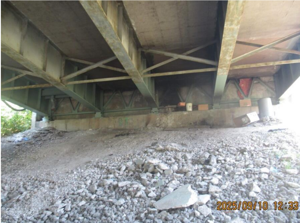
Photo 14: General Photo (Abutment A)
