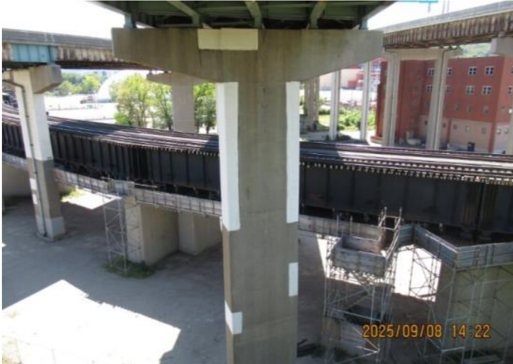
Photo 22: Typical concrete pier wall (Pier 17C)
