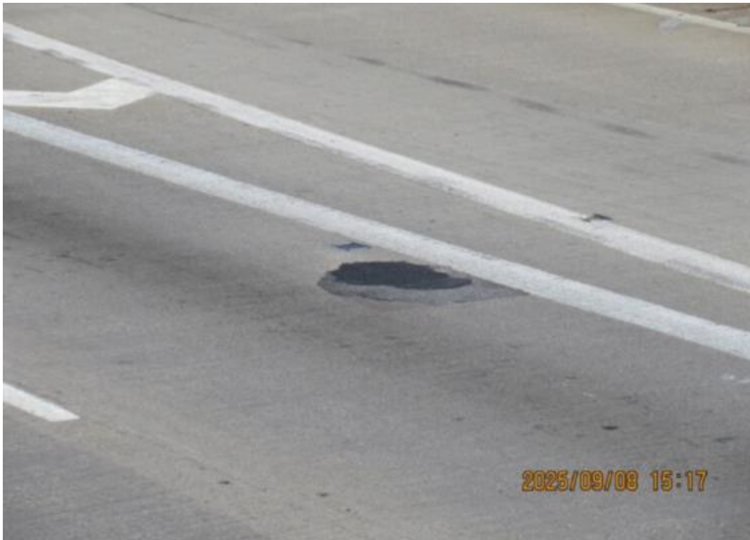
Photo 9: Typical asphalt patch (Span 22C shown)
