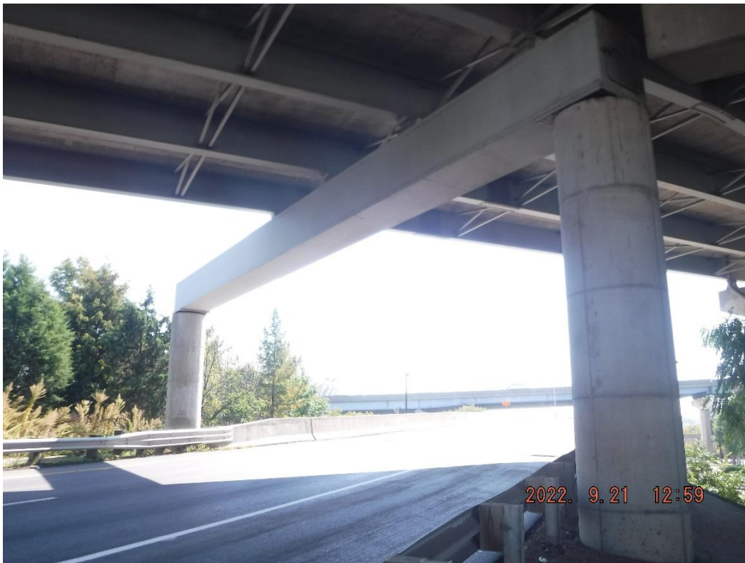
Photo 29: Pier Cap 25J looking south
