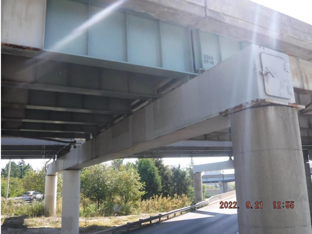
Photo 36: Pier Cap 26C/J looking south
