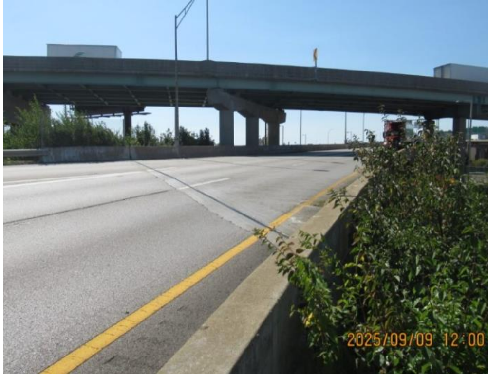
Photo 54: North approach slab looking east
