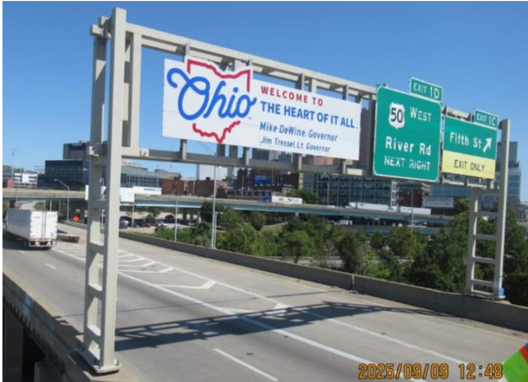
Photo 55: Overhead sign support mounted to railings near Pier 23C
