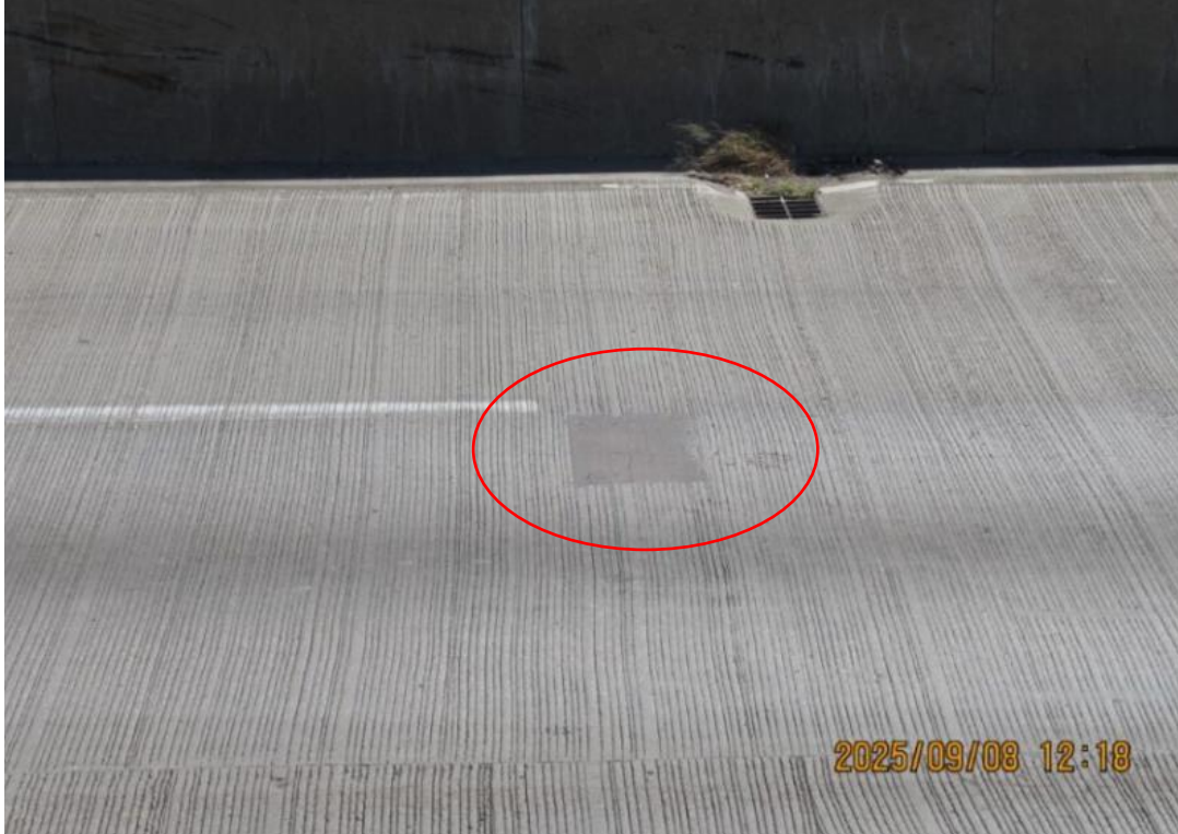
Photo 10: Typical concrete patch in good condition (Span 17C shown)
