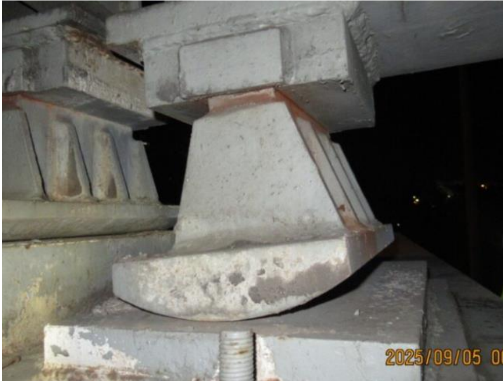
Photo 50: Bearing G expanded 6° at 55°F (Pier 26C/J)
