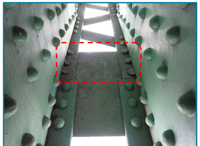
Photo 43 – Deformation of the rivet heads inside the lower chord (L32 of the South Truss, Span 9).
