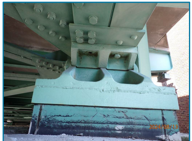
Photo 76 – Missing bolt attaching the sole plate to the girder (North Girder, Floorbeam 0, Span 4, looking west).
