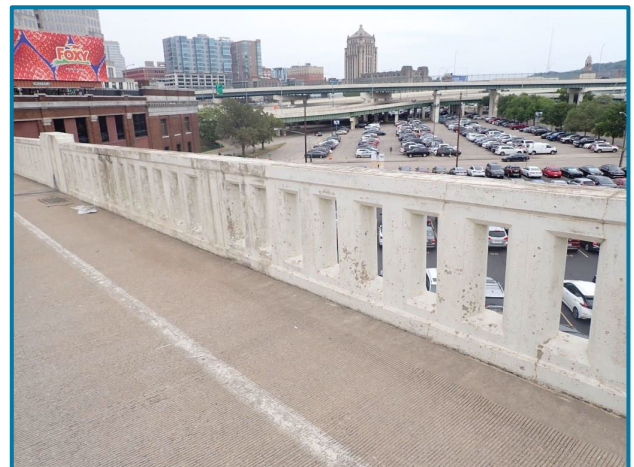
Photo 7 – Bridge railing (looking northwest).
