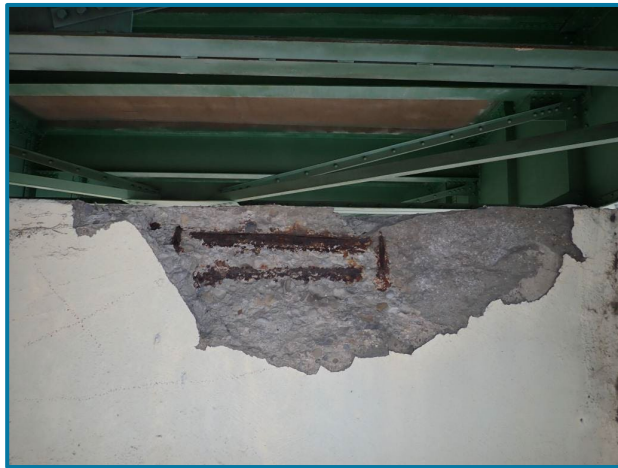
Photo 101 – 3'-8" L x 1'-1" H x 3" D spall with exposed rebar (Pier 16, East Face, looking west).
