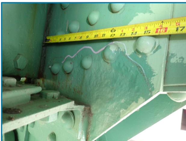
Photo 71 – 2'-4" L x 6" H x 3/16" D painted over pitting adjacent to the bearing (L20, South Truss, Span 6).
