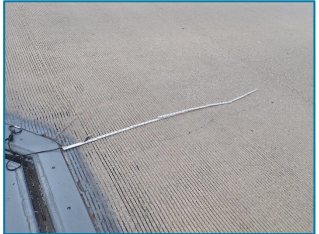
Photo 6 – Moderate to wide cracks near where the expansion joint armor bends (near Pier 10).
