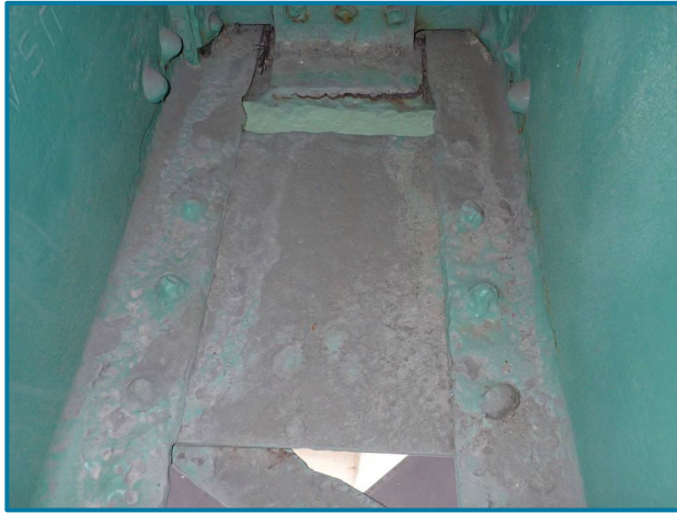
Photo 40 – Up to 50% section loss to the rivet heads inside the lower chord (L0L1 of the Center Truss, Span 7).
