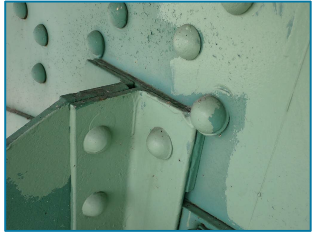
Photo 70 – Rivet deformation due to conflict with the sway bracing connection (L28, Center Truss, Span 8).
