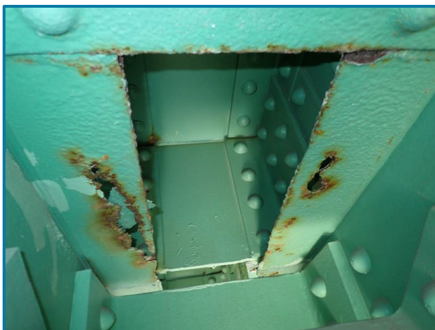
Photo 46 – Corrosion holes, pitting, and active corrosion to the bottom flanges (U0 of the Center Truss, Span 10).
