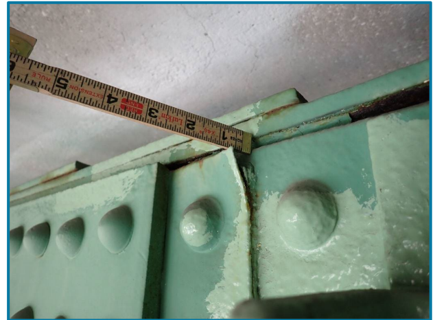
Photo 45 – Pack rust at the top splice plate and distortion at the fill plate (U12U13 of the Center Truss, Span 6).
