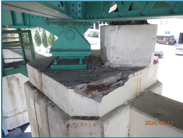
Photo 87 – 4' L x 8" W x 6" D spall with exposed rebar (Pier 5, Center Column, North Face, looking southwest).
