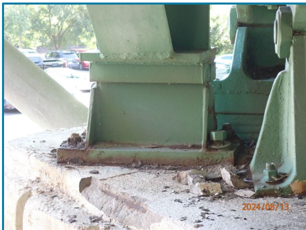
Photo 78 – 1 loose anchor nut and 2 with 30% section loss (Pier 4, North Girder, Span 3, looking east).
