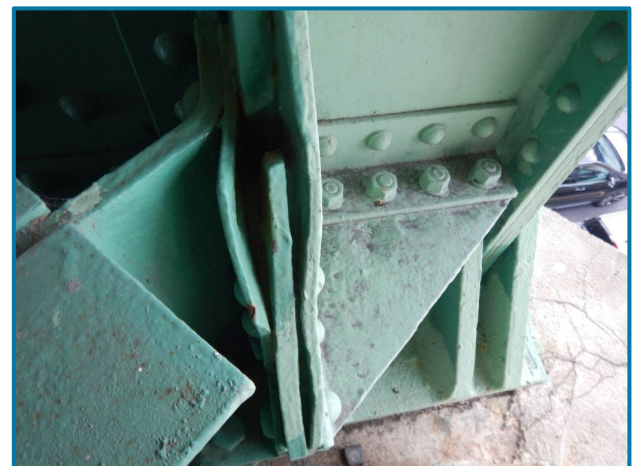
Photo 68 – 1" pack rust between the lower lateral bracing fill plate and the gusset plate (L0, South Truss, Span 5).
