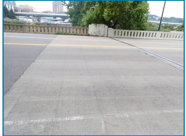
Photo 103 – Wear in the wheel lines of the approach slab (West Approach Slab, looking north).
