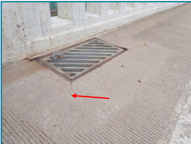
Photo 5 – Moderate to wide cracks propagating from the scupper grate corner (near Pier 10).
