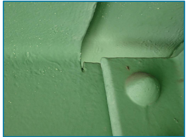
Photo 64 – 3/8" overcut in the floorbeam cope (south side of U39, Center Truss, Span 9).
