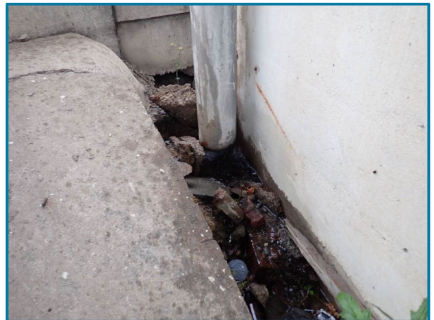
Photo 22 – Slope protection and adjacent approach slab are undermined (Pier 13 shown, looking west).
