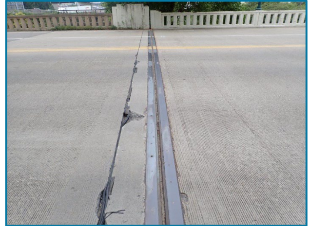
Photo 17 – Spalls in the joint header with damaged construction joint material (Abutment 1 shown, looking north).
