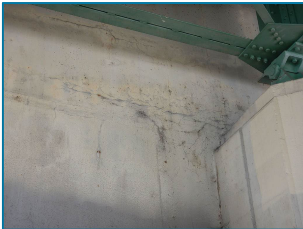
Photo 95 – Hairline map cracking over an area of 5' L x 2' H (Abutment 18, West Face, looking east).
