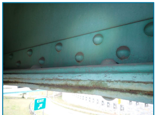
Photo 31 – 1/16" pack rust between the bottom flange cover plates (Span 16 shown, looking northwest).
