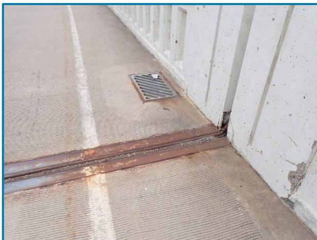
Photo 14 – Surface corrosion to the deck joint armour in the shoulder (Pier 16 shown, looking east).
