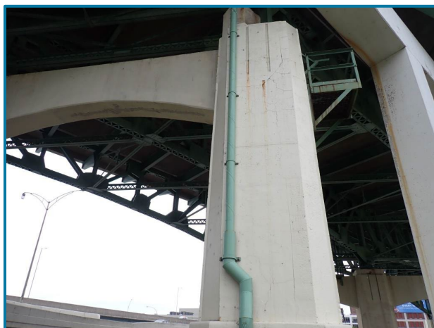
Photo 91 – Hairline cracking with rust staining (Pier 12, North Column, East Face, looking west).
