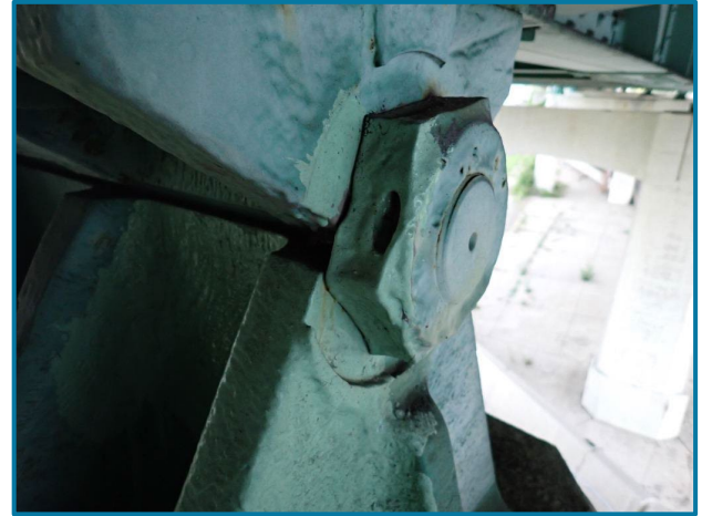
Photo 77 – Gouge in the pin nut with painted over pitting (Pier 12, Center Girder, Span 12, looking southwest).
