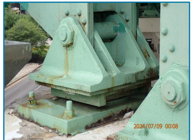
Photo 80 – Surface corrosion and rust staining to the bearing (L14, North Truss, Pier 8, looking southeast).
