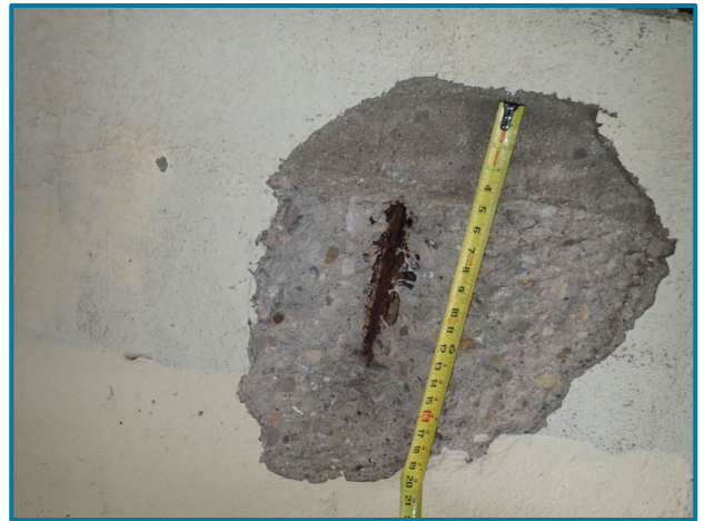
Photo 102 – 1'-8" diameter x 2" D spall with exposed rebar (Pier 16, West Face, looking east).
