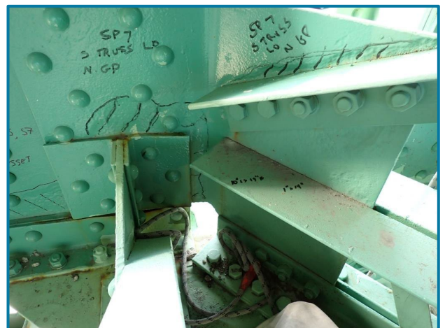
Photo 72 – 3/16" painted over pitting to multiple locations on the gusset plate (L0, South Truss, Span 7).
