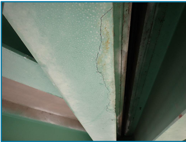
Photo 62 – 2' L x 3" W area of light surface corrosion to the bottom flange (Span 6 over Pier 7).
