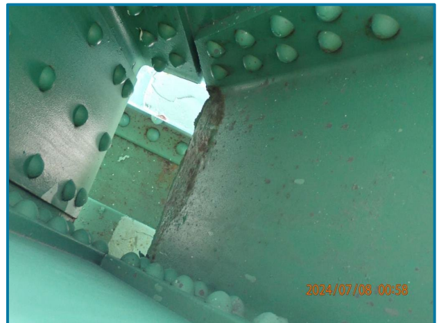
Photo 60 – Surface corrosion at the diagonal end with pack rust forming (U32L33 of the North Truss, Span 9).
