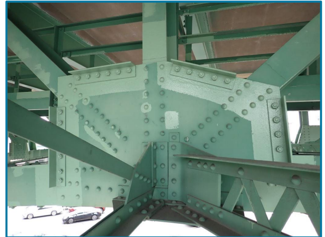
Photo 65 – Rehabilitation work to stiffen the gusset plates that were bowed (looking west).
