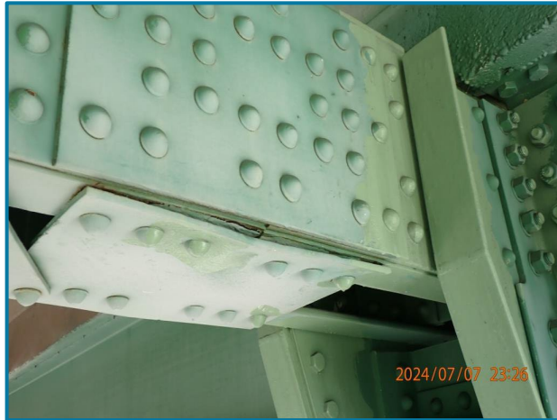
Photo 44 – 3/4" pack rust at the bottom batten plate (U42U43 of the North Truss, Span 9).
