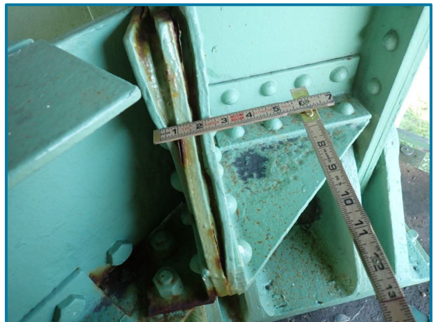
Photo 85 – Up to 1" pack rust at the connection to the truss (L20, North Truss, Span 11, looking northwest).
