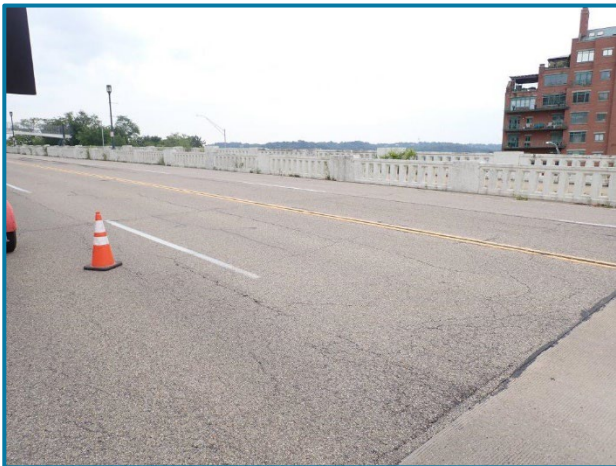
Photo 104 – Wide map and random cracking in the approach pavement (East Approach, looking southeast).
