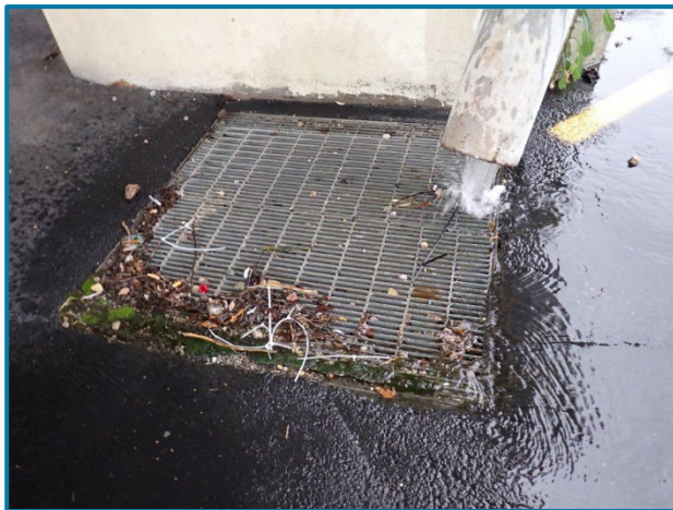
Photo 19 – Grate partially obstructed and drainpipe not directly aimed at grate center (Pier 5 shown, looking north).
