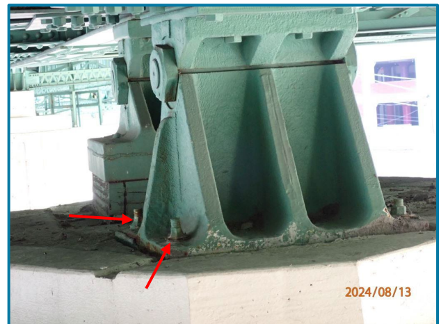
Photo 79 – Up to 40% section loss to the anchor nuts (Pier 4, Center Girder, Span 3, looking southeast).
