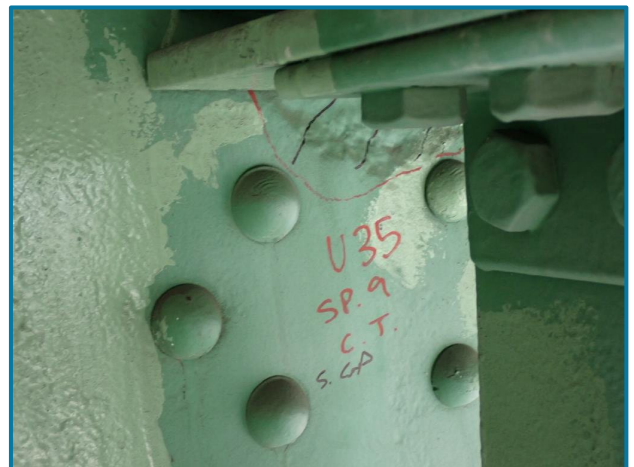
Photo 47 – 6" L x 2" H x 1/8" D pitting underneath the floorbeam connection (U35 of the Center Truss, Span 9).
