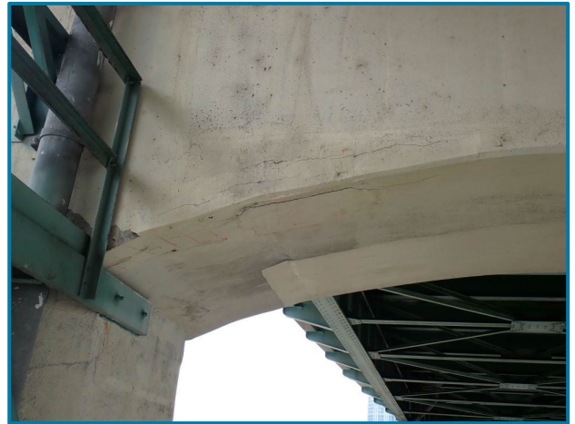
Photo 100 – 10' L section of cracked repair patch that extends 1' underneath (Pier 15, East Face, looking west).
