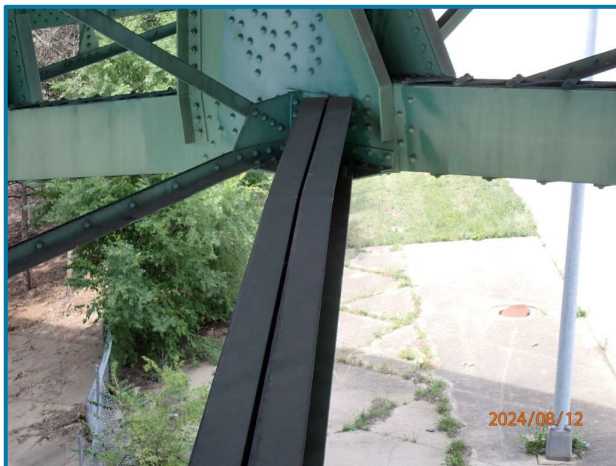
Photo 84 – Impact damage to the lower lateral bracing (6' south of L18, Center Truss, Span 8, looking north).
