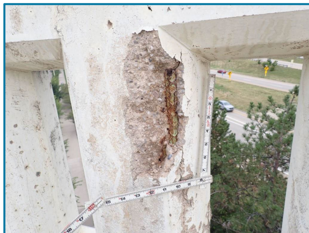
Photo 10 – Spall with exposed rebar in the railing stem (looking northwest at north railing).
