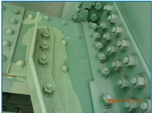
Photo 50 – Four plug welds on each side of the upper chord member (U25 of the North Truss, Span 8).
