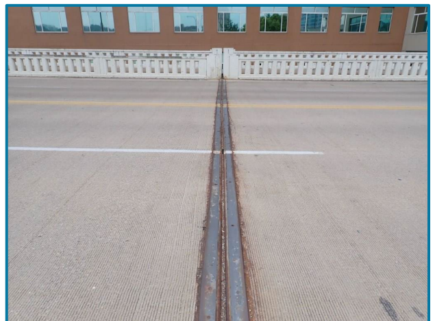
Photo 15 – Surface corrosion to the full length of the deck joint armor (Pier 2 shown, looking south).
