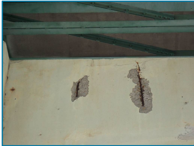
Photo 99 – 1' L x 3' H x 1" D and 1' L x 1' H x 1" D spalls with exposed rebar (Pier 13, East Face, looking west).
