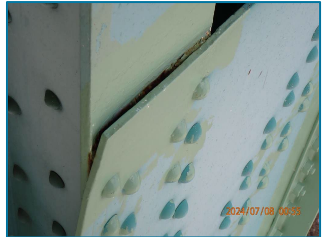
Photo 67 – Typical pack rust at the gusset plate causing distortion (L33, North Truss, Span 9).
