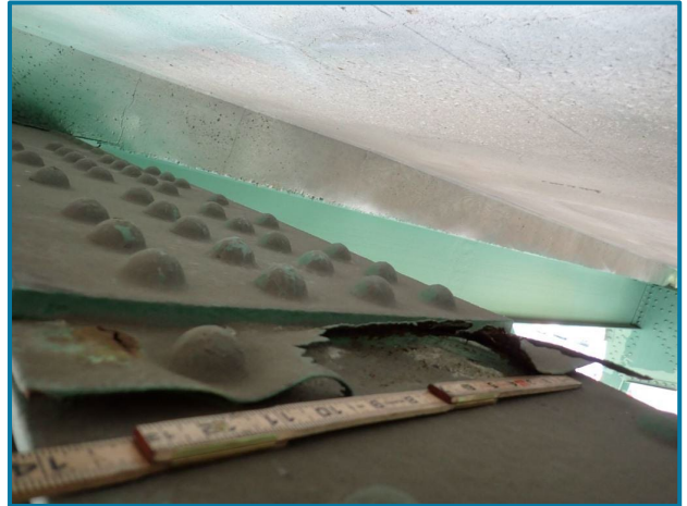
Photo 48 – 8" L x 2" W area of 100% section loss to the fill plate (U9U10 of the Center Truss, Span 6).
