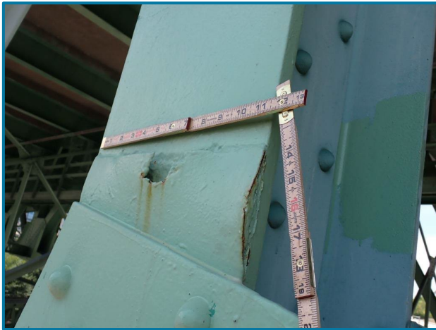
Photo 51 – 9/16” pack rust at the fill plate causing distortion to the plate (U13L13 of the South Truss, Span 7).
