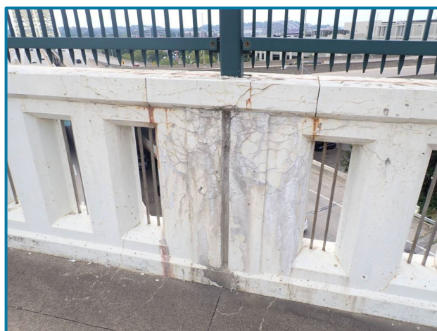
Photo 11 – Map cracking with efflorescence (possible ASR) in the concrete railing (looking south at the south railing).
