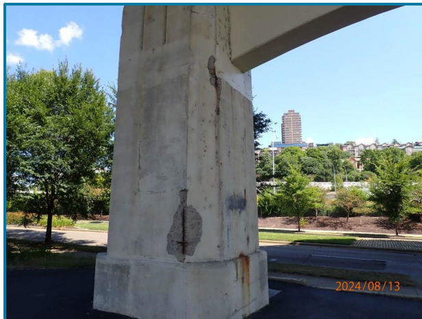
Photo 89 – Two spalls with exposed rebar (Pier 7, North Column, South and West Faces, looking northeast).
