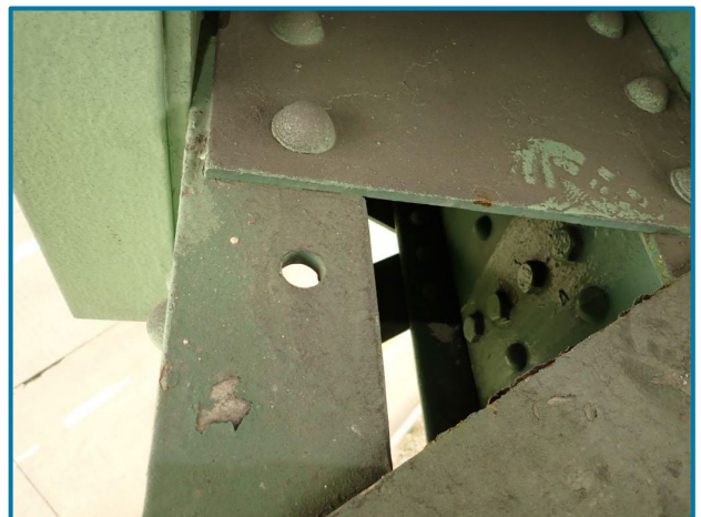
Photo 42 – Blind hole in the lower chord top flange near (L27L28 of the Center Truss, Span 8).
