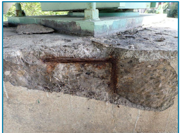
Photo 90 – 1'-9" L x 8" H x 2" D spall with exposed rebar (Pier 8, South Column, North Face, looking south).
