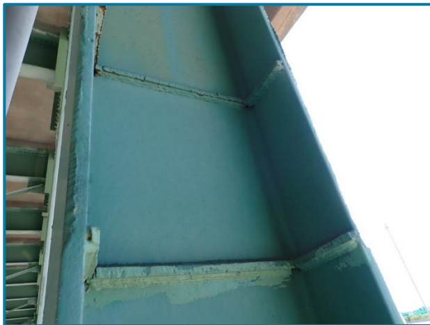
Photo 53 – Remains of a welded attachment (U0L0 of the South Truss, Span 10).
