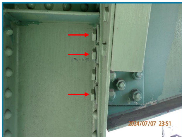
Photo 55 – Three bolts not properly snug (U40 of the North Truss, Span 9).
