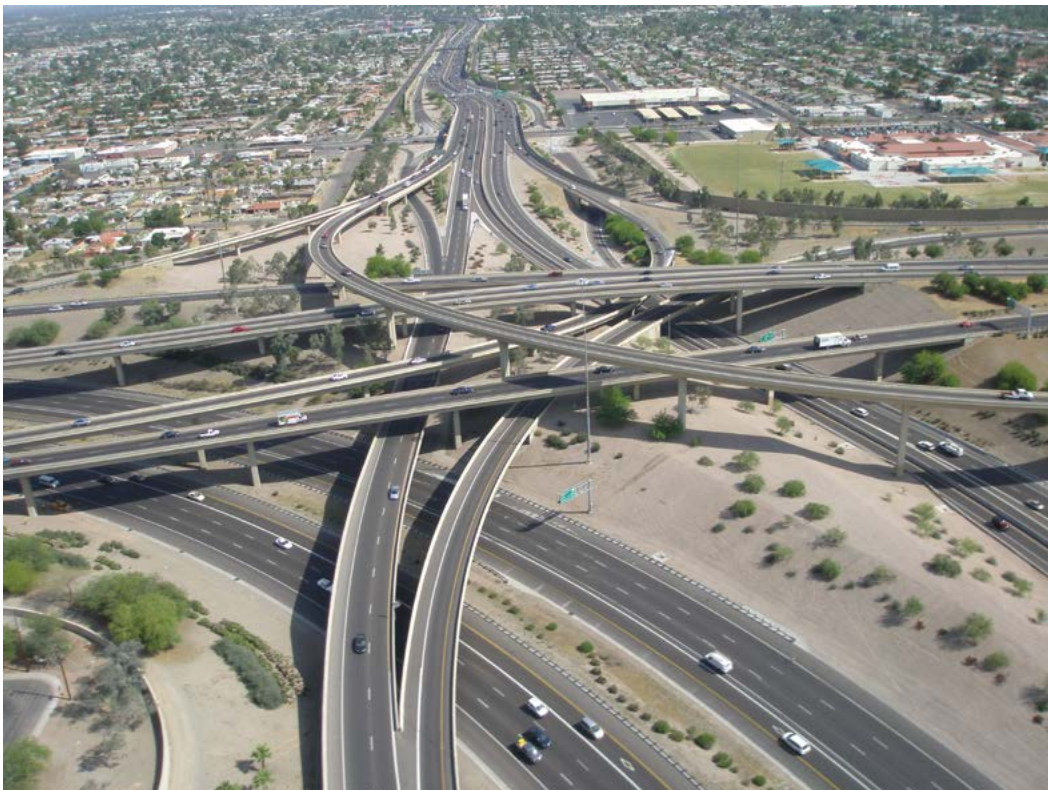
Figure 10-37. Four-Level Directional Interchange
