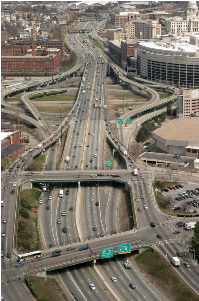
Figure 8-17. Combination-Type Freeway
