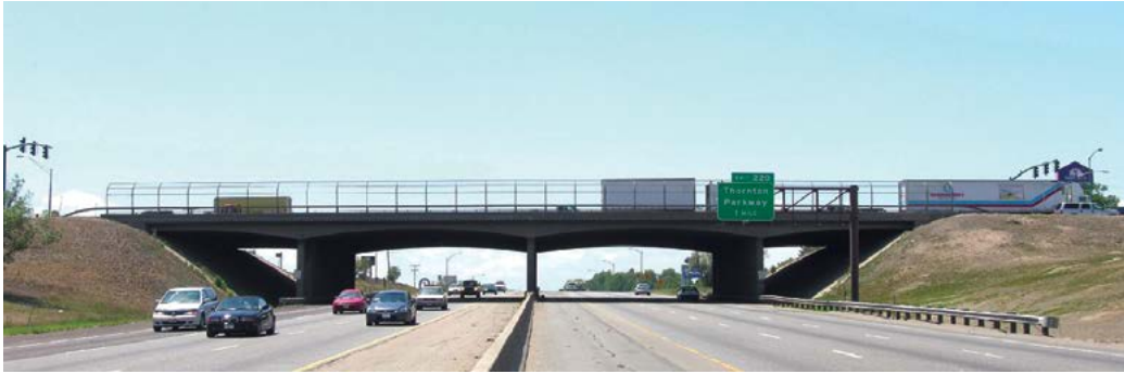
Figure 10-4. Typical Grade Separation Structure with Open-End Span
