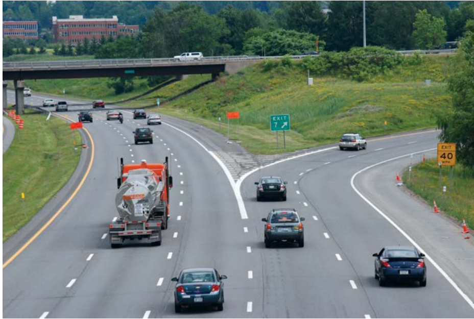
Figure 10-68. Gore Area, Two-Lane Exit
