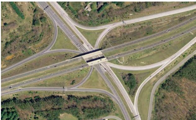
– B – Overpass SPDI
