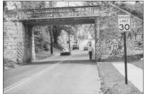
Exhibit 3-38. Undesirable Condition Due to Lack of Sidewalk Continuity (18).
