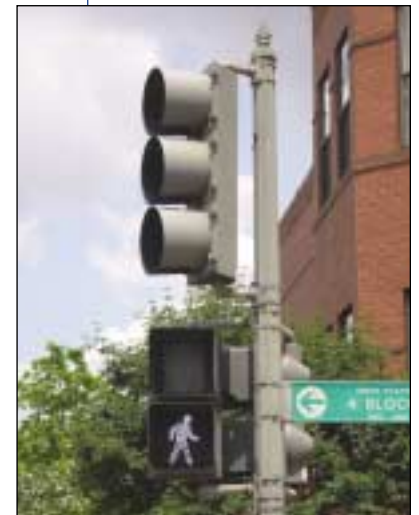
Exhibit 4-4. Vehicular Signal Heads Are Obscured So Pedestrian Signals Are Necessary. Photo courtesy of James T. McDonnell.
