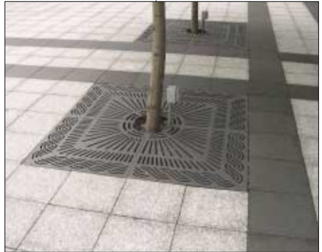
Exhibit 3-16. Well-Designed Sidewalk Tree Grate.
