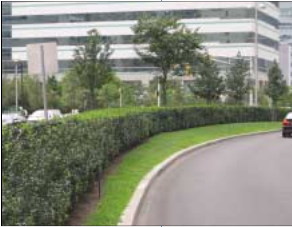
Exhibit 3-34. Median Plantings to Discourage Midblock Crossing (16).
