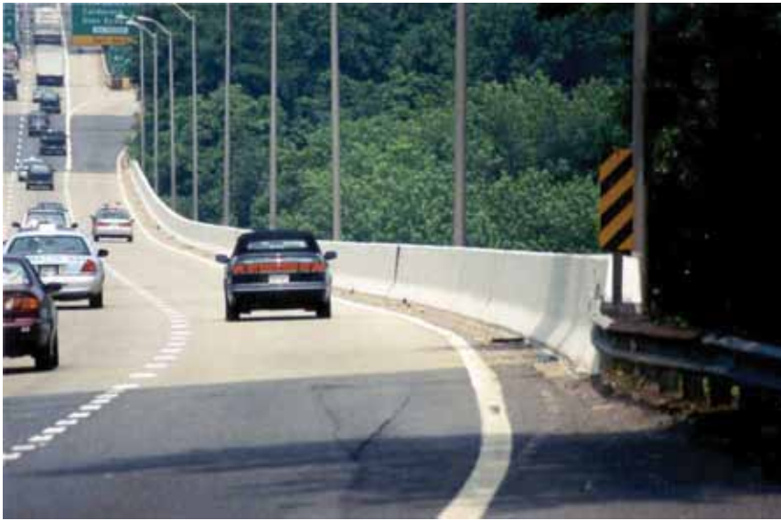
Figure 7-5. 1,067-mm [42-in.] Tall Concrete Safety-Shaped Bridge Railing
