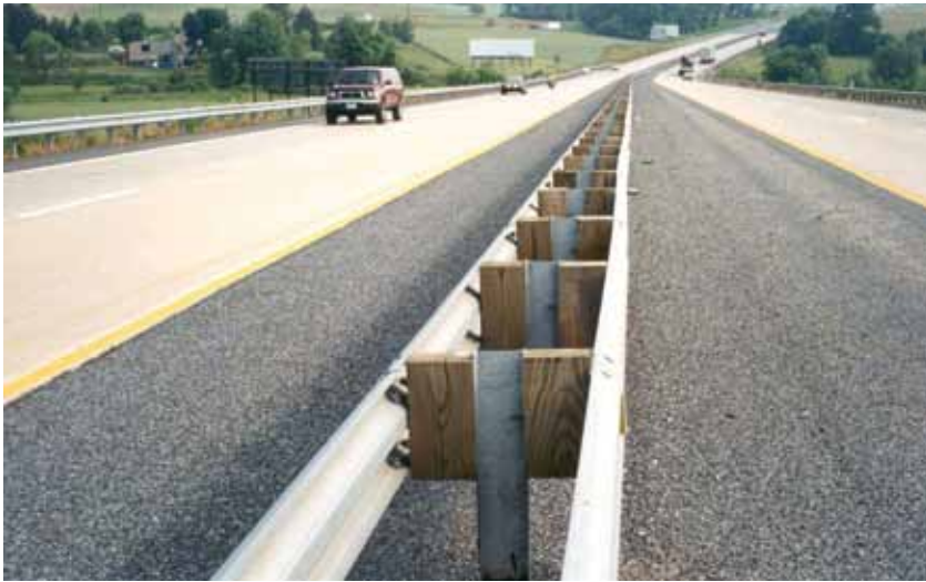
Figure 6-10. Strong-Post W-Beam Median Barrier
