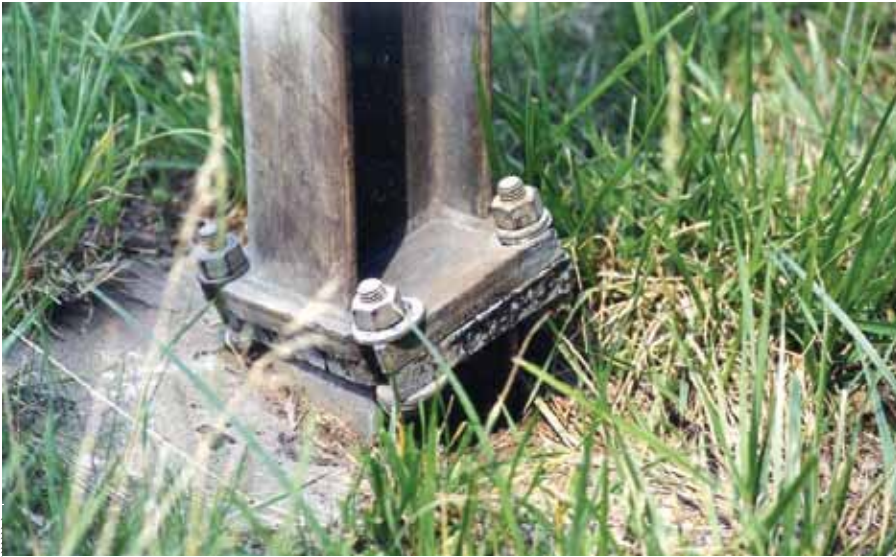
Figure 4-8. Unidirectional Slip Base for Small Signs
