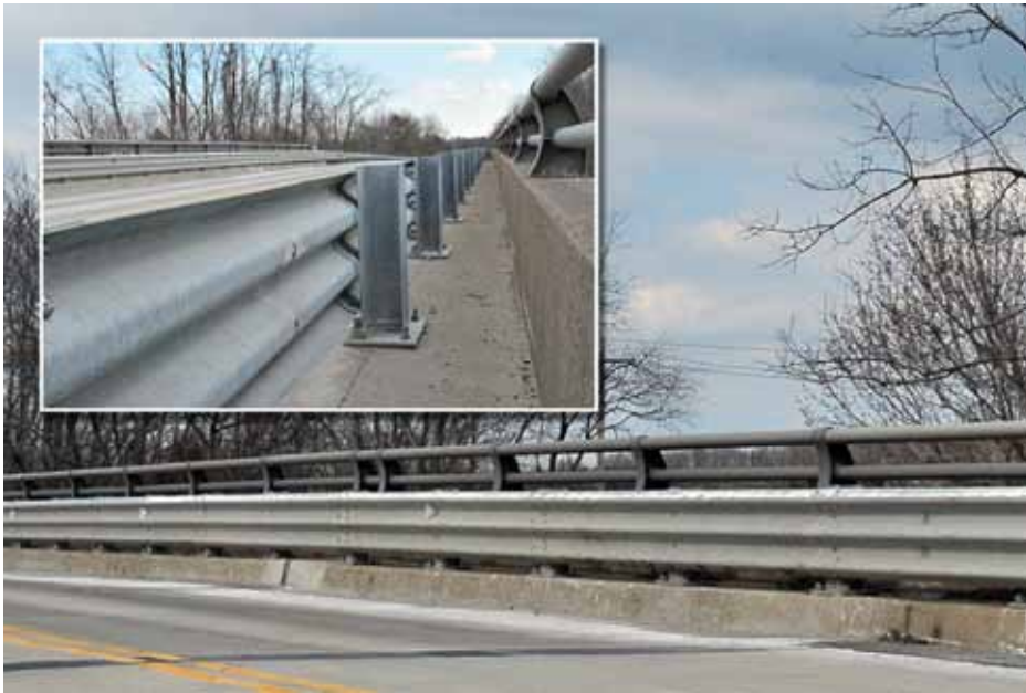
Figure 7-10. Delaware Thrie-Beam Retrofit
