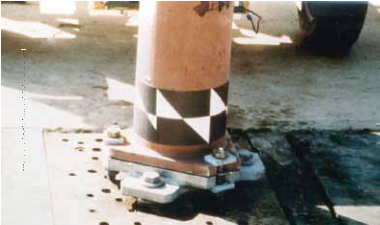
Figure 4-12. Example of a Luminaire Slip Base Design
