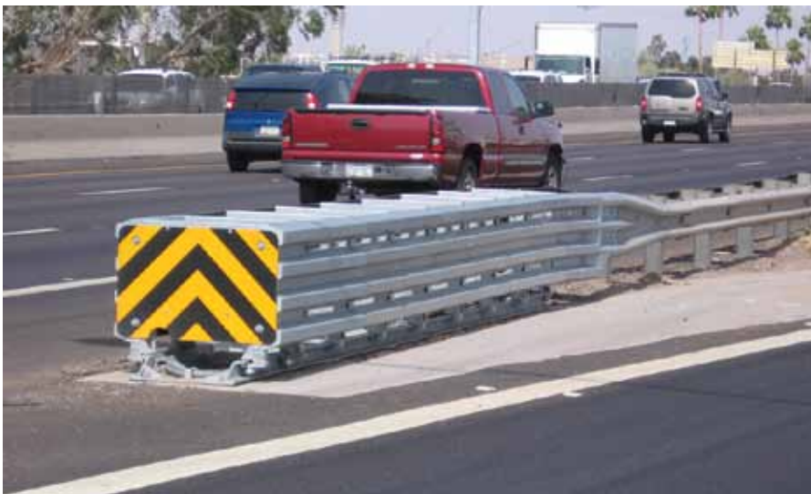
Figure 8-37. Smart Cushion Innovations (SCI-100GM) Crash Cushion
