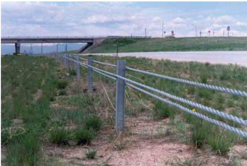
Figure 6-3. Three-Strand Cable Median Barrier
