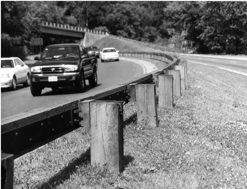
Figure 5-18. Backed Timber Guardrail
