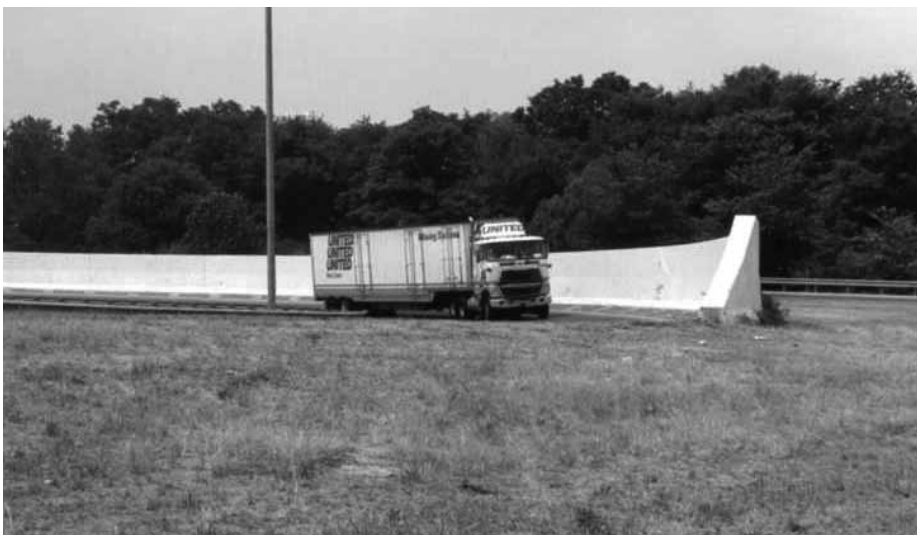
Figure 5-21. 2,290-mm [90-in.] New Jersey Barrier
