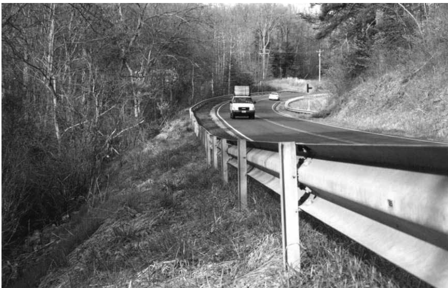
Figure 5-6. Weak-Post W-Beam Guardrail
