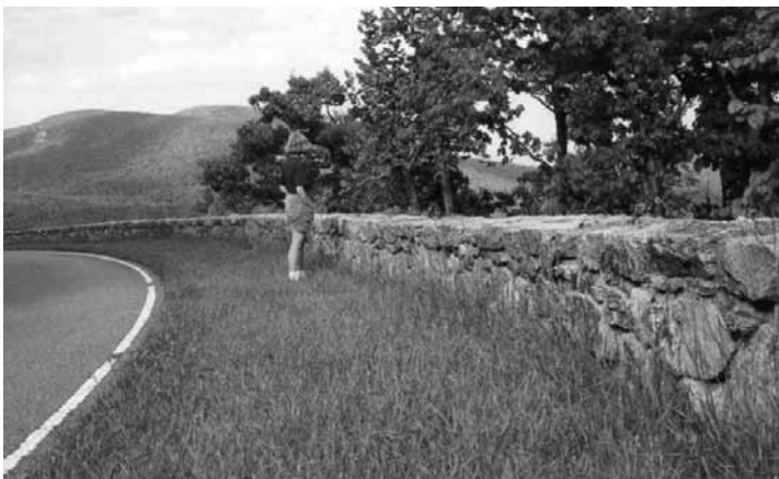
Figure 5-23. Stone Masonry Wall
