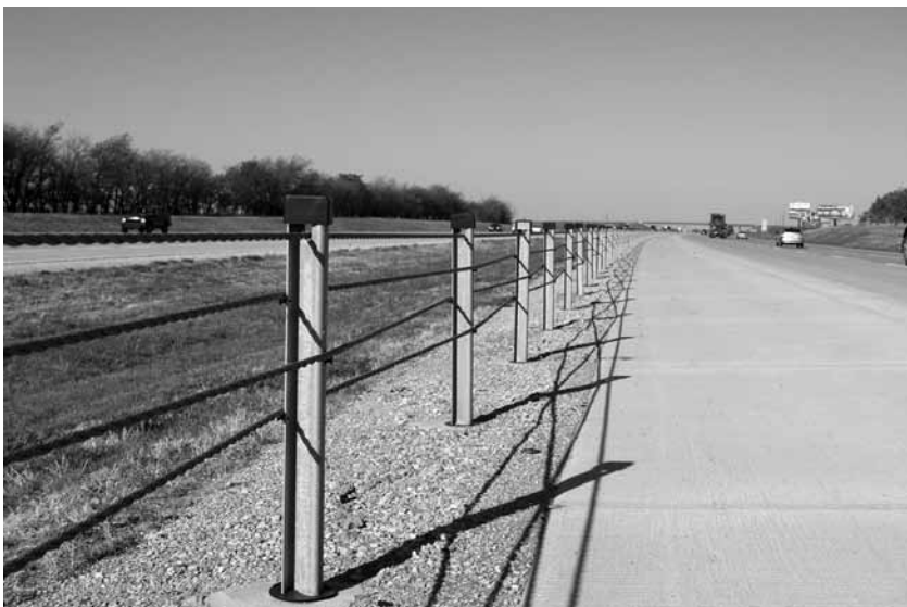
Figure 6-4. Brifen Wire Rope Safety Fence
