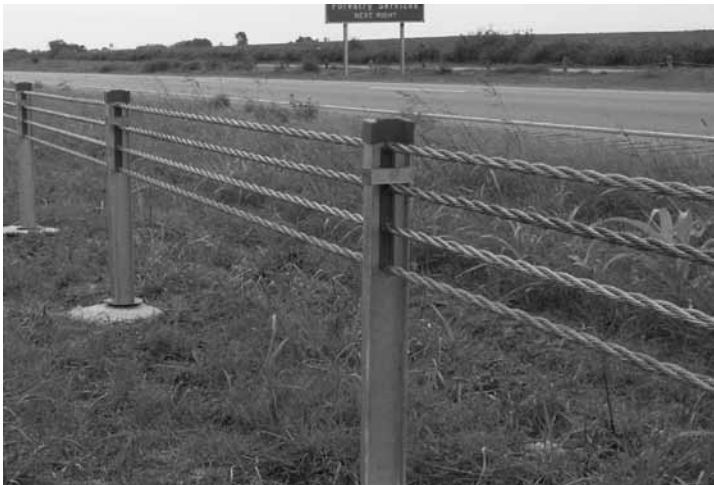
Figure 6-6. NU-CABLE™ High-Tension Cable System
