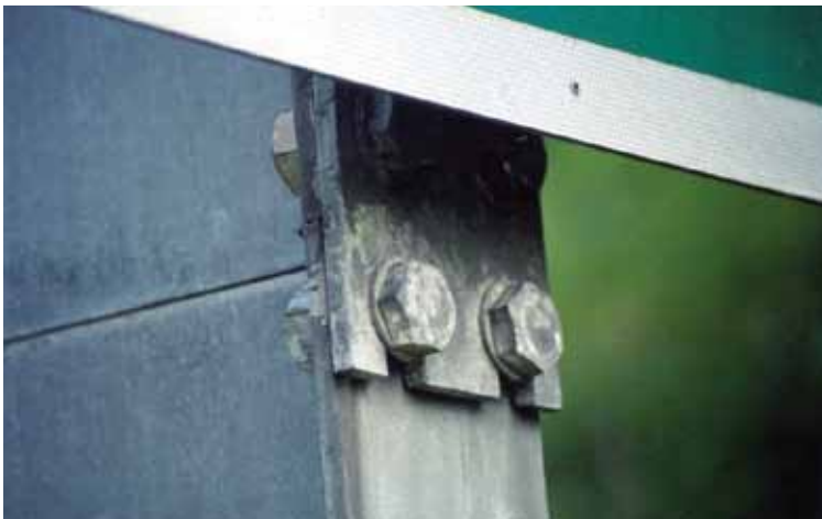
Figure 4-6. Slotted Fuse Plate Design
