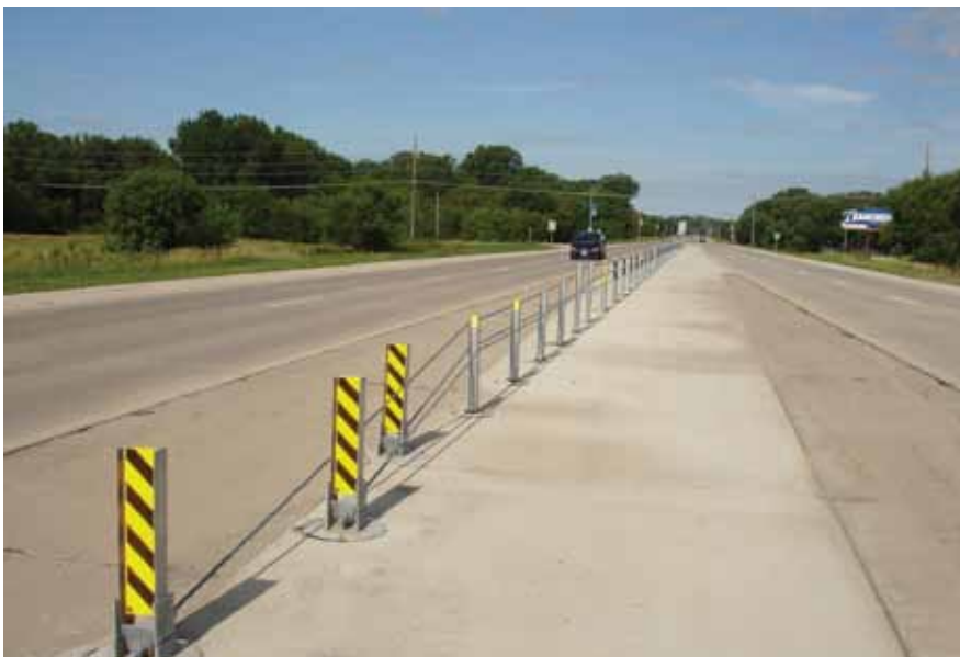
Figure 8-5. CASS™ Cable Terminal (CCT)
