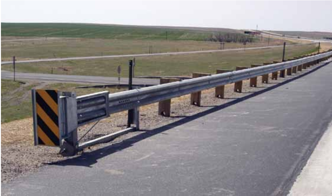
Figure 8-12. Extruder Terminal (ET-Plus™)
