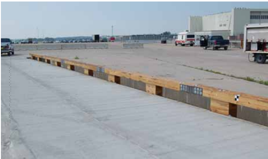
Figure 7-1. Curb Type Glu-Lam Timber Railing
