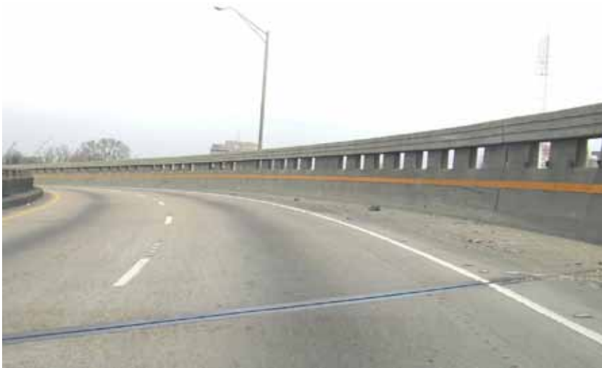
Figure 7-6. Texas Type TT Railing
