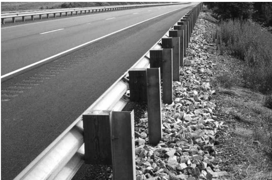
Figure 5-9. Steel-Post W-Beam Guardrail with Wood Blockouts
