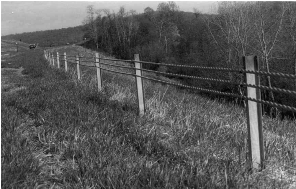
Figure 5-5. Three-Strand Cable Barrier
