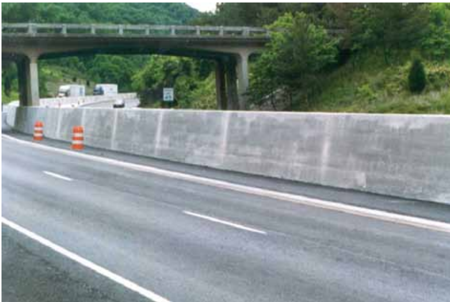
Figure 6-14. Single-Slope Concrete Median Barrier
