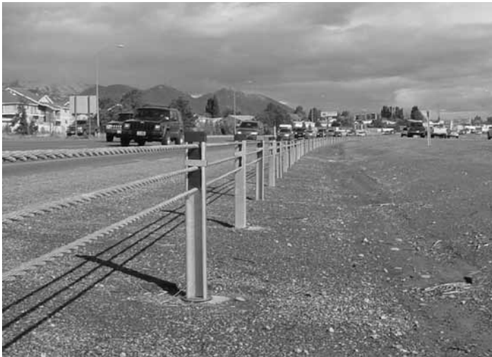
Figure 6-5. The Cable Safety System (CASS)
