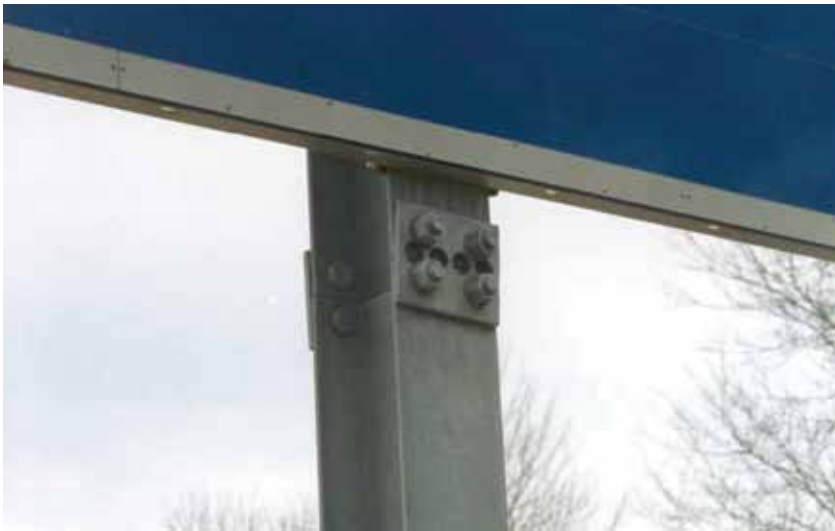
Figure 4-7. Perforated Fuse Plate Design
