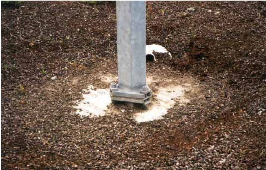
Figure 4-10. Oregon 3-Bolt Slip Base
