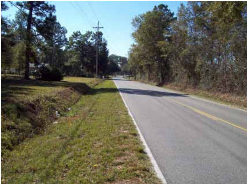
Figure 12-4. Typical Low-Volume Rural Roadway
