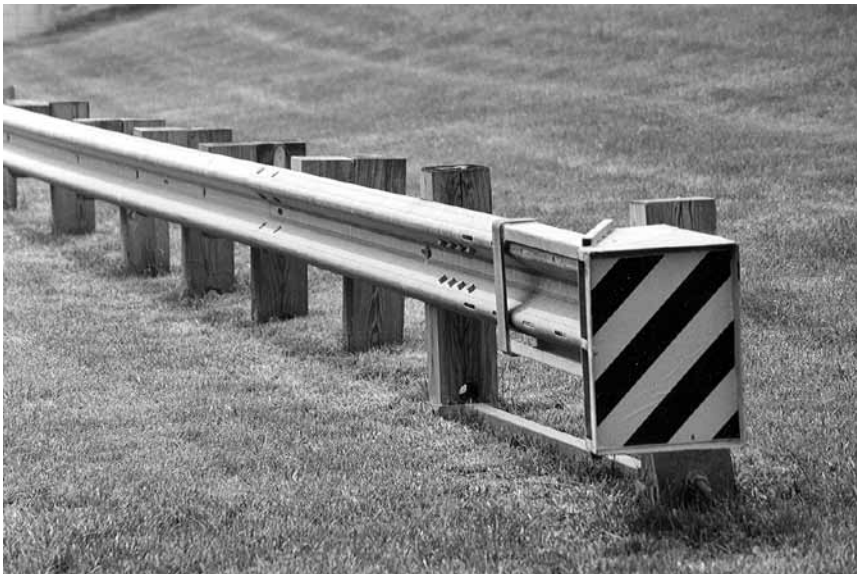
Figure 8-9. Flared Energy-Absorbing Terminal (FLEAT™)
