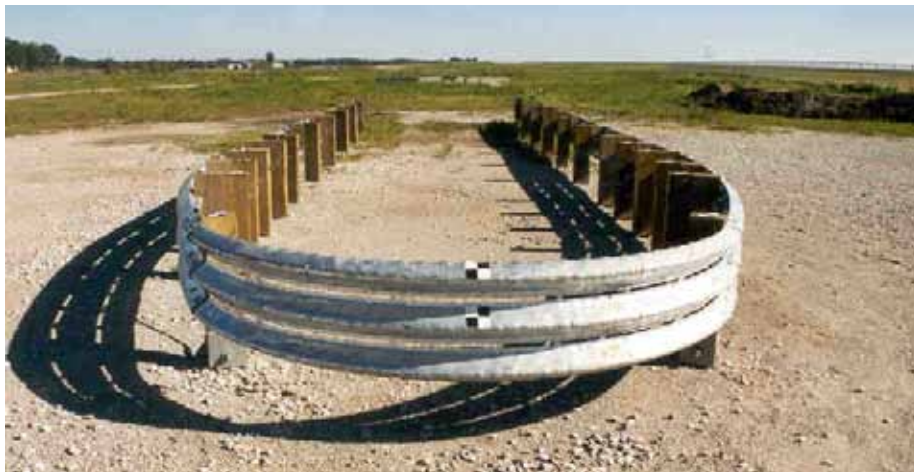
Figure 8-20. Bullnose Guardrail System
