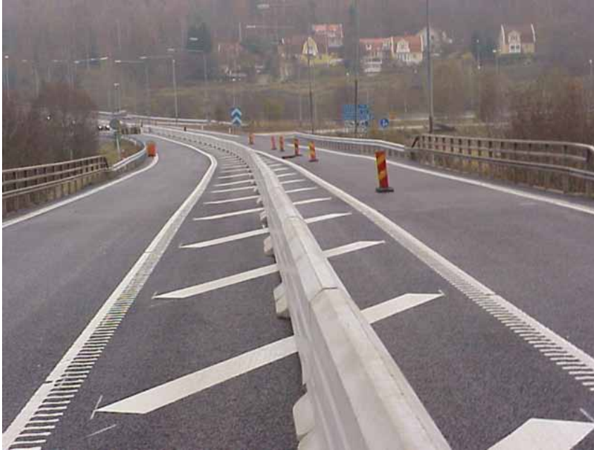
Figure 9-6. GPLINK® Pre-Cast Temporary Concrete Barrier
