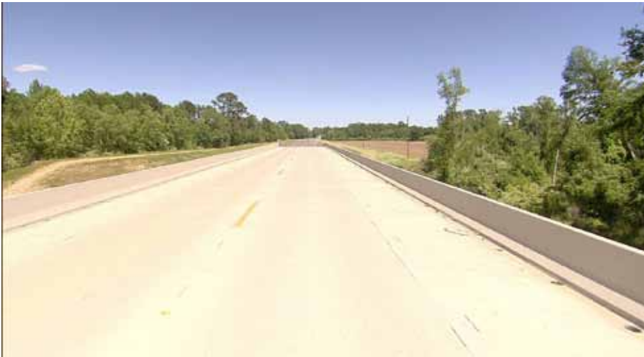
Figure 7-4. Concrete F-Shaped Bridge Railing
