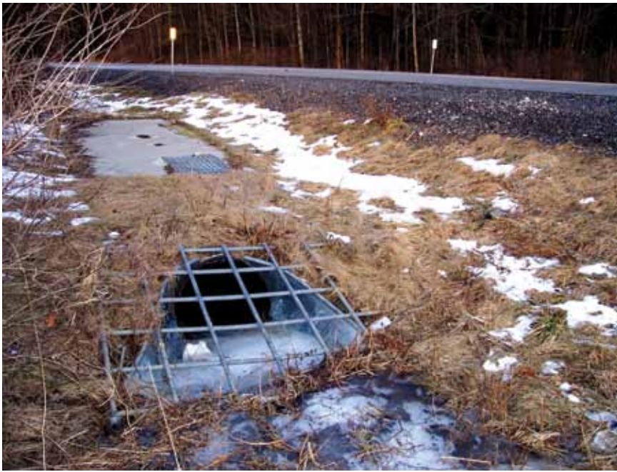
Figure 12-3. Reinforcing Steel Grate
