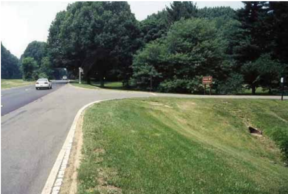
Figure 3-3. Suggested Design for Transverse Slopes
