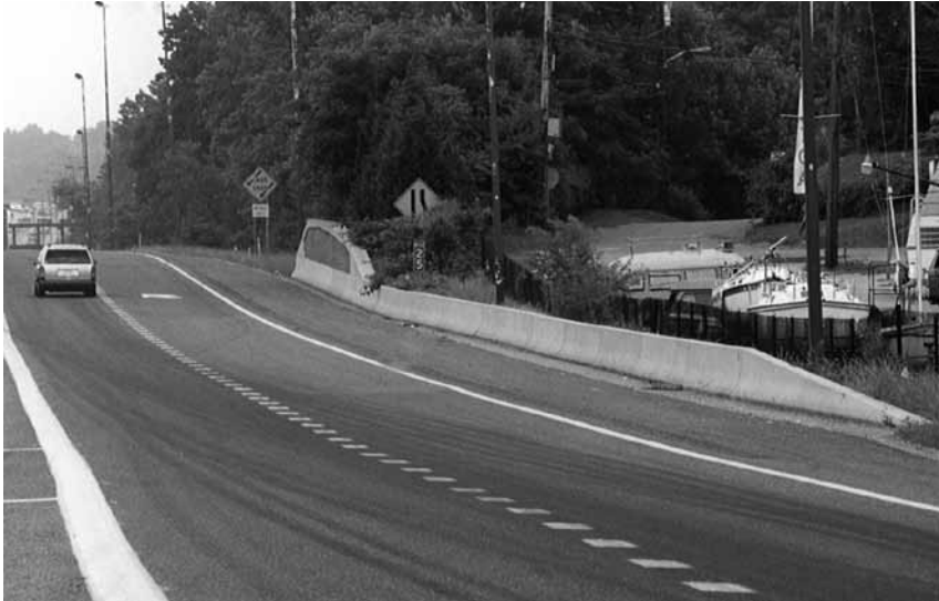
Figure 8-43. Sloped Concrete End Treatment
