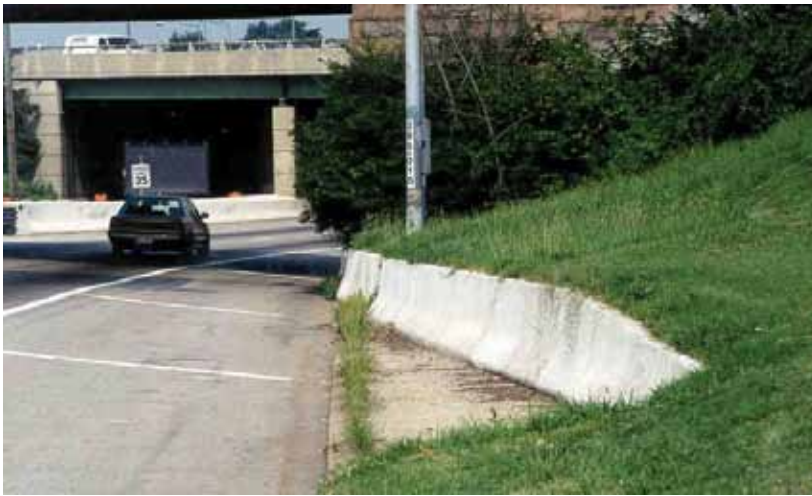
Figure 8-44. Barrier Anchored in Backslope
