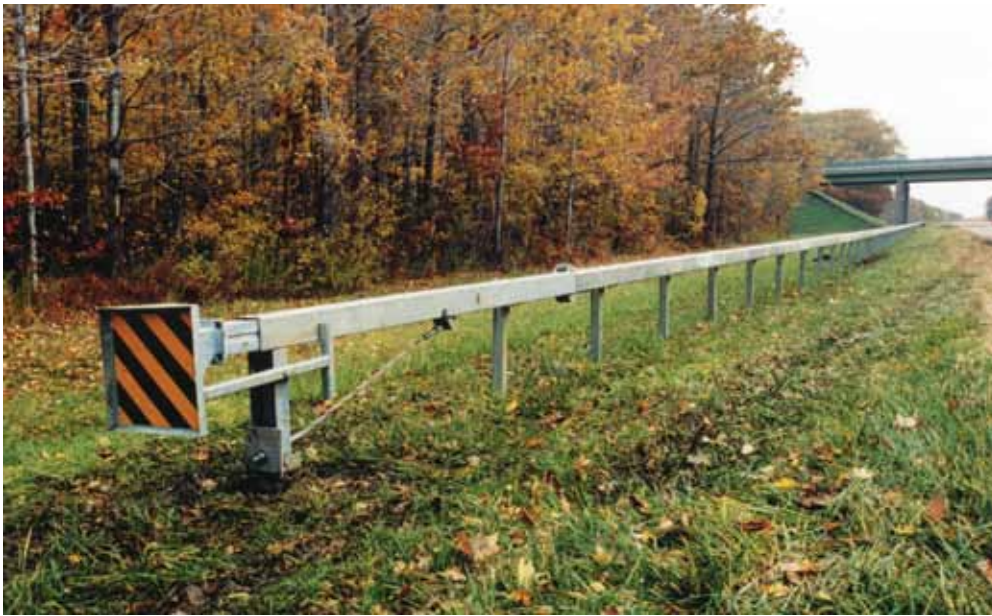
Figure 8-19. Bursting Energy Absorbing Terminal (BEAT™)
