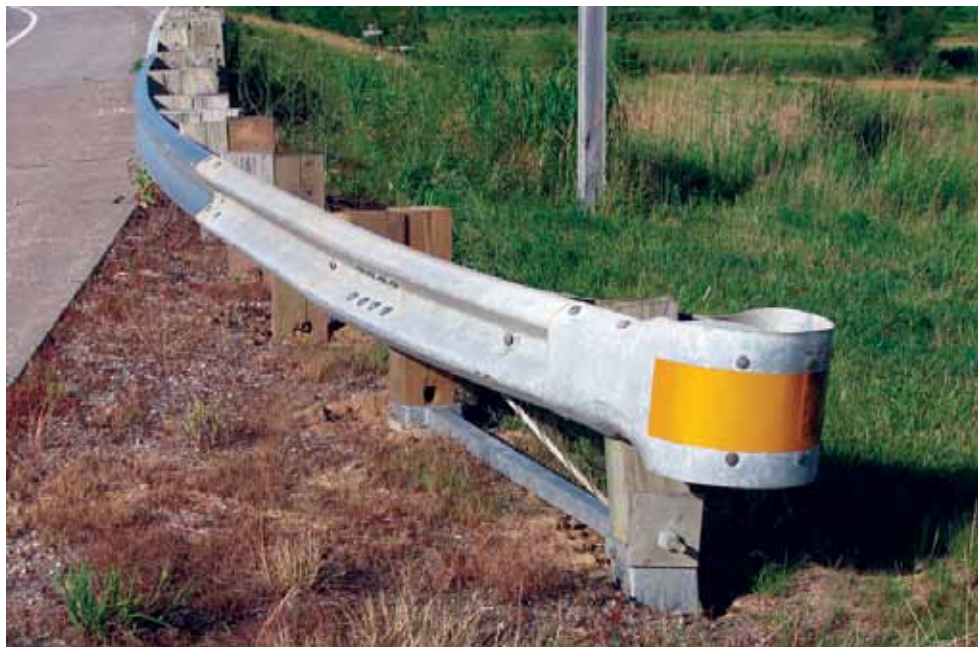
Figure 8-8. Modified Eccentric Loader Terminal (MELT)
