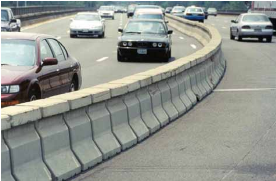
Figure 6-15. Standard Quickchange® Moveable Barrier System
