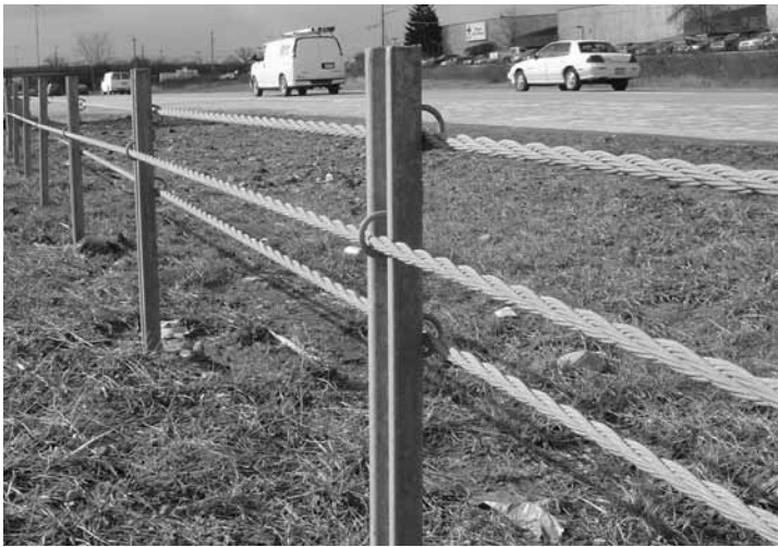
Figure 6-6. NU-CABLE™ High-Tension Cable System
