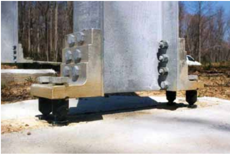
Figure 4-4. Multidirectional Coupler
