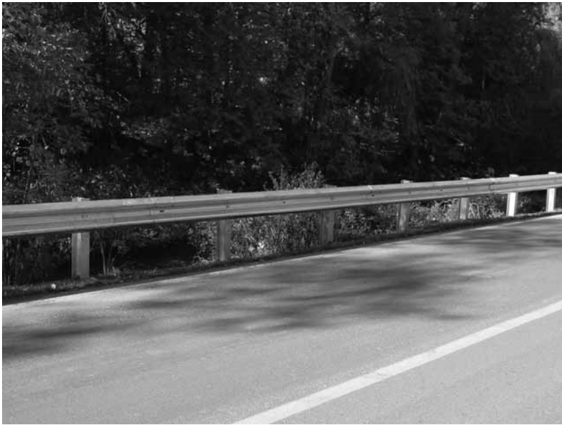
Figure 5-12. Trinity T-31™ Guardrail System
