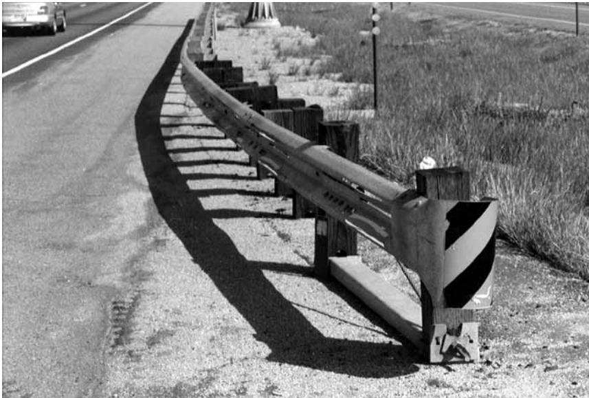
Figure 8-10. Slotted Rail Terminal (SRT-350™)
