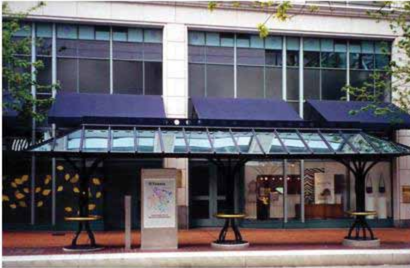
Figure 10-6. A Transit Shelter Located Curbside
