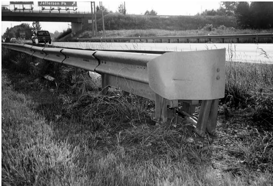
Figure 8-14. Brakemaster® 350
