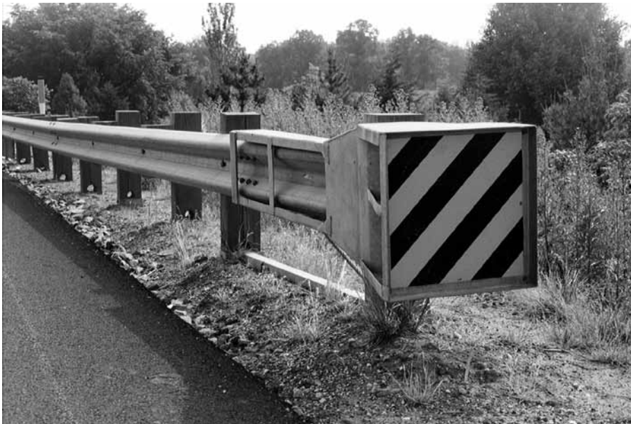
Figure 8-13. Sequential Kinking Terminal (SKT-350™)
