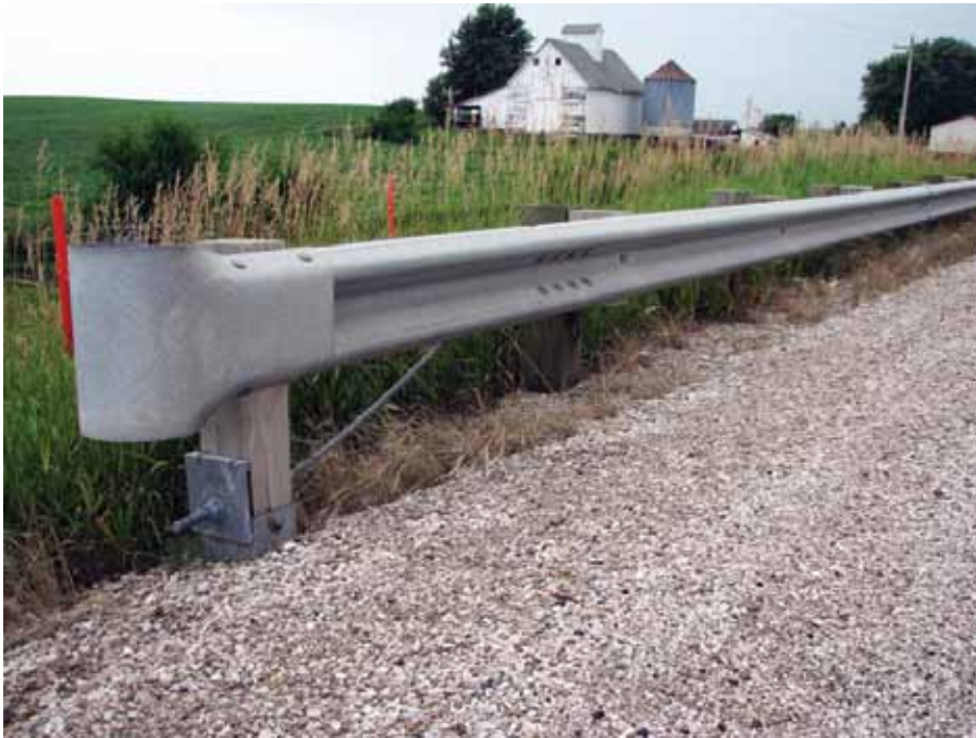
Figure 8-1. Trailing End W-Beam Guardrail Anchorage
