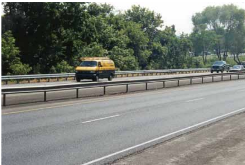
Figure 6-2. Weak-Post W-Beam Median Barrier
