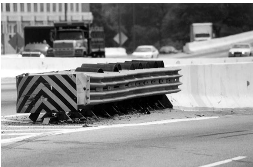
Figure 8-34. QuadGuard Elite
