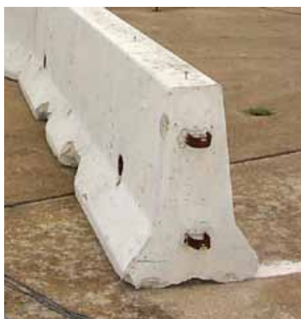
Figure 9-1. Iowa Temporary Concrete Barrier
