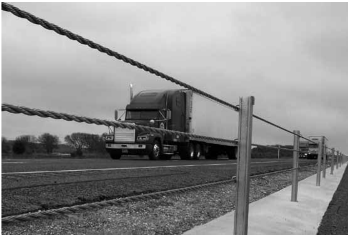
Figure 6-8. Gibraltar Cable Barrier System
