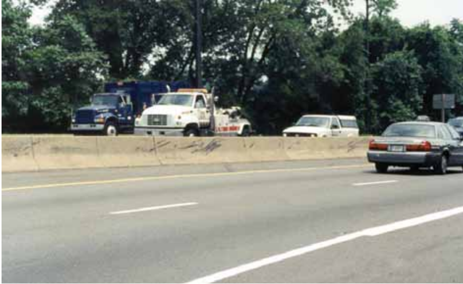
Figure 6-13. Concrete Safety-Shape Median Barrier
