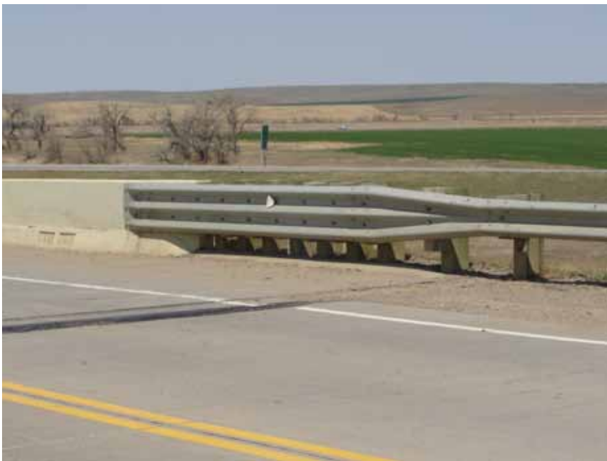
Figure 7-12. Thrie-Beam Transition to Modified Concrete Safety Shape
