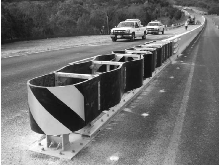
Figure 8-33. Hybrid Energy Absorbing Reusable Terminal (HEART™)
