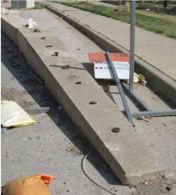
Figure 9-22. Slope-End Treatment for Low-Profile Portable Concrete Barrier
