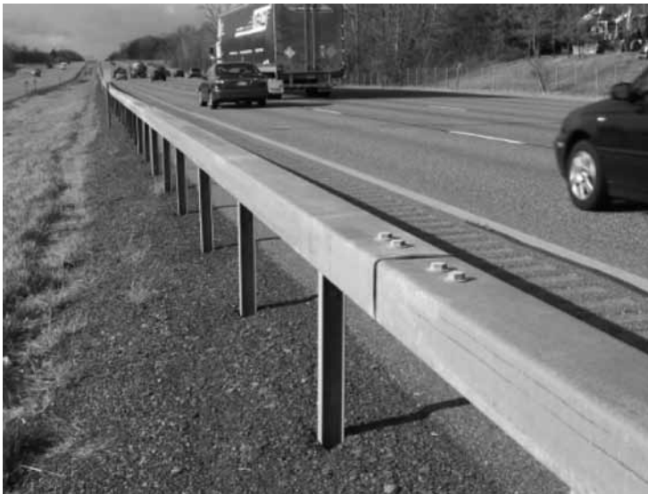
Figure 6-9. Box-Beam Median Barrier
