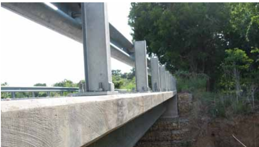
Figure 7-2. Texas T-6 Railing
