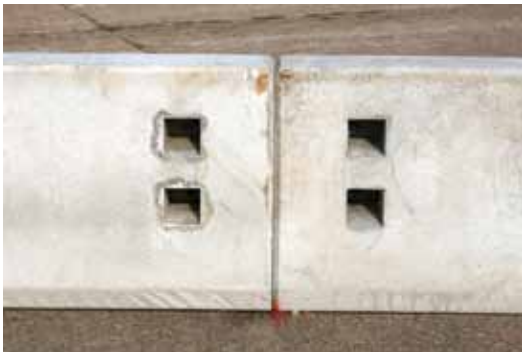
Figure 9-13. Quick-Bolt F-Shaped Concrete Safety Barrier
