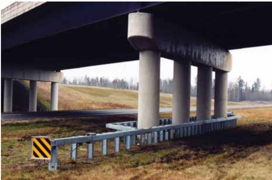
Figure 8-24. Bursting Energy Absorbing Terminal–Bridge Pier (BEAT-BP™) System
