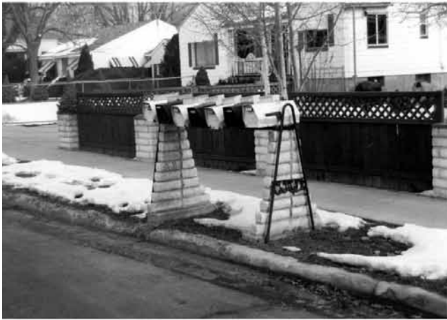
Figure 11-3. Examples of Hazardous Multiple Mailbox Installations
