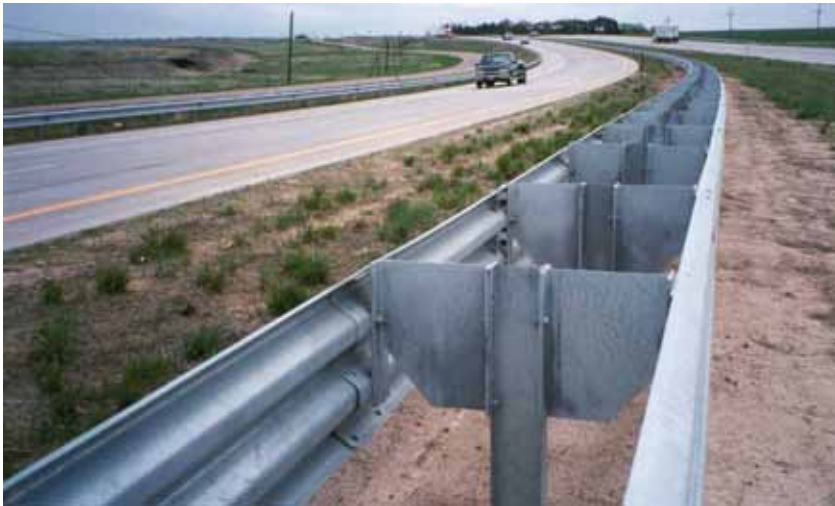
Figure 6-11. Modified Thrie-Beam Median Barrier
