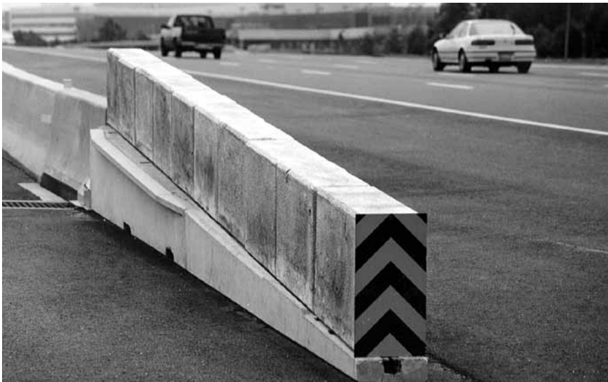
Figure 8-22. Advanced Dynamic Impact Extension Module (ADIEM™)
