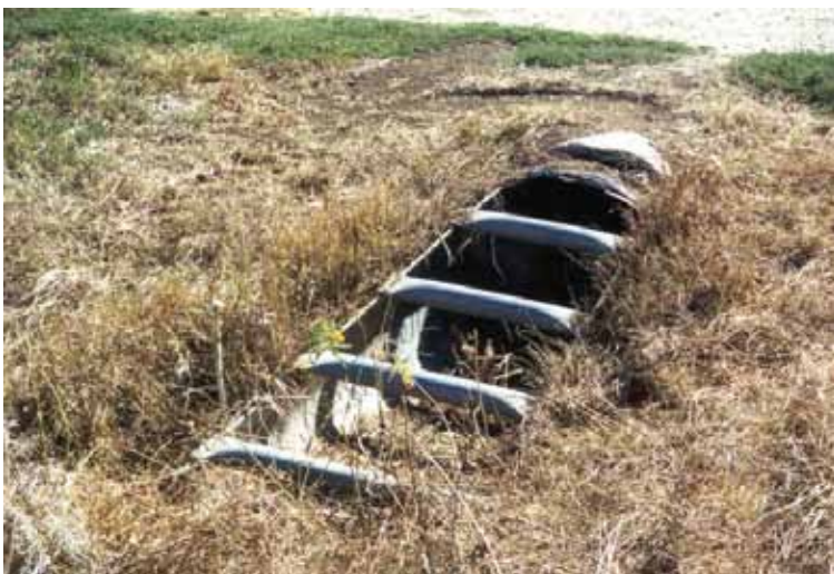
Figure 3-12. Safety Treatment for Parallel Drainage Pipe
