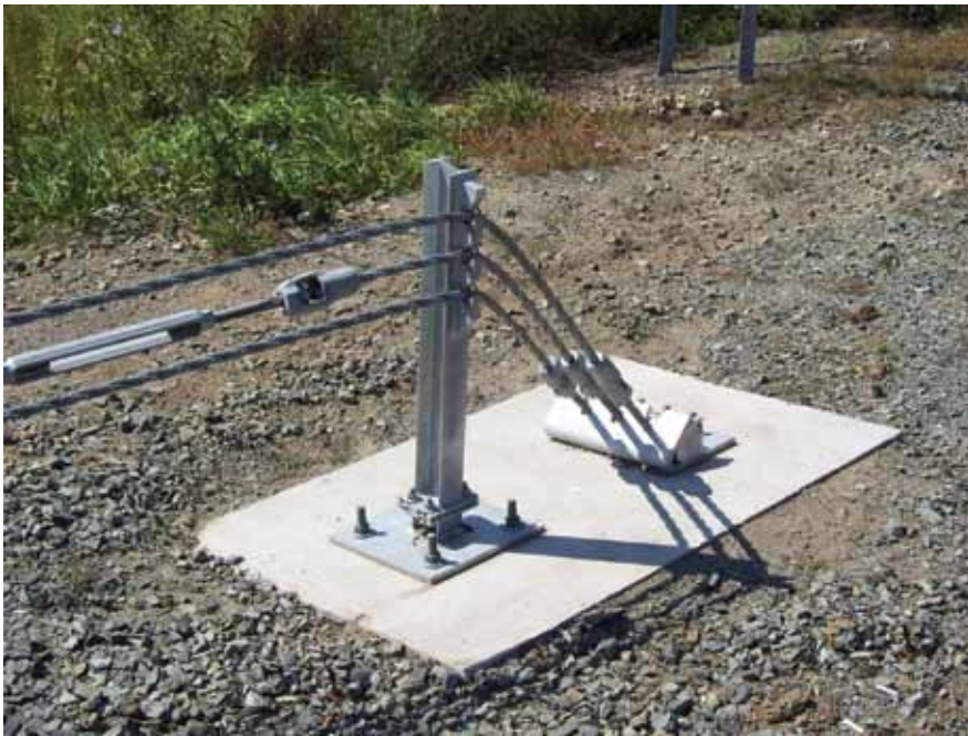
Figure 8-4. Three-Strand Cable Terminal
