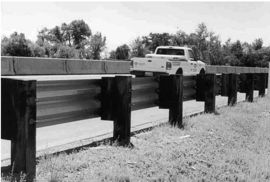
Figure 5-14. Wood-Post Thrie-Beam Guardrail
