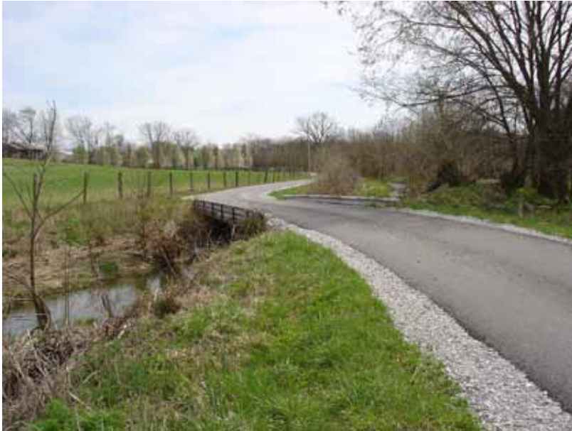
Figure 12-5. Typical Low-Volume Rural Bridge
