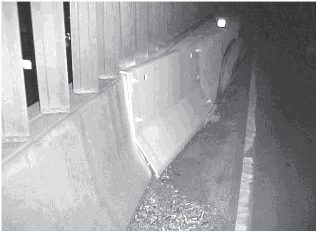
Figure 9-23. Portable Concrete Barrier Steel Plate Transition
