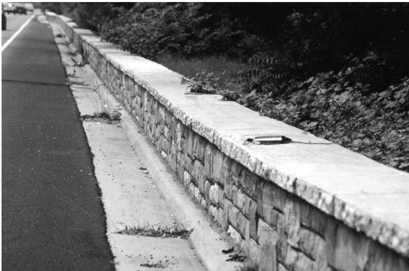
Figure 5-24. Precast Masonry Wall
