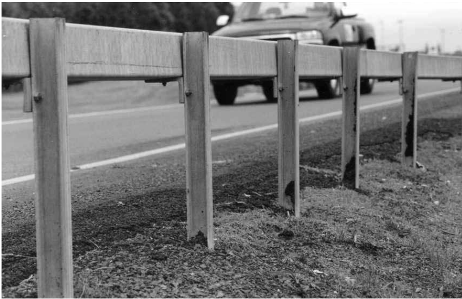
Figure 5-8. Weak-Post Box Beam Guardrail
