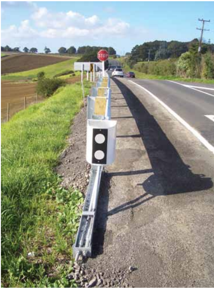
Figure 8-11. X-Tension Guardrail End Terminal
