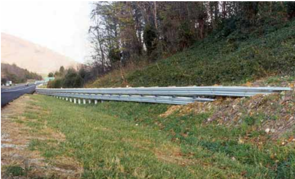
Figure 8-6. W-Beam Guardrail Anchored in Backslope
