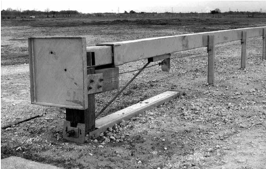
Figure 8-18. Wyoming Box-Beam End Terminal (WY-BET™)
