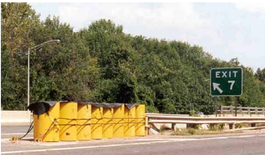
Figure 8-26. Narrow Connecticut Impact Attenuation System (NCIAS)
