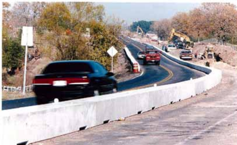
Figure 9-19. Low-Profile Barrier System
