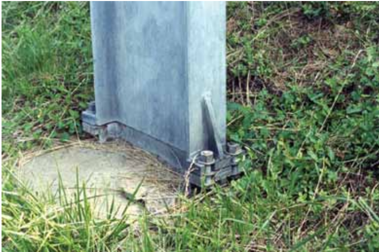
Figure 4-5. Typical Unidirectional Slip Base
