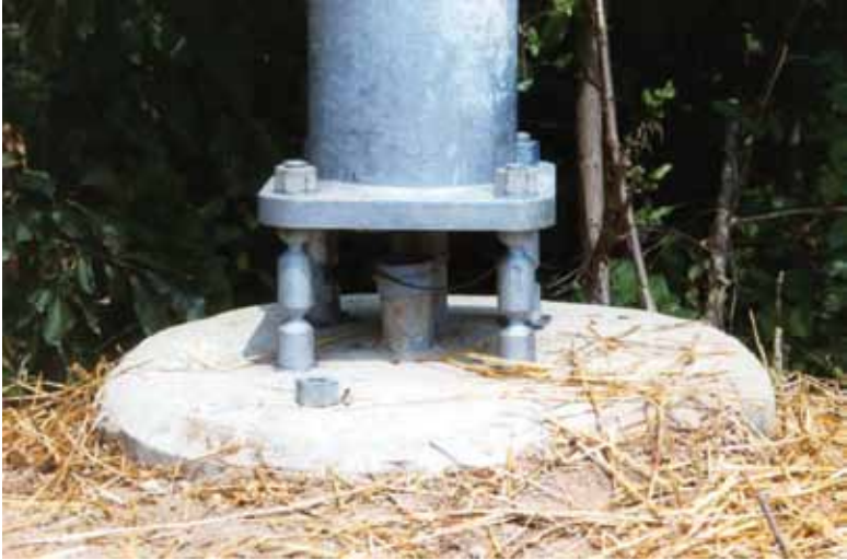
Figure 4-13. Example of a Frangible Coupling Design
