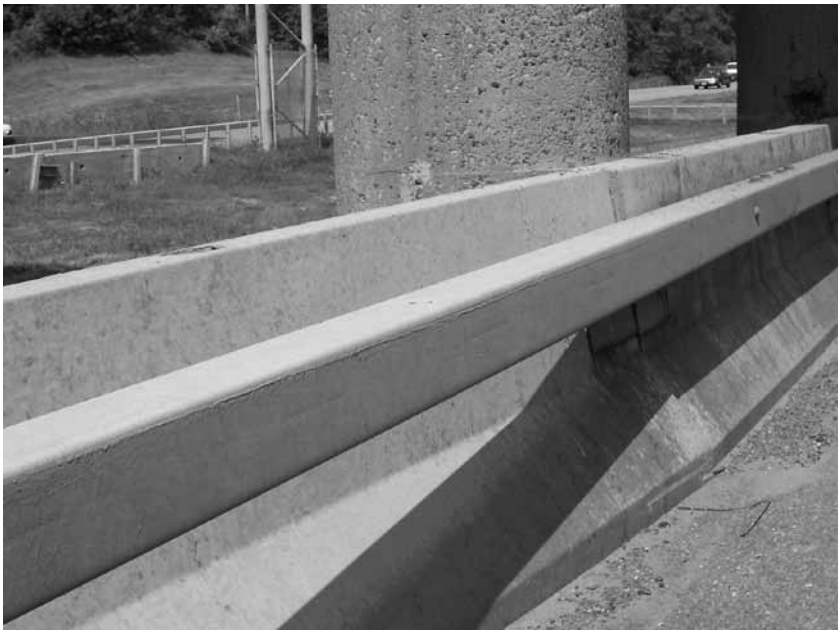
Figure 6-12. New York Modification of Concrete Barrier
