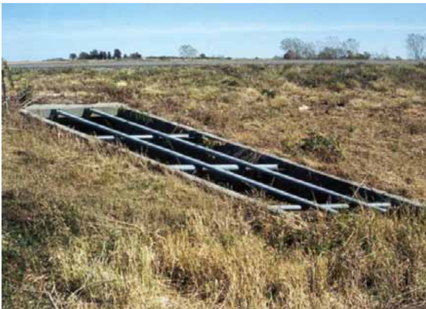
Figure 3-9. Safety Treatment for Cross-Drainage Culvert
