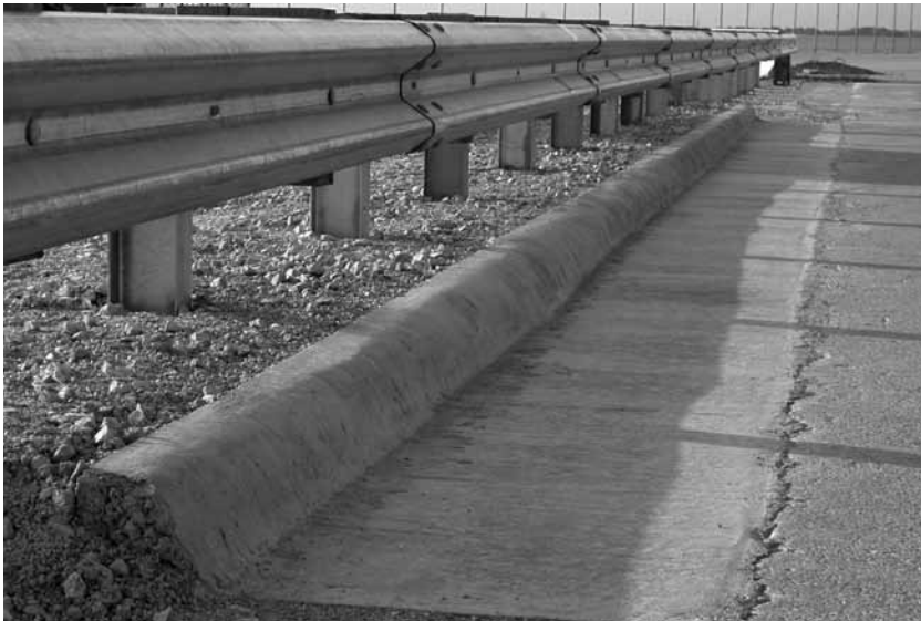
Figure 5-36. MGS Offset from Curb
