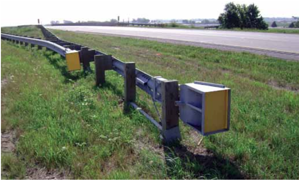
Figure 8-16. FLEAT Median Terminal (FLEAT-MT™)
