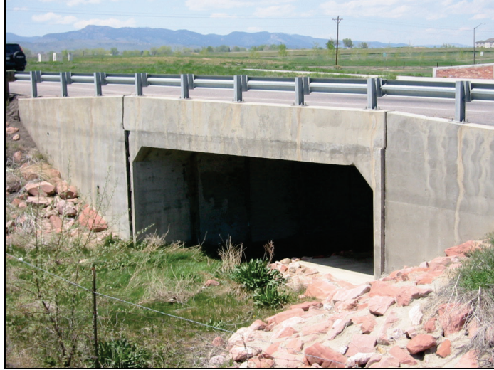
Figure 1.6. Concrete box culvert.
