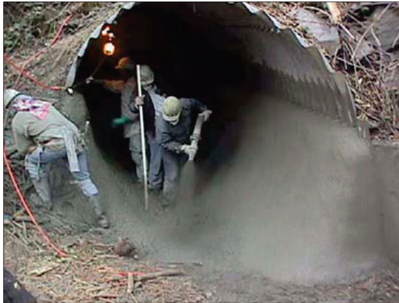
Figure 6.16. Spray-on mortar liner installation via person-entry (from CALTRANS).
