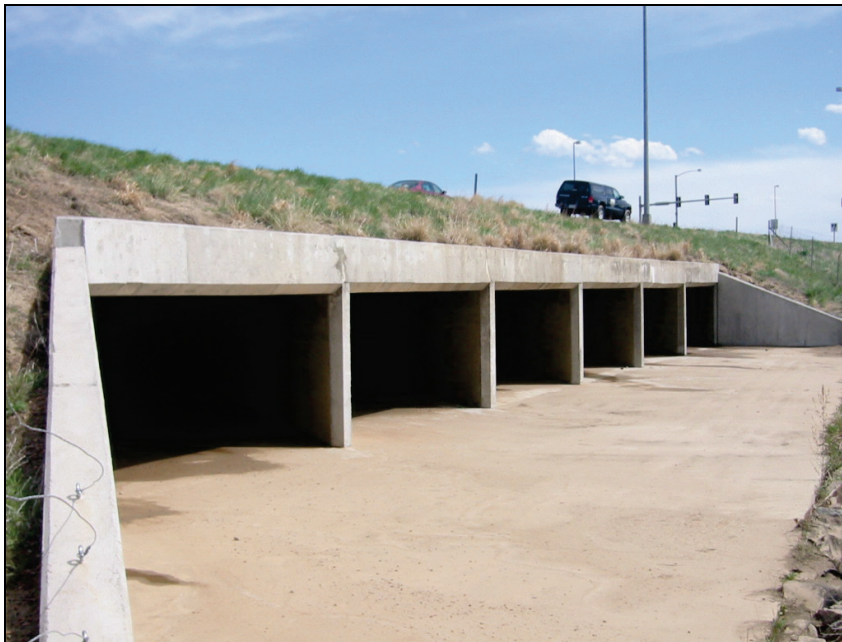
Figure 1.21. Multi-cell box culvert.
