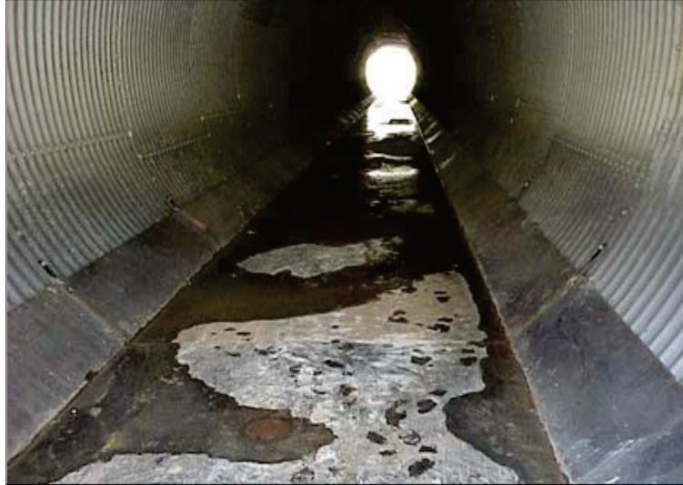
Figure 6.18. Invert repair of CMP using steel plating.
