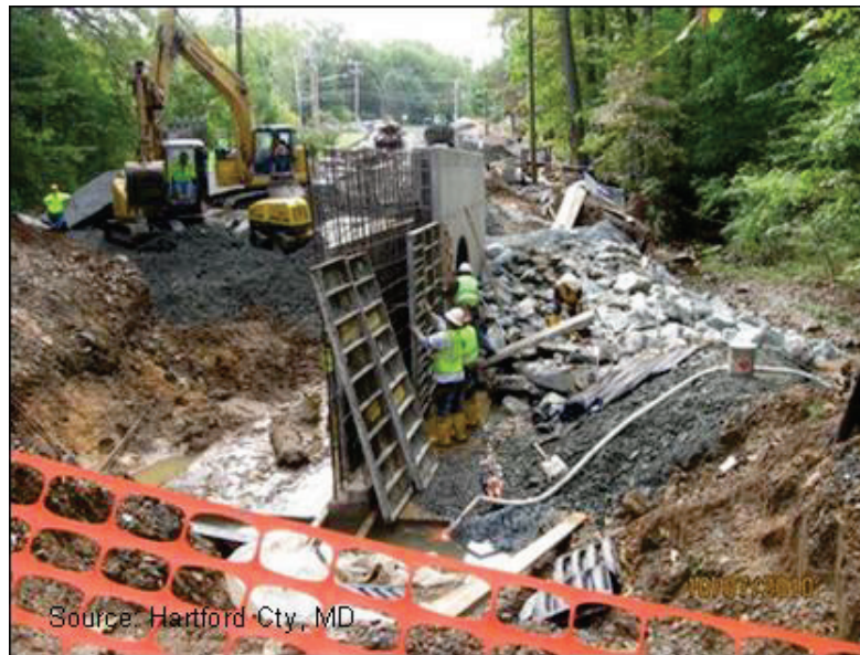
Figure 6.19. Concrete headwall and wingwall installation on pipe culvert.
