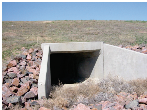
Figure 1.2. Typical concrete box culvert.
