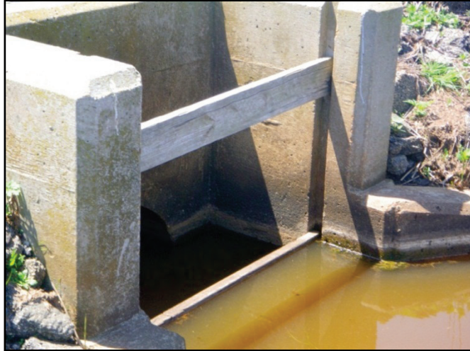
Figure 5.1. Culvert as outflow control device.
