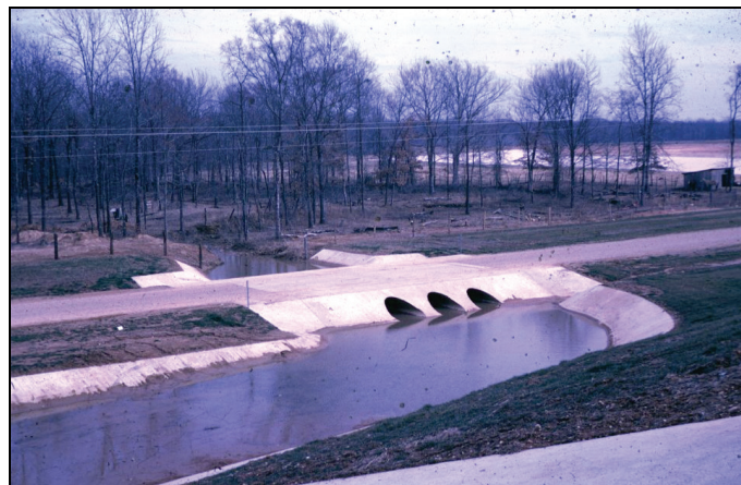
Figure 1.14. Vented low-water crossing.
