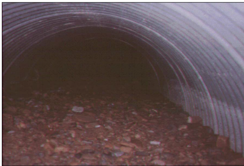
Figure 6.4. Barrel filled with sediment up to half its rise.
