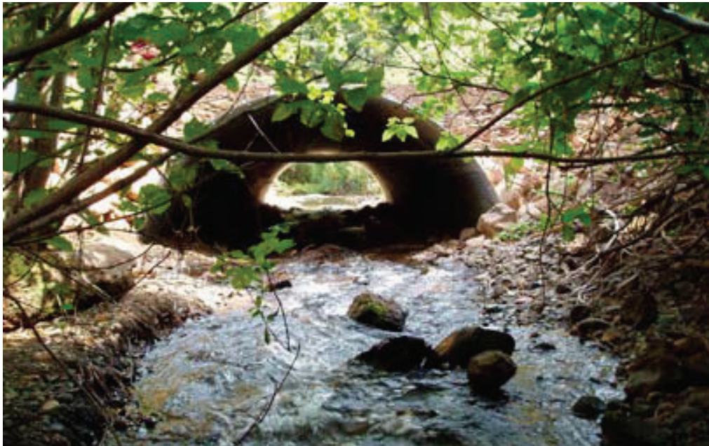
Figure 4.4. Completed open-bottom installation (from USFS 2008).
