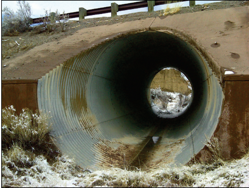
Figure 1.20. Structural plate culvert.
