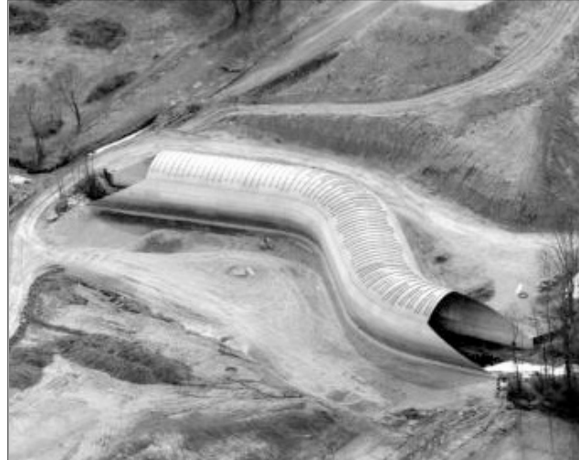
Figure 5.3. Culvert with a horizontal bend (Contech).
