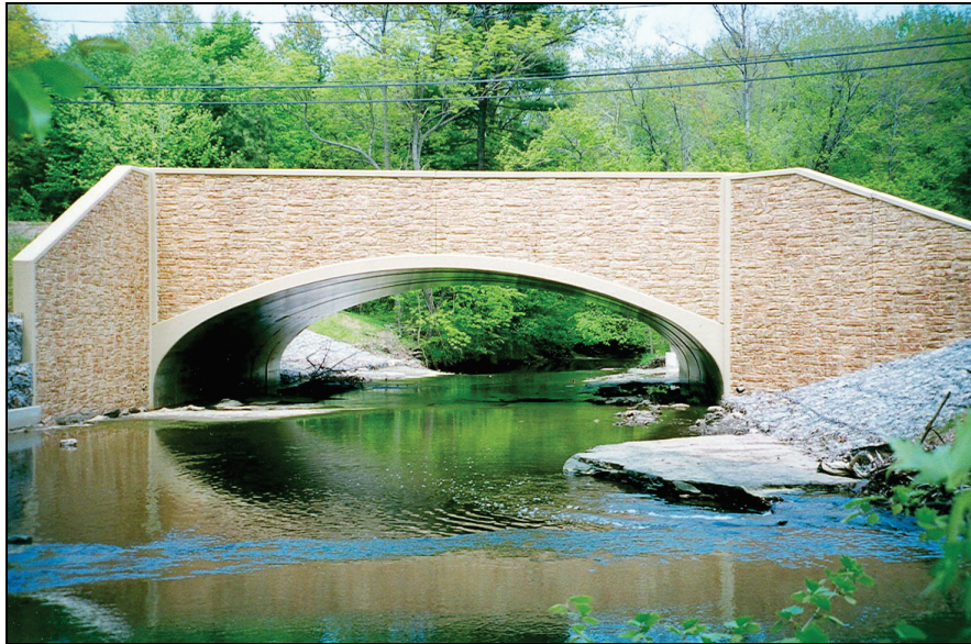
Figure 1.15. Long span culvert.
