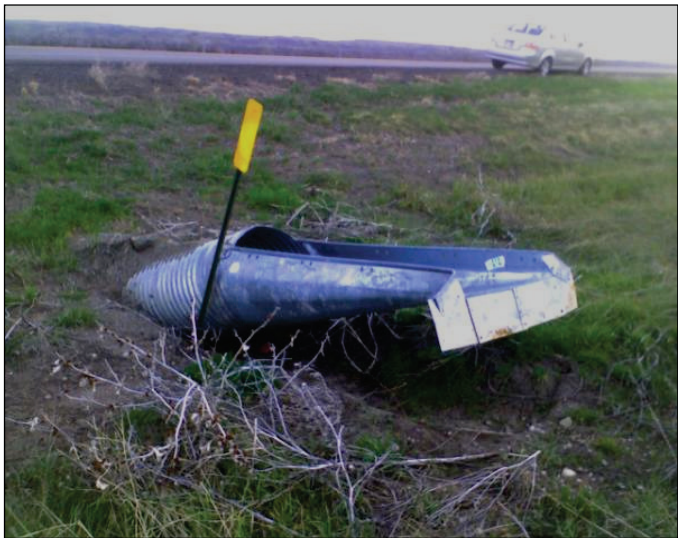
Figure 6.5. Buoyancy uplift.
