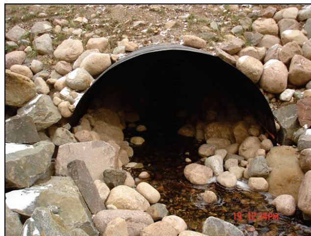
Figure 1.12. Embedded culvert (from WI DOT).
