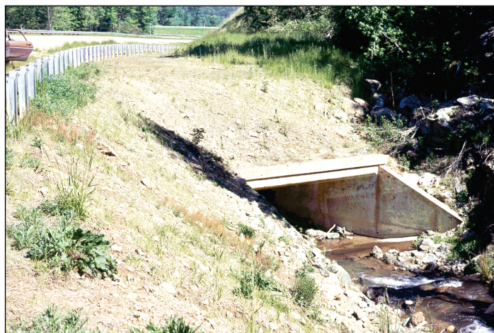
Figure 5.16. Fill warped to avoid inlet skew.
