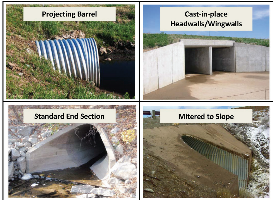
Figure 1.8. Four standard inlet types.
