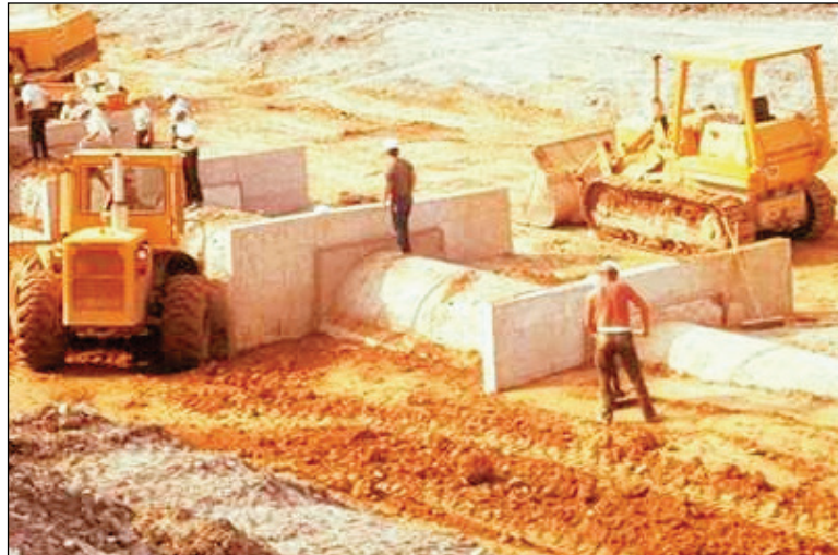
Figure 5.21. Anti-seep collars (FEMA 2005).
