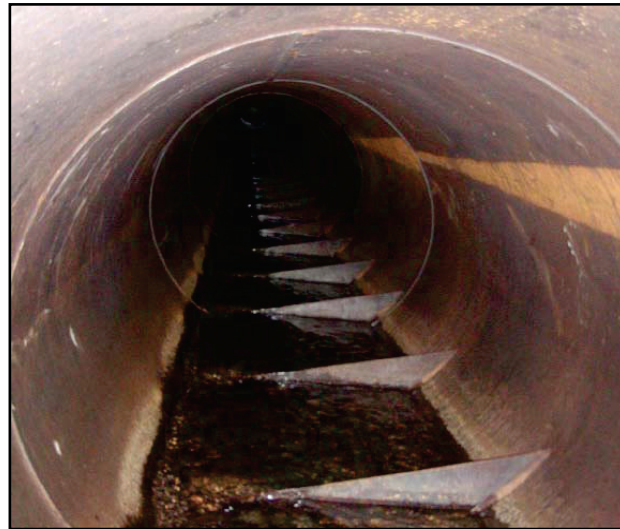
Figure 5.7. Angled baffles (from FishXing Users Manual).
