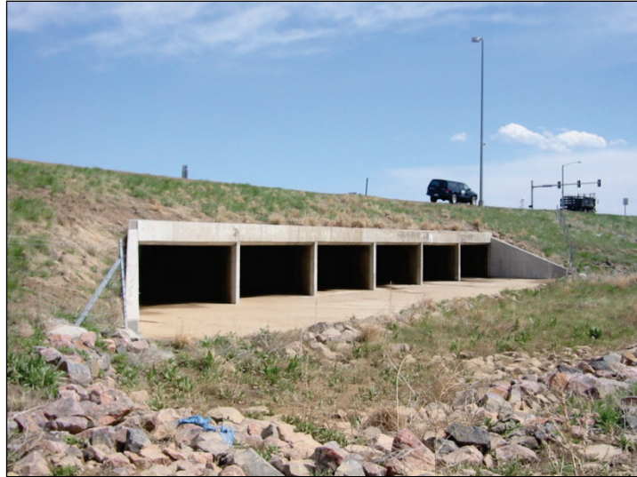
Figure 5.17. Multiple barrel box culvert.
