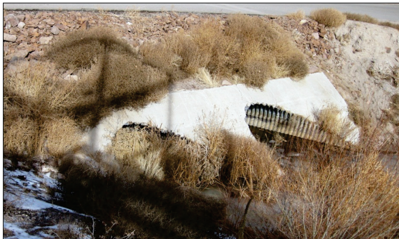
Figure 5.20. Slope paving around a mitered inlet.
