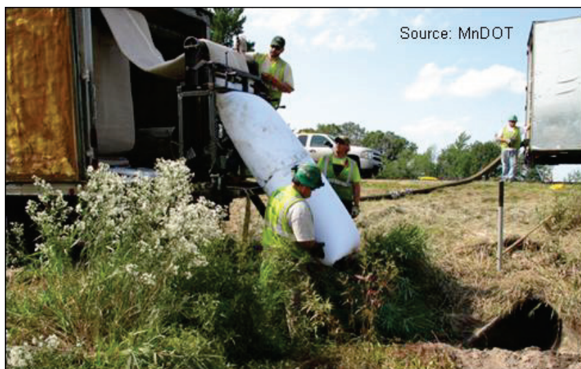
Figure 6.14. Cured-in-place liner installation.
