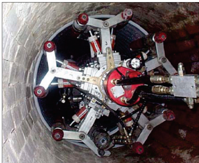
Figure 6.13. Close-fit spiral wound liner installation in a masonry pipe.
