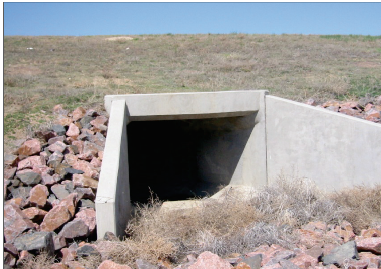
Figure 5.9. Inlet protection based on headwall, wingwalls and riprap.
