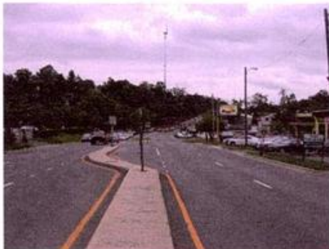
(a) Divided Suburban Multilane Highway Segment
