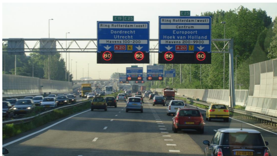
Exhibit 37-5 Variable Speed Limit Signs, Rotterdam, The Netherlands
