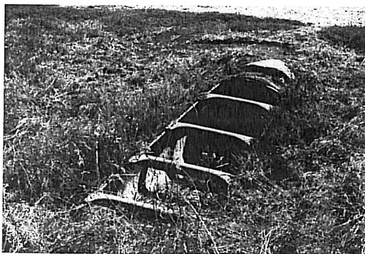
Figure 3-12. Safety Treatment for Parallel Drainage Pipe
