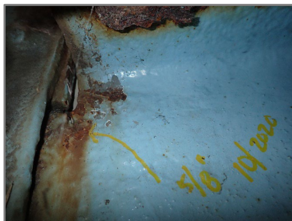
Photo D4 – Floorbeam 9 in Span 2 cracks in the forward top web cope at the Right Truss prior to grinding.
