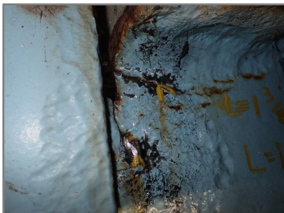
Photo D3 – Floorbeam 0 in Span 2 top 1 3/8" long crack in the rear top web cope at the Left Truss after grinding and magnetic particle testing.
