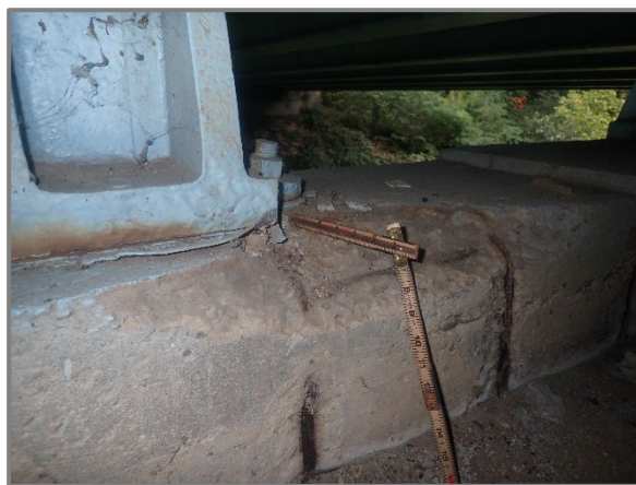
Photo 43 – Corner spall 24" wide by 3" high by 7" deep between Beams 7 and 8 on the forward face of the beam seat of the Pier 1 cap that undermines the Beam 7 bearing up to 1", looking northwest.
