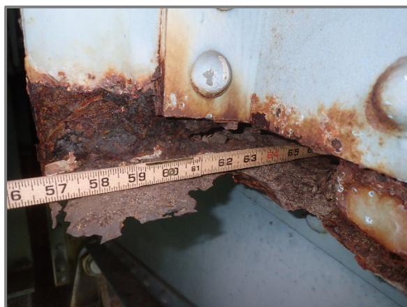
Photo 17 – Advanced section loss to Sidewalk Stringer 1 at Floorbeam 9 in Span 2 with 6" long by 2" wide corrosion hole in bottom flange and 10" long by 1" high corrosion hole in web, looking southeast.
