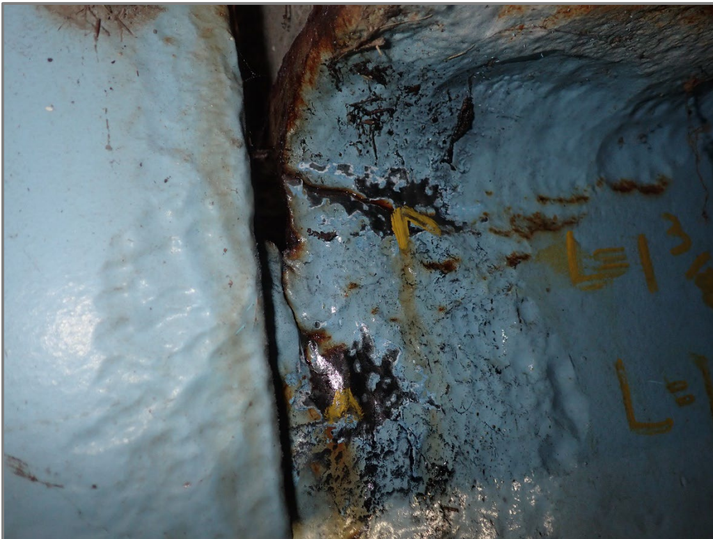
Photo 2 – Cracking in the web of a floorbeam at the upper cope (looking east at Floorbeam 0 in Span 2 adjacent to the Left Truss).
