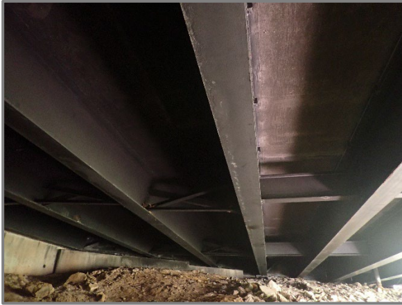
Photo 14 – Heavy soot staining on Beams 1 through 5 in Span 4 due to fire event, looking east.
