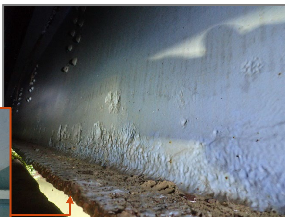
Photo 31 – Up to 1/4" deep pitting over 12' long by 6" high area on Floorbeam 0 in Span 2 rear web near Right Truss with up to 1/4" deep pitting over 2" width on the flange underside, looking northeast.
