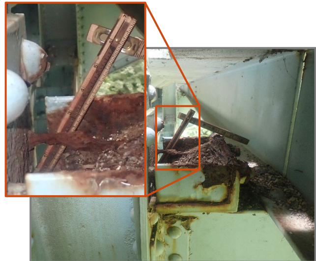
Photo 33 – Up to 95% section loss to the west tie bolt on the Floorbeam 8 cantilever connection to the Left Truss, looking west. Note heavy debris accumulation on top flange of cantilever.
