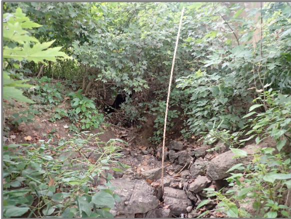
Photo 45 – Erosion gully up to 4' deep by 5' wide by 35' long in the west channel bank approximately 5' from the right column of Pier 1, looking west.
