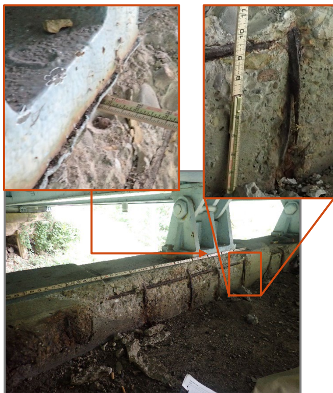
Photo 42 – Spall 68" long by 12" high by 3 3/4" deep with exposed reinforcement and one broken vertical bar between Beams 5 and 6 in Span 2 in Pier 2 beam seat, looking southeast. Note spall undermines Beam 6 bearing up to 3/4".
