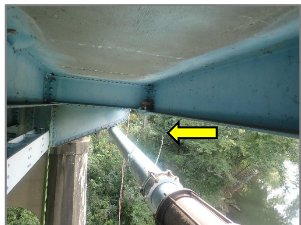
Photo 46 – Broken wire hanger for water main between Panel Points 7 and 8 on the right side of the truss, looking east.
