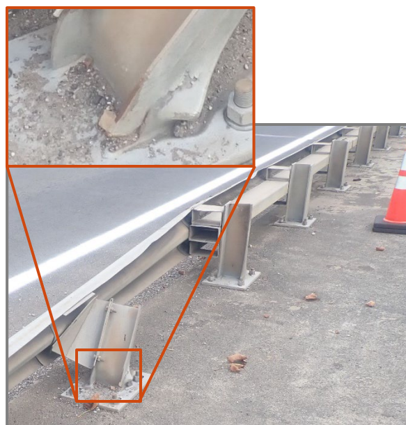
Photo 7 – Collision damage to first two posts of the right bridge rail at the rear end in Span 1, looking northeast. Note posts with tears at bases and rotated/twisted.
