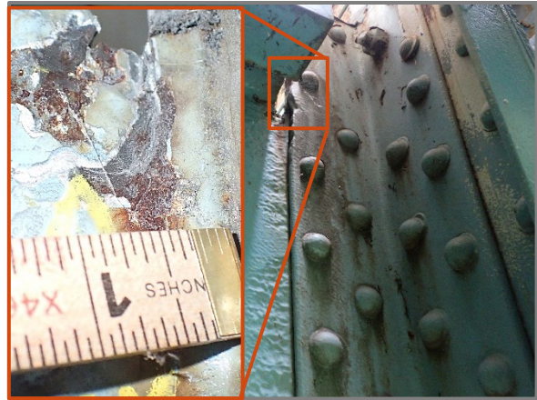
Photo 28 – 1\frac{3}{8} " long diagonal crack in the web cope of Floorbeam 9 in Span 2 at Left Truss with \frac{1}{8} " propagation since previous inspection, looking west.
