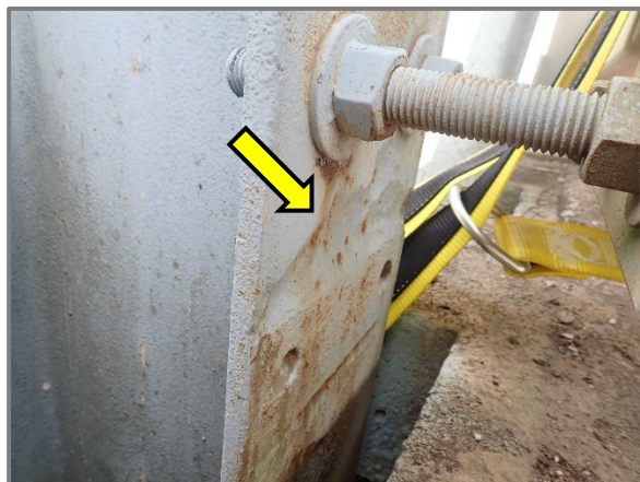
Photo 25 – Up to 1/4" deep pitting to the exterior of the inboard flange of L4-U4 on the Left Truss at previous guardrail connection, looking northeast.
