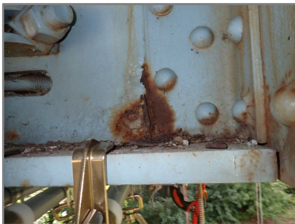
Photo 30 – Up to 3/16" deep pitting over 5" high by 3" wide area of the Floorbeam 4 in Span 2 forward web along bottom flange at the Left Truss that is beginning to reactivate, looking west.
