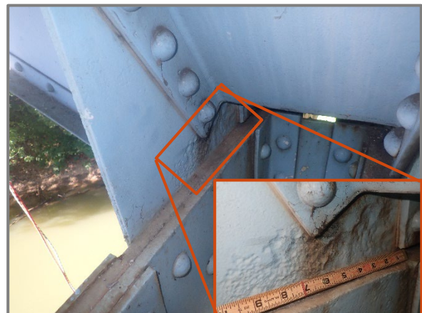
Photo 34 – Cleaned and painted pitting up to 3/16" deep over 10" long by 4" high area on interior of L5 outboard gusset plate along L5-L6 on the Right Truss, looking southwest.
