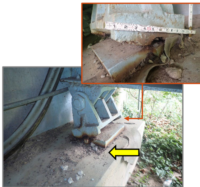
Photo 35 – Excessive expansion tilt of rocker bearing of Beam 1 in Span 1 at Rear Abutment, looking northwest. Note displaced lead sheet between masonry plate and cap.
