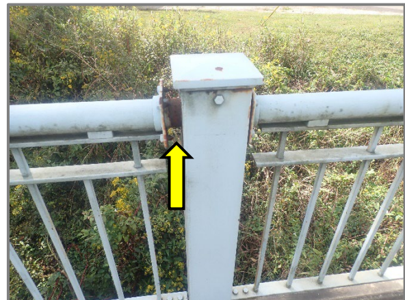
Photo 10 – Top connection plate on the east side of third post from rear end of Span 1 disconnected, looking south.
