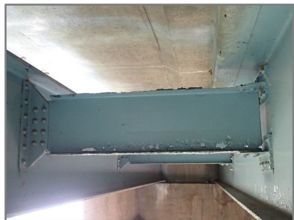
Photo 37 – Advanced section loss and corrosion holes in the diaphragm between Beams 7 and 8 in Span 4 near midspan, looking west.
