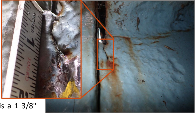
Photo 27 – 1\frac{3}{4} " long vertical crack in the web cope of Floorbeam 0 in Span 2 at Left Truss with \frac{1}{4} " propagation since previous inspection, looking east.
