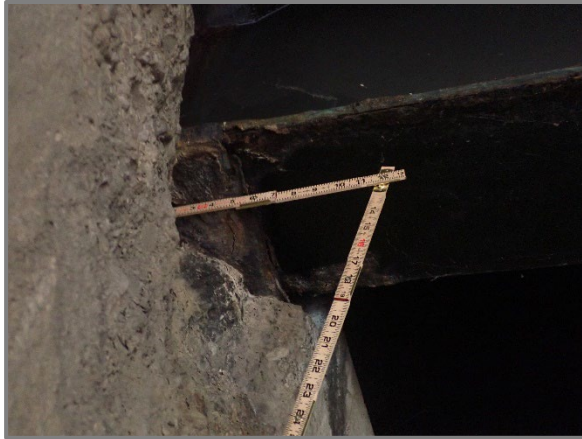
Photo 40 – Spall 15" high by 24" wide by 6 1/2" deep in the forward beam seat below Beam 4 in Span 4 that has undermined the bearing up to 5 1/2", looking northwest.
