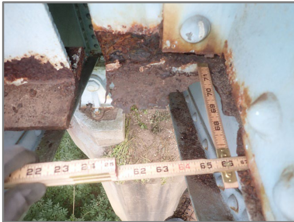
Photo 32 – Advanced section loss to Floorbeam 9 north sidewalk cantilever in Span 2 with 4" long by 1" wide corrosion hole in forward bottom flange, looking south.
