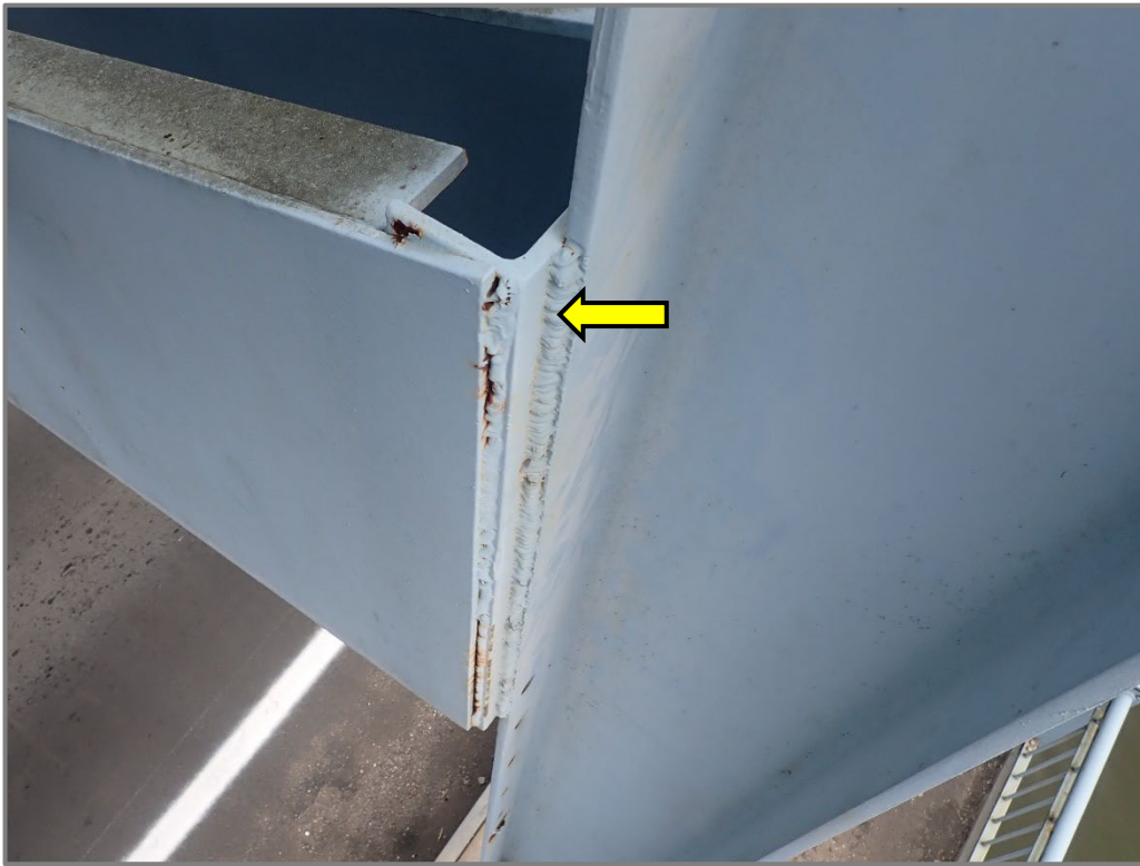
Photo 1 – Sway bracing connection angle attached by fillet welds with no transition radius (Category E). U6-L6 of the Right Truss is shown (looking northeast).
