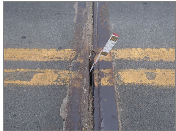
Photo 5 – Expansion joint over Pier 2 with heavy debris accumulation, laminate corrosion, plow damage, and approximately 1' long section of missing joint seal at roadway centerline, looking north.
