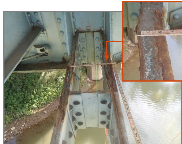
Photo 22 – Up to 1 1/8" thick pack rust between interior and exterior flange plates along top edge on L6-L7 of the Right Truss near L7, looking east.
