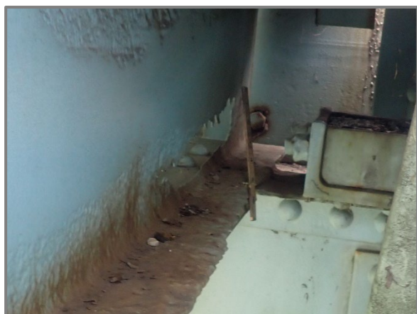
Photo 19 – Advanced section loss to Sidewalk Stringer 3 at Floorbeam 0 in Span 2 with 24" long by 4 1/2" high corrosion hole in web and knife edging to bottom flange, looking west.
