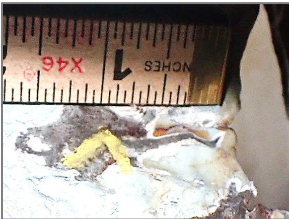
Photo D11 – Floorbeam 9 in Span 2 top 1" long crack in the rear top web cope at the Left Truss after grinding and magnetic particle testing.
