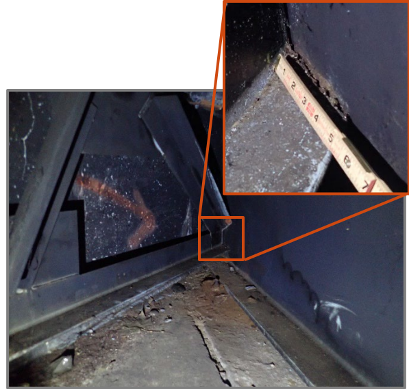
Photo 15 – Broken weld between the north face of the Beam 4 web in Span 4 and the crossframe bottom strut at the Forward Abutment, looking east. Note heavy soot staining on members.
