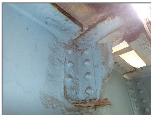
Photo 20 – Advanced section loss and corrosion holes throughout Sidewalk Stringer 3 stub cantilever in Span 3 at Pier 2, looking northeast.
