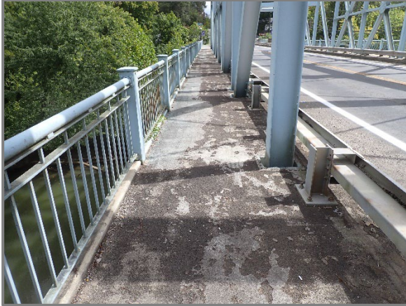
Photo 8 – Typical failing epoxy overlay on the left sidewalk in Span 2, looking east. Note areas of paint loss and minor corrosion on steel pedestrian railing.
