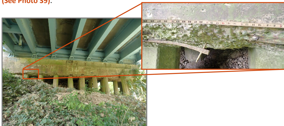
Photo 39 – Pier 3 pile cap with exposed reinforcement on the bottom rear edge due to shallow spalls and lack of cover, looking east. Note broken bar near north end of pile cap.
