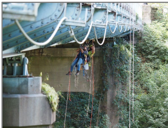
Photo 1 – Rope access inspection of Span 2 truss framing.
