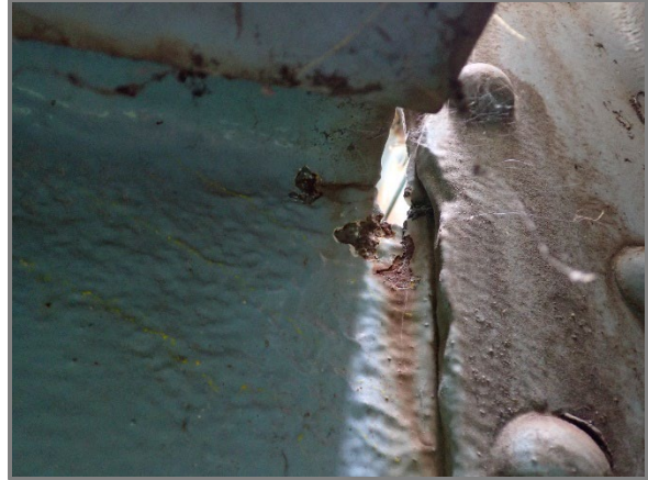
Photo D8 – Floorbeam 9 in Span 2 cracks in forward top web cope at the Left Truss prior to grinding.
