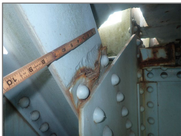
Photo 26 – Up to 3/16" deep pitting to the exterior of the inboard flange of U2-L3 on the Right Truss at the interface with the L3 gusset plate and 100% section loss to the thin fill plate, looking northeast.
