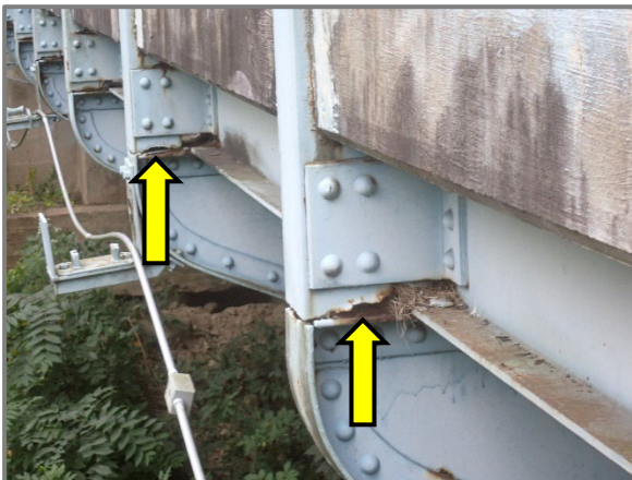
Photo 9 – Corrosion holes at the bases of the right pedestrian railing posts in Span 1, looking northwest.
