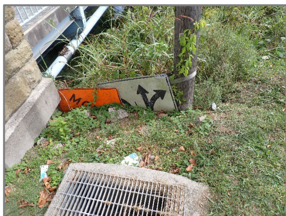
Photo 48 – Makeshift retaining wall consisting of roadway signs and ratchet straps at the southwest corner of bridge, looking east.
