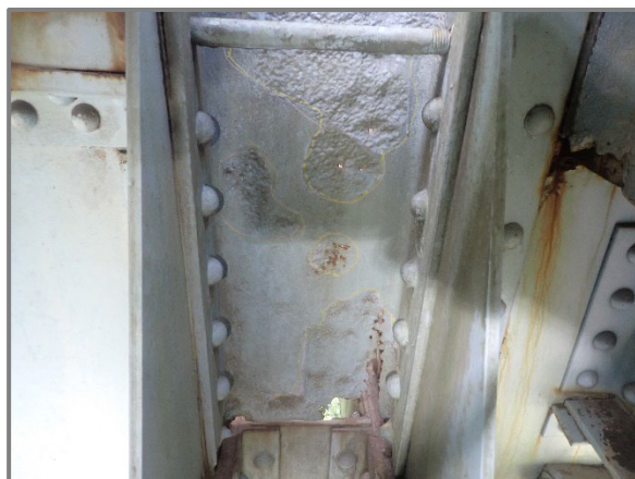
Photo 24 – Advanced section loss to L2-U2 web and flanges on the interior of L2 on Right Truss with isolated corrosion holes in web, looking west.
