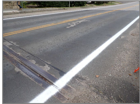
Photo 4 – Up to 6' long by 2' wide area of completely worn wearing surface in the eastbound lane of Span 4, looking northeast.
