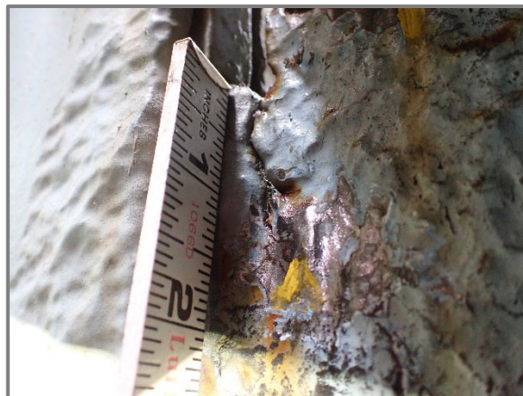
Photo D2 – Floorbeam 0 in Span 2 bottom 1 3/4" long crack in the rear top web cope at the Left Truss after grinding and magnetic particle testing. Note crack has propagated 1/4" since previous inspection.
