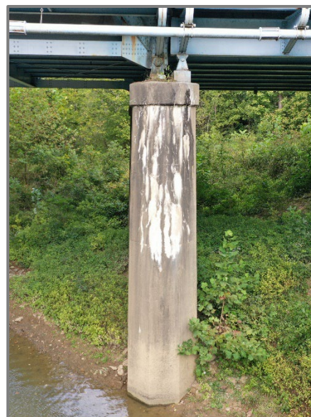
Photo 38 – Hairline cracks with heavy efflorescence on the south face of the south column of Pier 2, looking north.
