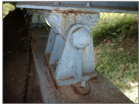
Photo 36 – Freckled pitting up to 1/8" deep throughout the fixed bearing of Beam 7 in Span 3 at Pier 2, looking northeast. Note active corrosion at the base of the casting.
