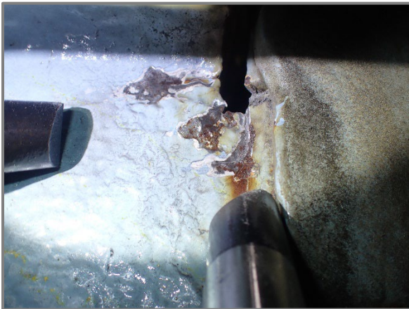
Photo D9 – Floorbeam 9 in Span 2 cracks in the forward top web cope at the Left Truss after grinding and magnetic particle testing.
