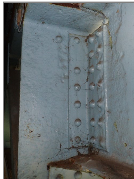
Photo 11 – End 12" of Beam 7 in Span 3 at Pier 2 with 1/8" deep cleaned and painted pitting to both faces of the web and 1/16" deep cleaned and painted pitting to top flange, looking north. Note advanced section loss and corrosion hole in adjacent diaphragm.
