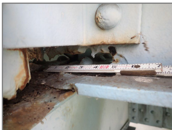
Photo 18 – Advanced section loss to Sidewalk Stringer 4 at Floorbeam 3 in Span 2 with 5" long by 1" high corrosion hole in the web and 80% loss to rivet head on bottom flange, looking north.
