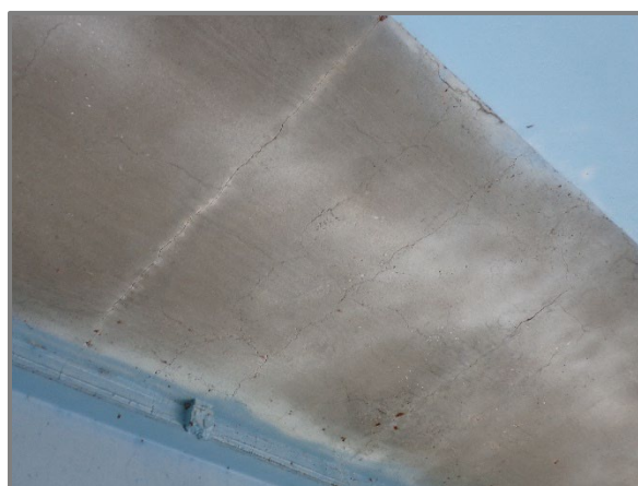
Photo 3 – Hairline to 1/32" wide map cracking spaced at 12" and transverse crack with minor efflorescence in the underside of deck between Stringers 3 and 4 in Bay 3 of Span 2, looking northeast.
