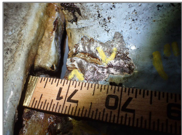
Photo 29 – 1" long and \frac{1}{4} " long cracks in the web cope of Floorbeam 9 in Span 2 at Right Truss, looking west.
