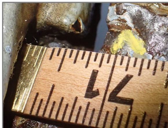
Photo D6 – Floorbeam 9 in Span 2 middle 1/4" long crack in the forward top web cope at the Right Truss after grinding and magnetic particle testing.
