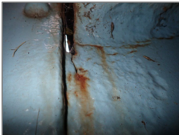
Photo D1 – Floorbeam 0 in Span 2 cracks in the rear top web cope at the Left Truss prior to grinding.
