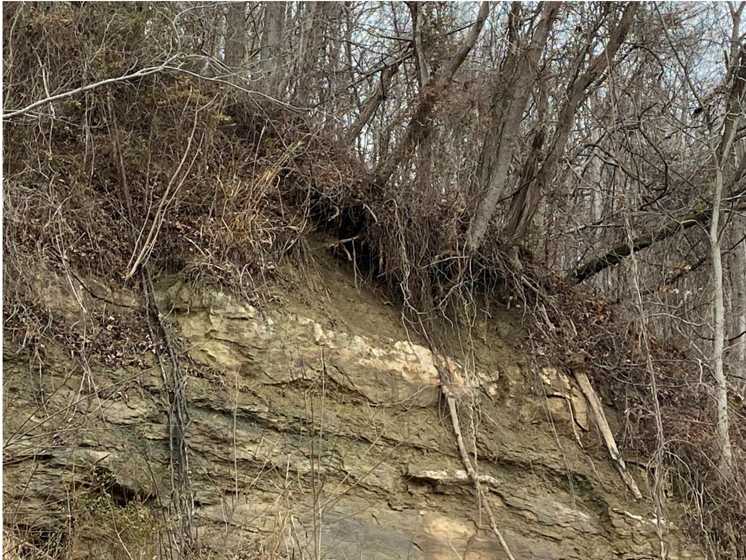
Photograph 3: Photograph of typical rock exposure, and overhanging debris/trees from upper portion from slope within “The Narrows” taken in 2022.
