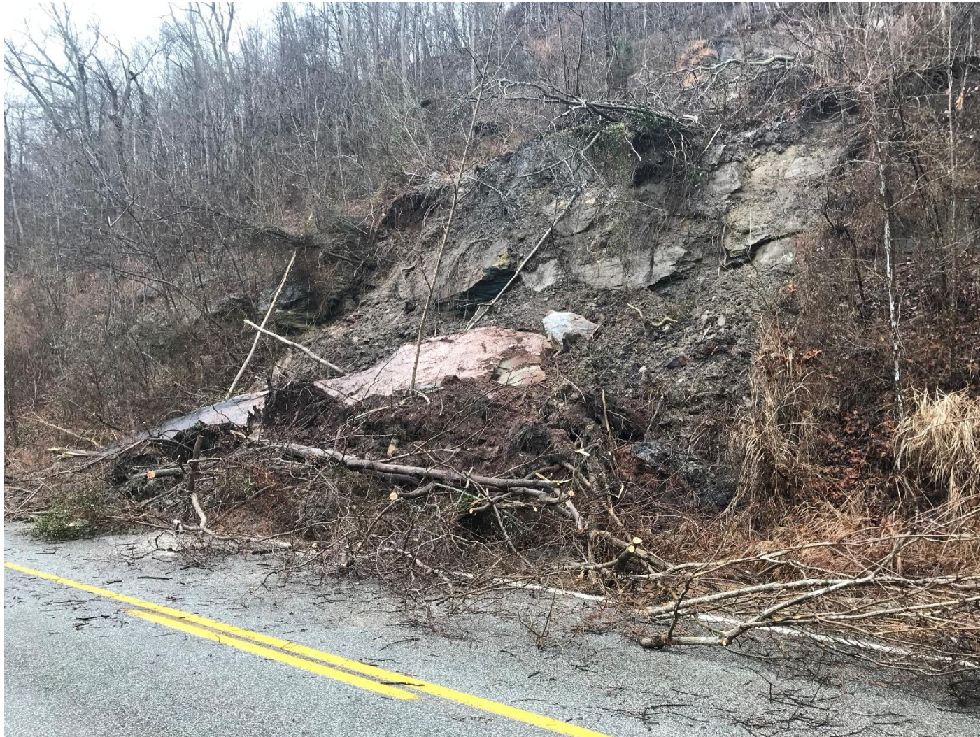
Photograph 5: Historical photograph of debris/rock slide from February 2019 within “The Narrows.”
