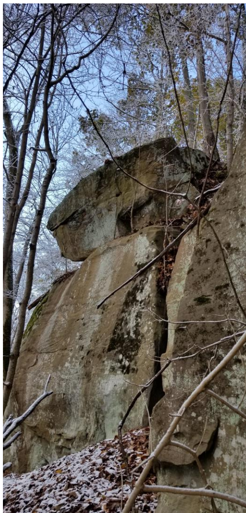
Loose block on top of vertical sandstone block Approx. size 14' wide x 4.5' high x 6' deep
