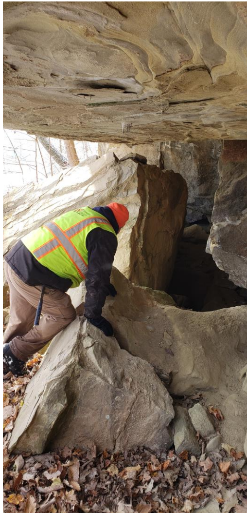
35' wide x 12' high x 18' deep – Rock blocks with overhang above large slab already fallen 8-foot overhang about 7-feet above ground – 4' joint parallel to road
