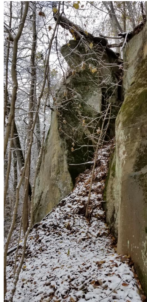
Large jointed block pulling away from slope – 2-foot joint near base, but joint near top is 7-foot wide Total block size is 26' wide x 30' high x 16' deep
