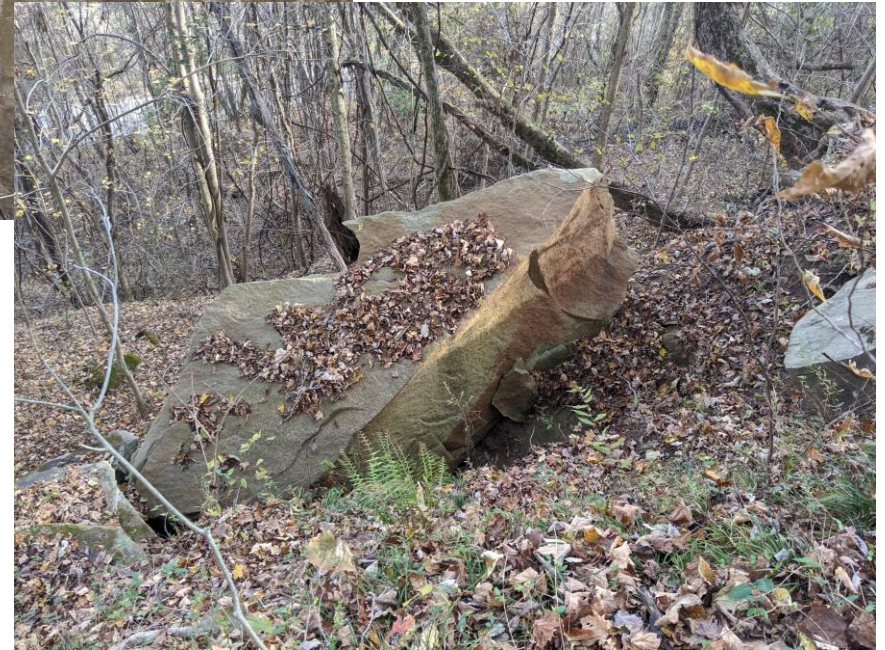
30' wide x 18' high x 13' deep Fragmented boulders that fell backward, kicking front face towards slope edge
