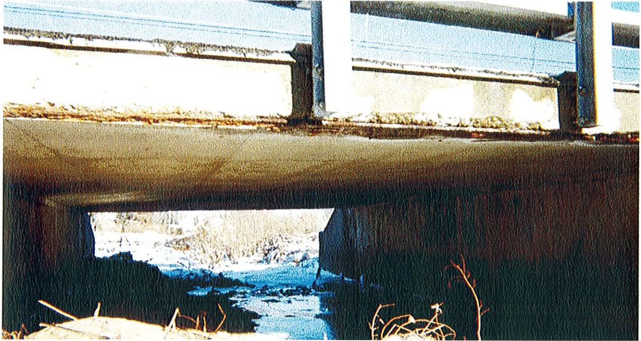
CULVERT ON US 50, EAST OF PROJECT
