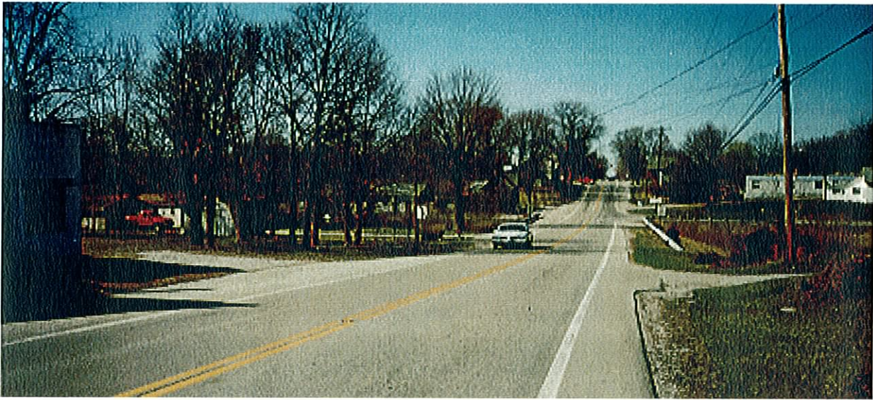
LOOKING WEST ON USR 50 800 FEET FROM INTERSECTION
