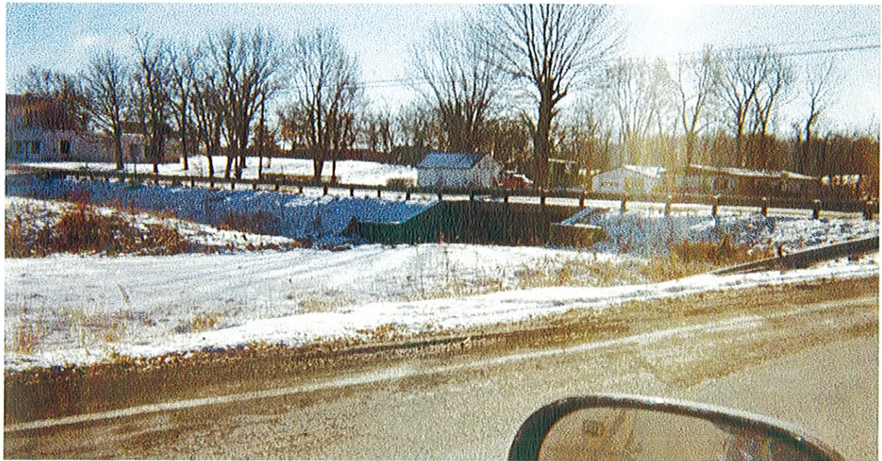
CULVERT ON US 50, EAST OF PROJECT
