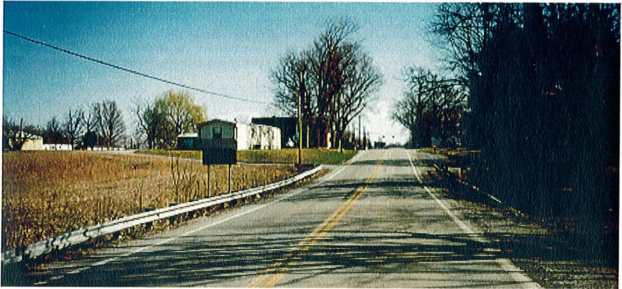
LOOKING EAST ON USR 50 600 FEET FROM INTERSECTION
