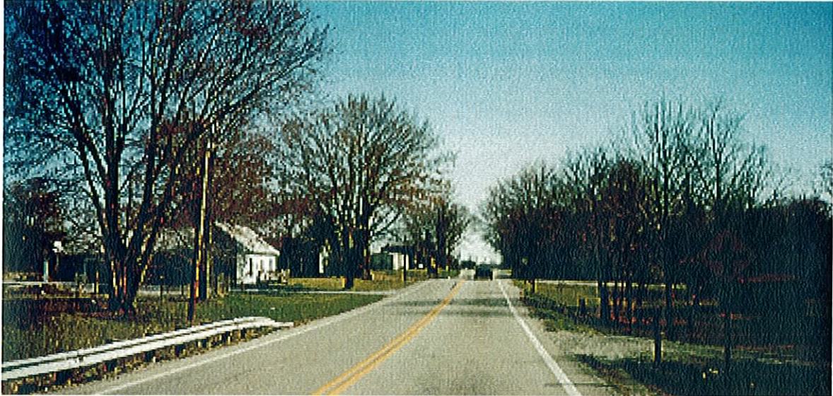
LOOKING EAST ON USR 50 1,000 FEET FROM INTERSECTION
