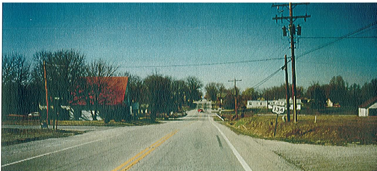
LOOKING WEST ON USR 50 1,000 FEET FROM INTERSECTION
