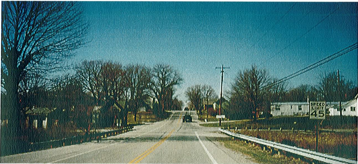
LOOKING WEST ON USR 50 600 FEET FROM INTERSECTION
