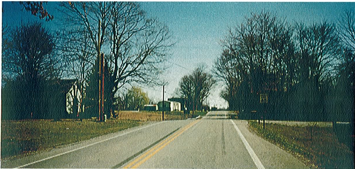
LOOKING EAST ON USR 50 800 FEET FROM INTERSECTION
