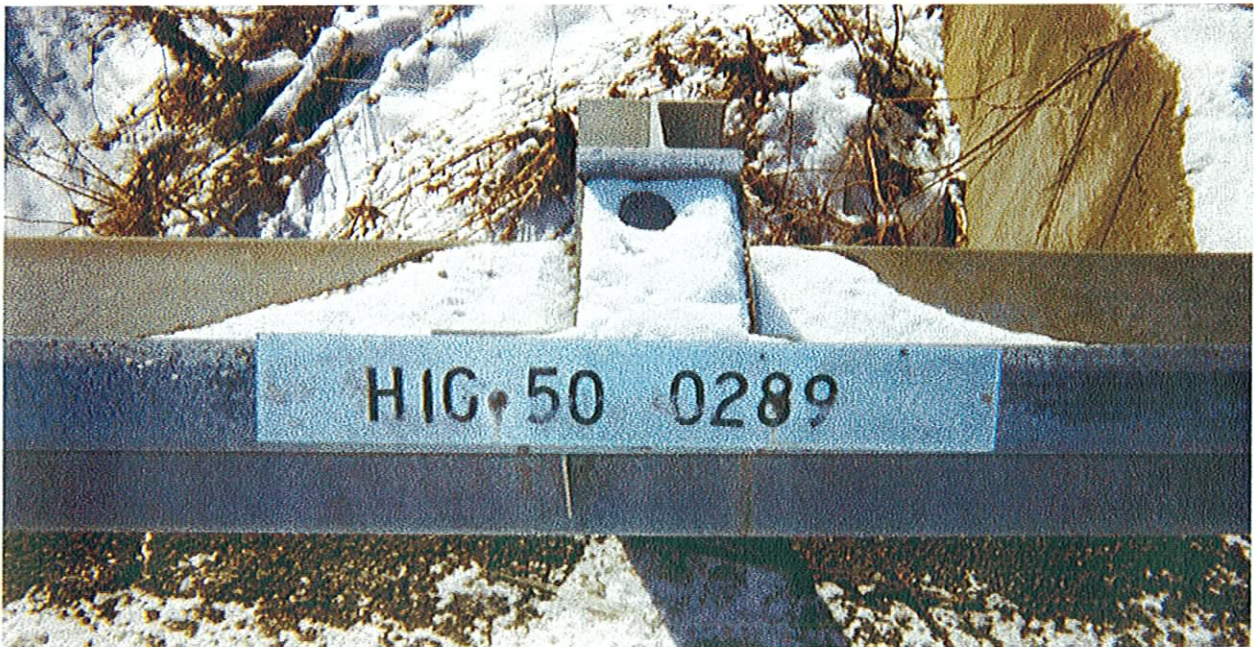
CULVERT ON US 50, EAST OF PROJECT
