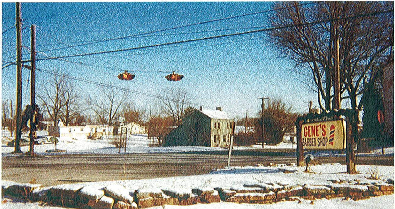
INTERSECTION CONTROL BEACON (WEST INTERSECTION)
