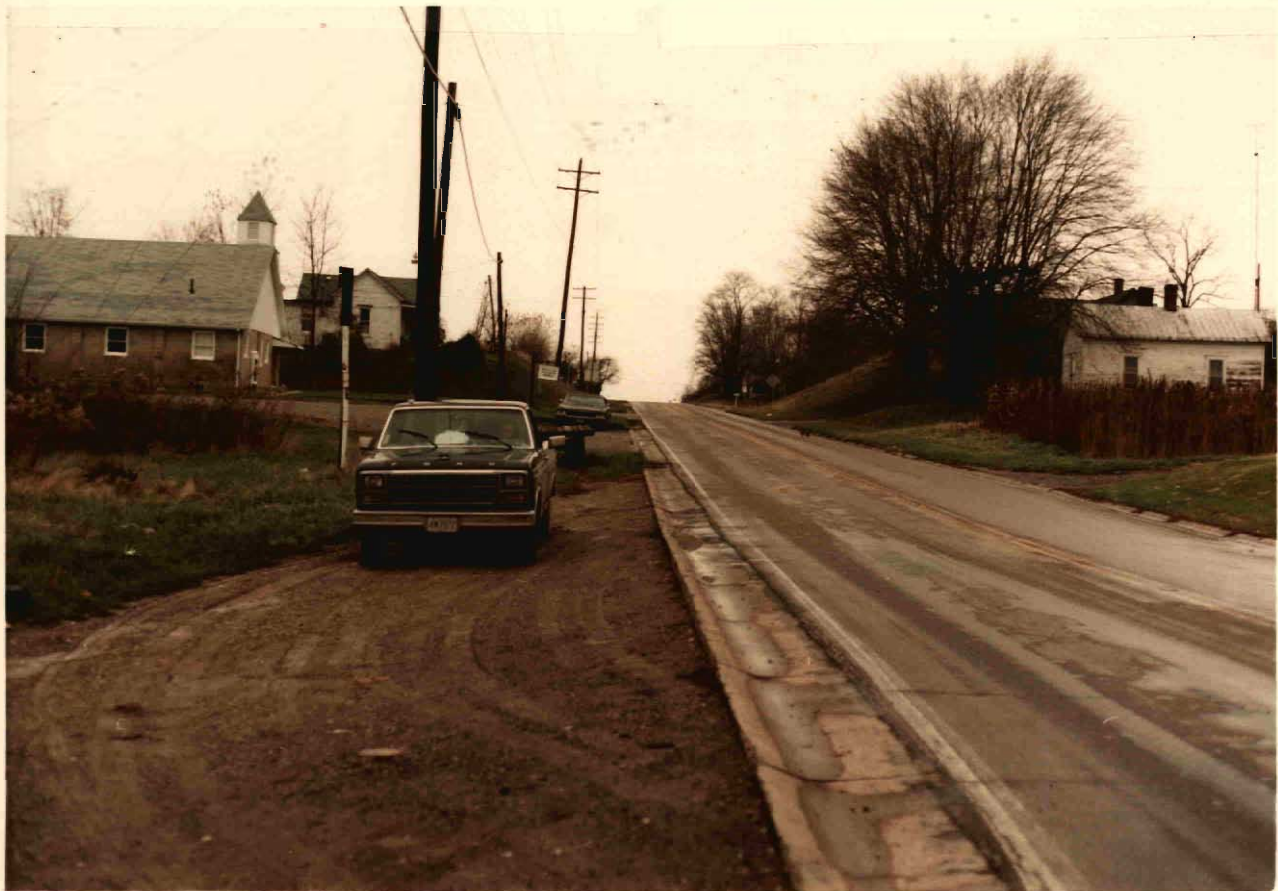
S.R. 327 North of S.R. 124 Looking North
