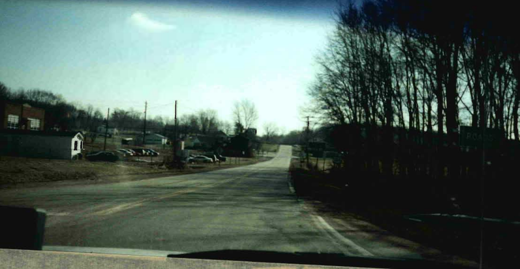
Looking East on S.R. 124 800' from Intersection
