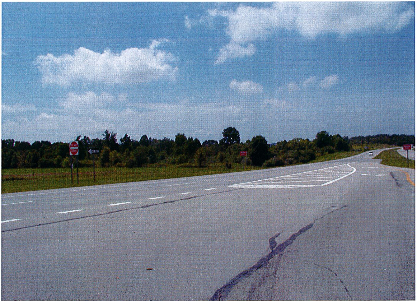
Looking west from median
