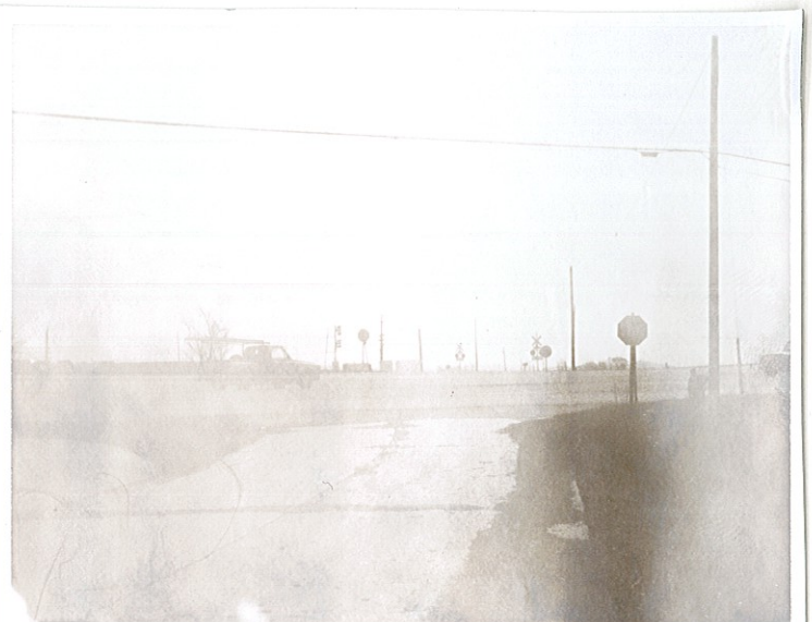
SOUTHERN AVE. LOOKING WB.
